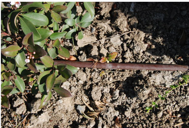
Fig. 1.11 Line source in-line drip irrigation tube for landscape irrigation with the emission point near the middle of the picture
