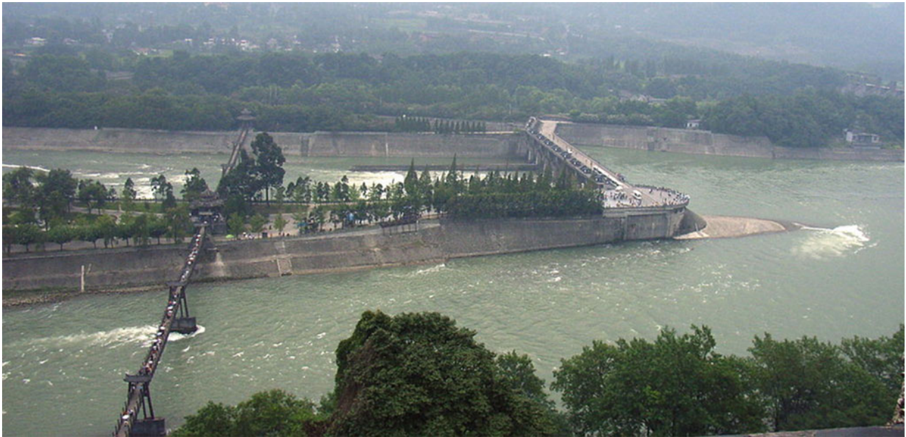
Fig. 1.2 Diversion structure (Dujiang Weir) for Dujiangyan irrigation system. “Dujiang Weir.” (Credit: Huowax at zh.wikipedia)
