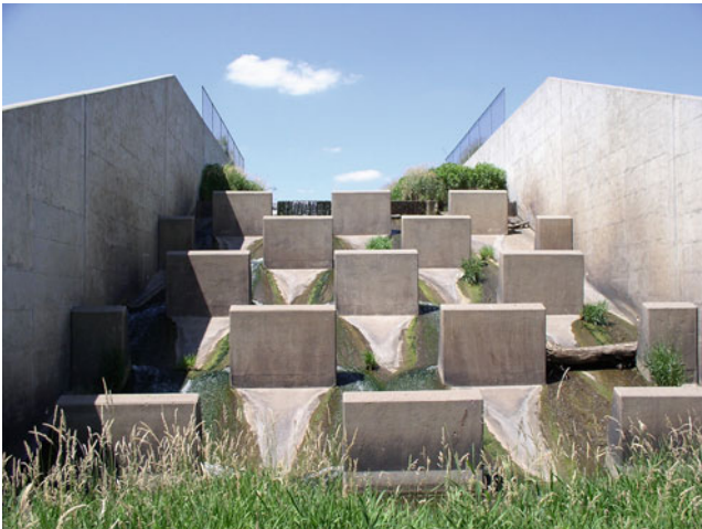
Fig. 11.16 Baffle chute energy drop structure (Wikipedia)
