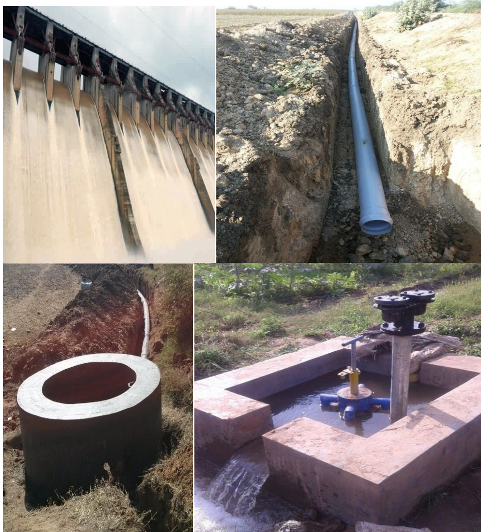
Connecting the Last Mile through Underground Pipelines
