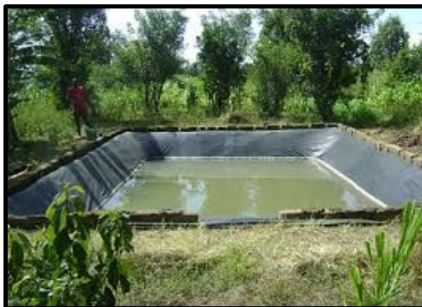
Figure 11.2 Water storage tank
