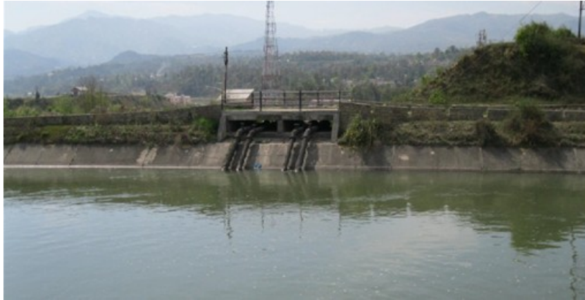
Figure 6.11 Water is drawn from Canal Intake through Syphonic action in Balh Valley Medium Irrigation Project in HP
