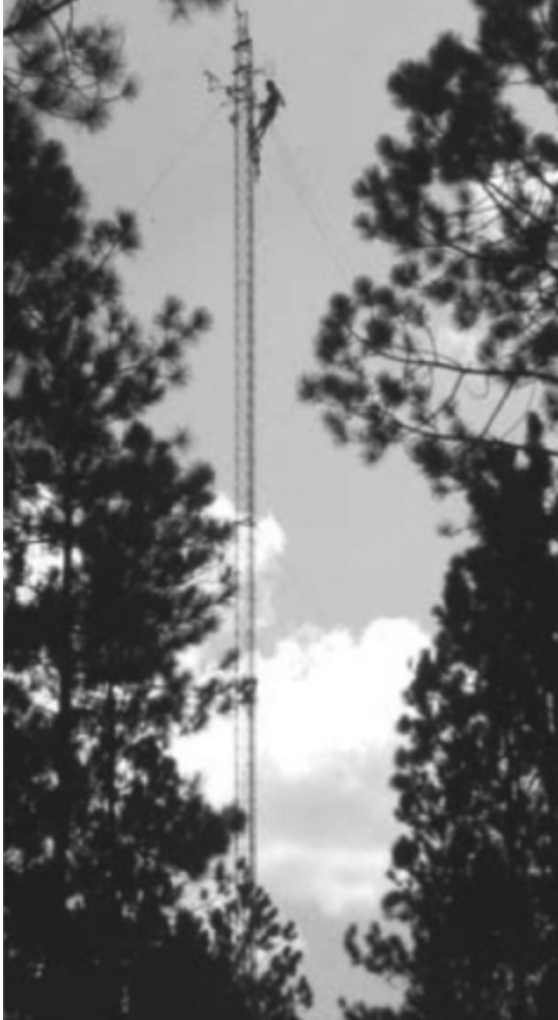
FIGURE 15.6 Evapotranspiration station being serviced by hydrologic technician.
