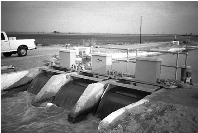
Fig. 2-2. Armtec overshot gates at the Imperial Irrigation District, California, USA, in the early 1990s. The weight of the water pushes the gate down; the cables provide uplift to raise the weir. The gate is hinged at the floor
