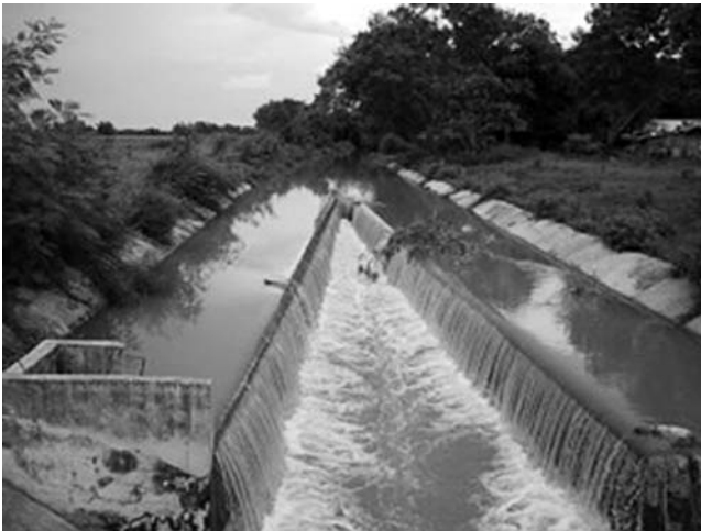
Fig. 2-16. Long-crested weir that lacks silt flushing gates on downstream ends at the Solana Irrigation project in Colombia, South America
