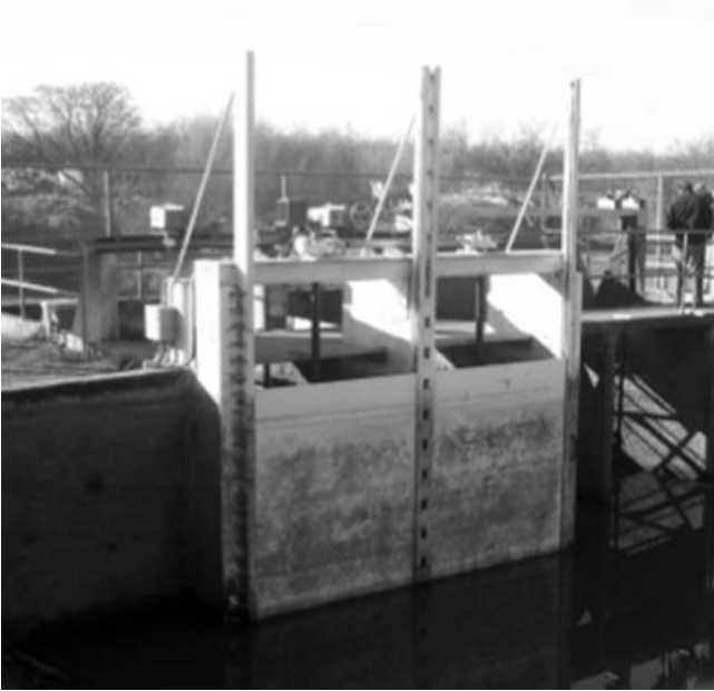
Fig. 2-12. Special configuration of the shaft on a sluice gate (two gates on the left) at Merced Irrigation District, California, USA. The shaft is connected to the bottom of the gate rather than to the top. The shaft is also offset from the gate. This enables the structure to be much shorter than with a typical sluice gate. The motor and actuator are set at a level that makes them serviceable
