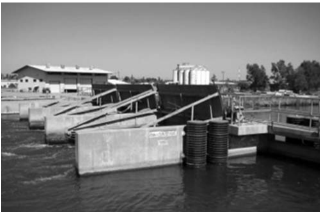
Fig. 2-13. Three radial gates in parallel at Glenn-Colusa Irrigation District, California, USA
