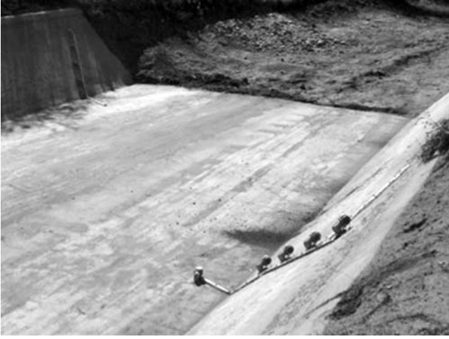
Fig. 2-45. Transit time measurement device; beams are transmitted across the channel
