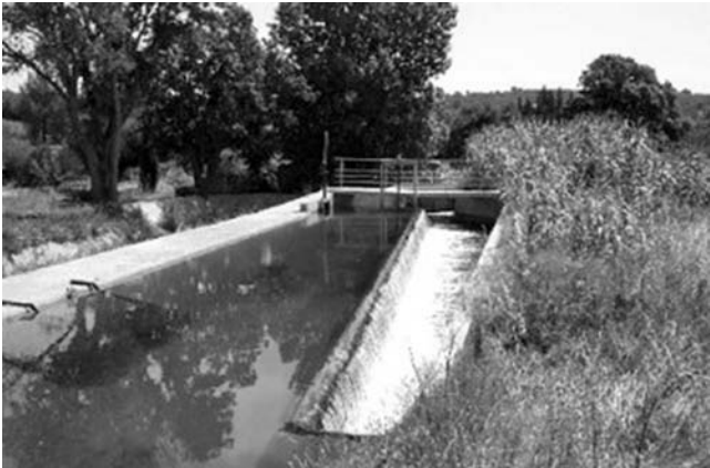
Fig. 2-18. Long-crested weir, ended with a movable sluice gate for sediment and algae flushing at Gignac Canal, France
