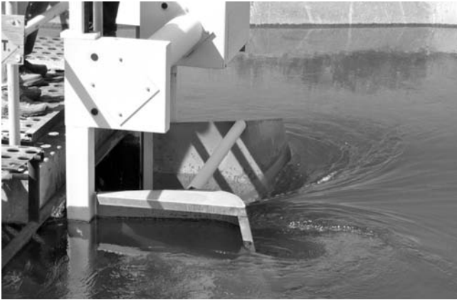
Fig. 2-33. Example of how water can converge at a gate entrance; if the sensor measures the water level at or within the entrance, the depth is quite different from that of the upstream pool. This can be a problem with pre-constructed units that have a water level sensor built into the gate structure
