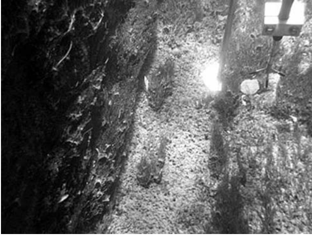
Fig. 2-39. Bryophytes on canal bank and bottom at Gignac Canal, France. Variations of Manning's roughness coefficients reach 30% between spring and summer
