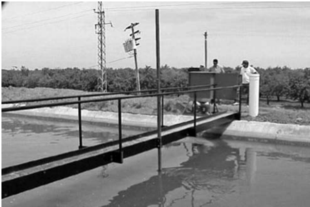
Fig. 2-44. Special section of concrete lining into which an ADVM is placed; the bridge is used for current measurement with a current meter to calibrate the ADVM
