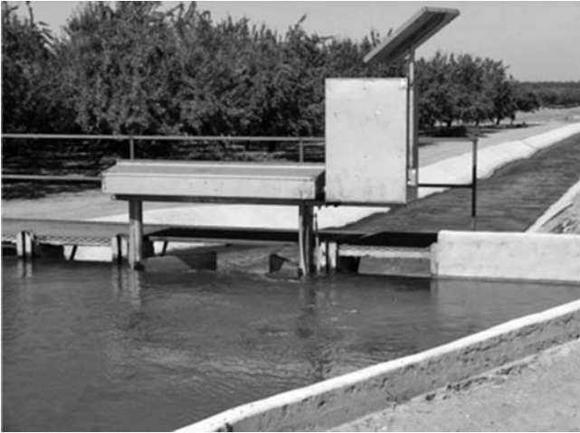
Fig. 2-15. Lopac gate seen from upstream side at South San Joaquin Irrigation District, California, USA
