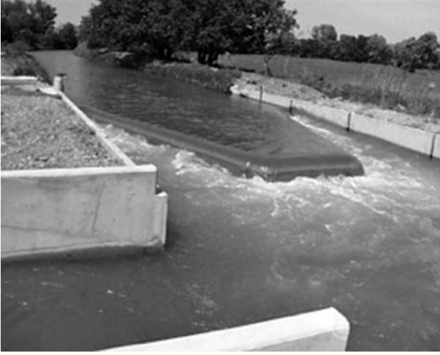
Fig. 2-17. Long-crested weir, duckbill type at Canal du Congrès, France. This design would quickly fill up with sediment if the water was not extremely clean
