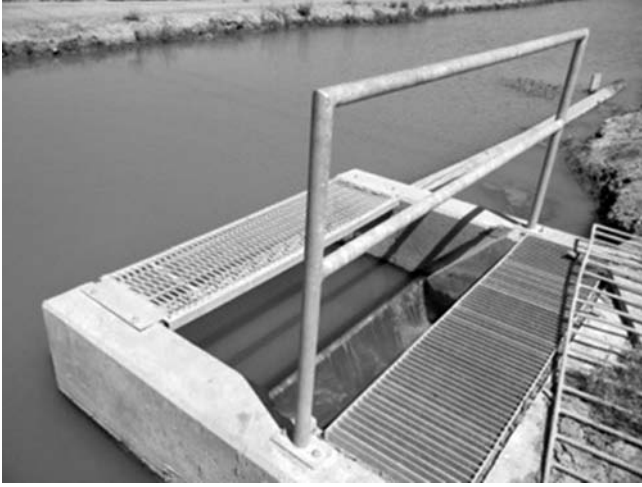
Fig. 2-47. Recirculation spill from a pool downstream of lift pumps, back to the inlet pool. This maintains the water level in the downstream pool, even though the pump flow rate is excessive
