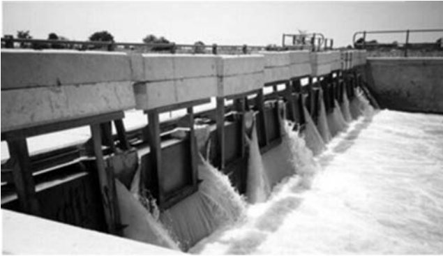
Fig. 2-23. Begemann gate at Hadejia Valley Irrigation Project, Nigeria Source: Photo courtesy of Xavier Litrico, Centre R&D de Lyonnaise des Eaux à Bordeaux, France; reproduced with permission
