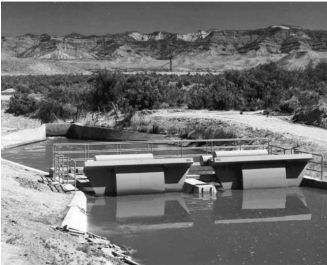
Fig. 2-20. AMIL gates at Government Highline Canal, Grand Junction, Colorado, USA
