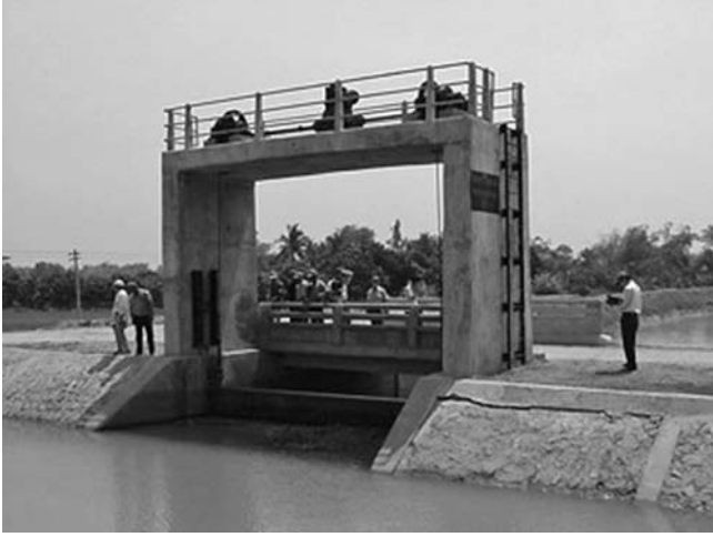
Fig. 2-8. Large motorized sluice gate in Chainat, Thailand. Equipment is difficult to access. A large structure is needed to manipulate the heavy gate
