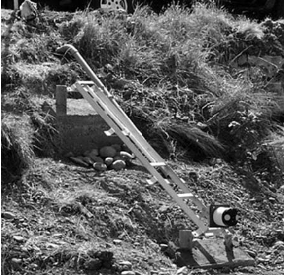
Fig. 2-43. Secure frame that allows the ADVM to be removed from the channel for maintenance and then replaced at the original depth and aspect
