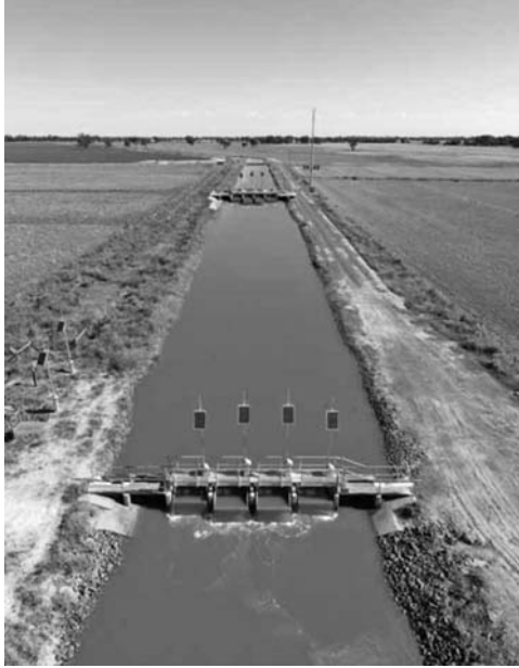
Fig. 8-1. An entire automated canal system in Australia showing automated checks, turnouts (left foreground), and communications tower (background) Source: Photo courtesy of Austrade, Sydney, Australia; reproduced with permission
