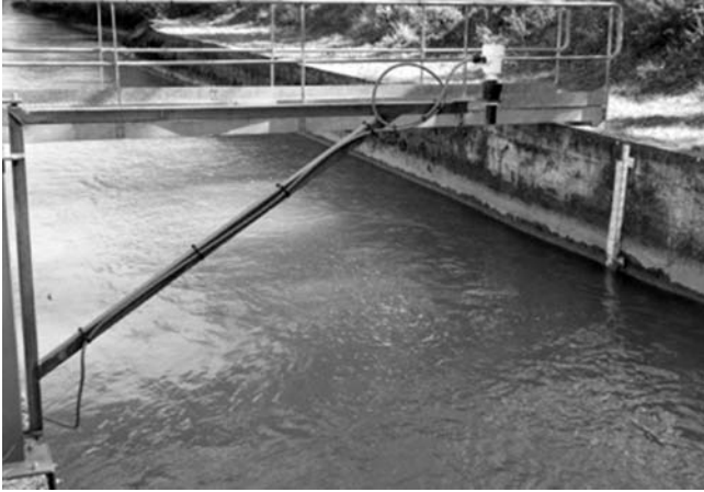
Fig. 2-32. Radar level sensor at the Canal de Marseille, France Source: Photo courtesy of Gilles Belaud, International Center for Higher Education in Agricultural Sciences, Montpellier, France; reproduced with permission
