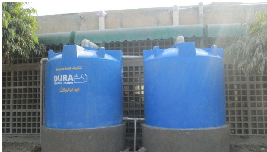
Fig. 15.11 Storage Tank with Inlet and Overflow Pipes
