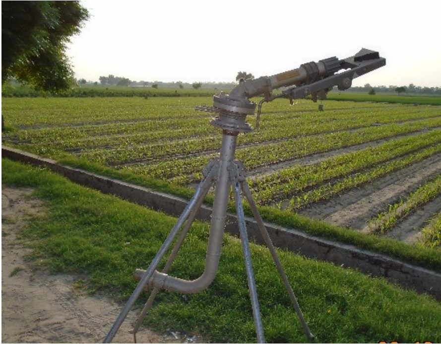
Fig. 13.12 Rain-Gun Sprinkler Irrigation System
