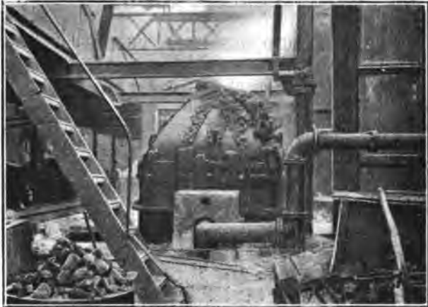
Fig. 30.—Bessemer Converter while Blowing.
