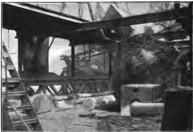
Fig. 35.—Charging Lime into a Bessemer Converter.
