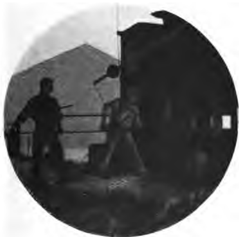
Fig. 48.—Men Charging Steel Furnace.
