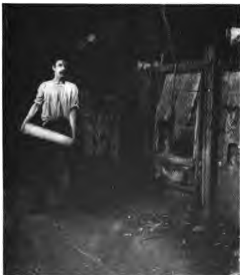
Fig. 6.—Charging a Puddling Furnace.
