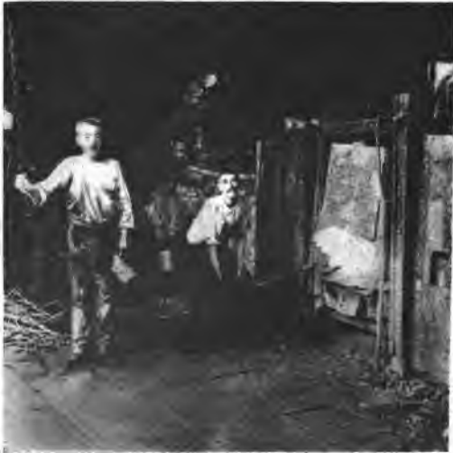
Fig. 9.—Drawing Puddled Ball from Furnace.
