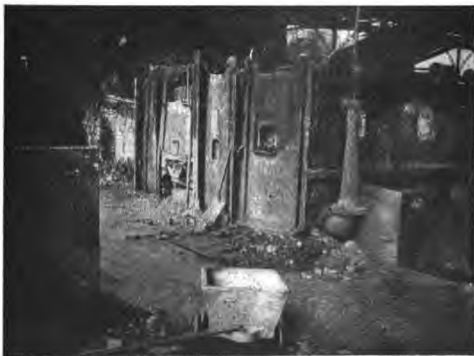
Fig. 1.—General View of Puddling Furnace.
