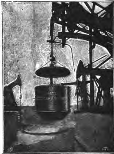
Fig. 98.—Charging Bucket being placed in position at top of Blast Furnace.
