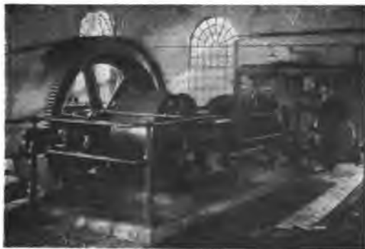
Fig. 96.—Engine Worked by Blast-furnace Gas.
