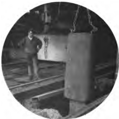
Fig. 51.—Stripping Steel Ingot.
