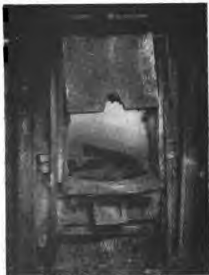
Fig. 7.—Pig Iron in Puddling Furnace.
