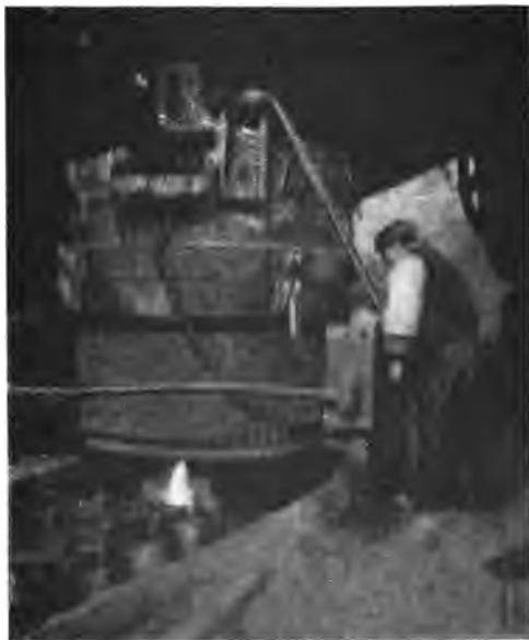
Fig. 50.—Teeming Steel into Ingot Moulds.
