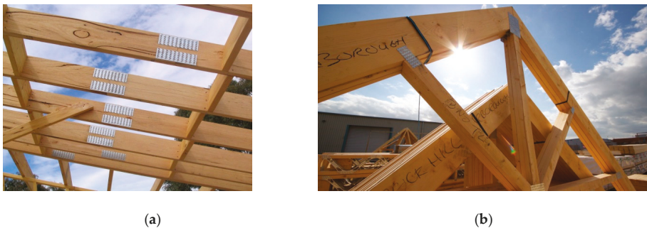
Figure 16. Examples of connections made with nail-plates [51,52].
