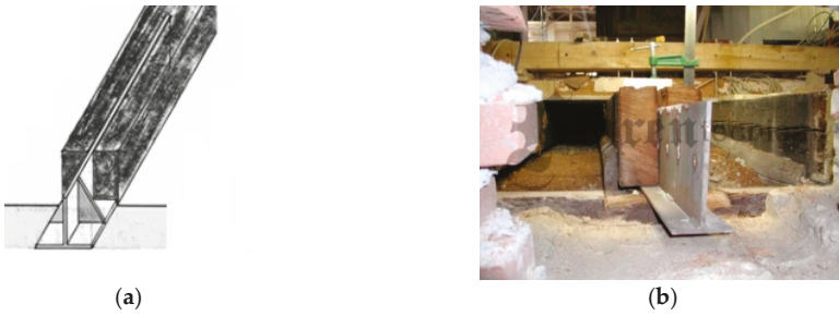
Figure 12. A stainless steel flitch plate inserted into a timber beam and bolted side-to-side: detail of the steel profile used at the beam ends [44,45].
