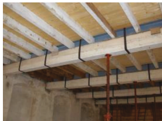
Figure 19. Reinforcement of a timber beam using a stainless steel H-shaped beam applied on the compressed area.
