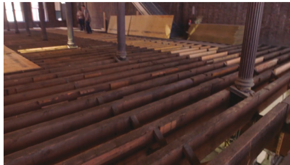
Figure 3. Historic joist floor.
