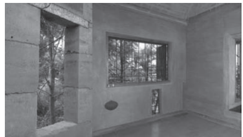
Figure 5. Walls with the visible joints during construction and after rendering.
