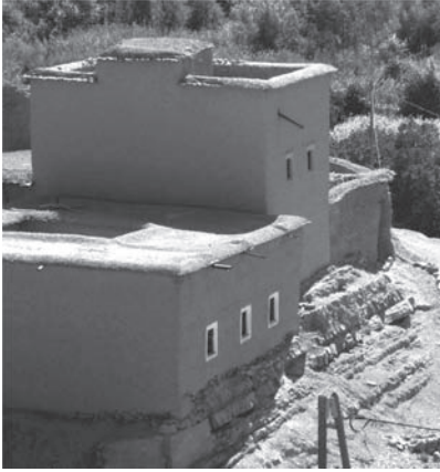
Figure 8. New construction houses made of earth in Immi n-Ouaqqa. Author: J. M. López Osorio.
