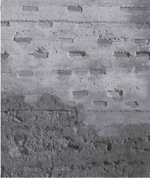
Figure 9. Example of tapia valenciana volumetric reconstruction. Mascarell city wall, Castellón (Author: Cristini & Ruiz Checa).
