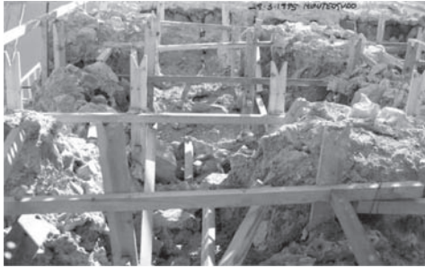
Figure 6. Monteagudo. Putlogs reinforcing the lime concrete.
