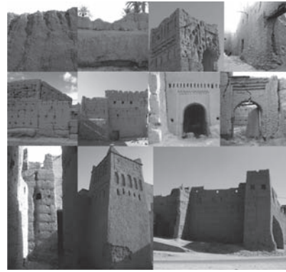
Figure 3. Earthen construction pathologies in the Drâa Valley (credit by CERKAS 2005 and E. Baglioni 2009).
