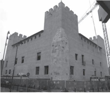
Figure 1. View of the castle in the final processes of the restoration works. In this image we can notice the extension of the of the valencian rammed-earth in the walls.
