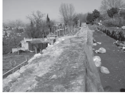
Figure 11. View towards the north. Filled interface.
