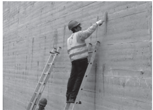
Figure 11. Reparation of small voids and defects. Autor: Vier arquitectos SLP.
