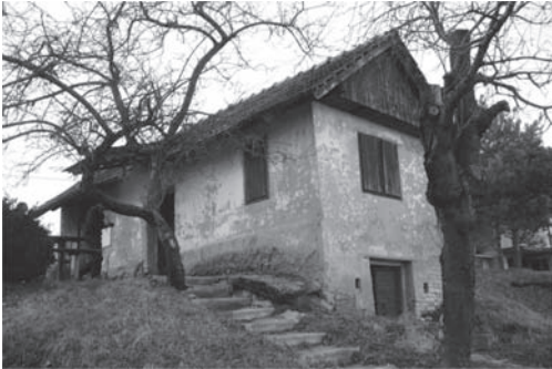
Figure 8. Blatnjača, a cob house, as vine cellar.
