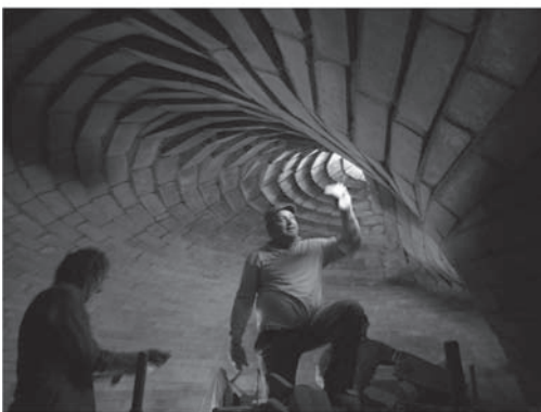
Figure 7. Building Nubian domes without formwork.
