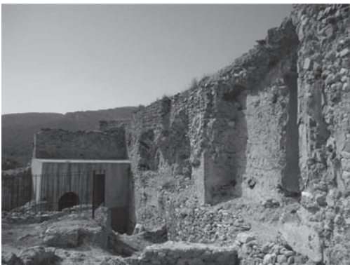
Figure 2. Original view inner side of the wall.
