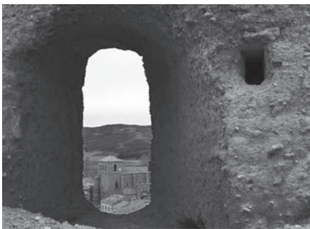
Figure 8. Arrowslit void in the north wall.
