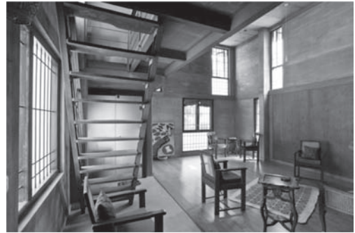
Figure 16. Form work reused for intermediate floor Building 6. Inferences.
