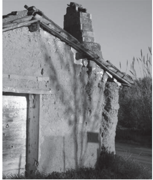
Figure 3. Moscufo, rural building in Contrada Colle di Giogo: the chimney corner.
