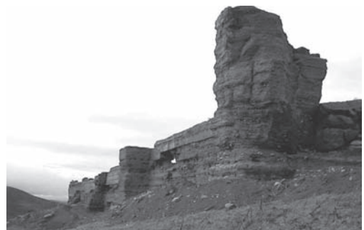
Figure 1. Southwest walls and towers, before work.
