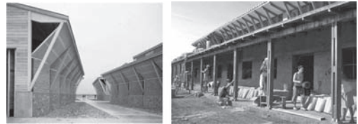
Figures 7 and 8. (Left) Bodega Los Robles, San Fernando, Chile. Source: José Cruz Ovalle. Sandra Bestraten and Emilio Hormias USF. (Right) Universidad Indígena de la Chiquitanía, Bolivia. Source: Sandra Bestraten and Emilio Hormias USF.
