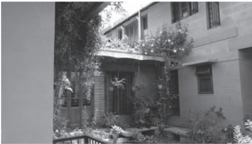
Figure 7. Mud paint rendering on rammed earth walls of Building 4.
