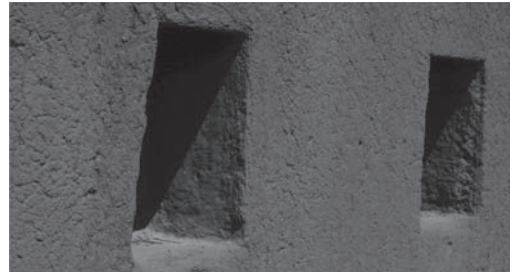
Figure 6. Examples of trapezoidal opening in rammed earth stores; Huchuy Qosco archaeological site, Cusco Province (Cristini Ruiz Checa).
