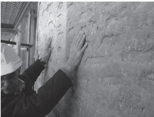
Figure 6. Cleaning tests to remove the existent painting by means of aluminium silicate projection.
