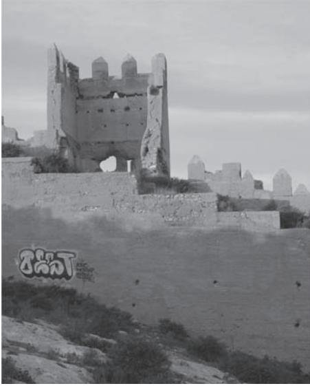
Figure 2. Walls of the San Cristóbal, Almería (2012).
