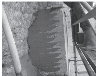
Figure 6. New rammed-earth section. We can see the limed mortar line after ramming. Work of reintegration wall. Church of 'San Nicolas de Bari'. (Pinés & Jové-Architects).
