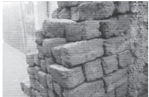
Figure 8. The adobe walls. N. Abderrahim Mahindad.
