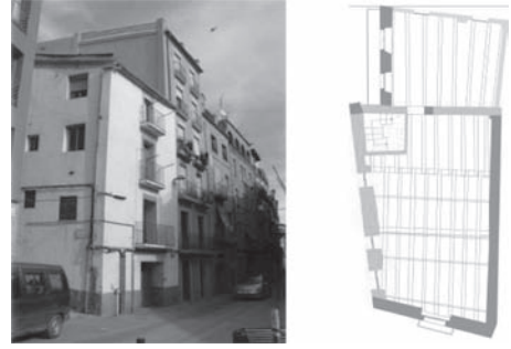
Figure 3. Earth building in the centre of Manresa (Barcelona) partially built in rammed earth. Picture: Cristina Fernández (Final Degree Project-UPC, Tutor: Emilio Hormías).
