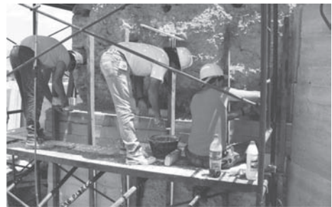
Figure 9. Specifications. Replacement of the crust.
