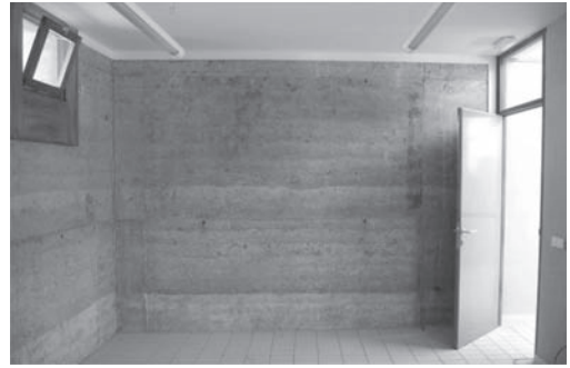
Figure 8. Finished rammed earth wall in library room.
