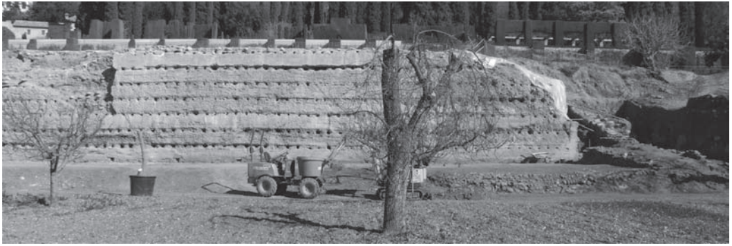
Figure 14. View from the west. South end with remains of the ramp.
