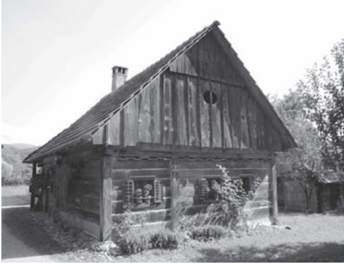
Figure 11. A wooden construction, sealed with clay is useful, successful and decorative. The final decoration in lime is the crosses around the window, made with the fingers.
