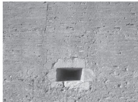
Figure 4. Aspect of the original finish on the tower of the Portal de l'Horta, with the pocket described in the contract.
