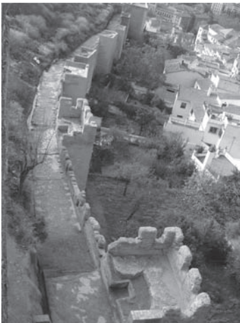
Figure 6. View from tower 8 to tower 14 after the restoration.
