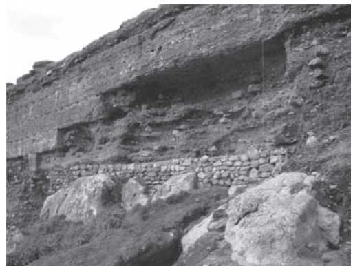
Figure 2. Erosion in rammed earth walls. Here we can see the difference between the two types of raw material used in lower rows and in the upper rows.
