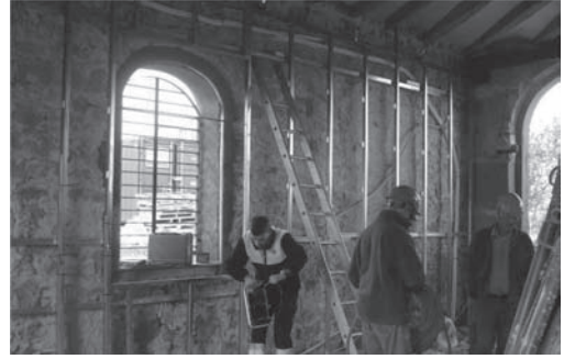
Figure 15. Intervention in Can Muscó. Vilanova del Camí, in the proximities of Igualada (Barcelona). Example of conservation of the bearing function and later new wall. Architect: Josep Vendrell.
