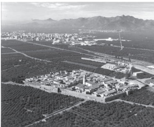
Figure 2. Mascarell (Nules, Castellón). Overview, photo GVA.
