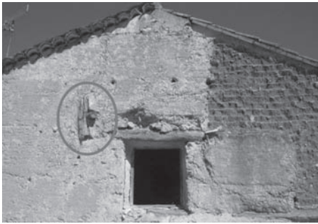
Figure 2. Façade detail of the house with reeled brace.
