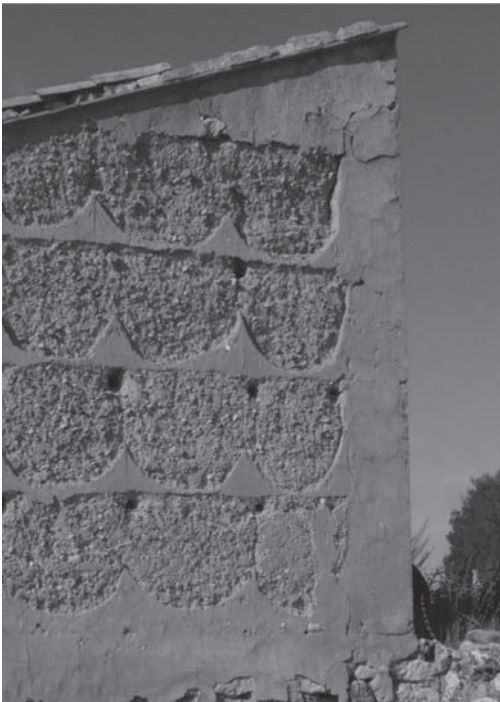
Figure 4. Rammed earth wall with rafas or embedded pilasters at the corner (Vegas & Mileto).
