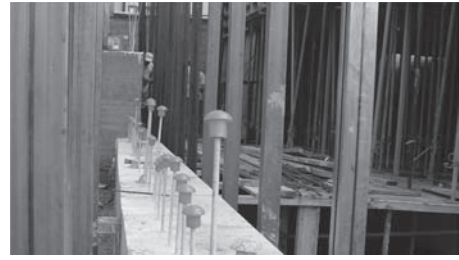
Figure 5. Reinforced concrete foundations with metallic connectors. Autor: Vier arquitectos SLP.
