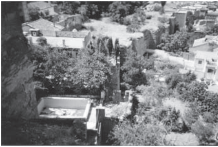
Figure 5. View from tower 8 to tower 14 before the restoration.
