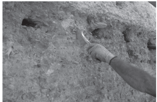
Figure 7. Hand cleaning of the wall with no crust conserved.
