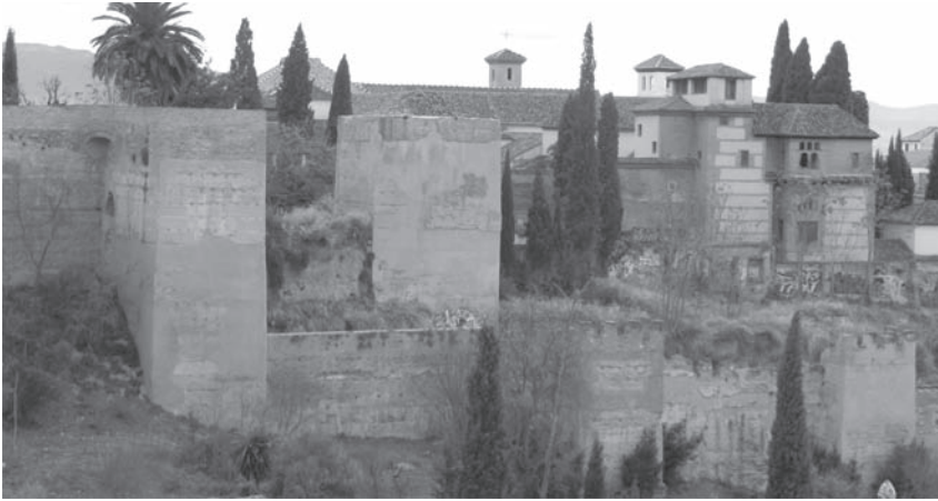
Figure 4. View of the central section after the restoration.
