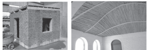
Figures 9 and 10. Reinforced module for seismic simulation tests. Lima, Peru. Source: Marcial Blondet. Domocaña ceiling on Housing in Humay, Peru. Source: Raquel Barrionuevo.
