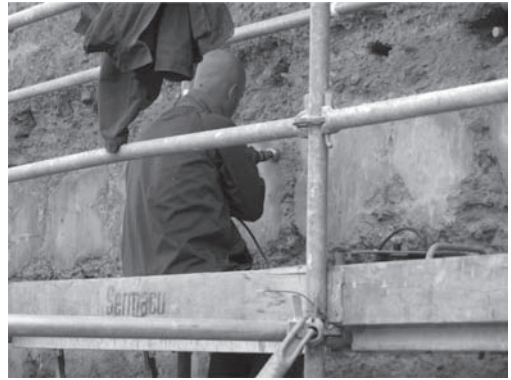
Figure 6. Mechanical cleaning of the crust conserved.
