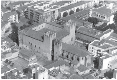
Figure 2. Air view of the castle before starting the restoration works, where can be noticed the northwest tower inexistence.
