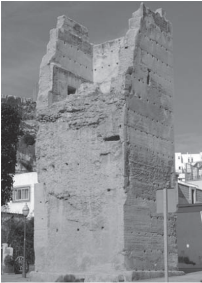
Figure 6. Tower in the district of La Chanca, Almería (2012).
