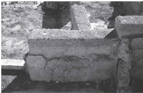
Figure 4. Wall rebuilt with its own rammed earth as Siyasa.
