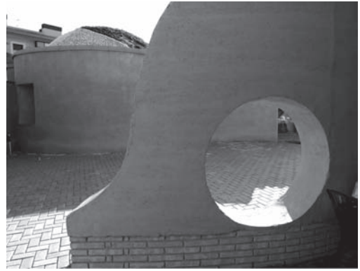
Figure 5. Rammed earth with reserve for a hole.
