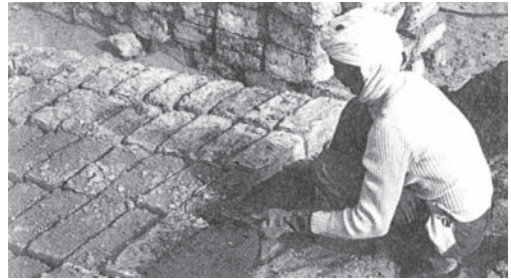
Figure 4. Manufacture of earthen bricks or "Touba" (adobe). N. Abderrahim Mahindad.
