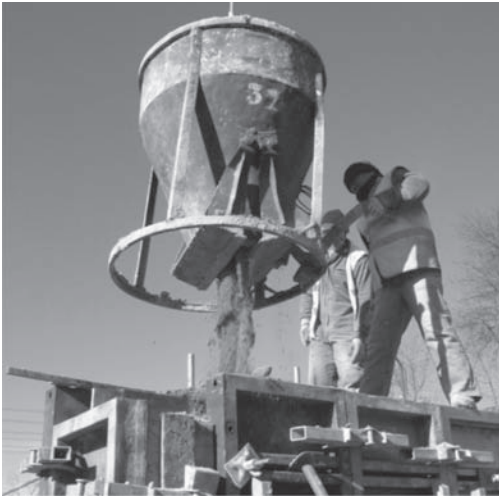
Figure 6. Lifting and pouring earth mix.
