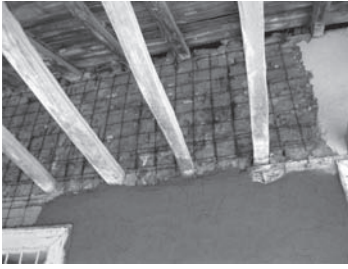
Figure 7. The structural reinforcement technique used by the Chilean architecture studios Arias Arquitectos and Marcelo Cortes (Baglioni E., 2011).
