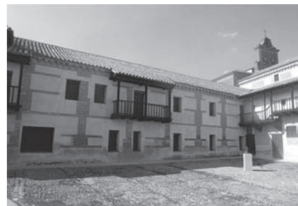
Figure 8. Restored building at the first patio of the Palace of Juan II at Madrigal de las Altas Torres (Ávila, Spain) (Vegas & Mileto).
