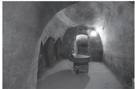
Figure 7. Repnice in Slovenia, artificial caves are cut into the hard, compressed clay. Or is it actually soft stone. photo: Domen Zupančič.
