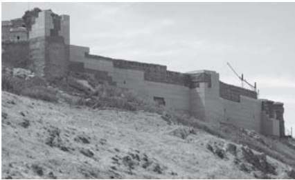
Figure 8. Completion of works on northeast walls and towers.
