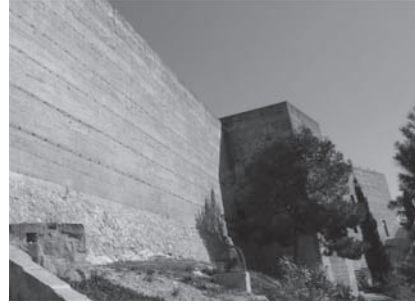
Figure 9. Restored wall of the castle of Petrel (Alicante, Spain) (Vegas & Mileto).
