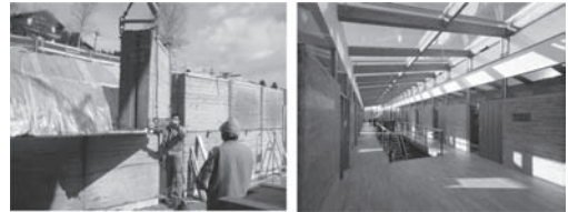
Figures 5 and 6. Prefabricated rammed earth building wall. Printing Gugler. Melk, Austria. Source: Martin Rauch.
