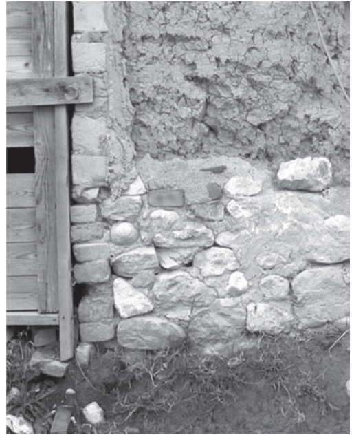
Figure 6. Casalincontrada, rural building; basement created using more resistant materials.
