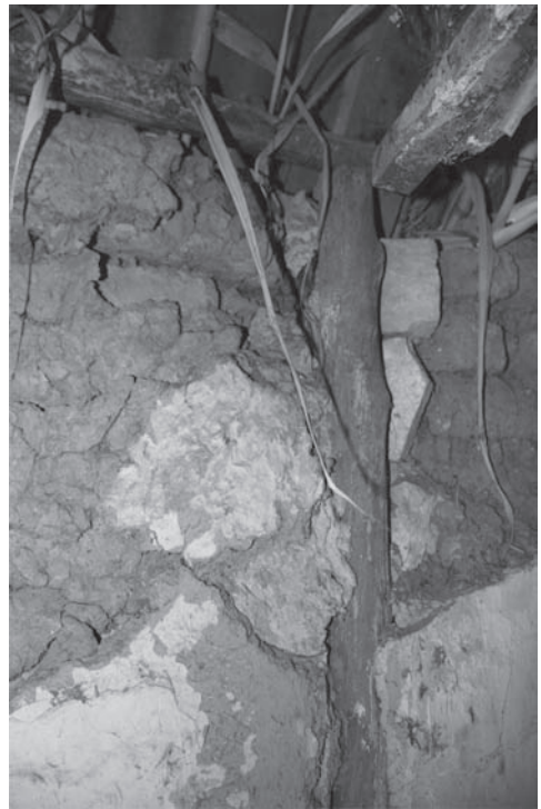
Figure 4. View of a wall reinforced with logs (Pastor, 2012).
