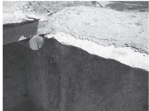
Figure 7. Creation of the protective stone cap.
