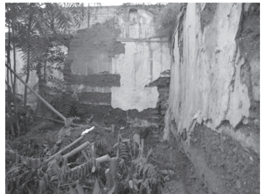
Figure 4. Separation walls alternating mortar joints in ChercHELL. (Aliche, S., 2011).
