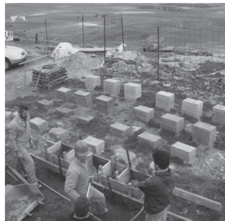
Figure 4. Rammed earth samples, made on site.
