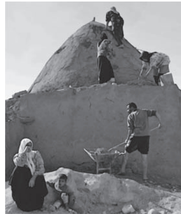
Figure 5. Traditional practice of plaster maintenance (autor: Lupi, L. 2009).
