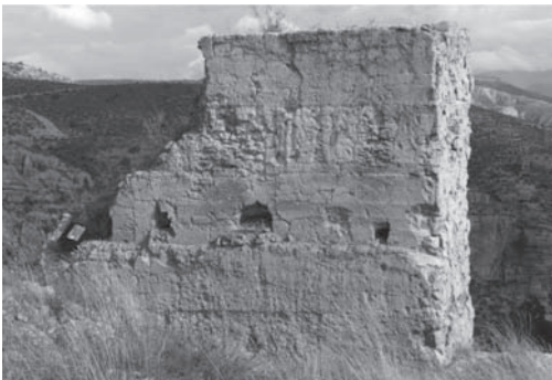
Figure 9. Massive gypsum wall built with formwork for defensive purposes (Vegas & Mileto).
