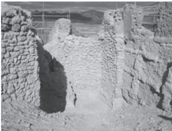
Figure 3. Three types of walls built up with gypsum in different state (stone, binder) and proportion among them, in the northeast angle of the “Castillo Mayor”.
