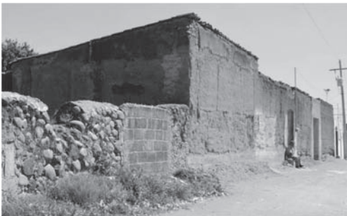
Figure 3. Façade of a vernacular house. Calpan, Puebla.
