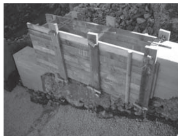
Figure 7. Tapia formwork used for restoration.
