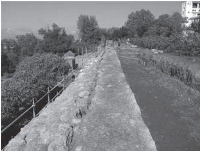
Figure 10. View towards the north. Half-filled interface.
