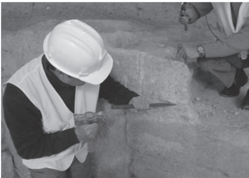
Figure 2. Manual extraction system with chisel and hammer.
