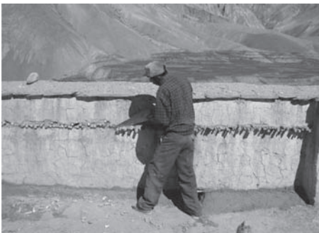
Figure 4. Cutting the protruding wooden elements along the perimeter wall.
