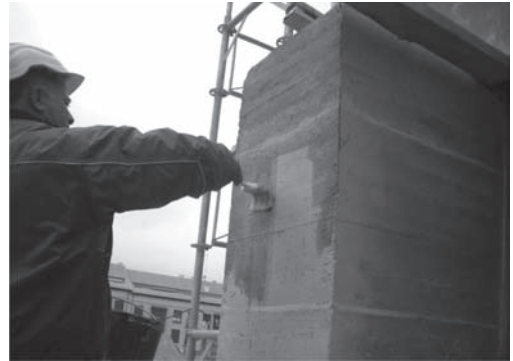
Figure 10. Application of a hydrophobic and fungicide impregnation. Autor: Vier arquitectos SLP.
