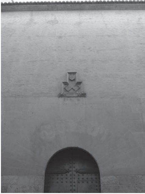
Figure 4. Xàtiva's Almudín façade, in which the valencian rammed-earth wall can be seen, built on the ashlar brickwork.
