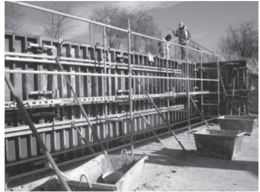
Figure 5. Usual formwork in the construction of concrete walls.
