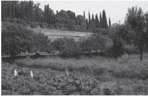
Figure 4. View from the NW before the intervention. The wall, half hidden behind the vegetation at the beginning of the autumn.
