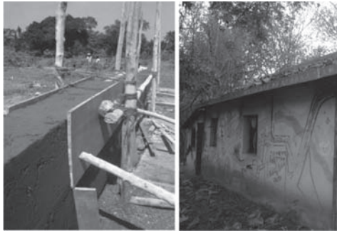
Figure 1. The rammed earth wall and formwork and finished wall in Building 1.
