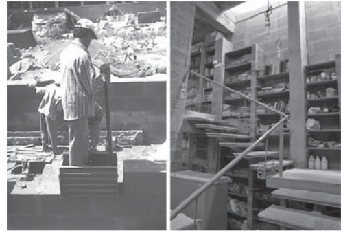
Figure 2. Rammed earth block making and walls in Building 2.
