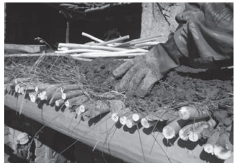
Figure 1. Traditional realization of the roof.
