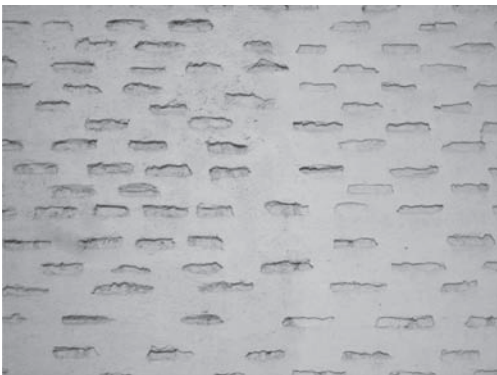
Figure 3. Tapia valenciana wall restored with a protective coating ( Almudín , Valencia). Here two walls from different periods can be perceived.
