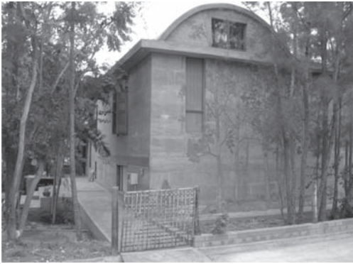
Figure 6. Exterior view of Building 3 with mud cement mural.
