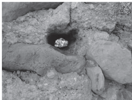
Figure 3. Lime mortar and rough stone with the trace of a putlog in a ruined tapia .
