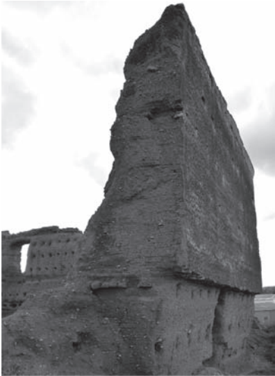
Figure 5. North wall ruins. We can observe the difference of the thickness and the lack of external layer of clay. We can also observe the stones that form the putlog holes in which there were the wood cross ties.
