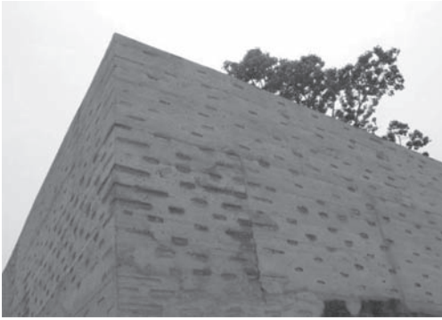
Figure 6. Detail of the wall.
