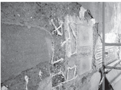
Figure 6. Wall tie elements for rendering.
