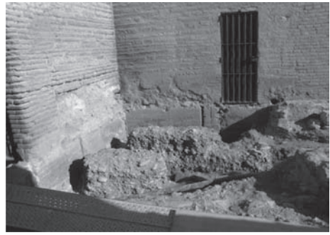
Figure 9. Tapial wall conserving the imprints of the construction process, such as the marks of wood and nails. It is noteworthy that on all the walls there are numerous imprints of the costales which joined vertically the wood of the frames.
