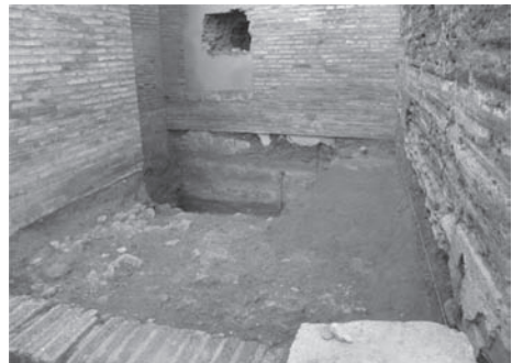
Figure 10. Section in ruins of the wall, constructed in tapial calicastro , which was the union of the three towers.
