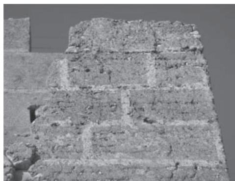
Figure 9. Tower crown with consolidation and reintegration treatments (Vegas & Mileto).
