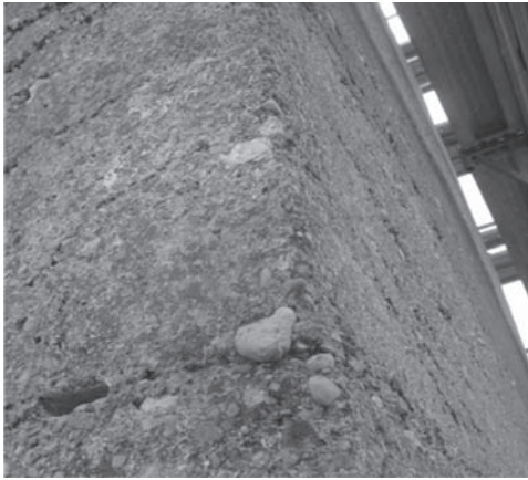
Figure 2. Corner of the tower that shows the continuity of the rammed earth wall (Vegas & Mileto).
