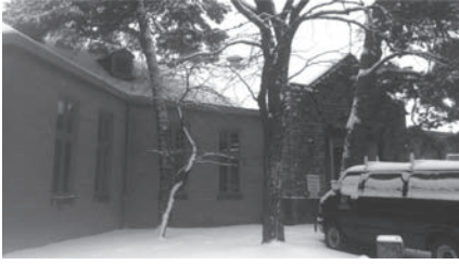
Figure 4. The Mud Hut, Marvin Studios, University of Kansas; built primarily of compressed earth blocks. Photo by author.
