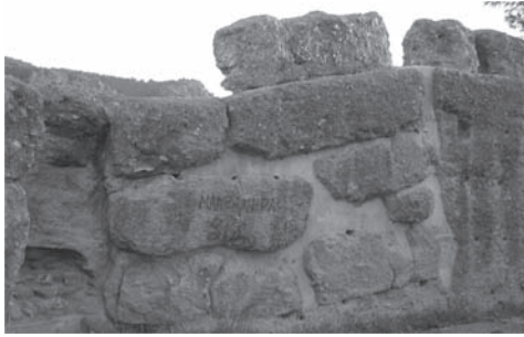
Figure 10. Murcia. La Luz. Rammed earth pieces placed on top of one another.
