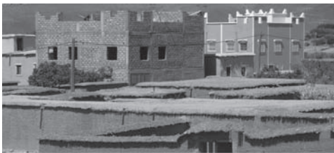
Figure 16. Reinforced concrete house in Alemdoune.
