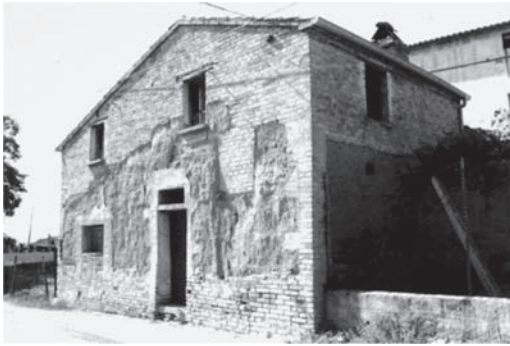
Figure 10. San Omero, building in Locality Case Alte: the original earthen building is increased by a brick raising.
