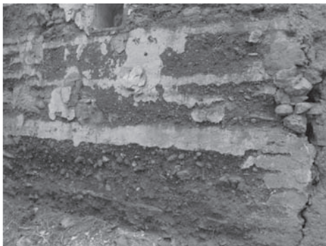
Figure 5. Party wall with alternating mortar layers pattern in ChercHELL. (Alliche, S., 2011).
