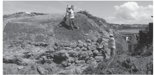
Figure 4. Ramparts: volume repositioning sediment compaction, Forte do Zambujal, Mafra, 2009 (Ana Catarina Sousa).
