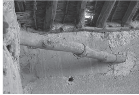
Figure 4. Reeled brace. View from the inside. Brace.
