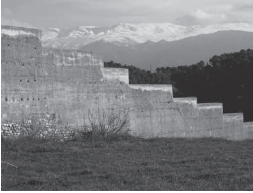
Figure 3. Stepped disposition adapted to the slope of the terrain. (Source: author).
