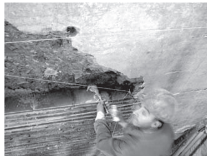
Figure 5. Insertion of the wall ties with plaster and hemp.
