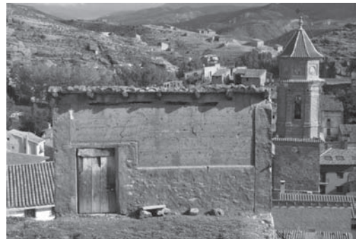
Figure 7. Gypsum thin wall built with formwork between two structural gypsum buttresses in a common auxiliary building (Vegas & Mileto).
