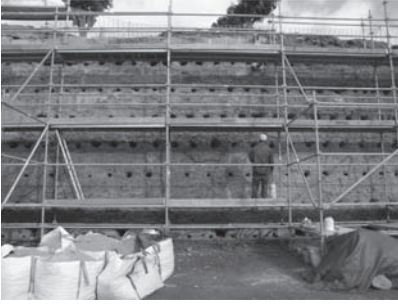
Figure 8. Irrigation with lime wash.
