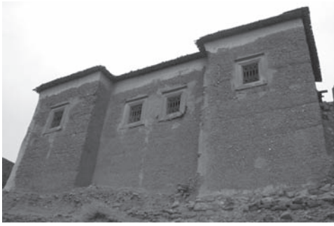
Figure 15. Type III: House in Ait Youb.
