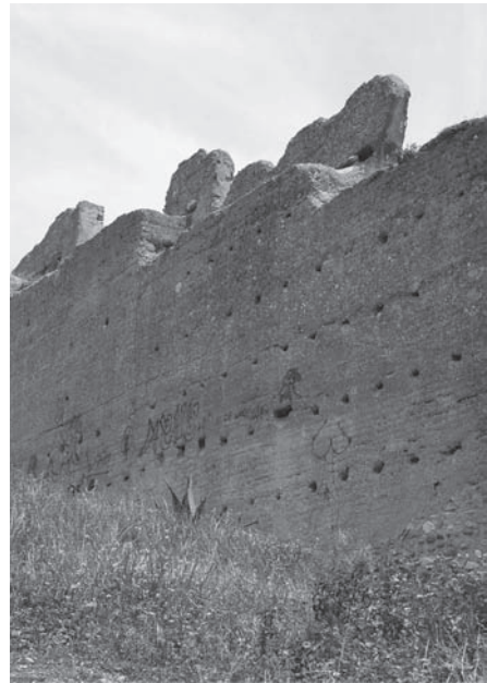
Figure 2. Traces of the crenellated parapet of the Nasrid ramparts. (Source: author).
