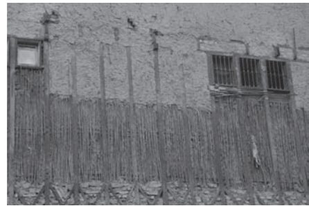
Figure 11. Details of the wicker screens, filled with earth, in a quincha wall, Lima (Authors: Cristini & Ruiz Checa).
