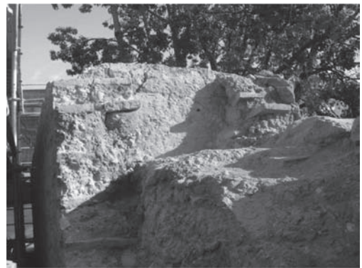
Figure 3. Detail of the original section in the union of two rammed earth walls.
