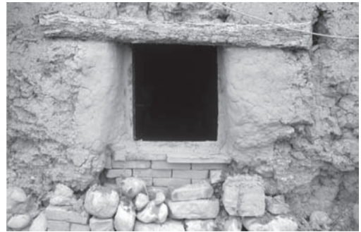
Figure 7. Casalincontrada, rural building; basement created using more resistant materials.
