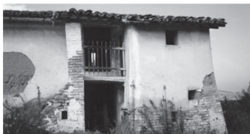
Figure 1. Casalincontrada, a loggia built with baked bricks.
