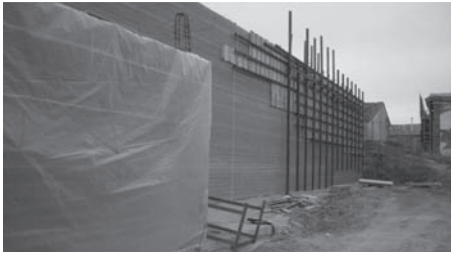
Figure 8. Protection of the wall with plastic sheeting. Autor: Vier arquitectos SLP.
