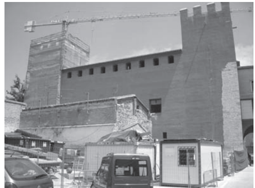
Figure 10. Image of the fourth tower during the reconstruction process.
