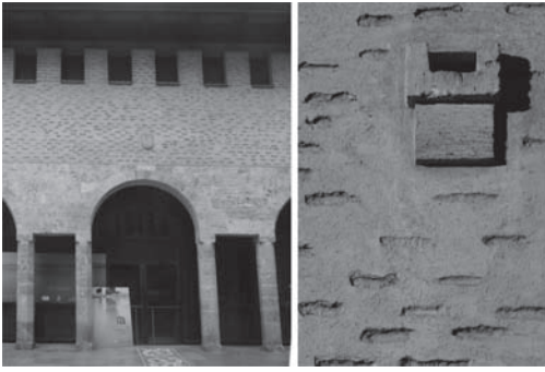
Figure 6. A surface detail, simulating header bricks. Almudín , Valencia (Medieval Granary) (Authors: Cristini & Ruiz Checa).
