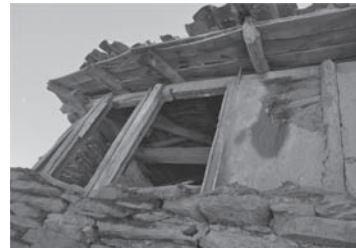
Figure 3. The quincha wooden structure (Jorquera N., 2011).
