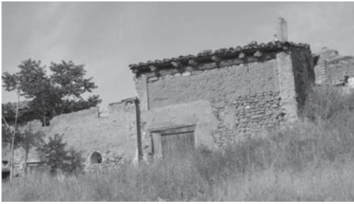
Figure 1. Simple rammed earth wall at Torrebaja standing on a masonry socle between two structural gypsum buttresses that bear a coping girder on which the roof is laid. The presence of the structural buttresses leaves the rammed earth wall free from any structural function (Vegas & Mileto).
