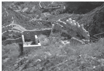
Figure 4. View of the lower albacar after restoration.
