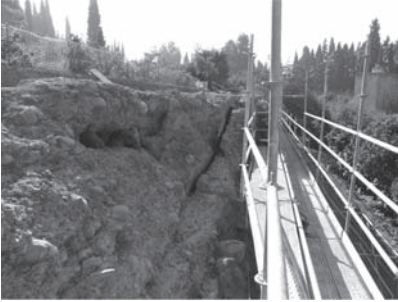
Figure 9. View towards the south. Separation between the two walls. V.
