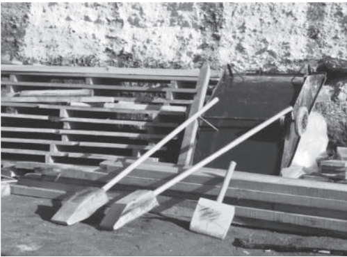
Figure 6. Newly produced formwork and rammers.
