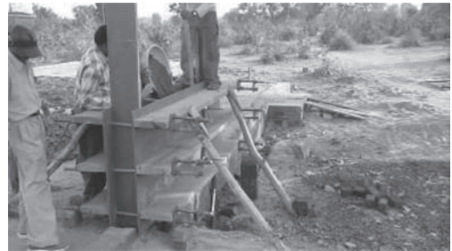
Figure 12. Formwork used in Building 5.
