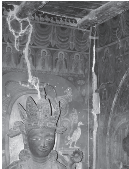
Figure 3. Degrading action on the earthen wall decorations caused by infiltrations of water inside the temple.
