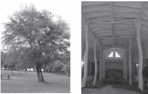
Figure 14. Guarango tree and a covering structure, made with this timber. (Authors: Cristini & Ruiz Checa).
