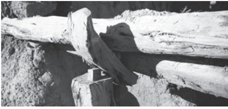
Figure 7. Column, capital and beam.
