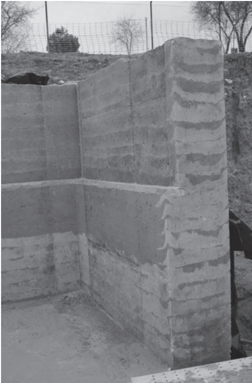
Figure 4. Wall calicostrado. Lime mortar surface finish.
