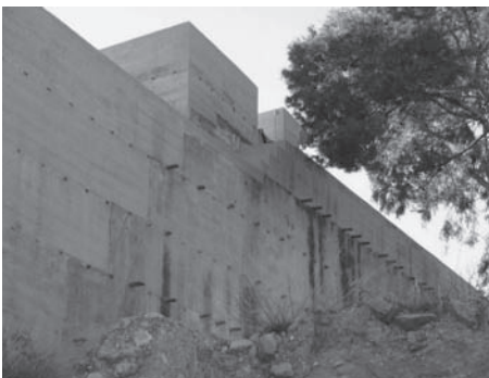
Figure 7. Part of the external wall of the castle of La Mola (Novelda, Alicante, Spain) with the regularization of the volumes (Vegas & Mileto).
