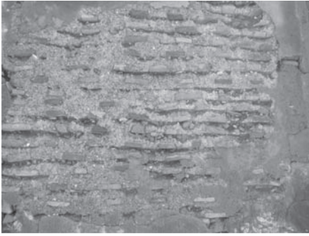
Figure 8. Arrangement of bricks in the wall according to the variant with facing alternating brick and mortar. (Chennaoui. Y., 2007).
