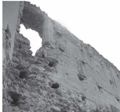
Figure 3. Original view of the outer face of the wall.
