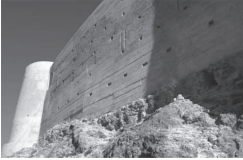
Figure 8. View of the outer face of the wall.
