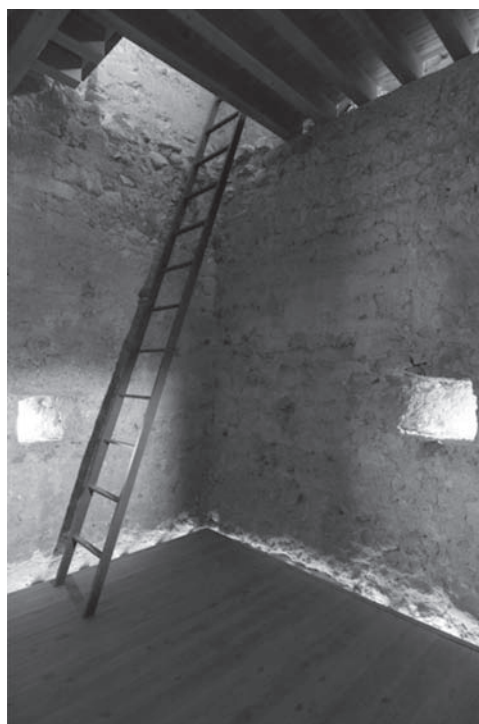
Figure 10. New floors and ladder in the interior of the tower (Baeza).
