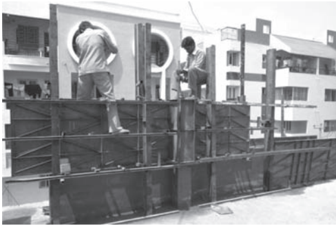
Figure 15. Form work used in Building 6.
