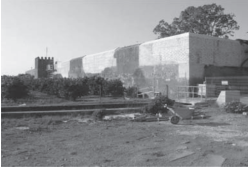
Figure 5. Appearance of finished wall.
