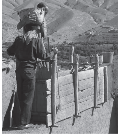
Figure 3. Hauling and pouring the earth.
