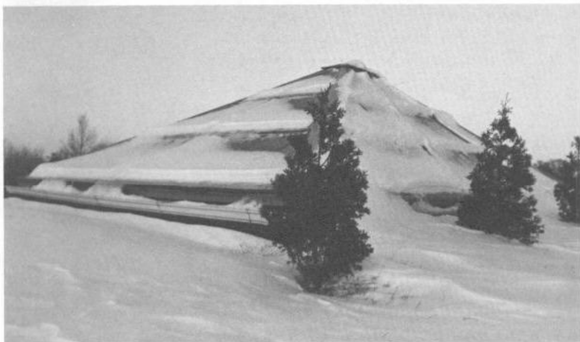
Fig. 18-13. The dome is still in place after six years; snow, wind, and hail haven't phased it.
