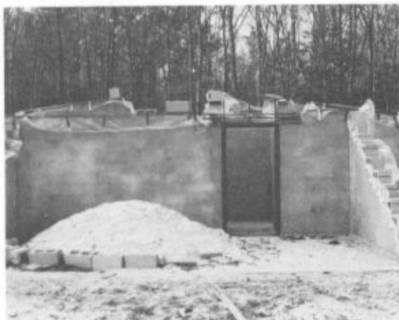
Fig. 2-13. Underground construction above virgin grade.
