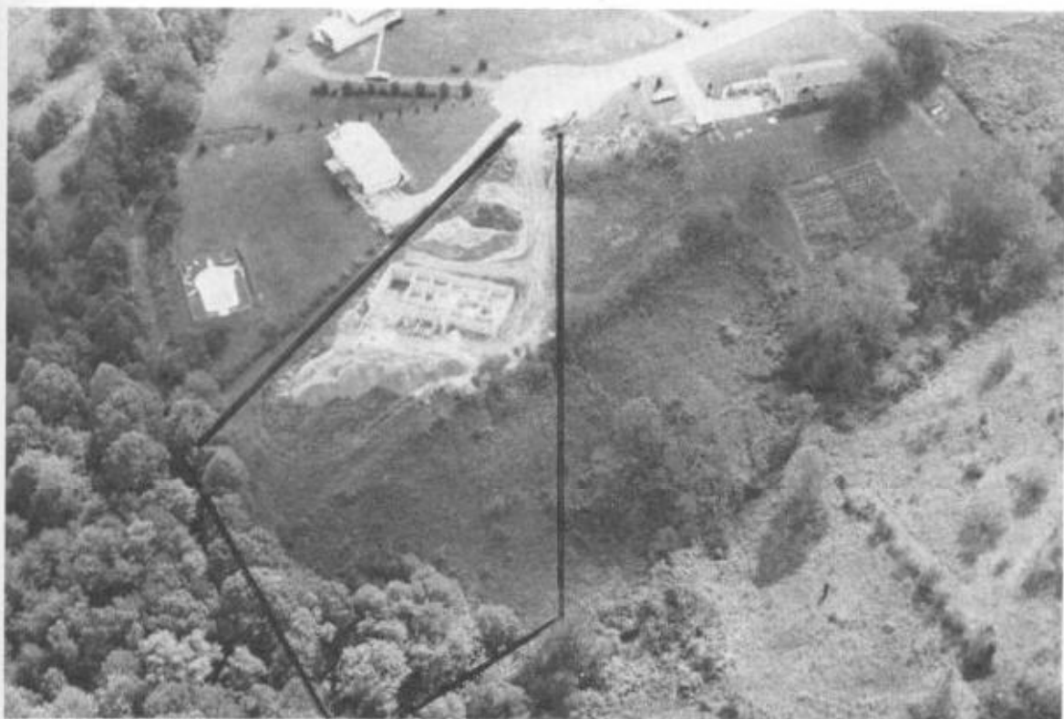
Fig. 2-1. My house under construction. The black line indicates the property line.
