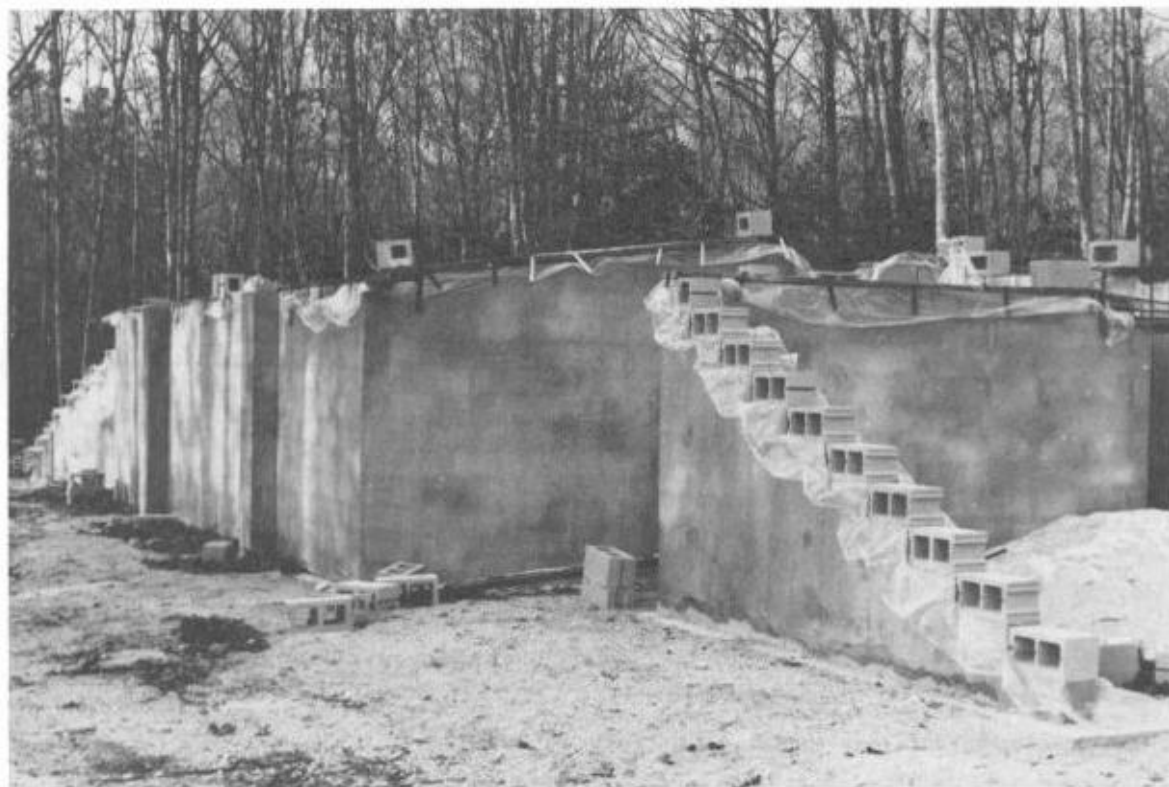
Fig. 2-10. David and Debbie Greenlaw are actually building above ground and then covering the home with earth.
