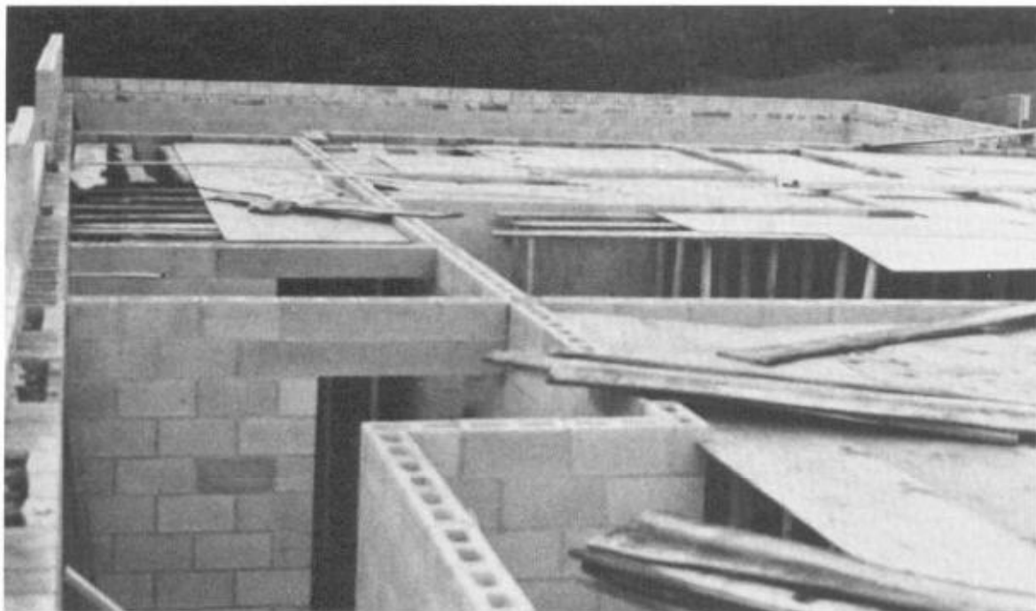
Fig. 9-1. Once interior walls are complete, the wooden shoring structure is started.
