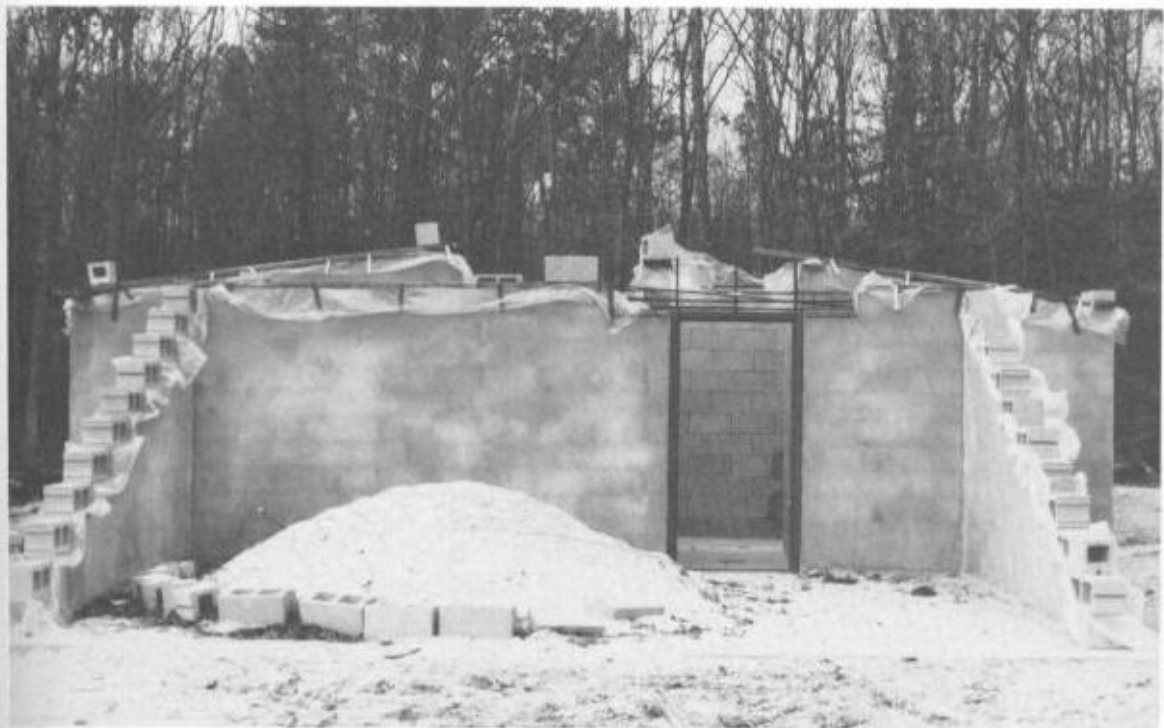
Fig. 10-8. Front view of block construction.
