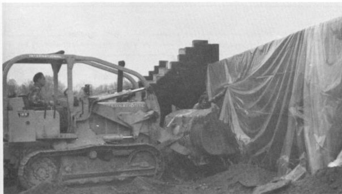
Fig. 13-2. Polyethylene sheets are difficult to keep smooth.
