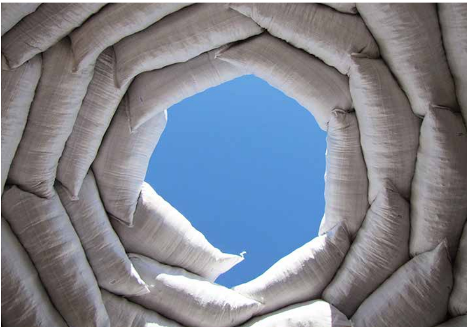
Fig. 2.1: Looking straight up inside an earthbag dome shows the spiraling pattern of bags closing in to cap the dome. This was a small, mostly underground dome with earthen fill situated in the desert southwestern United States. CREDIT: KELLY HART
