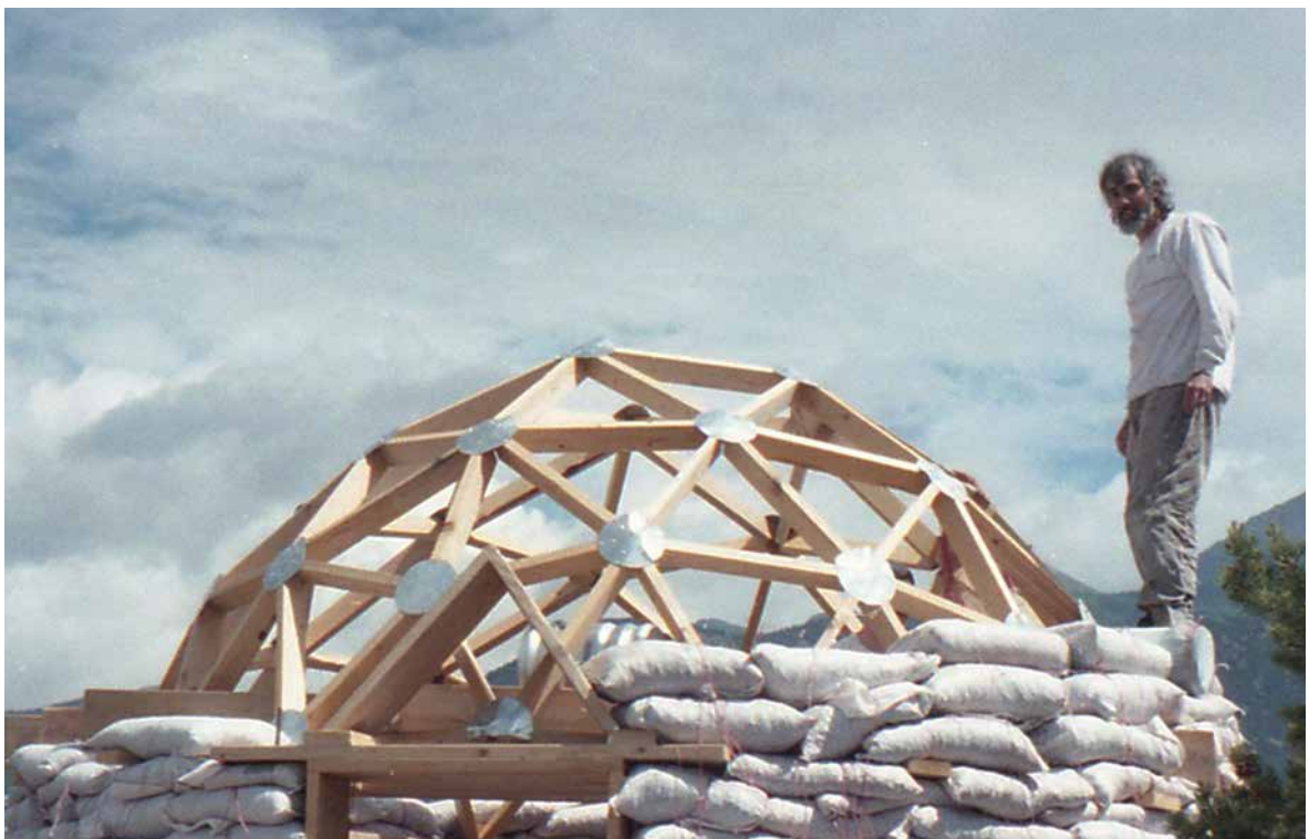
Fig. 8.2: The top of this dome was finished with a hemispherical rigid geodesic framework that remained visible from inside the dome.
