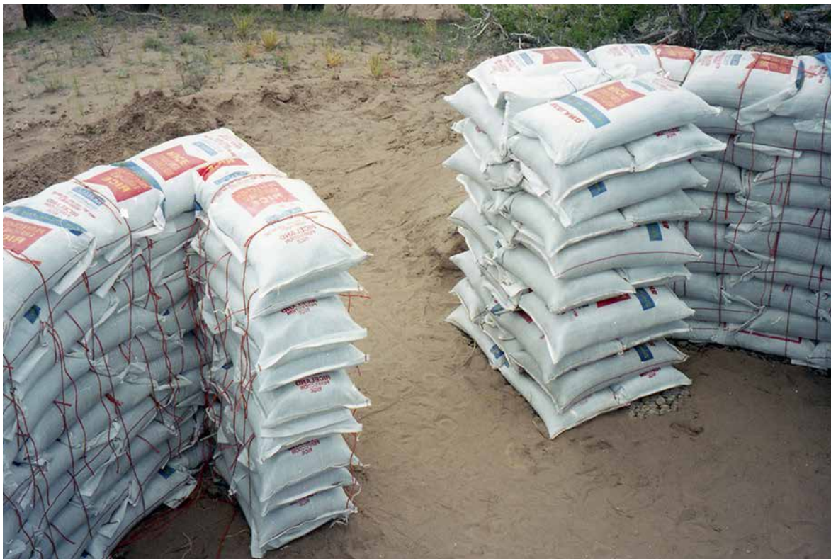
Fig. 8.5: This photo shows two different ways to provide doorway buttressing in a dome; the more massive column on the right is somewhat more stable. Both of the columns are interlaced with the dome wall.
