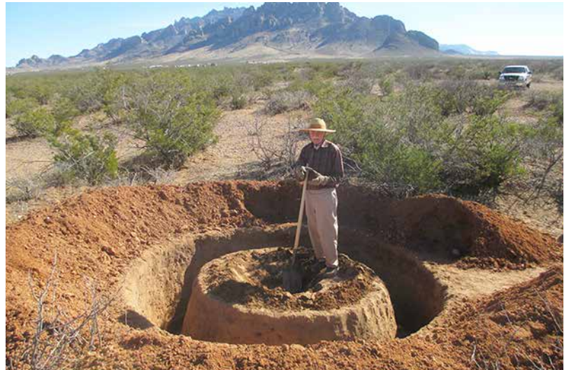
Fig. 8.19: The author is making a mostly underground small earthbag dome on this desert property. He is about ready to start laying bags at the bottom of the trench, using the central column of soil as fill material.
