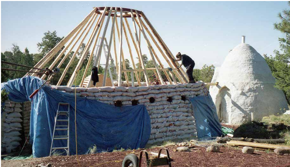
Fig. 8.1: On the left is the large elliptical dome I built with a permanent pole frame structure to hold the shape rigid. On the right is a much more inherently stable circular bedroom dome.
