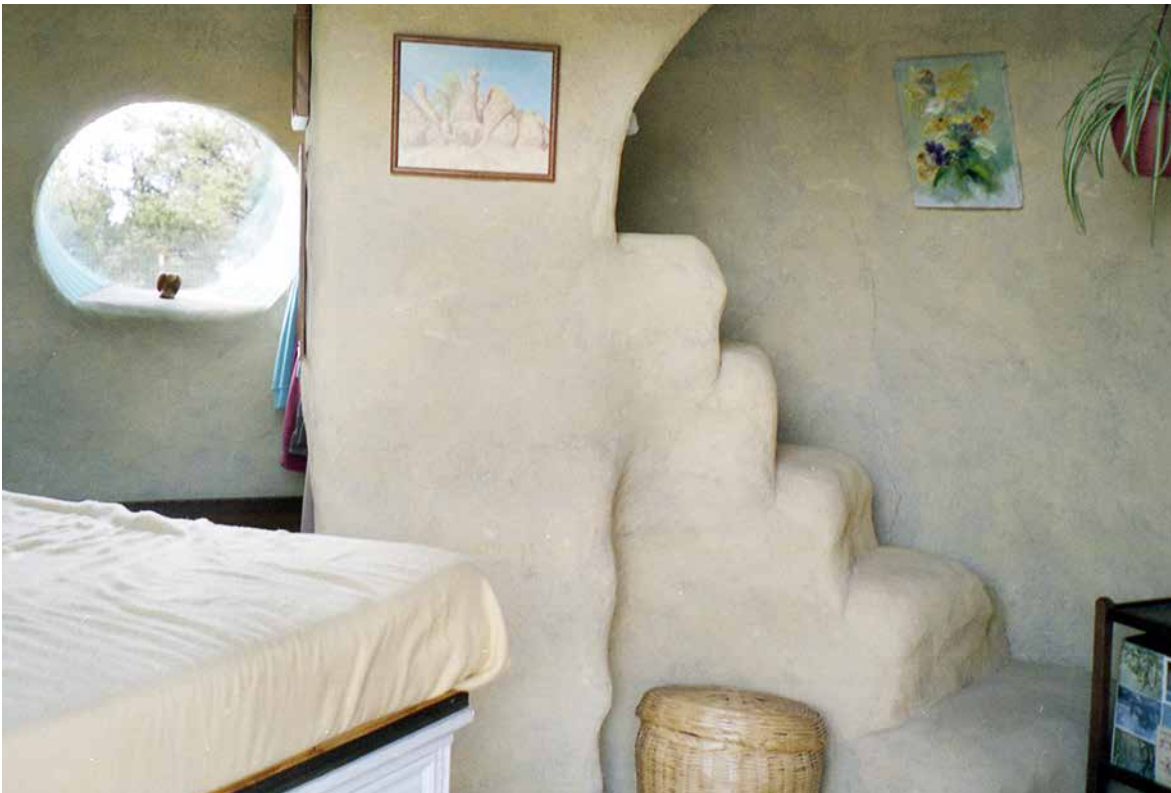
Fig. 11.2: This spiral stairway to a small loft in the bedroom was constructed of earthbags filled with soil to provide a considerable column of thermal mass for the passive solar design.
