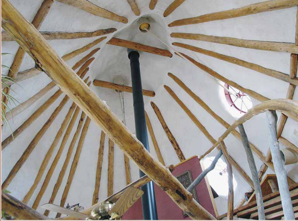
A view toward the loft of the large elliptical dome of the author's house shows the rigid pole framework used to stabilize the shape. CREDIT: KELLY HART
