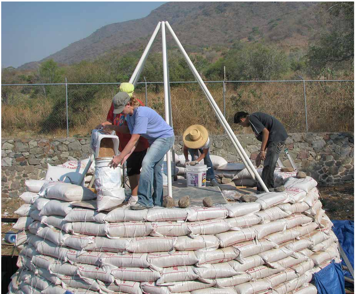
Fig. 7.2: The bags on this dome are being filled in place with buckets of soil. You can see how the bag is placed on a metal slider in such a way that it can be laid down against the previously placed bag. The workers are standing on the loft platform that was already in place.
