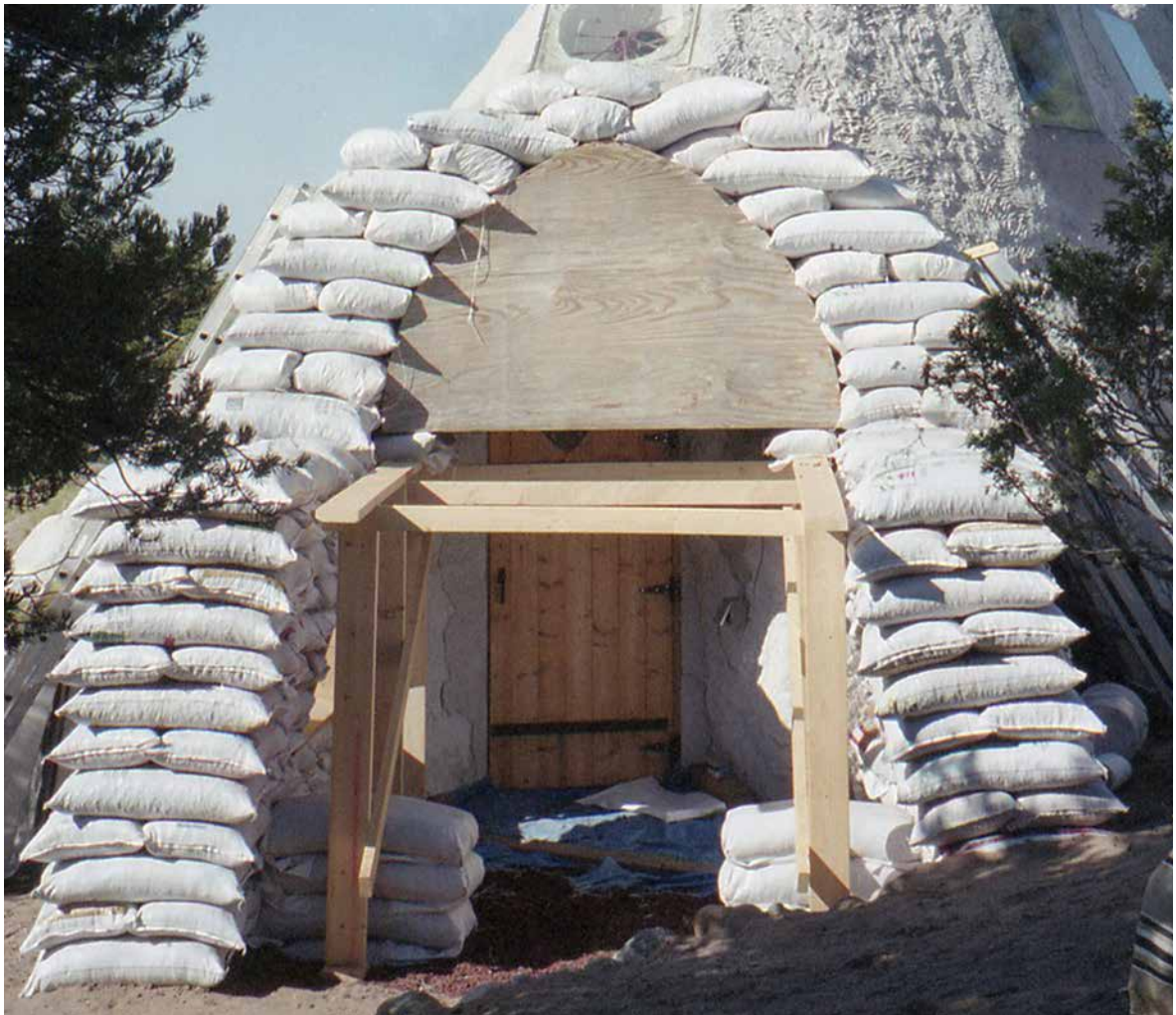
Fig. 8.4: This vaulted entryway spanned 8 ft. (2.4 m) at the base and utilized a 6-ft. (1.8 m) wide Gothic arch form with a sliding track to move it forward. With the inclined sides and massive construction, it was self buttressing.
