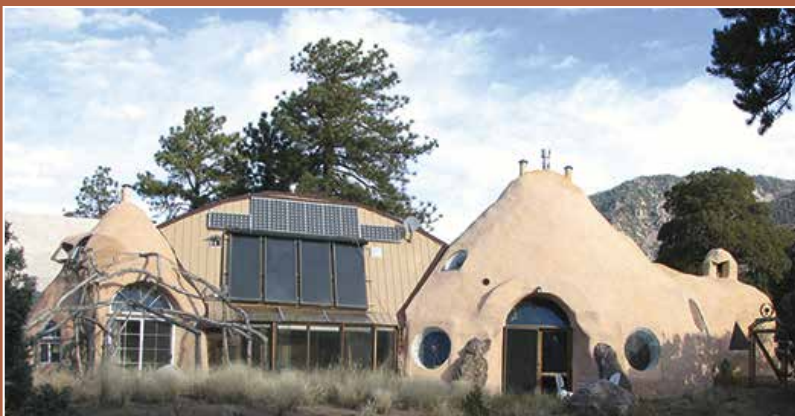
The southern view of the domed earthbag house built by the author shows its passive solar aspects. CREDIT: KELLY HART
