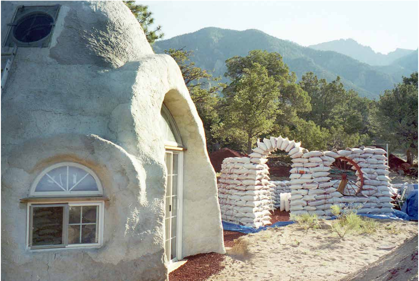
Fig. 1.1: The author's earthbag dome home under construction in 1999.
