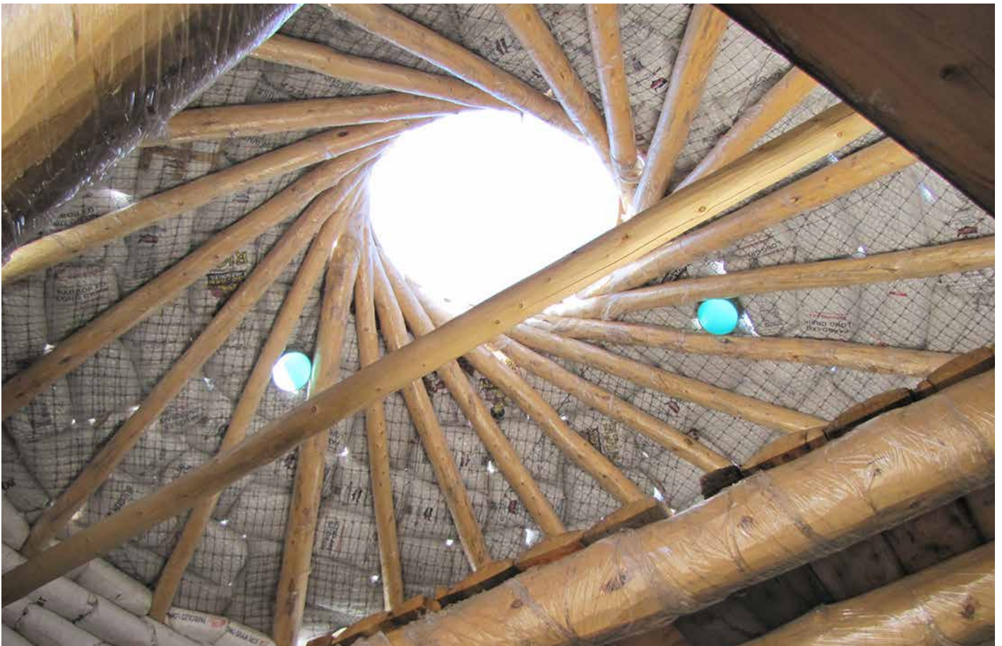
Fig.10.4: This reciprocal roof is actually supporting earthbags filled with lightweight insulating scoria. CREDIT: KELLY HART
