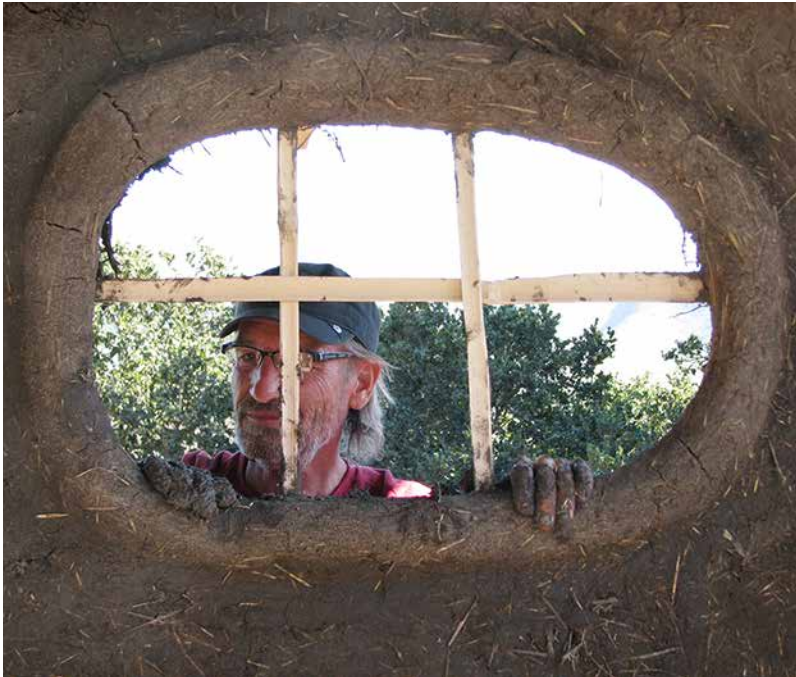
Fig. 9.2: An initial rough coat of earthen plaster is being applied to this wall. CREDIT: KELLY HART
