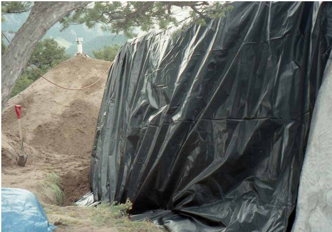
Fig. 8.19: The author is making a mostly underground small earthbag dome on this desert property. He is about ready to start laying bags at the bottom of the trench, using the central column of soil as fill material.
