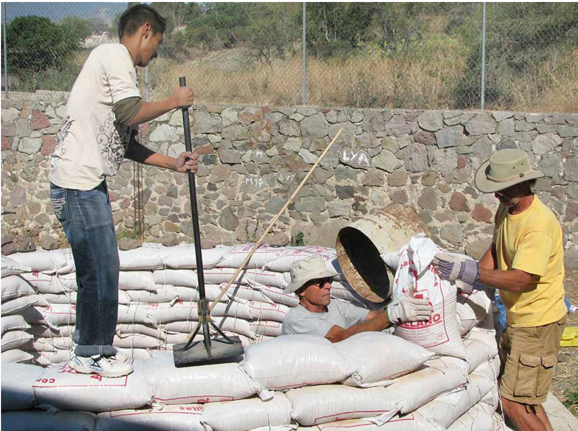
Fig. 7.8: Tamping is usually best done while standing on the wall to be able to put some force into the stroke.
