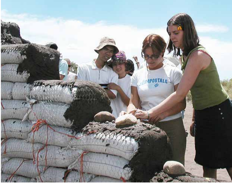
Fig. 4.9: These participants in an earthbag workshop are inserting personal mementos into the freshly plastered wall. On the reverse side of the wall you can see how the chicken wire mesh was tied into place with pieces of twine.
