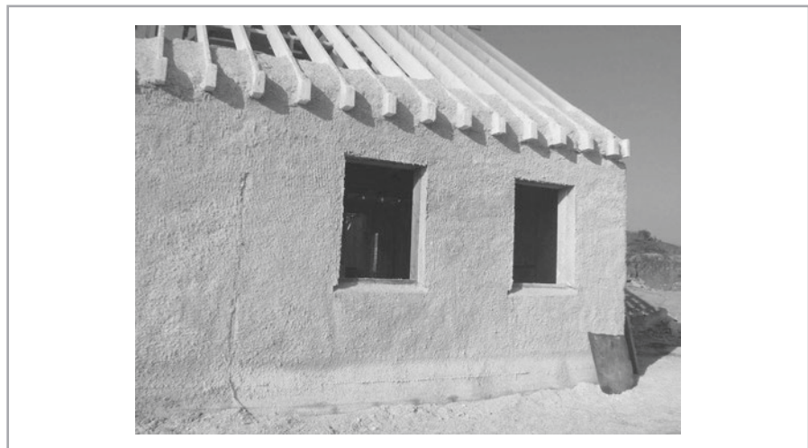
Figure 13.8 External walls coated with sprayed hempcrete.
