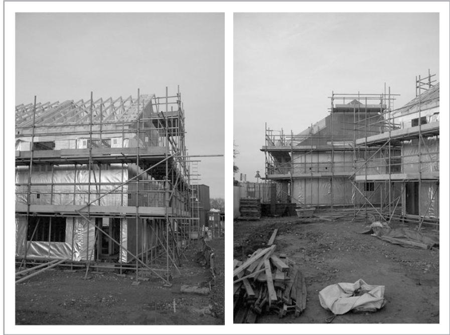
Figure 13.2 Timber framed house construction.
