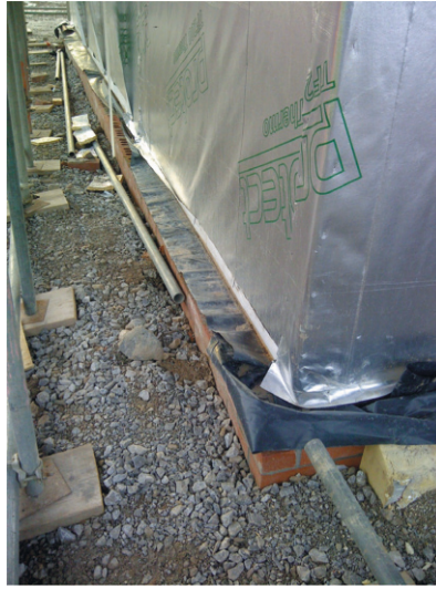
Plate 17: Timber frame at DPC level
