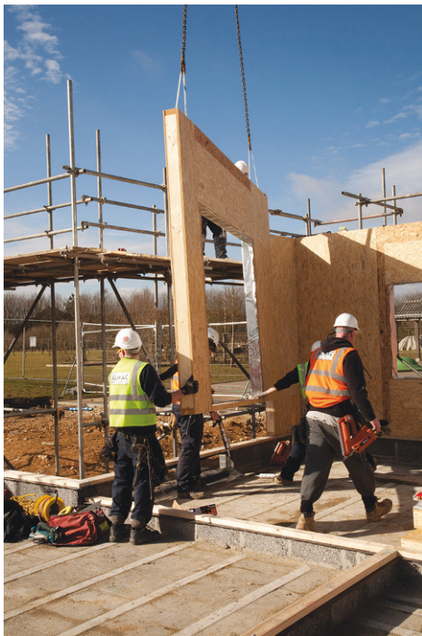
Plate 31: SIP panels positioned
