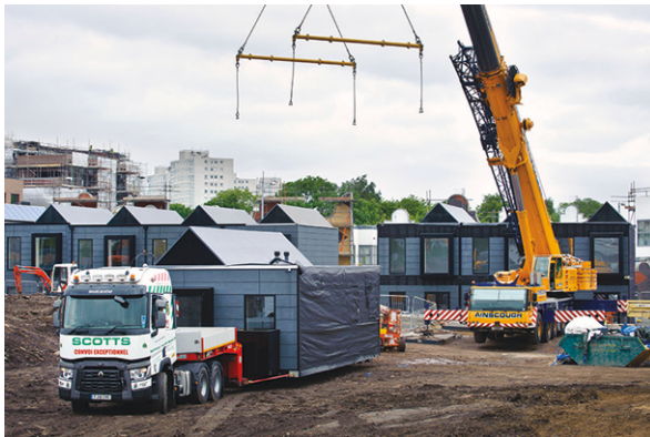
Plate 37: Storey height units delivered by lorry
