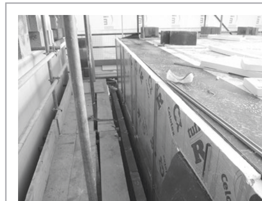
Figure 7.53 Warm frame for a building.
