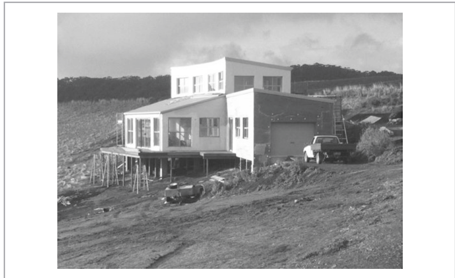
Figure 13.7 Hemp house under construction.
