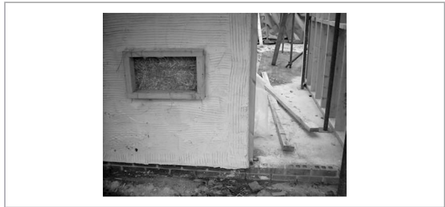
Figure 13.6 Straw bale wall construction.
