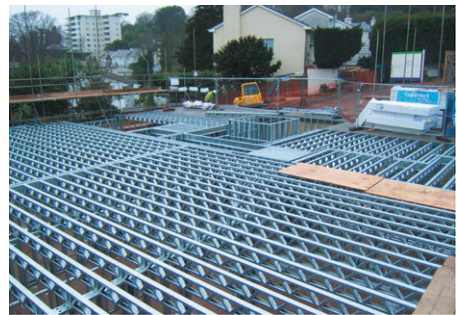
Plate 27: Upper floor structure
