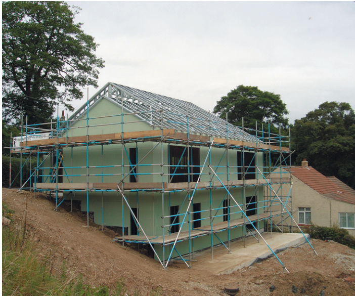
Plate 25: Frame nearing completion
