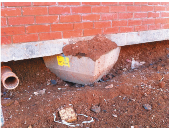
Plate 3: Precast proprietary concrete foundations
