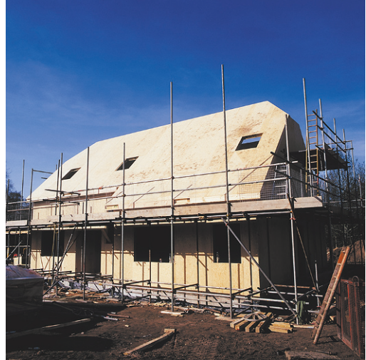
Plate 36: Enclosure awaiting cladding
