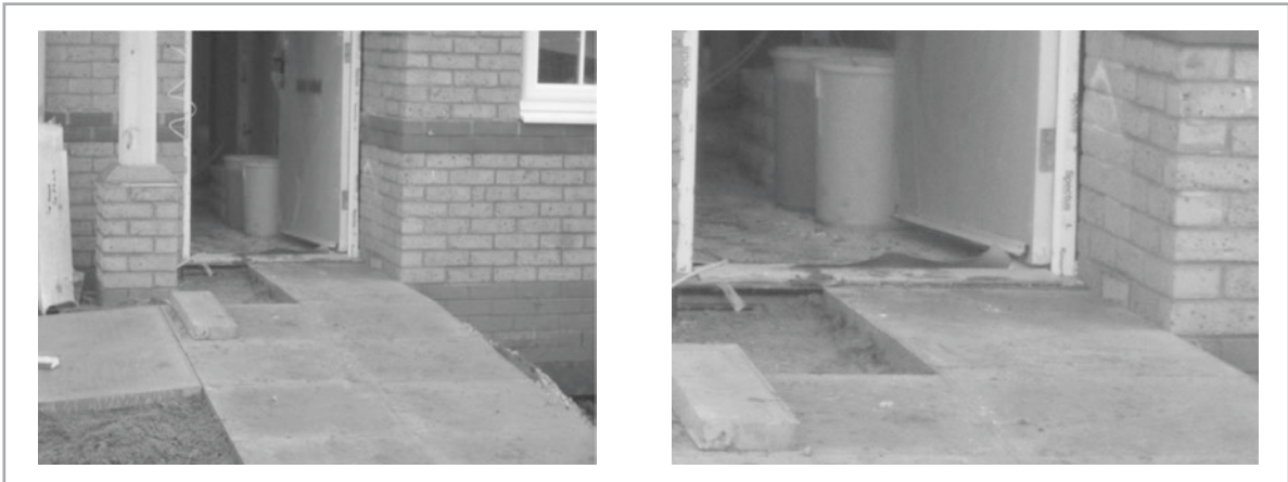
Figure 6.11 Level threshold example during construction.
