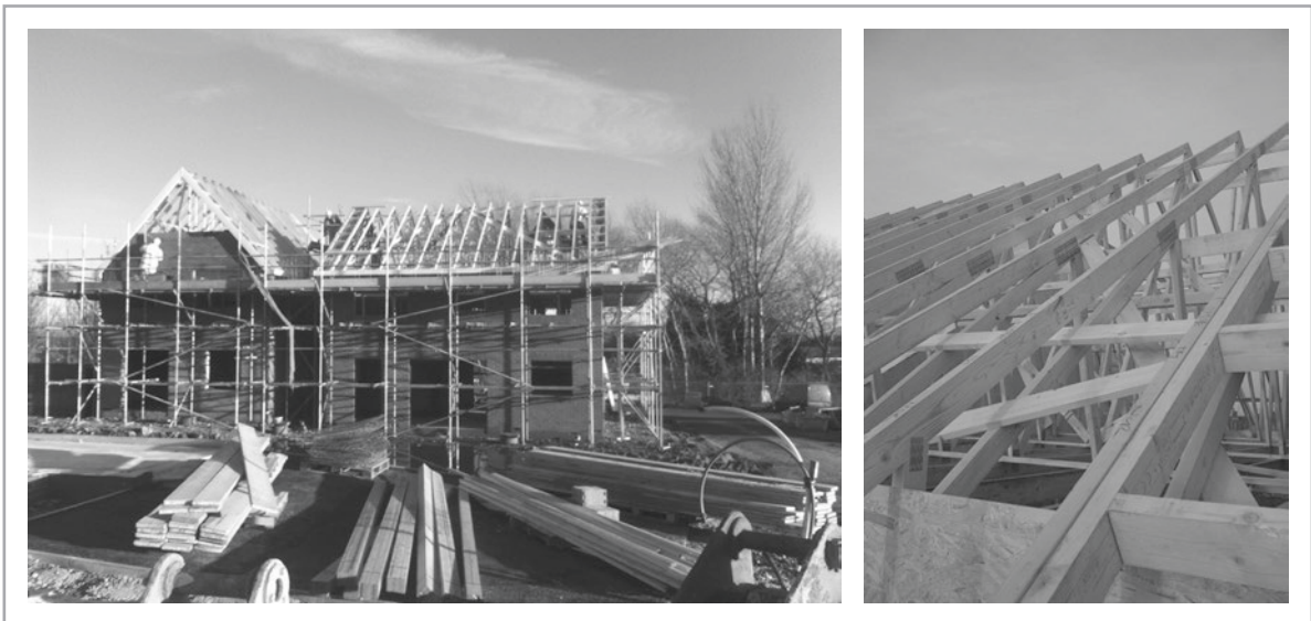
Figure 10.18 Trussed rafter roof during construction.
