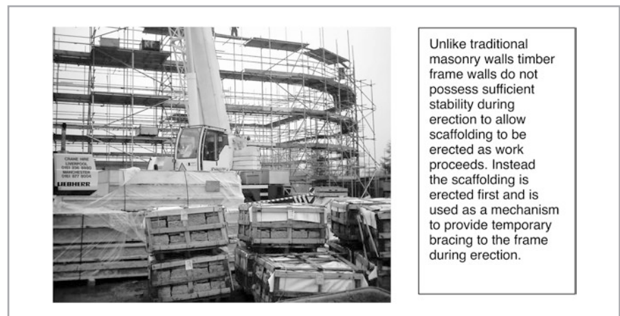
Figure 7.26 Use of scaffolding in erection of timber frame walls.
