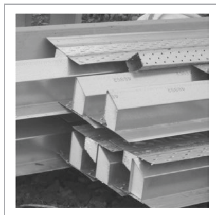
Figure 7.70 Insulated steel lintels stored on-site.
