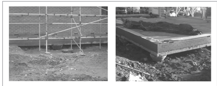
Figure 13.1 Proprietary foundation system.
