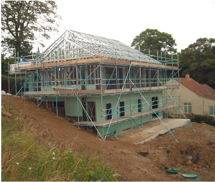
Plate 24: Insulation applied to the frame
