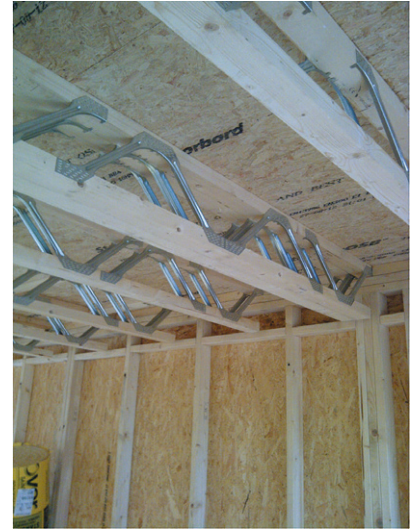
Plate 18: Upper floor construction
