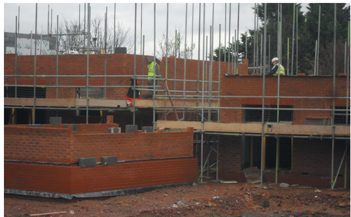
Plate 12: External wall construction
