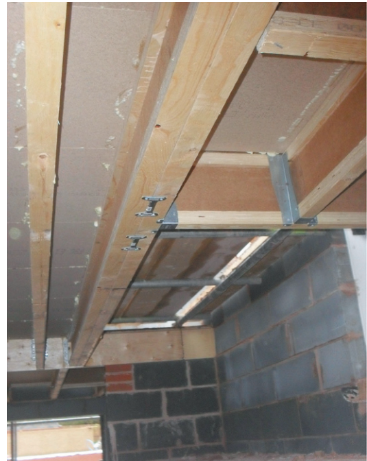
Plate 10: Upper floor construction
