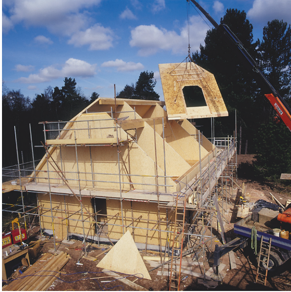
Plate 35: Roof Panel placement
