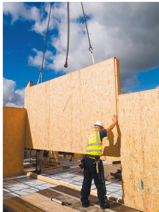
Plate 32: Panel connections made
