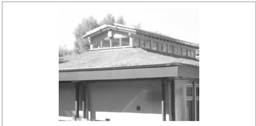
Figure 13.17 Extensive green roof.
