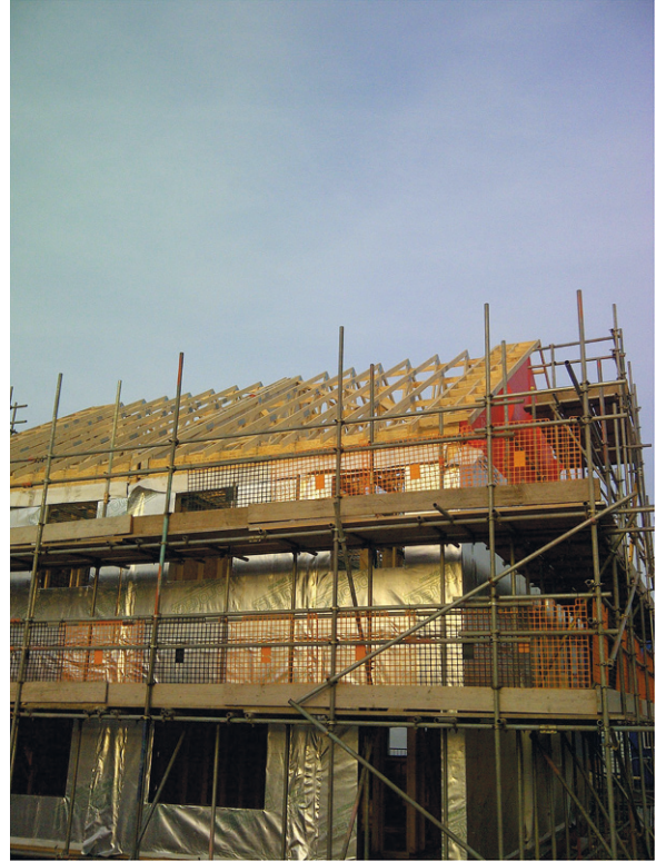
Plate 22: Timber frame nearing completion
