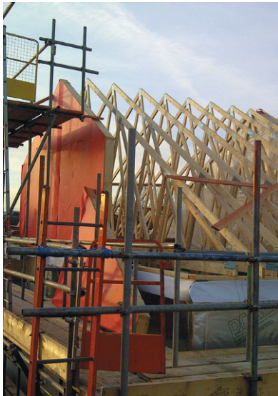
Plate 19: Trussed rafter roof
