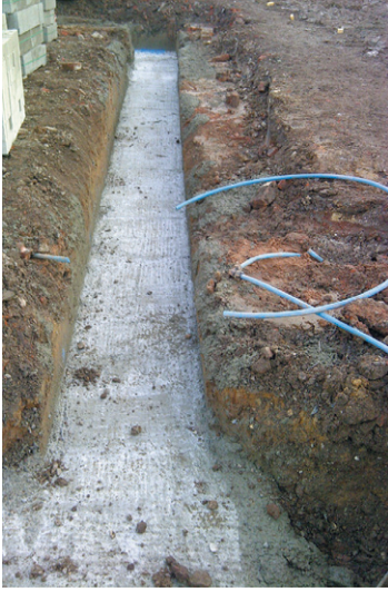
Plate 16: Mass concrete strip foundation
