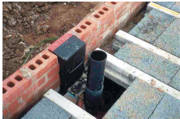
Plate 4: Beam and block ground floor
