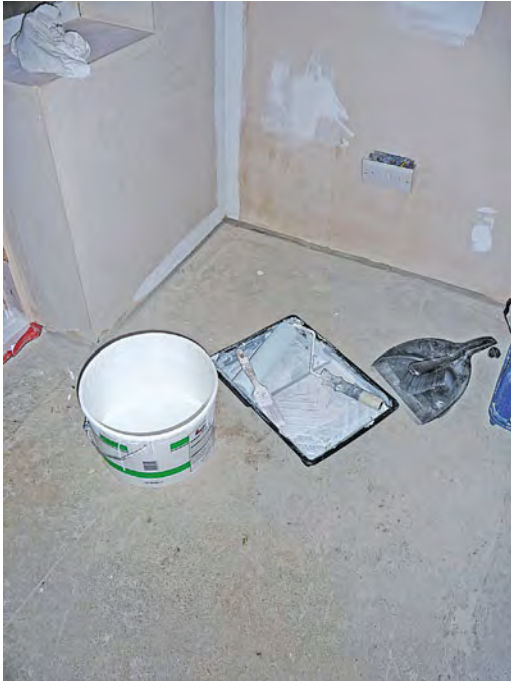
Vinyl-based emulsion paints are popular, cost effective and easy to use. Rollers and brushes are the most common means of application.
