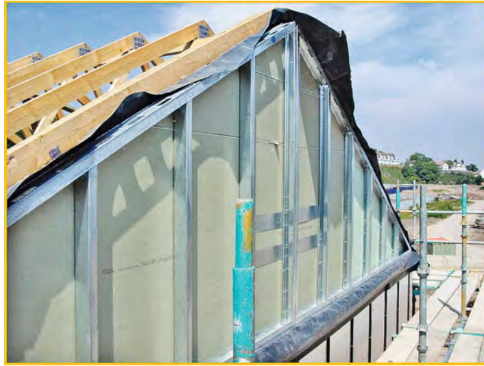
Part of the separating wall (party wall) can be seen here.
