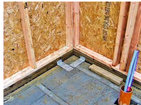
This photograph shows the clips which can be used to secure the sole plate. In this example the floor is pre-cast beams and blocks.
