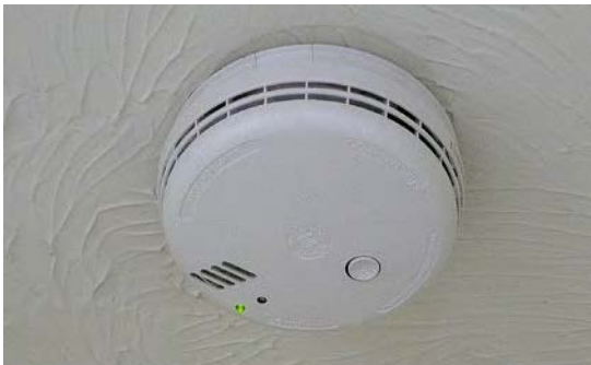
A typical smoke detector: the button is for the occupier to test the system to ensure that it is working.
