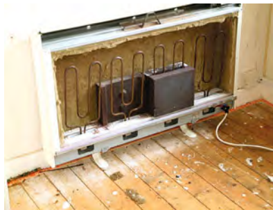
A storage radiator from the 1970s showing the heating elements and some of the clay bricks.
