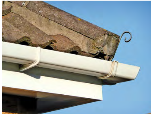
Bonnet hip tiles with a slip tile, but no mortar or hip iron in place beneath the bottom hip tile. On the right, mortar and a hip iron are in place.
