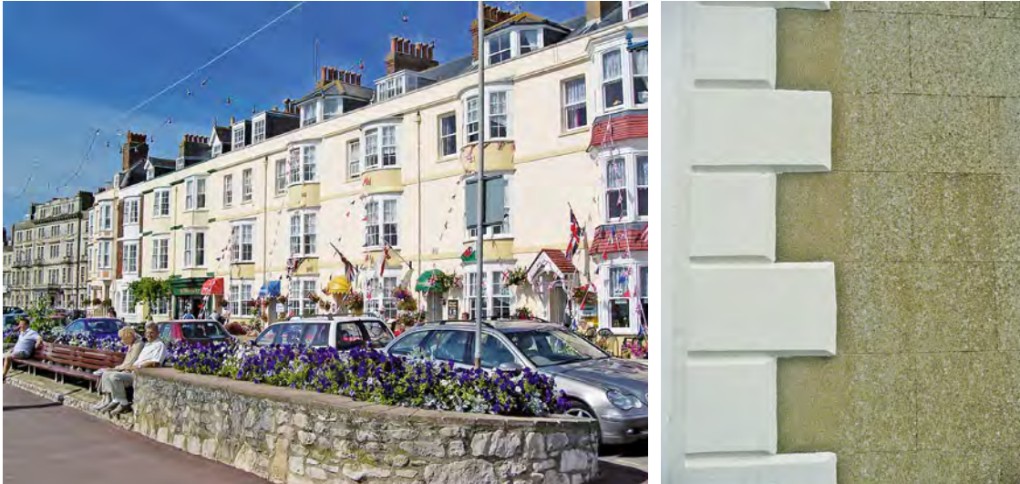
During the Regency period (early 1800s) it became fashionable to render buildings. The render usually hides rough and ready brickwork or rubble. Brighton and Cheltenham are two good examples of Regency towns. Fine lines were sometimes incised into the render to give the appearance of more expensive stonework. This technique is still common today.
