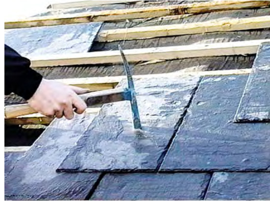
Note: The zax has a pointed end for forming the hole and a hammer end for fixing the nail.
