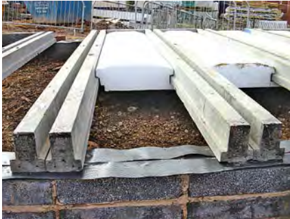
Pre-cast beams span between loadbearing walls.
