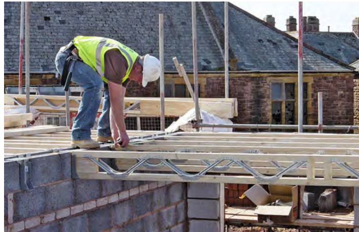
Metal web joists being fixed on joist hangers.
