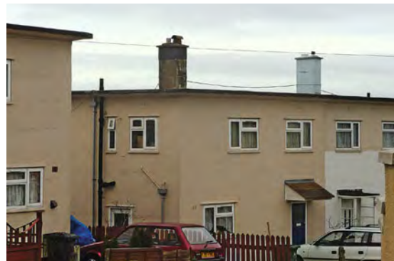
Post-war houses (1960s) constructed with flat roofs.
