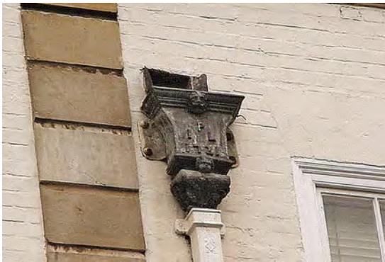
Hopper head to a parapet wall on a Georgian building.
