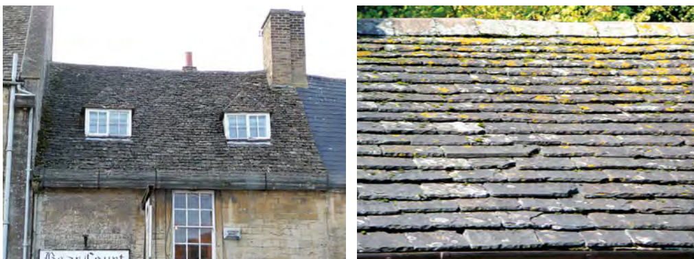
Stone slates can be found in many rural areas. For example, limestone slates, such as those above left, are found in the Cotswolds, while the sandstone slates on the right can be seen in parts of South Wales. Note the considerable thickness of each slate and the diminishing size as the coursing increases in height.
