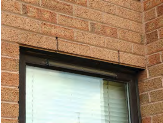
Weepholes above a window.
