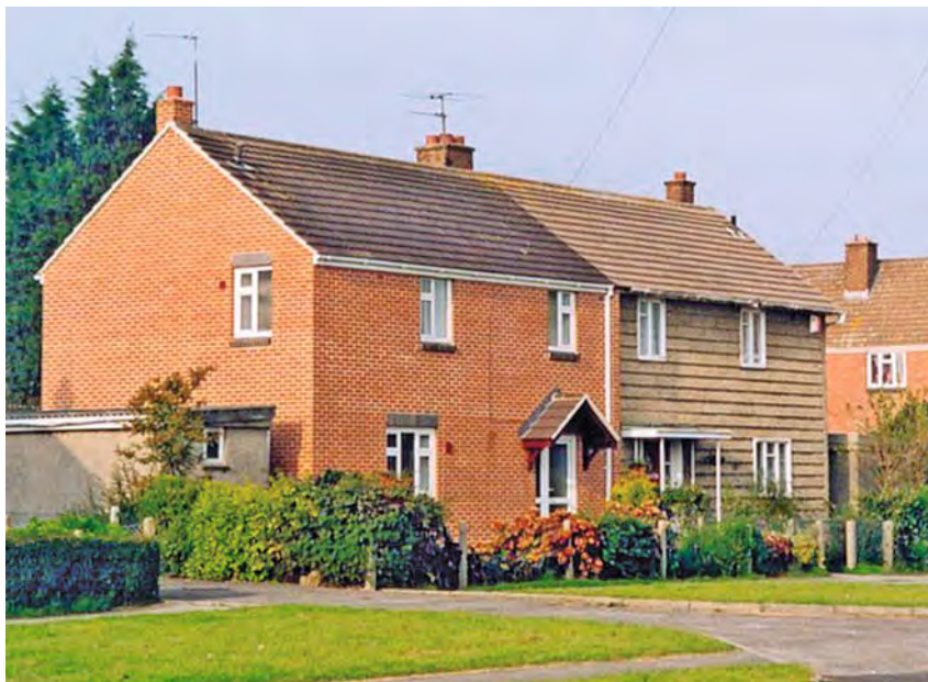
A pair of Airey system-built houses – the left-hand house has been reconstructed with a brick cavity wall, while the right-hand house is as originally built with pre-cast horizontal concrete panels and columns. Some 26,000 units were built.
