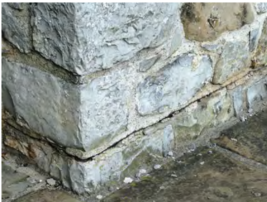
Bitumen felt DPC (in a stone wall).
