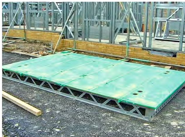
This photograph shows a floor 'cassette'. Three or four of these are typically required for each dwelling. Notice the pre-formed holes for services.
