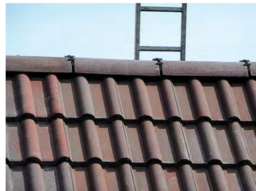
A dry ridge system (over double Roman clay tiles).
