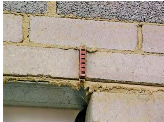
Weepholes above a window.
