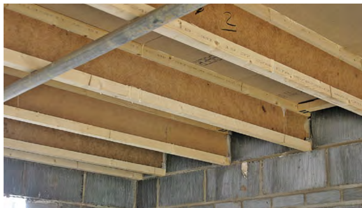
I-joist built into wall.
