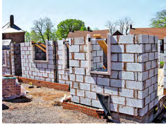
Window sub-frames in the process of being built in.
