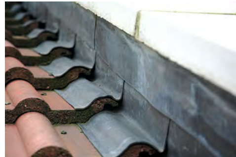
Each tile has a soaker fitted and all are covered by a cover flashing (in this case, it has not been stepped)
