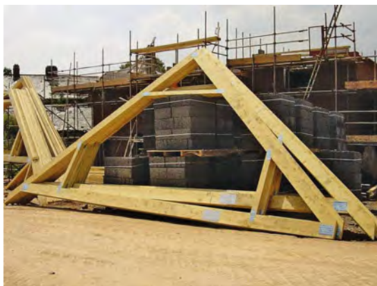
An attic truss.
