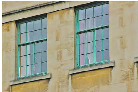
Ungalvanised steel windows from the 1930s.
