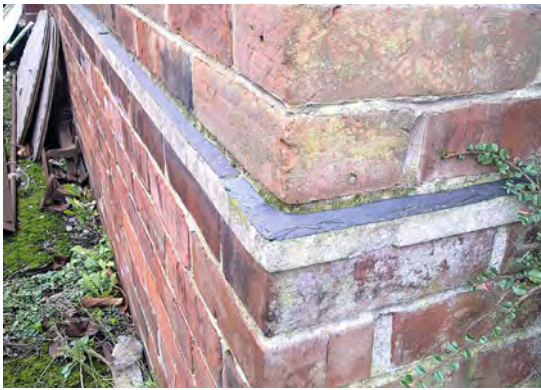
Slate DPC on a house from the early twentieth century.
