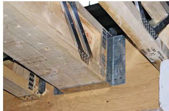
Web joists supported by hangers. Photograph courtesy of Truss Form (Midlands) Ltd.
