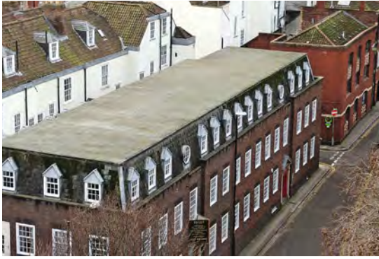
Built-up felt covered flat roofs (above and below).
