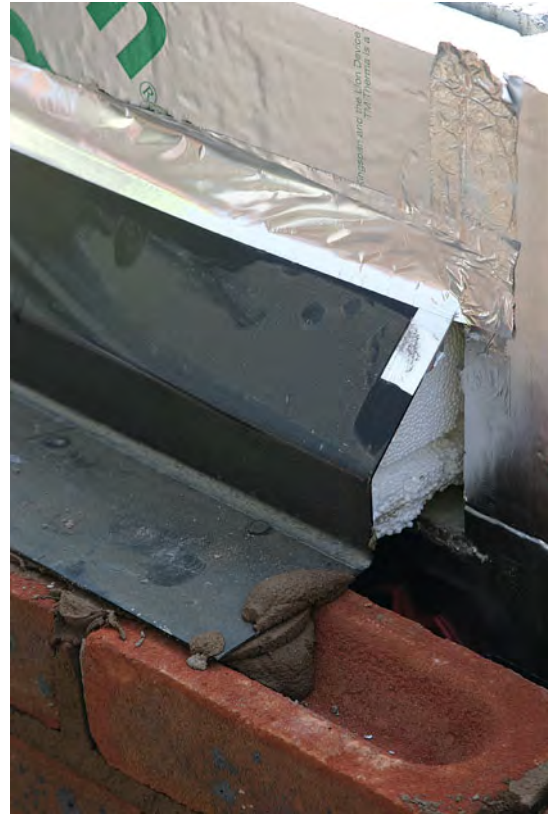
Note the thermal insulation to the lintel.
