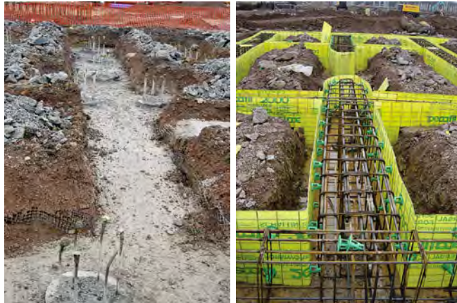
Plan showing pile layout and ground beam.
