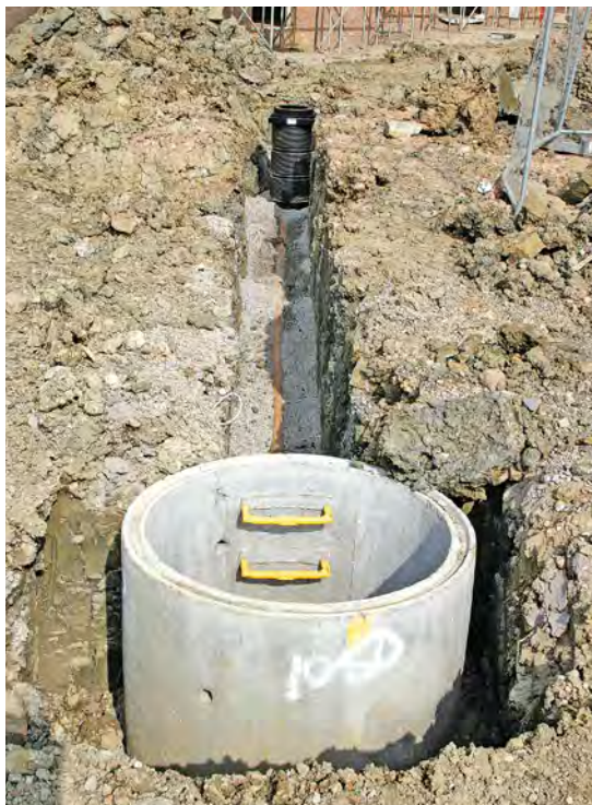
Manholes on new housing developments are usually constructed in pre-cast concrete, as shown in the two photographs above.
