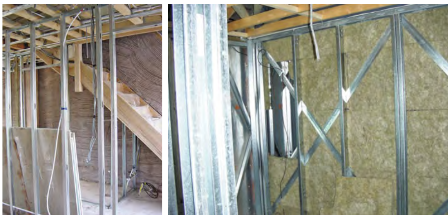
The diagram shows details of a typical steel framed system.
