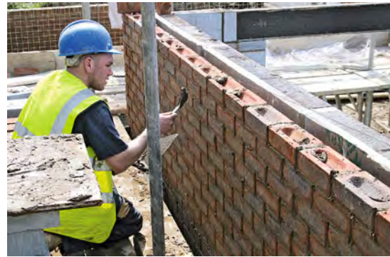
Brickwork in the process of being jointed.
