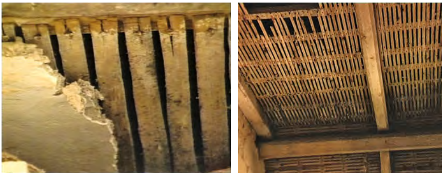
This was the most common method of forming ceilings until the 1950s. The timber laths form a mechanical key for the plaster. The first coat, the 'pricking up' coat, squeezes through the lath and forms the key. Two subsequent coats were required to provide a smooth, even finish.
