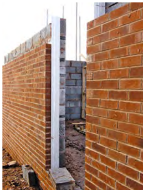
Modern extruded sections save the need to close the cavity with cut blocks.
