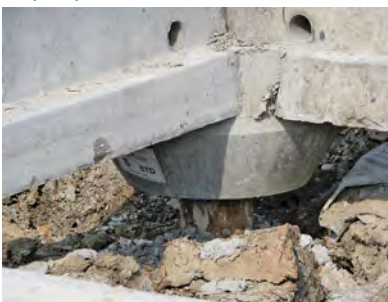
External and internal loadbearing walls require piles.
