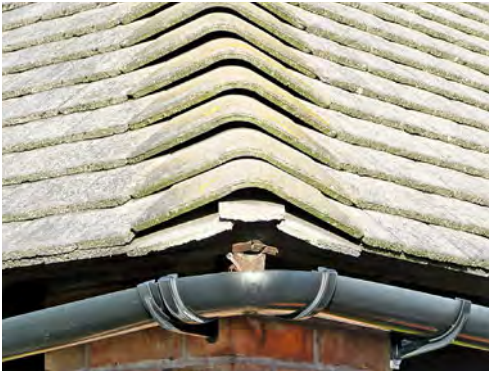
Bonnet hip tiles with a slip tile, but no mortar or hip iron in place beneath the bottom hip tile. On the right, mortar and a hip iron are in place.
