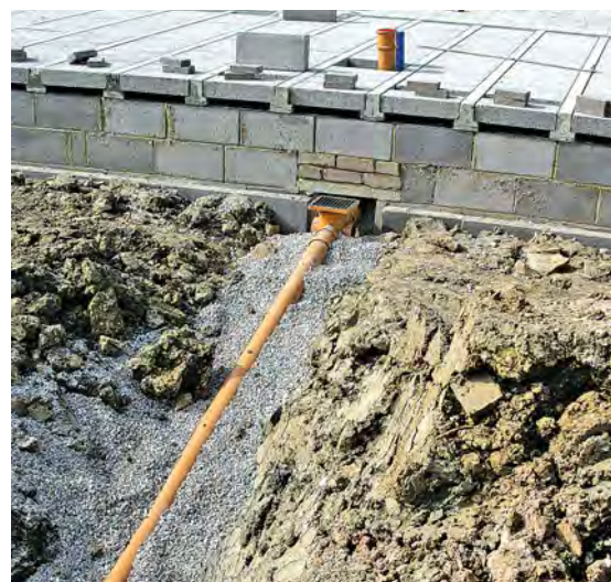
Bedding to drainage pipes.
