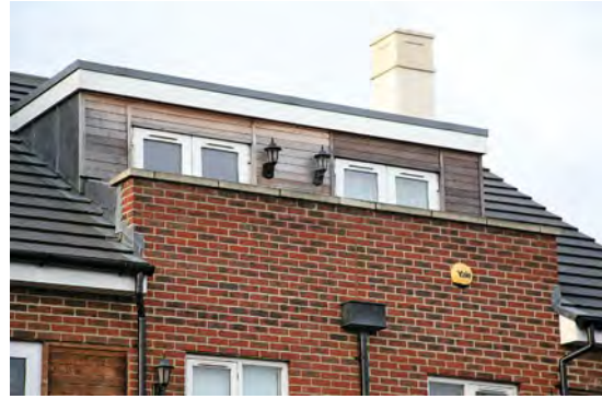
Parapet wall to the balcony of a new house.
