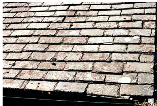
The laminated structure of slate can clearly be seen in the photograph above.
