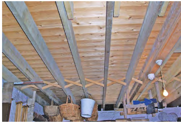
Strutting to a traditional cut joist upper floor.
