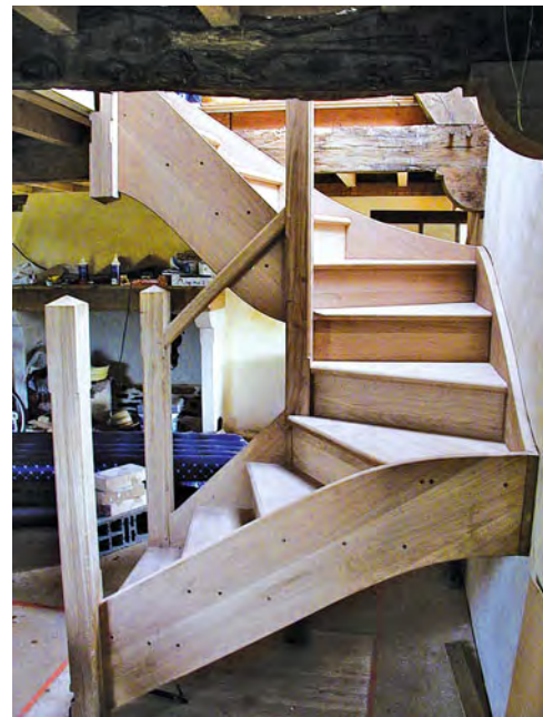
Some stairs consist entirely of winders. The strings (left photograph) are cut, shaped and grooved. The photograph on the right shows the assembled stairs. The balustrades will be fitted next.
