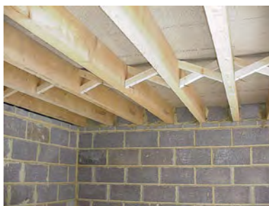
The photograph (left) shows strutting to a modern floor. The principle has not changed although stainless steel struts are sometimes used in place of their timber counterparts. If the strutting is to be effective, the floor structure needs to be braced against the adjacent wall(s). Traditionally, this was achieved by inserting folding wedges between the wall and the end joist.
