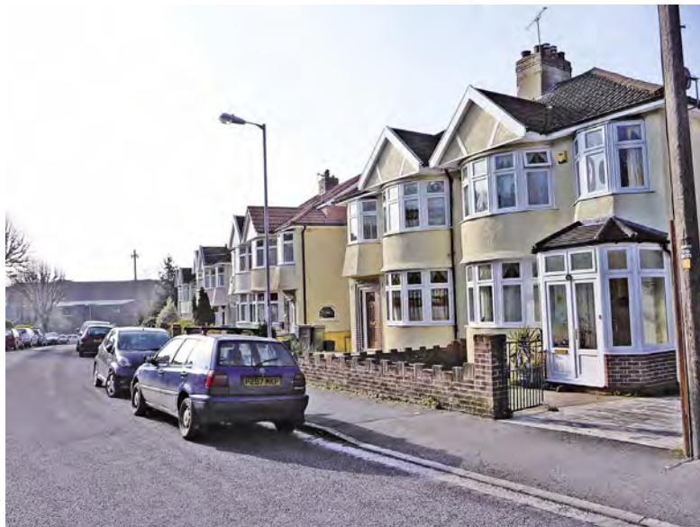
Interwar houses, from the 1920s and 1930s, often made use of roughcast render.
