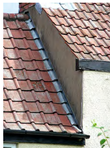
On the left are clay single Roman tiles, whilst those on the right are clay double Roman tiles.
