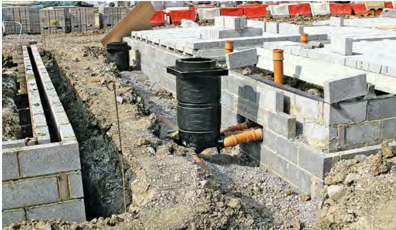
Drainpipes running through wall in gap formed with concrete lintel.
