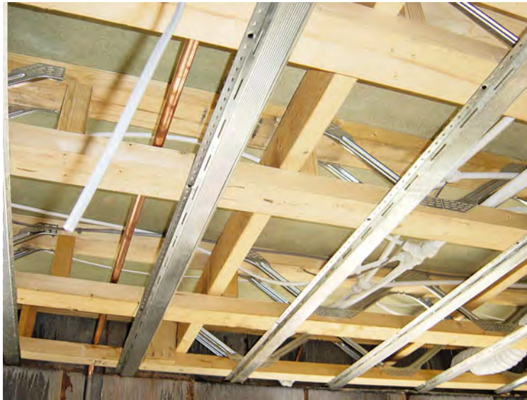
Services are easily run through the open web in metal web joists.
