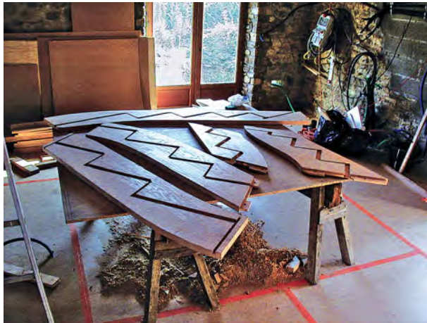
Some stairs consist entirely of winders. The strings (left photograph) are cut, shaped and grooved. The photograph on the right shows the assembled stairs. The balustrades will be fitted next.
