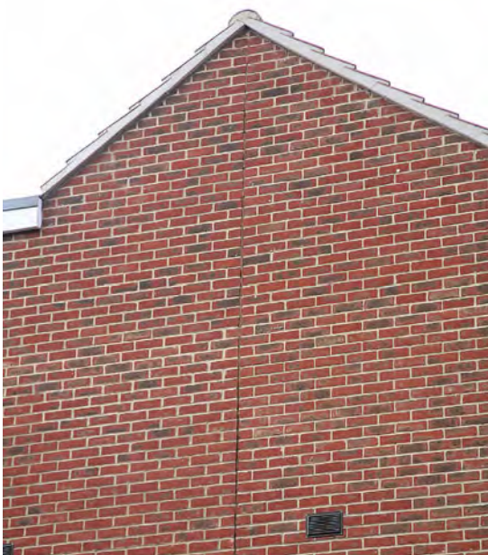
(left and right above) The vertical line stretching from the ridge downwards in this gable wall is a movement joint.
