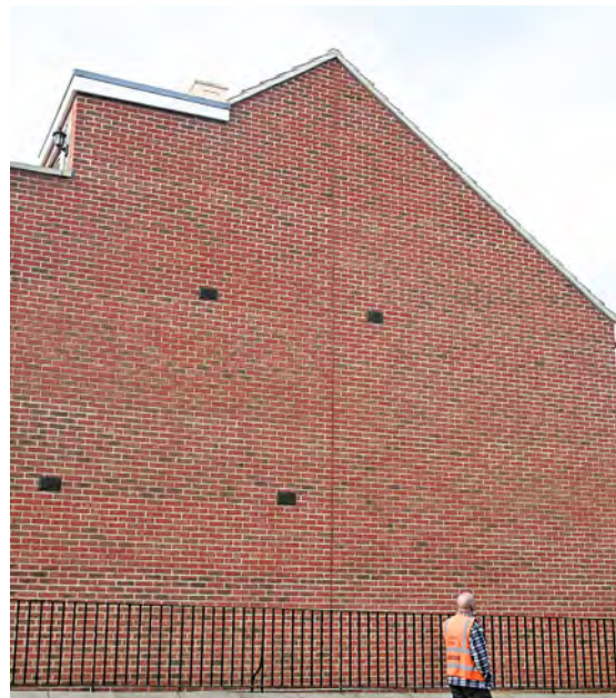
Detail of movement joint to gable wall shown below. Note the joint stops at DPC level.
