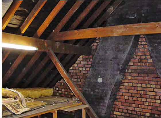
The purlins are built into the party walls (this is a terraced house). The purlin should not run completely through the party wall. This reduces the possibility of fire spread. A collar, just above the struts, keeps the roof rigid in high winds. The rendered brickwork (to prevent smoke leakage) on the party wall shows how the flues are 'gathered' below the chimney stack.
