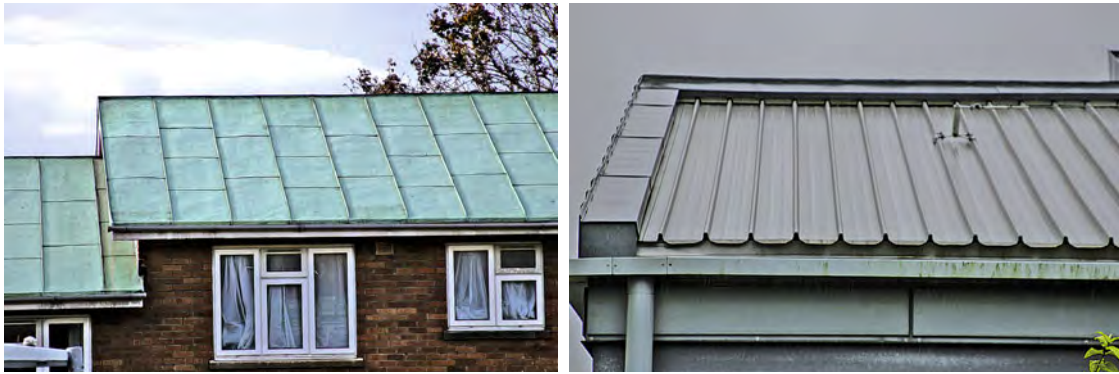
These two photographs show different types of standing seams secured with secret fixings. On the left is an older copper roof clearly showing the individual sheets, while on the right is a recently installed profiled steel roof.
