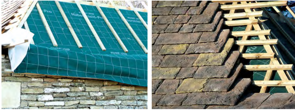
Microporous underlays (breather membranes) are very popular. In the left-hand photograph a breather membrane has been secured with counter-battens, while the right-hand photograph shows a further stage of the roofing process – stone slates have been fixed to battens over the counter-battens with breather membrane beneath.
