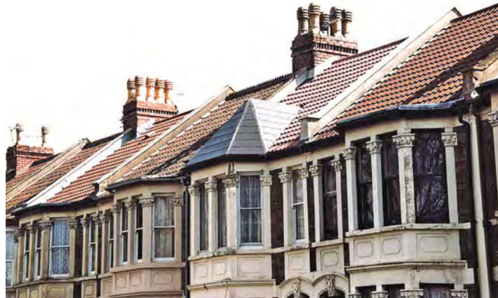
Note how the party walls are extended upwards by means of parapet walls to prevent fire spread between the roofs of this terrace of Victorian houses.
