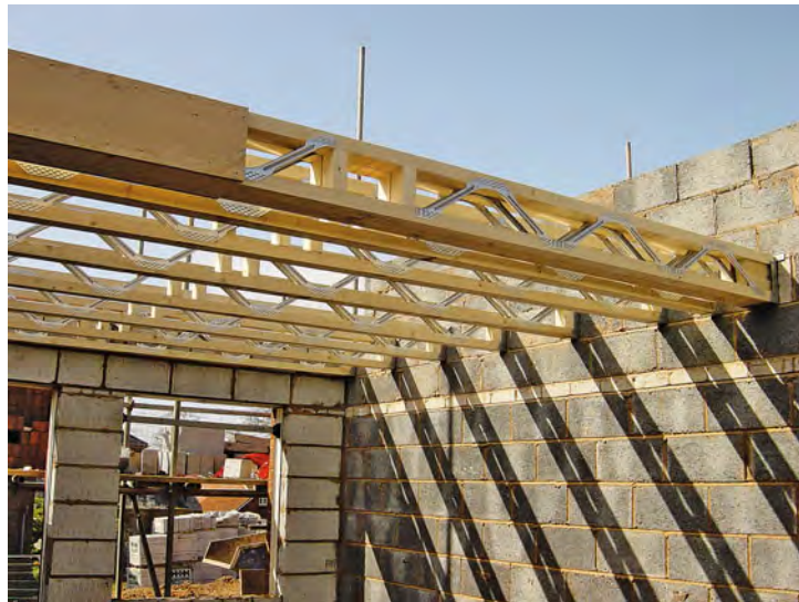
Metal web joists.
