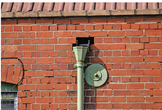
Hopper head to a parapet wall gutter.
