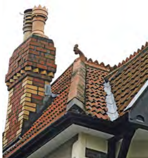
The manufacturers of plain and other tiles (both concrete and clay) produce a number of ornamental tiles and other decorative features, such as this finial forming the top of a hip.
