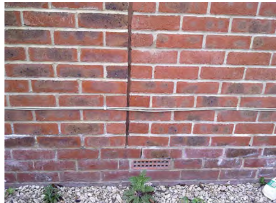
Detail of movement joint to gable wall shown below. Note the joint stops at DPC level.
