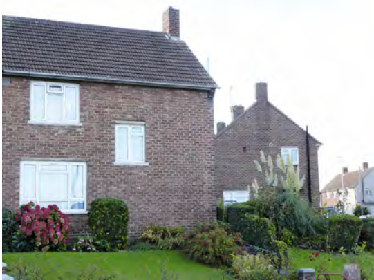
These three images are of 1950s houses with concrete lintels.
