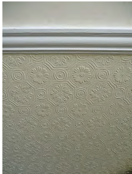
A modern reproduction Anaglypta paper beneath a dado rail. This wallpaper is embossed and designed to be decorated. In this particular case, as it is located in a hallway, a water-based eggshell paint has been selected for its hardwearing and durable qualities.
