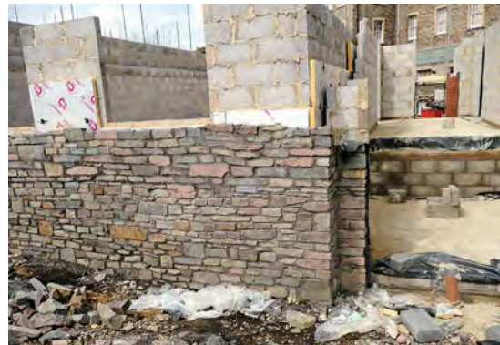
Rubble stonework being used on a new development in a conservation area.
