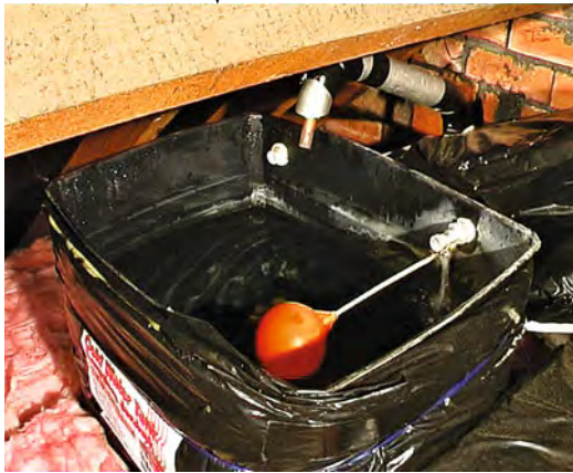
Lid and insulation removed to show water and ball float.
