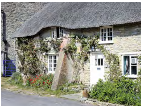
Thatched roofs should have at least a 50° pitch to aid water run-off and need a substantial overhang at the eaves to throw the water clear of the walls.
