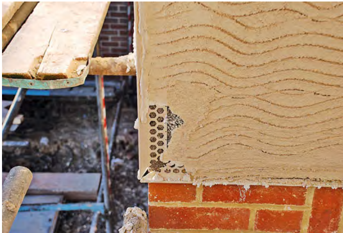
A plastic 'bellcast' bead fixed just above DPC level, together with plastic edge beads at the quoin. These are plugged and screwed to the wall prior to the application of the render. Plastic is increasingly being used for reasons of both cost and durability. The drawing shows an edge stop-bead, which are also frequently plastic rather than galvanised steel.
