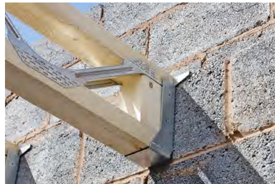
Web joist on hanger.
