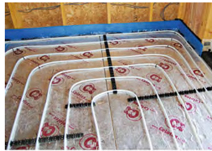
Within the building the heat from a heat pump is often distributed via an under floor heating coil.
