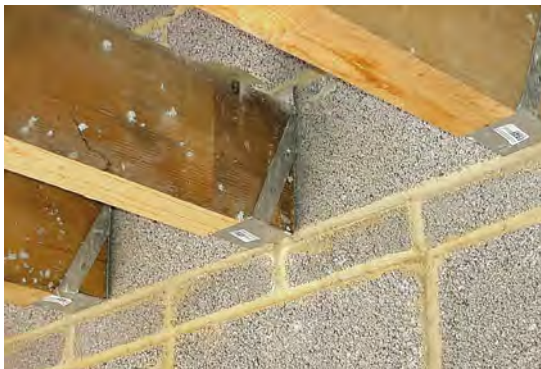
Joist hangers supporting solid timber joist.
