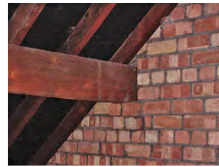
The purlins are built into the party walls (this is a terraced house). The purlin should not run completely through the party wall. This reduces the possibility of fire spread. A collar, just above the struts, keeps the roof rigid in high winds. The rendered brickwork (to prevent smoke leakage) on the party wall shows how the flues are 'gathered' below the chimney stack.
