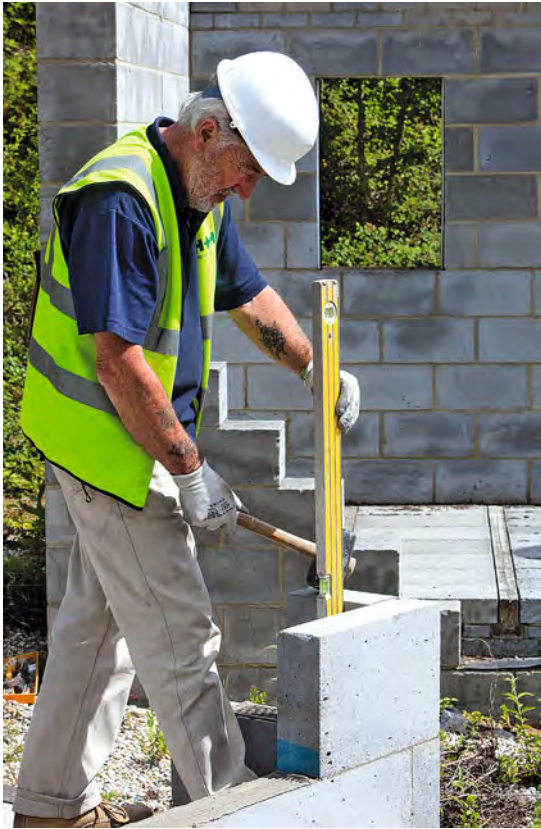
(left and above) Blockwork wall under construction using a thin joint system. Photographs courtesy of H+H UK Ltd.
