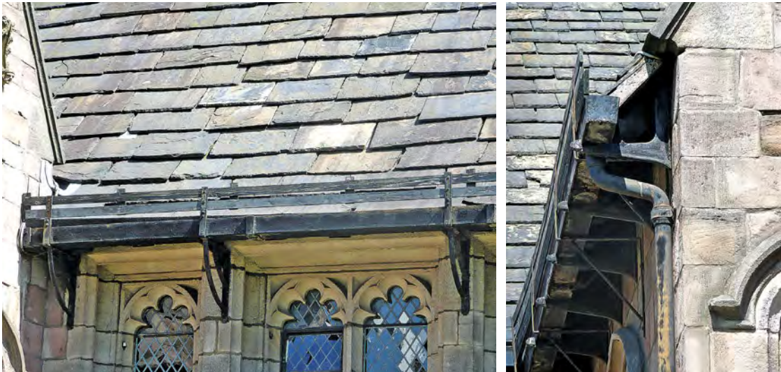
Lead box gutter on a seventeenth-century house.
