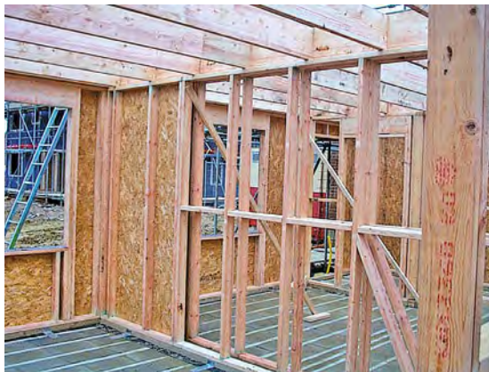
The detailing of the party (separating) walls will vary from one design to another, but must recognise the need for adequate sound and fire resistance. These panels are partly sheathed to improve racking resistance across the frame.
