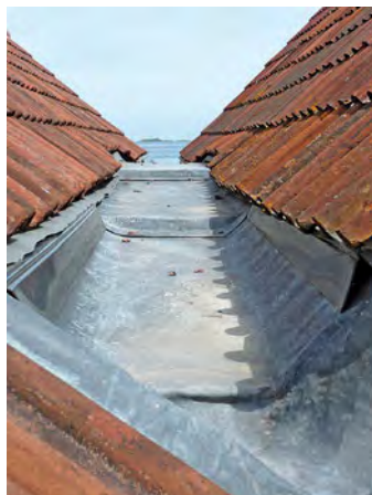
The left-hand valley is lead and the individual bays and steps can be seen. The right-hand one is made from glass fibre and is laid over the felt. When the tiles have been cut to the correct profile, they are bedded and pointed in mortar. This is not a skilled job (unlike leadwork) and it is relatively cheap. However, its durability is, as yet, undetermined.
