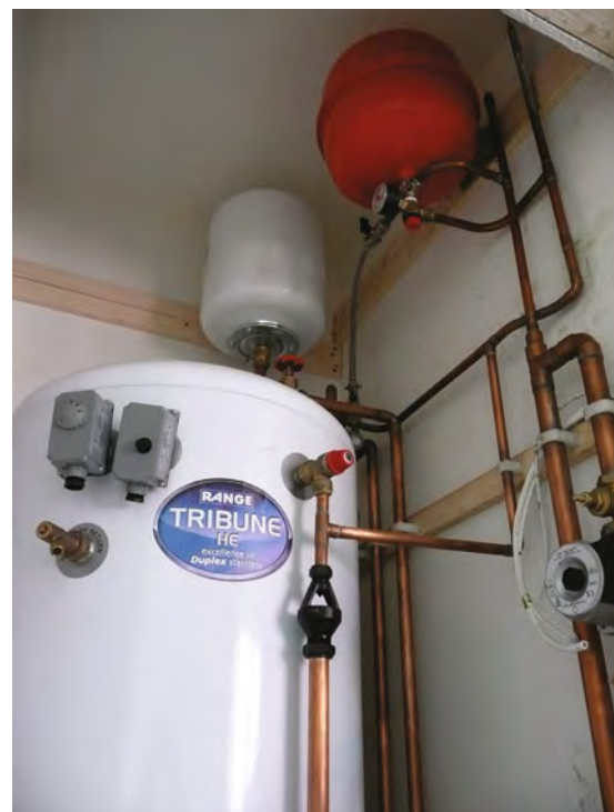
An unvented cylinder in situ.
