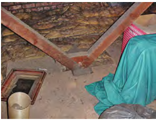
This roof dates from the 1950s and is a good example of a strutted purlin roof. The purlins are supported by two sets of angled struts bearing on a loadbearing wall (see below).
