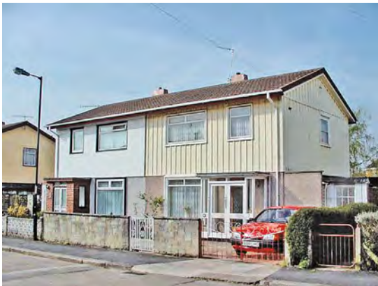
A pair of BISF houses, the one on the left has been re-clad and had a modern porch added, the appearance of the one on the right is more or less as-built.
