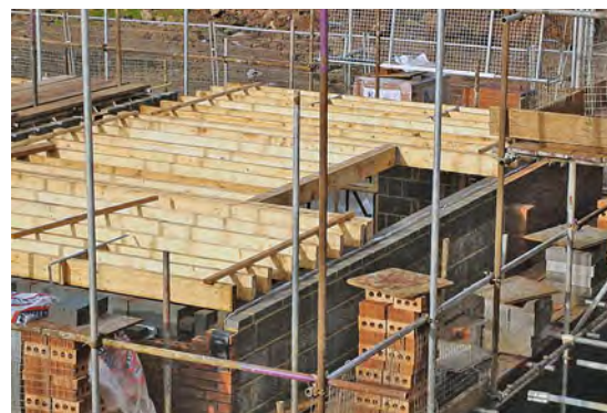
Staircase opening in a traditional cut floor.
