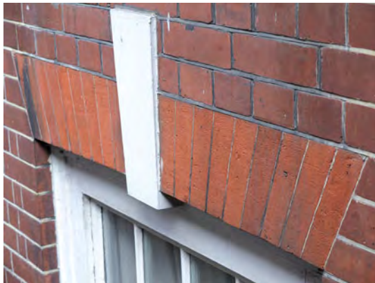
Gauged arch with rubbed bricks.
