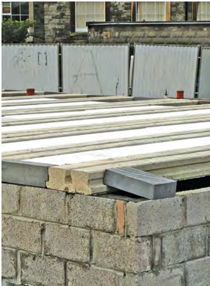
(left and above) Polystyrene blocks placed between pre-cast concrete beams.
