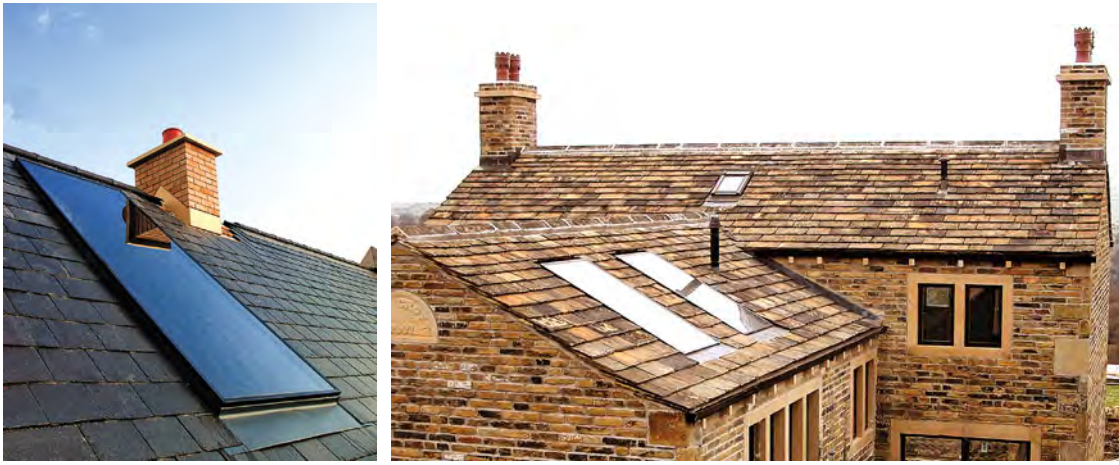
Flat plate collectors. Photographs courtesy of Viridian Solar.
