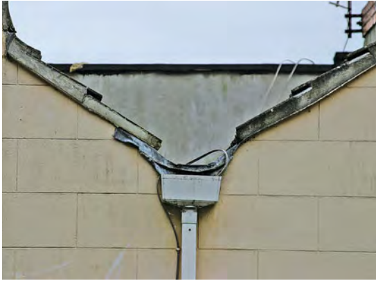
Hopper head to a Victorian butterfly roof.
