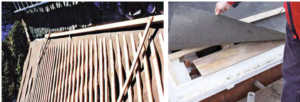
Two examples of reinforced bitumen felt. On the left, a felted and battened roof is ready for slating. On the right, a felted and battened roof is ready for interlocking tiles to be laid. The felt has been lifted back to reveal the tilting fillet at the eaves.
