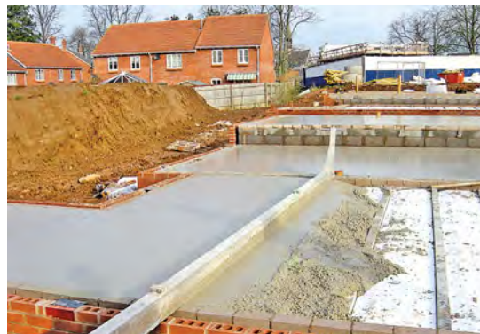
In situ concrete topping placed over beams and polystyrene blocks.
