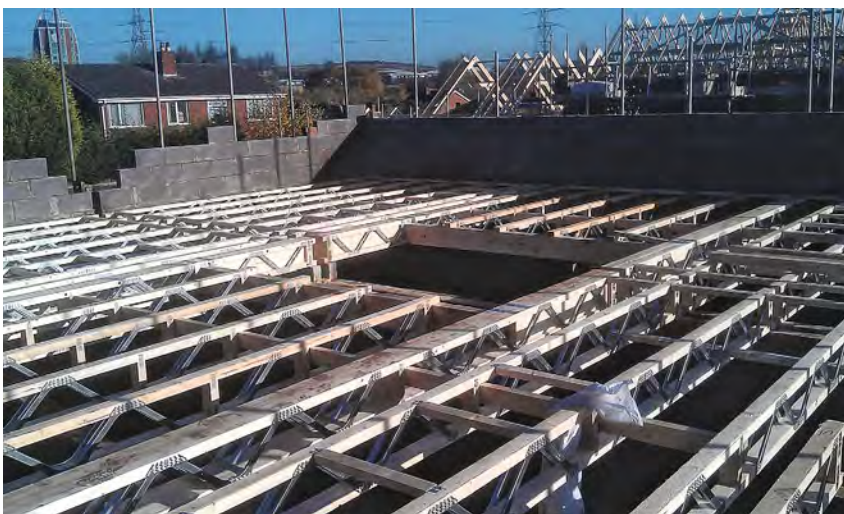
(left and below) Staircase opening being formed with web joists. Photographs courtesy of Truss Form (Midlands) Ltd.
