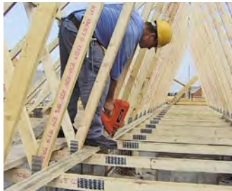
Horizontal brace (100 x 25mm) being fixed in position with a nail gun.
