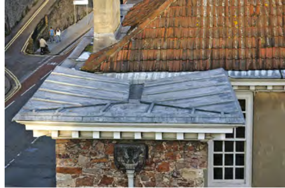
Lead flat roof on a seventeenth century building.
