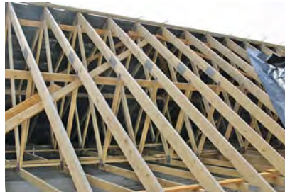
The diagonal brace keeps the roof structure rigid. The pattern of bracing depends on the roof size.
