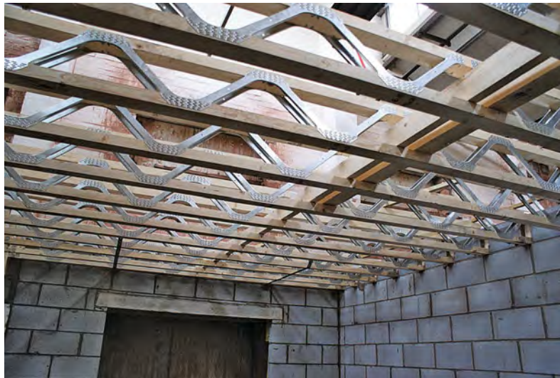
The image above shows the strongback running at right angles through the metal web joists. It is usually fixed to a vertical timber block that has been inserted in each joist and therefore all the joists are connected and stiffened. Image courtesy of Truss Form (Midlands) Ltd.
