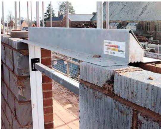
Insulated lintel from a house built in 2005.
