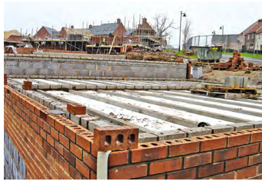
(left and above) Polystyrene blocks placed between pre-cast concrete beams.
