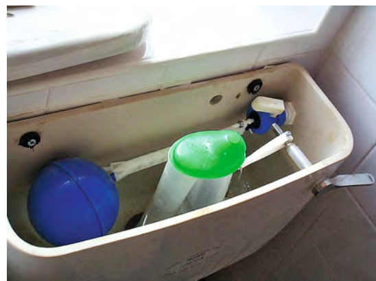
A typical ball valve used in a modern WC. The float controls the water level. The siphon tube is in the centre of the cistern. An overflow or warning pipe (just out of picture on the left) allows water to escape if the float or ball valve becomes defective.
