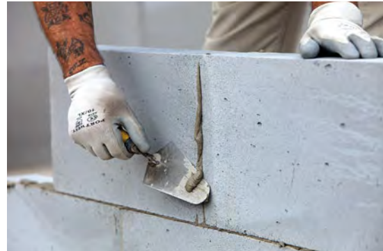
(left and above) Blockwork wall under construction using a thin joint system. Photographs courtesy of H+H UK Ltd.
