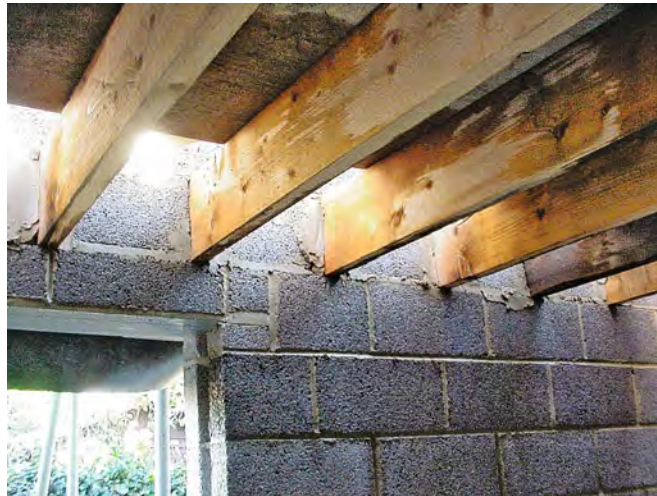
Joists can be built into the wall as long as any gaps around the joists are sealed to prevent air leakage.
