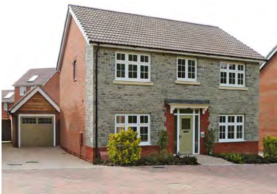
Rubble stonework on the front elevation of a new house – presumably to introduce variety into the estate.
