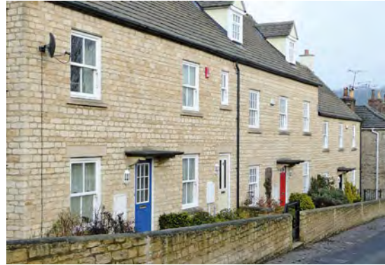
Stonework on a new development – in this case used to reflect the local building materials.
