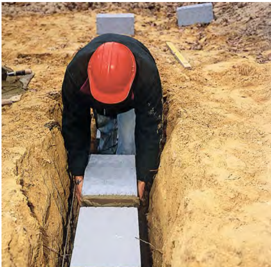
The two images above show aerated trench blocks being laid. Photograph courtesy of H+H UK Ltd.
