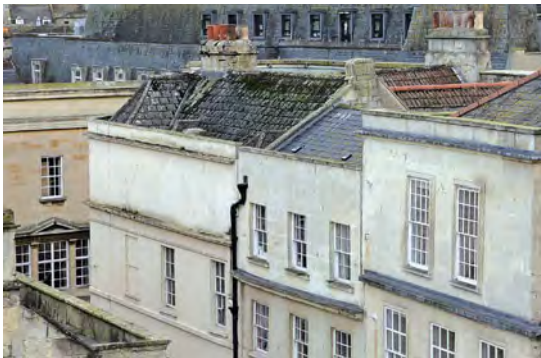
(above and right) Georgian houses with parapet walls.
