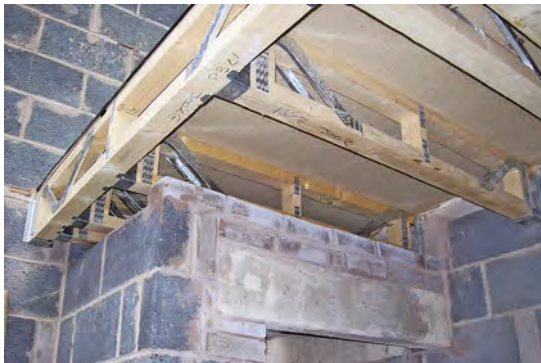
Metal web joists using hangers on block wall and on joists where attached to each other. Photograph courtesy of Truss Form (Midlands) Ltd.
