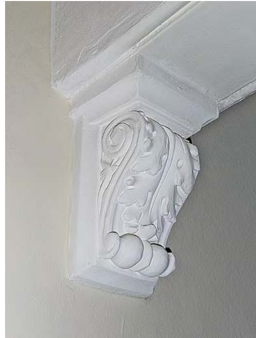
Plaster of Paris console bracket used for decorative effect.
