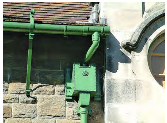
Hopper head to an eaves gutter.
