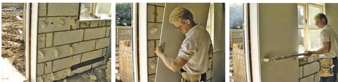
Typical pattern of adhesive dabs and adhesive band behind skirting. Sequence of the images below dry-lining being applied to a wall.
