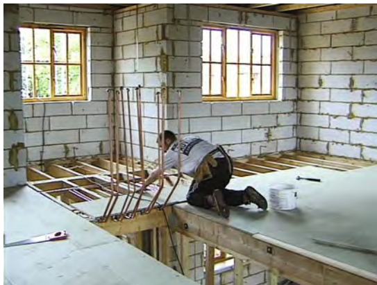
Chipboard flooring being fixed (glued) in place.
