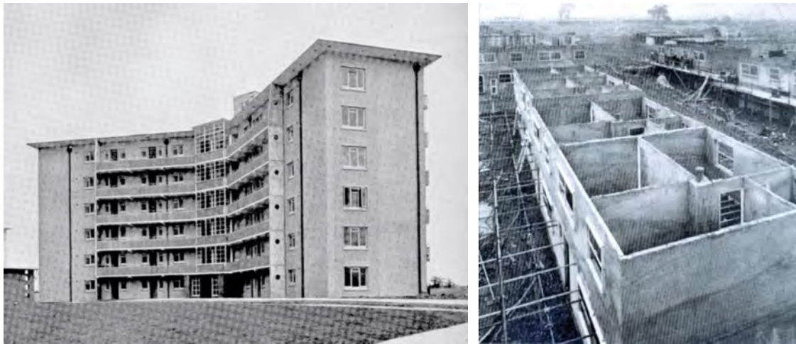
Typical no-fines high-rise homes can be seen in the left-hand photograph. In the 1960s, a number of other companies developed their own in-situ systems. The photograph on the right shows a low-rise system which was based on aerated lightweight concrete. Apparently, the concrete finish was so good that the internal walls could be papered without the need for a plaster finish. The shells were usually clad in facing brick.
