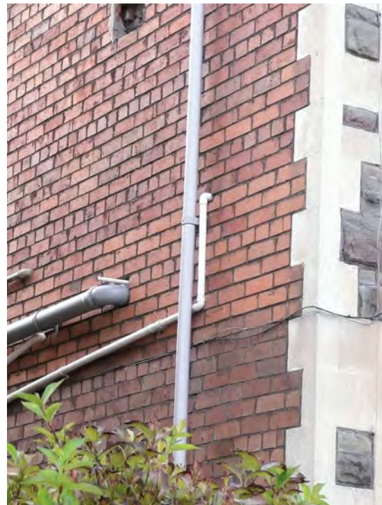
English garden wall bond to the side of a Victorian house with a rubble stone elevation.
