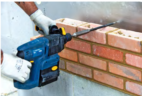
The two images above show wall ties being mechanically fixed into the thin-joint blockwork in line with the bed joint of the exterior skin of brick. Photographs courtesy of H+H UK Ltd.
