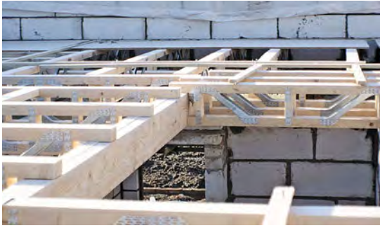
Stair opening formed in a metal web joist floor.
