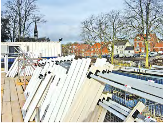
A range of sub-frames awaiting placement on site. Each one is designed to suit a specific window size, enabling it to be effectively fixed within the sub-frame once the masonry construction is completed.
