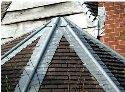
In slated and plain tiled roofs, lead is often used for hips and ridges.
