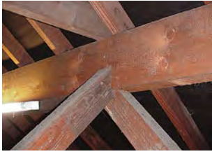
This roof dates from the 1950s and is a good example of a strutted purlin roof. The purlins are supported by two sets of angled struts bearing on a loadbearing wall (see below).
