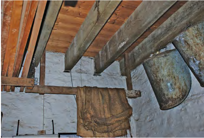
Upper floor joists built into an external wall.
