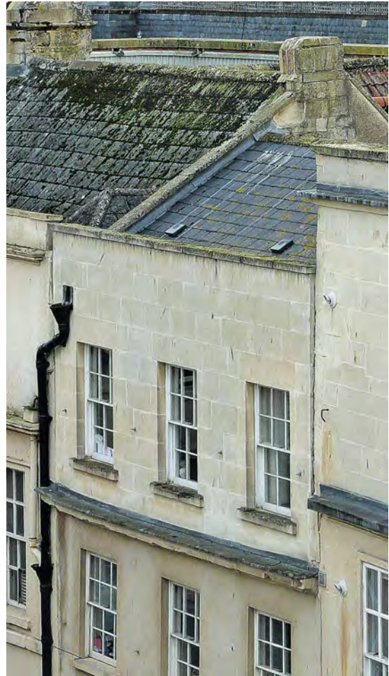
Hopper head to a parapet wall on a Georgian building.
