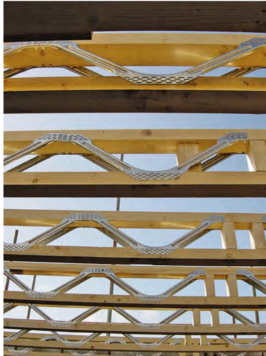
Metal web joists.
