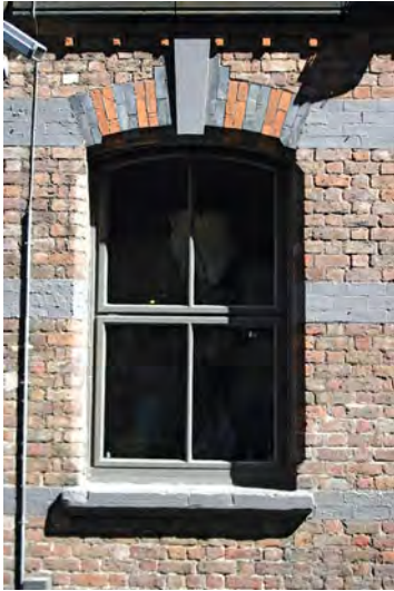
Segmental arch (i.e. it is a segment of a circle).
