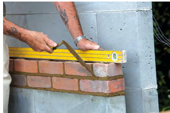
This image shows reinforcement mesh in the horizontal joint of the blockwork. Photograph courtesy of H+H UK Ltd.
