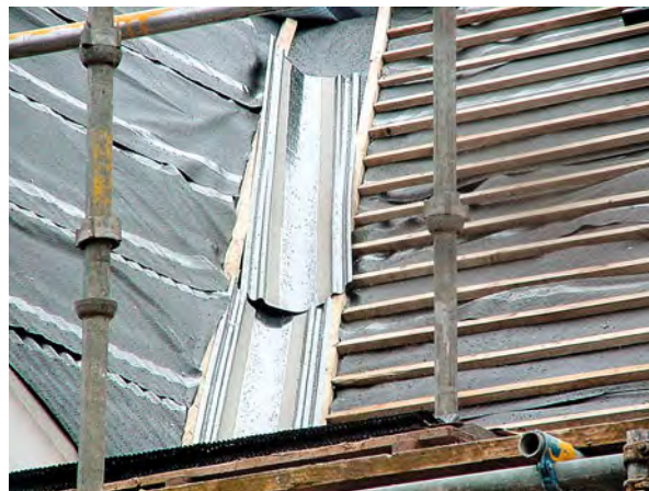
The left-hand valley is lead and the individual bays and steps can be seen. The right-hand one is made from glass fibre and is laid over the felt. When the tiles have been cut to the correct profile, they are bedded and pointed in mortar. This is not a skilled job (unlike leadwork) and it is relatively cheap. However, its durability is, as yet, undetermined.
