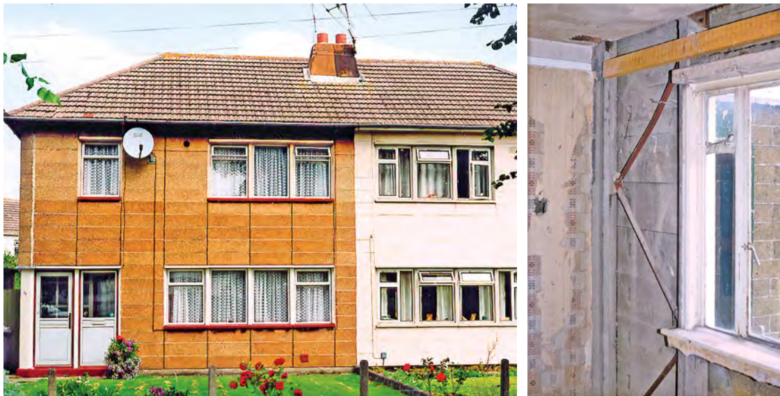
These two photographs show a Unity system-built house. Some 15,000 of these were erected, mostly in the 1950s. They comprised pre-cast horizontal concrete panels supported on pre-cast columns with steel bracing to prevent racking.
