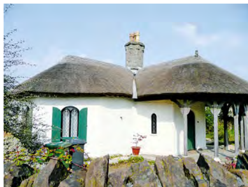
Thatched roofs should have at least a 50° pitch to aid water run-off and need a substantial overhang at the eaves to throw the water clear of the walls.
