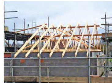
The diagonal brace keeps the roof structure rigid. The pattern of bracing depends on the roof size.
