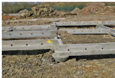
Typical pile centres are 2.4 to 3.0 metres.
