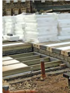
Polystyrene blocks waiting to be laid between pre-cast beams.
