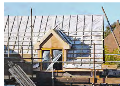
A roof in the process of battening and counter-battening.
