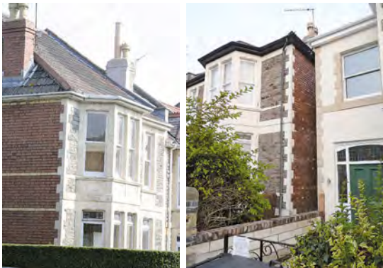
Brick side wall on a stone-fronted Victorian house.
