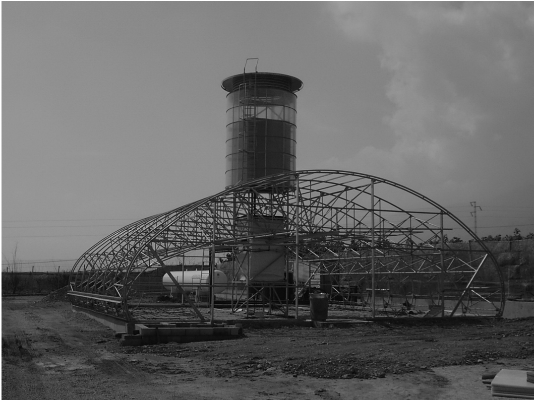
FIGURE 9.3 Watery greenhouse under construction (Almería, Spain). In the middle, the heat exchanger tower, harvesting heat during the day and releasing heat during the night. (Courtesy of Gerrit van Straten.)
