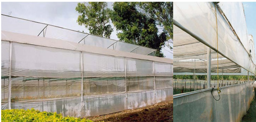
Fig. 9.8 Ropes and plastic-covered steel ropes as holder for the rollup vent against the structure
