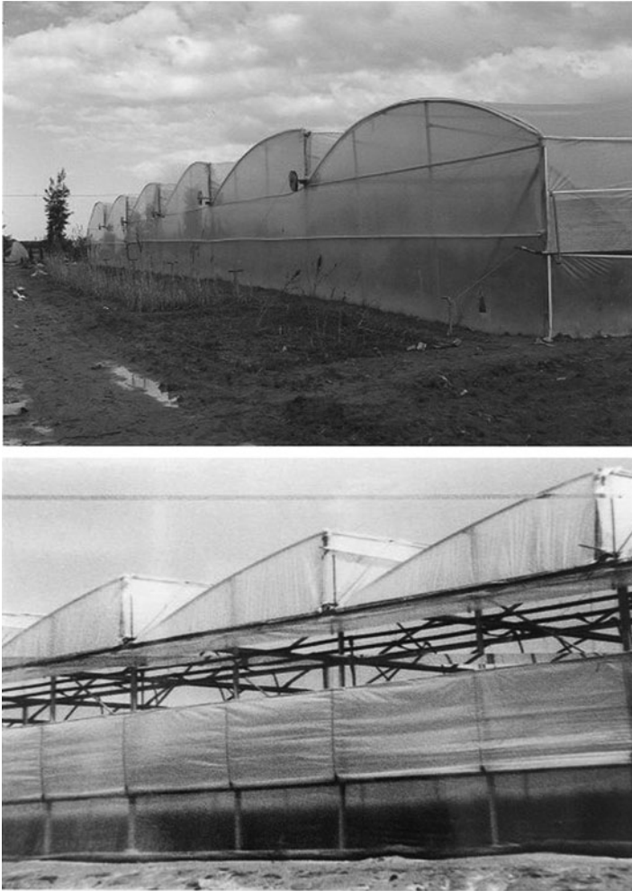
Fig. 5.50 Shed roof with roll-up ventilation at vertical ridge in Israel and Tunisia
