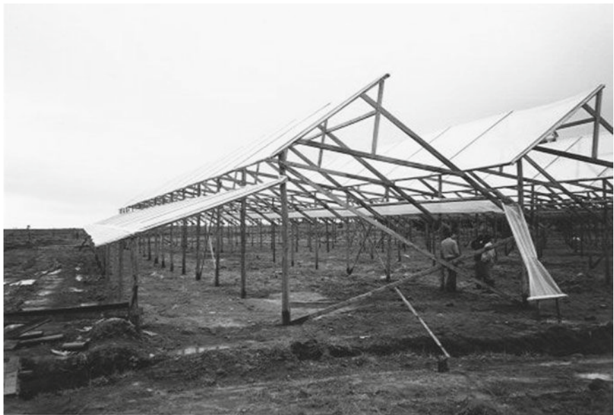
Fig. 5.35 Wooden structure from Kenya: 6.4 m ridge height, high volume and a canopy for rain protection on the weather side. The plastic film gutter is not advisable because of getting water pockets. The canopy at the side wall against sloping rain fall is highly recommendable
