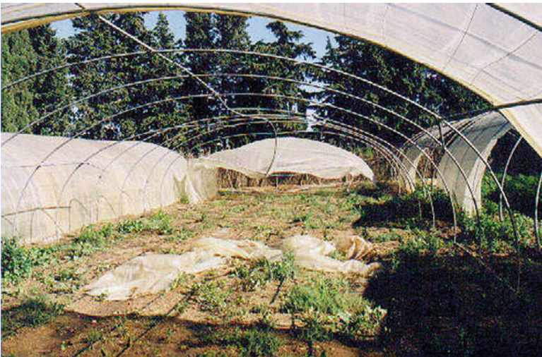
Fig. 4.1 Too weak tunnel structure damaged by wind
