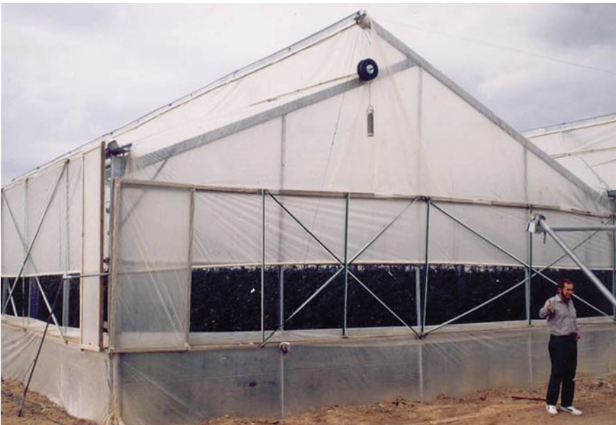
Fig. 9.16 Vertical ridge vents for a saddle-roof structure (Israel). Each roll up tube of the vents has a counterweight to pull and hold the roll-up tube down
