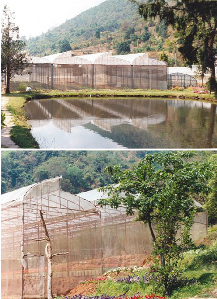
Fig. 5.38 Steel tube structure in Thailand with 5 m gutter height, ridge ventilation and nets against birds
