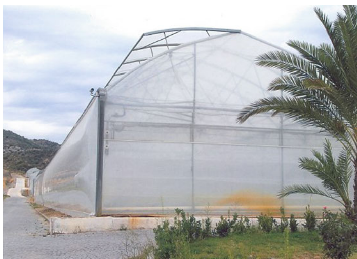
Fig. 5.54 Greenhouse with flap ventilation and high side wall in Turkey. The side wall is double-inflated
