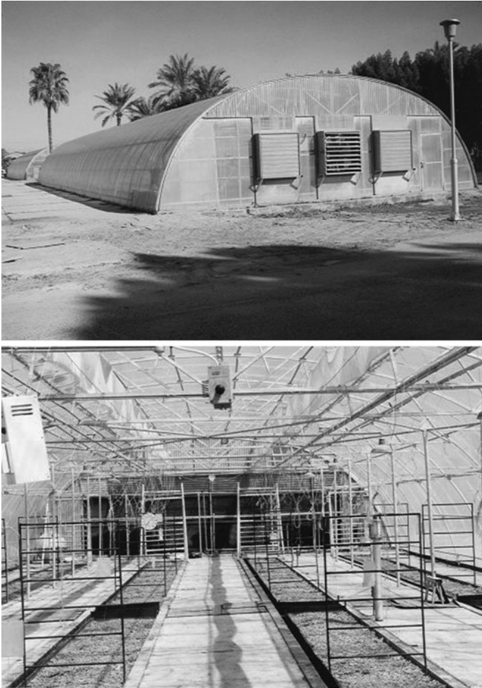
Fig. 5.60 Round-arched tunnel with fan and pad cooling at gable ends in Kuwait
