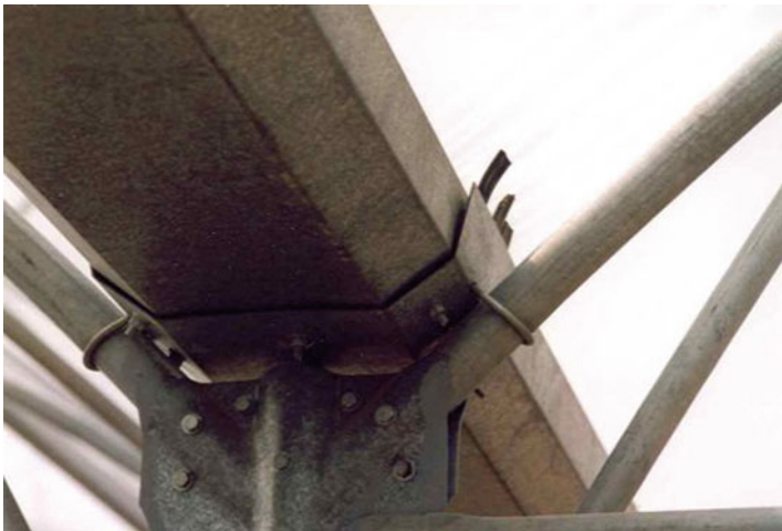
Fig. 8.12 All parts of the gutters have to be connected tightly by rubber tapes or by silicon to avoid dripping of rainwater
