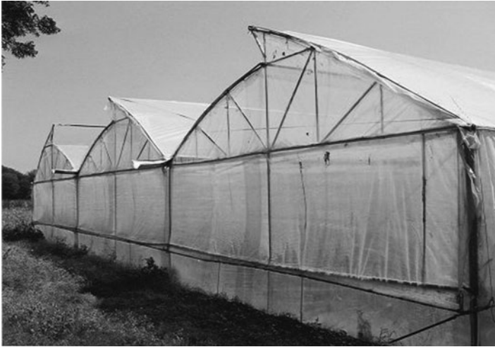
Fig. 5.39 Steel tube greenhouse on farm in Bangalore, India, covered with insect screens. The ridge vents at the gable ends have alternate opening directions for better ventilation efficiency
