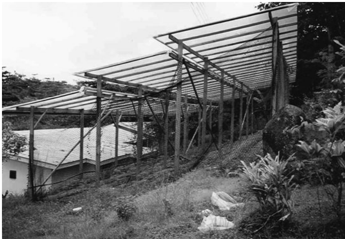
Fig. 5.77 Wooden structure for terrace shelter with nailed-on plastic film in the Seychelles
