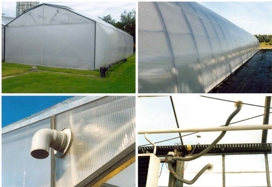
Fig. 8.24 Double-inflated plastic film is a recommendable method for stretching and stabilising the film as well as for saving energy
