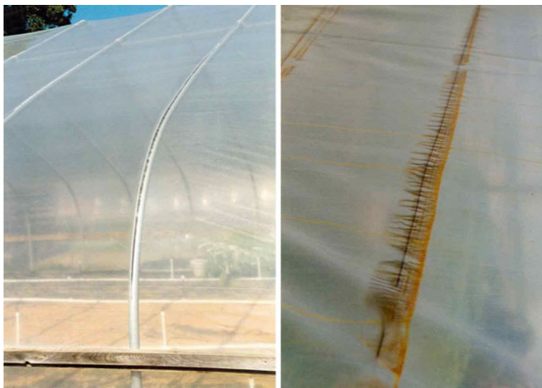
Fig. 8.26 Direct contact of the plastic film with steel tubes is a problem, in particular on hot days. The steel pipes can be heated up to 70°C by direct solar radiation. The plastic film can be destroyed earlier. In addition, the plastic film rubs on the steel tubes and the wires, and becomes black. This causes destruction of the film. It is recommendable to put some plastic tapes between film and steel pipes (Fig. 4.4). Another possibility is to paint the plastic white at the contact point to the steel pipes to prevent them from becoming too hot
