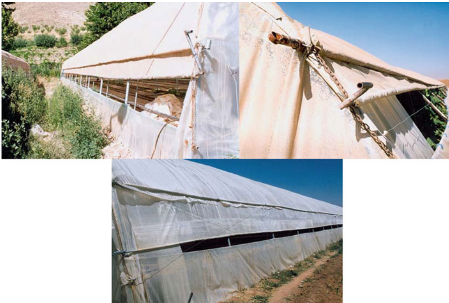
Fig. 9.10 Roll-up vents at side walls, 40–60 m long, where the plastic film of the roll-up side wall vent as well as the plastic film of the roof are fixed by rolling them up on one tube only. This method is very recommendable, because the roof plastic film can be stretched in summer
