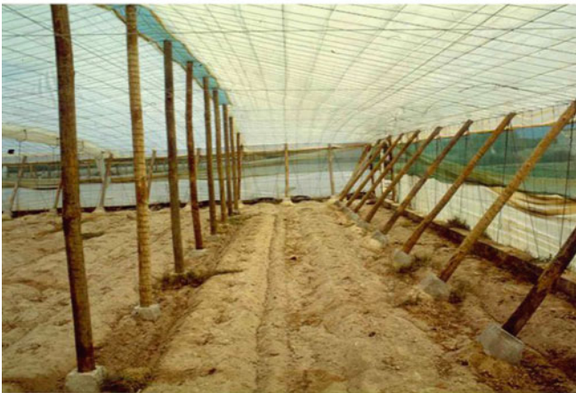
Fig. 5.68 Parral-type greenhouse in Almeria with flat roof
