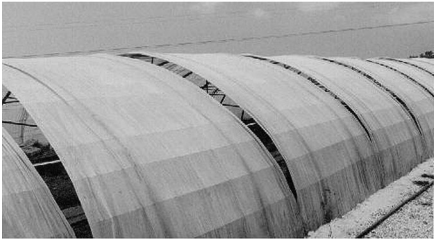
Fig. 5.10 Ventilation by parting the overlapping film over the whole arch is not sufficient
