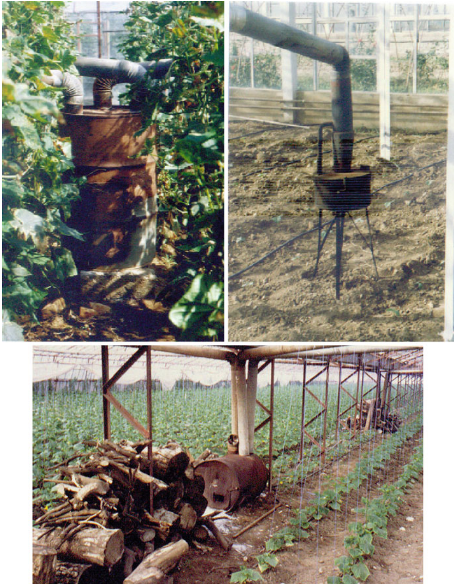
Fig. 12.2 Simple but not sufficient heating systems. These heating systems are still used in several countries
