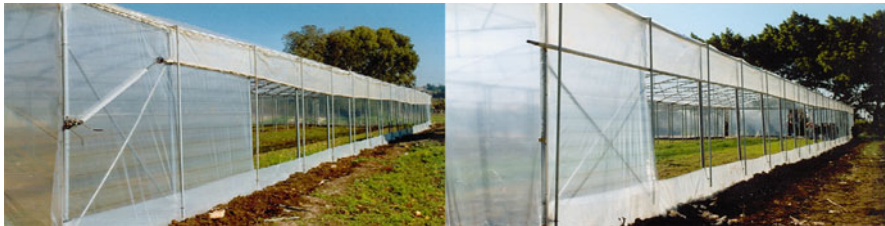
Fig. 9.4 Very well-designed roll-up ventilator with sufficient overlapping at the gable end to prevent leaks and destruction by wind forces. The horizontal roll-up tubes are nearly straight at a length of about 30 m
