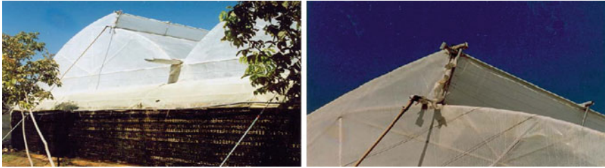
Fig. 9.15 Roll-up ventilation at the ridge of a round-arched greenhouse that has fan and pad cooling at the same time (Iran). The natural ventilation is for transit times, and has to be closed when fan and pad cooling is on
