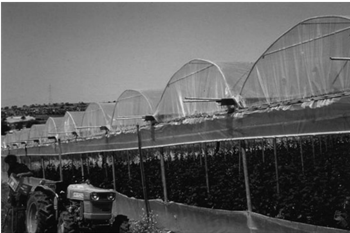
Fig. 5.48 Multi-span structure with roll-up ventilation in Cyprus
