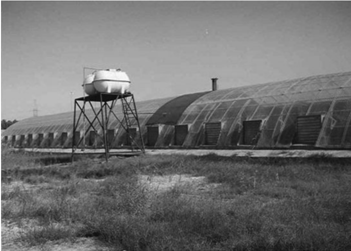
Fig. 5.61 Round-arched tunnel with fan and pad cooling at side wall in Kuwait
