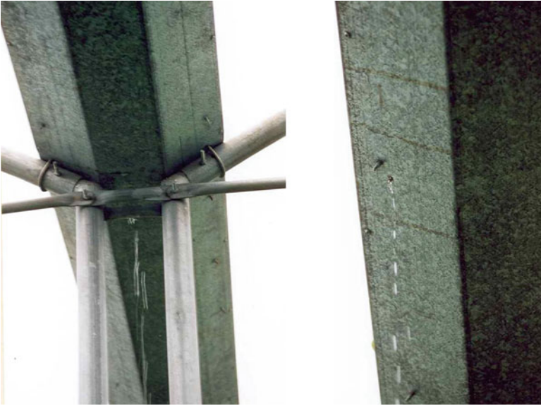
Fig. 8.13 Leaky gutter connection, bare holes or rusted-through holes cause water penetration into the greenhouse, flooding, and destruction of the crop
