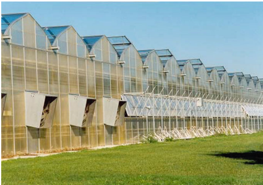
Fig. 9.41 Fans for forced ventilation ( left side ) and air inlet flaps ( right side ) combined with roof flaps for natural ventilation (USA)
