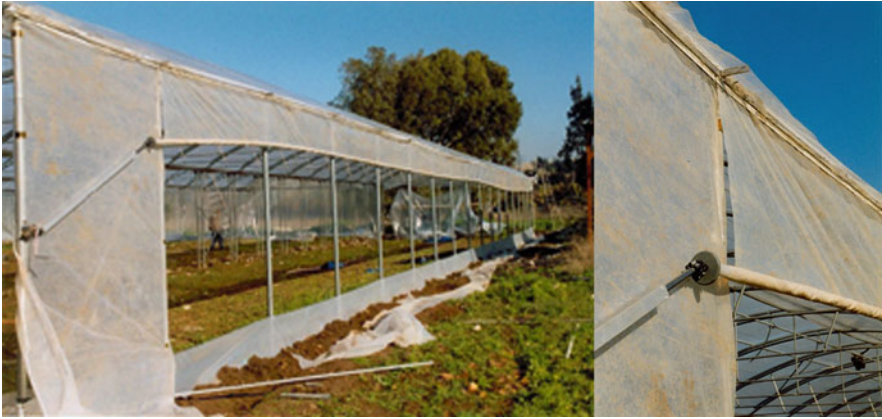
Fig. 9.5 Although a plastic film is fixed over 1.5 m from eave to bottom, there is no overlapping with the roll-up vent, with the consequence of leaks, danger of destruction and cold air infiltration
