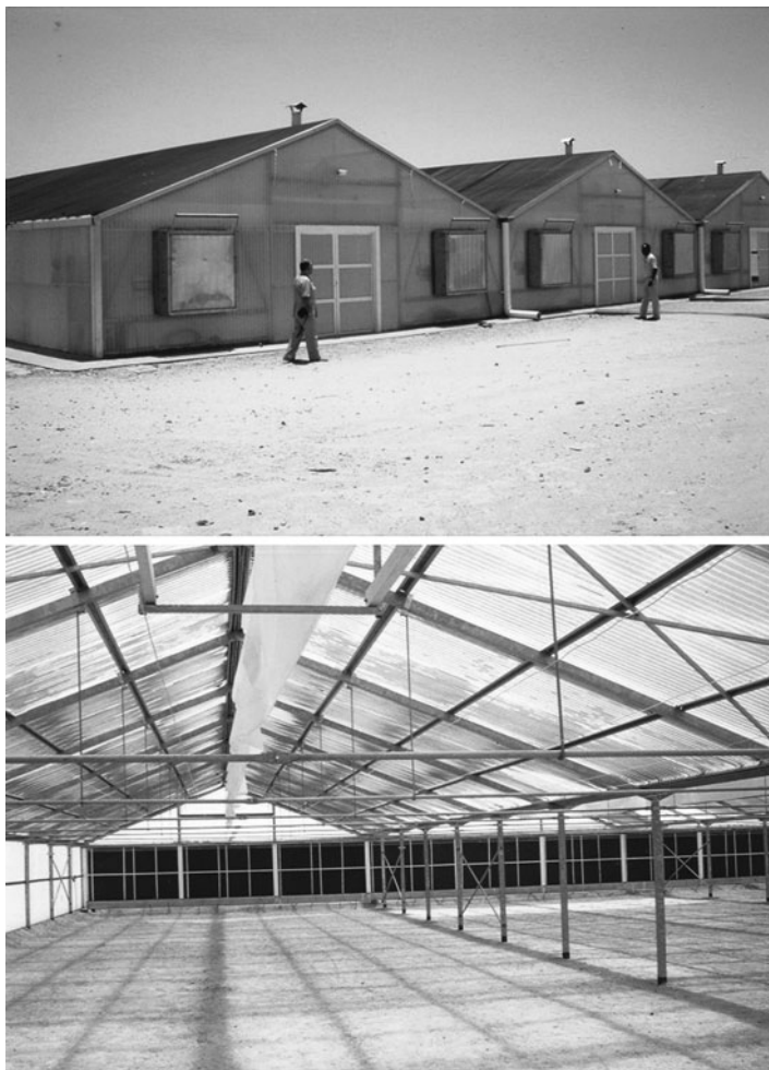
Fig. 5.57 A greenhouse structure for desert regions in Kuwait, covered with rigid plastic sheets and equipped with fan and pad cooling
