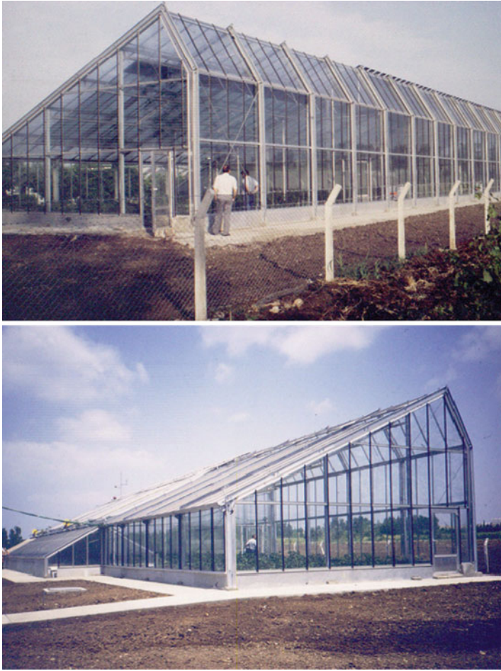
Fig. 15.11 Closed-system greenhouse type Hannover
