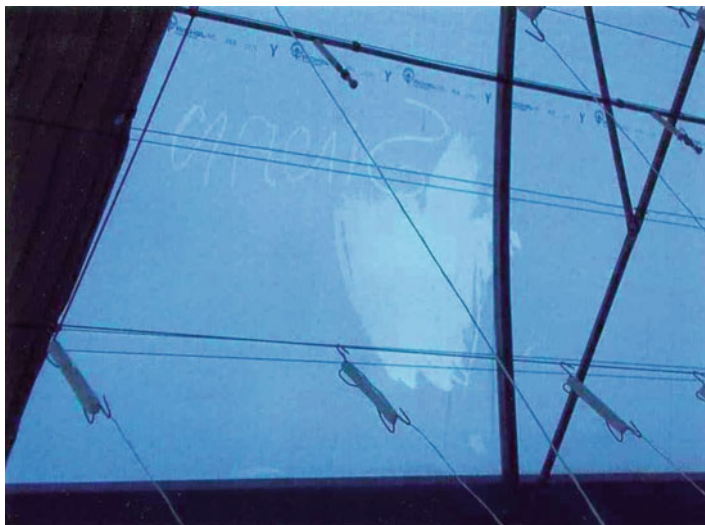
Fig 7.1. Plastic film greenhouse with heavy dust accumulation in an industrial region
