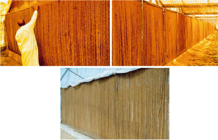
Fig. 11.11 A pad made from vertical ropes
