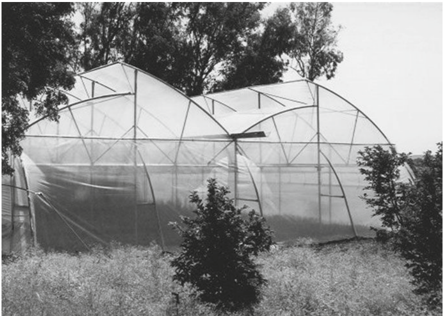
Fig. 5.40 Very stable steel tube structure from India, with bent roof and side wall tubes
