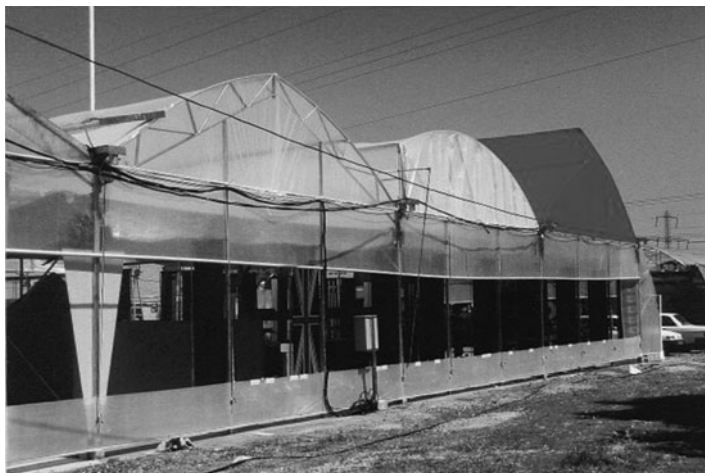
Fig. 5.53 Greenhouse structures with different ventilation openings at roof and ridge in Israel. The gutter height is 4 m minimum
