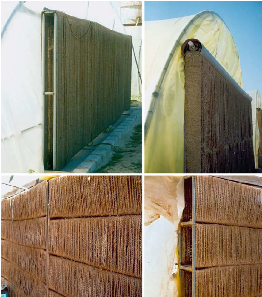
Fig. 11.13 Double- or multi-layer rope pads are recommended
