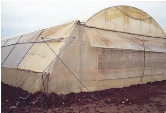
Fig. 5.18 Sloped side walls covered with insect screens and rolling-up ventilation in Jordan
