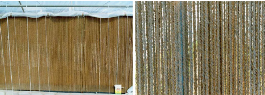
Fig. 11.12 A single row rope pad is not sufficient because of free entrance for air and low efficiency
