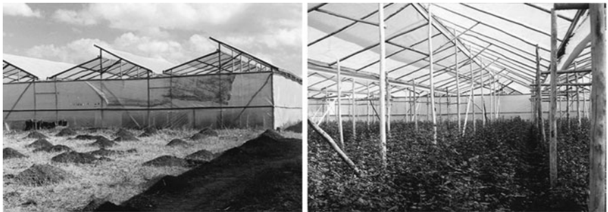
Fig. 5.37 Greenhouse for roses in Malawi with open space only in the roof and gable area, to protect the flowers from wind and sloping rainfall
