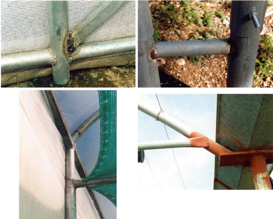
Fig. 8.11 Galvanised steel components welded together (see Sect. 8.2.1.1)
