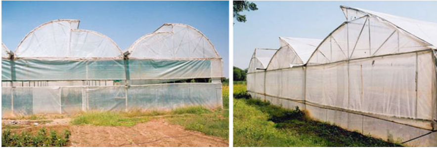
Fig. 9.19 Growers in India found that ventilation efficiency can be improved if the vertical ventilation openings at the ridge are directed in alternate directions. In most cases, the ridge vent of the last span is directed alternately. The openings of the ridge vents are open, while the side wall vents have roll-up vents
