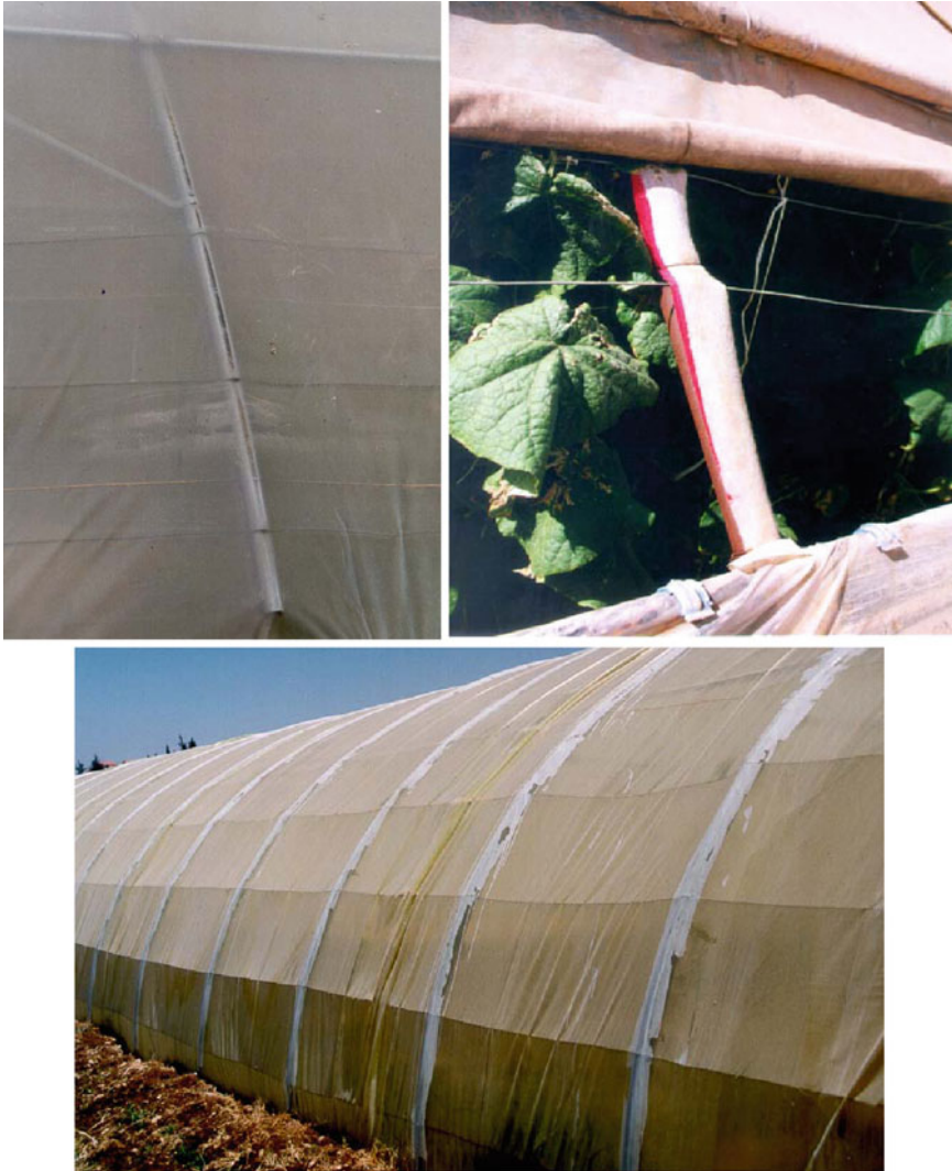
Fig. 4.4 Insulation of steel components or protection by white painting of the plastic film
