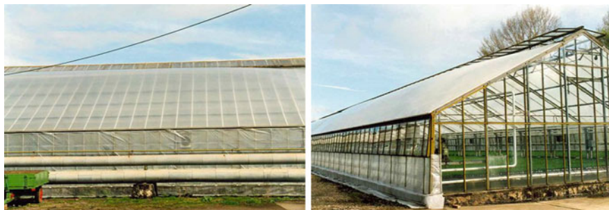
Fig. 8.25 Double-inflated film can also be used to repair and to use old structures, for example old glass houses. The old cladding material will be removed and double-inflated film installed
