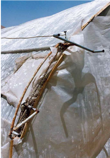
Fig. 8.20 One can fasten and stretch the plastic film from the roof side and side wall by rolling them up on one tube only. This method is a very elegant one
