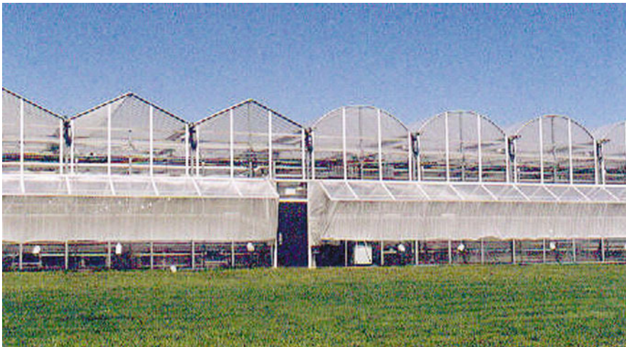
Fig. 10.4 Screened side wall vent openings (USA)
