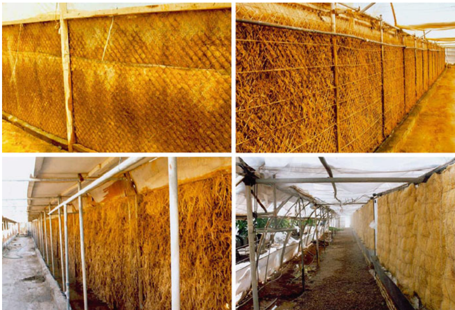
Fig. 11.10 Pads from natural plants and wood excelsior
