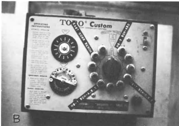
Fig.5-36 A and B. Two types of automatic watering controllers. (A) Electrical, each button representing one or more benches to be watered. Length of irrigation is set by the left dial. (B) Operates hydraulically, and can be preset to water on specified days and one or more times each day. Length of irrigation period can be regulated independently for each unit
