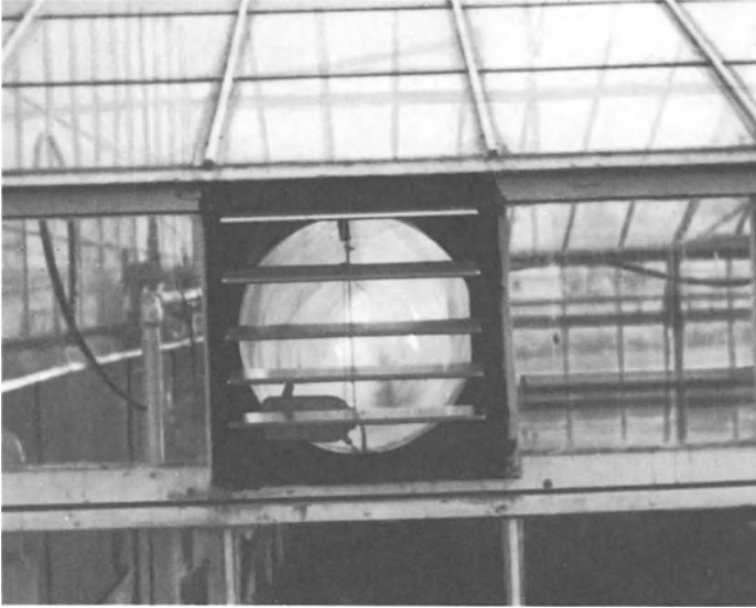
Fig.4-47. Motorized louver in series with the first stage cooling fan or energized by a step controller as the first stage of cooling where a poly tube pressurizing fan is used
