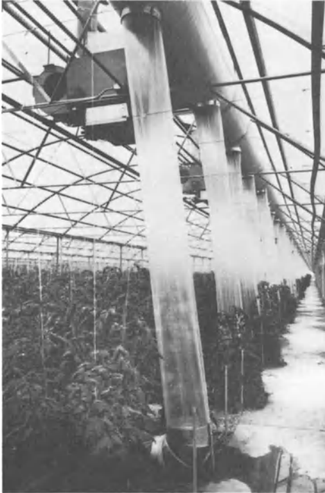
Fig.4-34. Horizontal temperature pattern produced at bud height (4 ft) by horizontal unit heater with the polyperforated tubing running the length of the greenhouse. Note relatively cool area produced near the heater during the “on” portion of the heating cycle (Bark and Carpenter, 1969)
