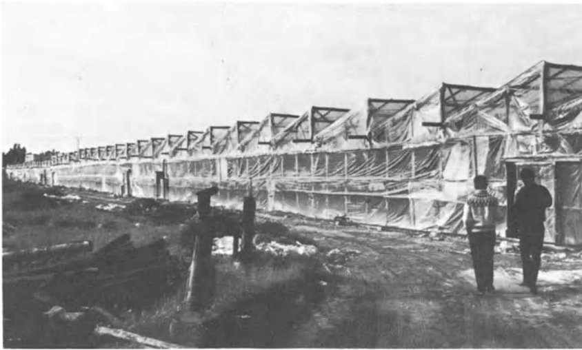
Fig. 1-3. Inexpensive greenhouse construction in warm climate, largely for protection from rain
