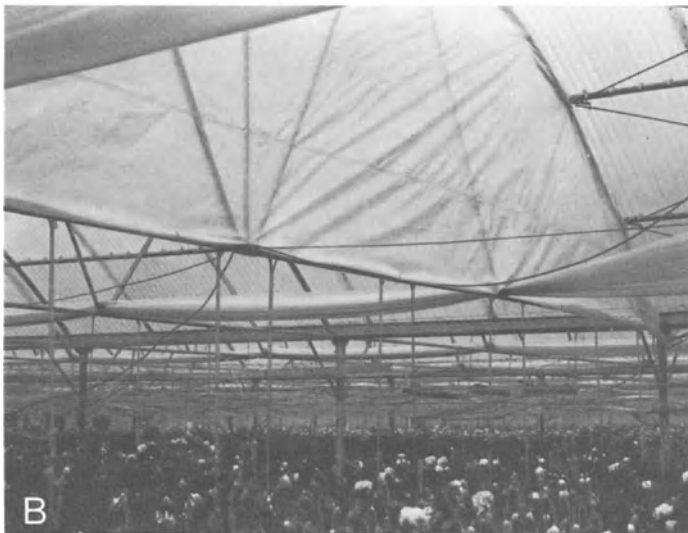
Fig.4-44. (A) Cross and longitudinal flow designs (Augsburger et al., 1975). (B) Clear plastic baffle attached to a truss
