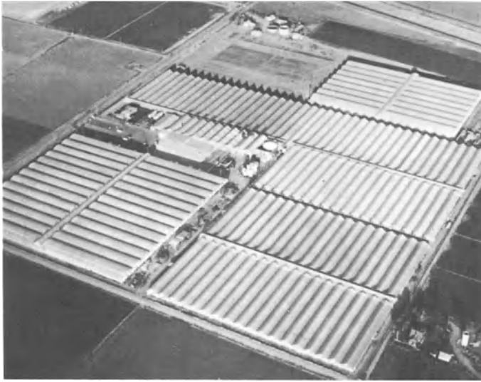
Fig. 1-4. Greenhouse production range exceeding 150000 m 2 , fiberglass covered in a climatic region requiring complete heating and cooling systems
