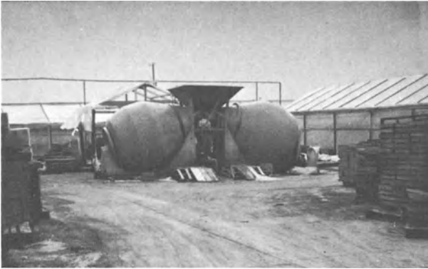
Fig.6-13. Surplus concrete mixers installed to mix several cubic yards of potting substrate at a time. Front-end loader charges mixers from center, and unloading occurs onto conveyor belt between the two and under loading hopper
