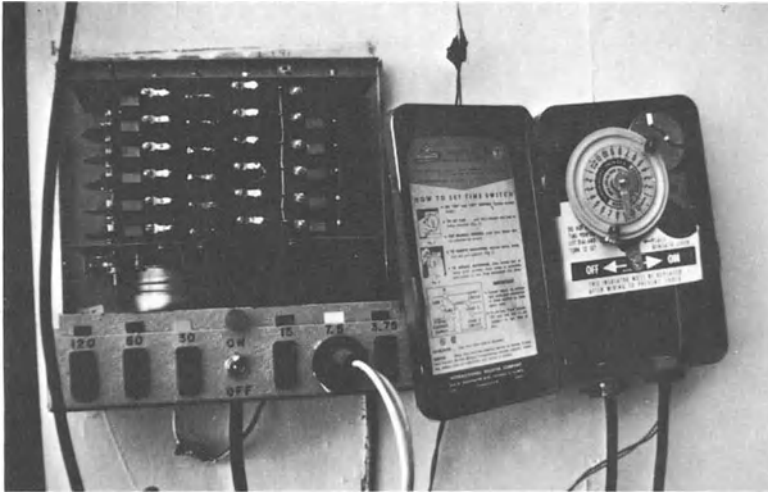
Fig. 5-16. Example of automatic mist control system for mist propagation. Right : 24-h clock turns system on in morning and off in evening. Left : clock controls time mist is on, and interval between cycles
