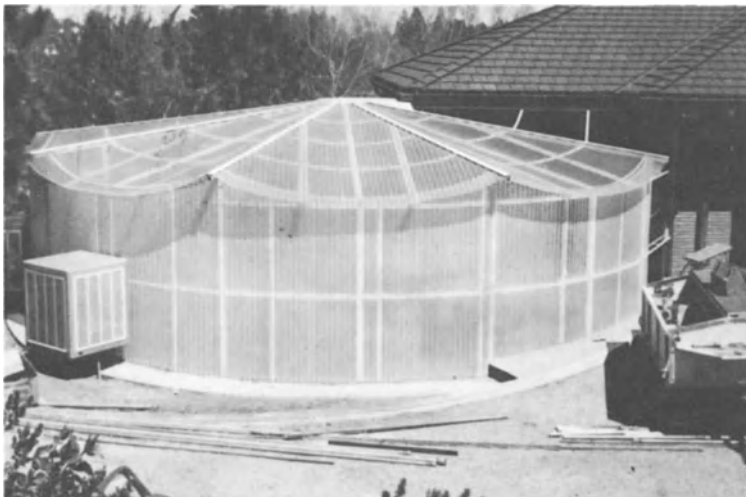
Fig.1-9. An esoteric greenhouse design, probably covering a swimming pool. Note that cooling uses an evaporative cooler, forcing the air into the structure. This system is seldom feasible on a large scale. Greenhouses may assume many shapes and styles
