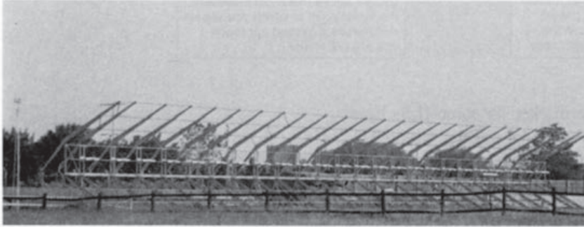
Figure 27-3 The localizer transmitting antenna.
