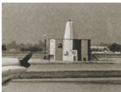
Figure 17-5 A VOR ground station.
