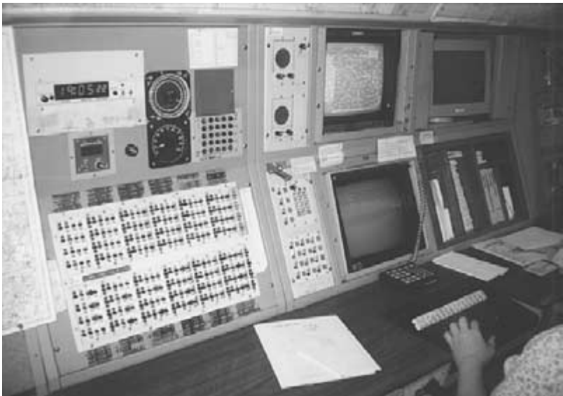
Fig. 26-4. This is the bank of 48 frequency lights that the in-flight position must monitor.
