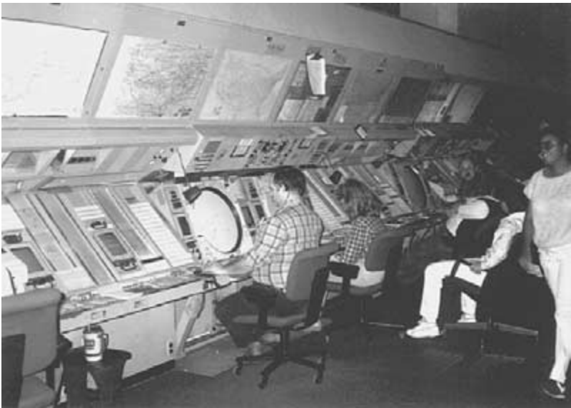
Fig. 22-5. As much as a darkened room will permit, this picture illustrates the elements that make up a sector suite in a typical Air Route Traffic Control Center.
