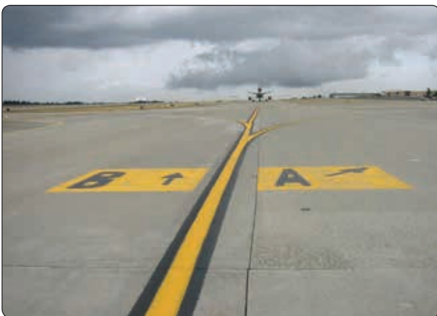
Figure 14-19. Surface painted taxiway direction signs.
