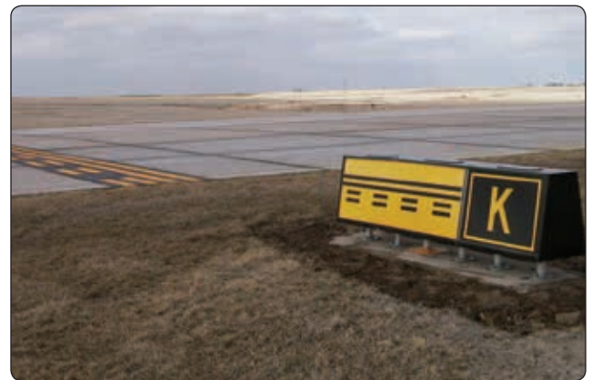
Figure 14-8. Runway safety area boundary sign and marking located on Taxiway Kilo.
