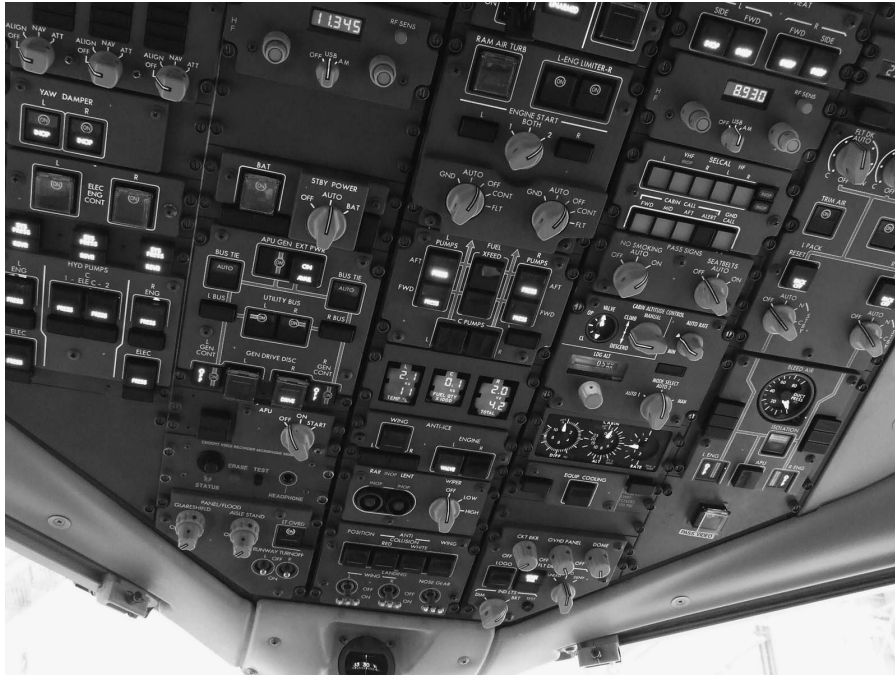
Figure 13.12 Air conditioning system control (right/centre of overhead panel)
