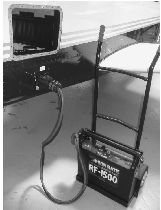
Figure 8.7 External ground power from a battery pack
