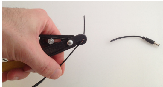
Removing Wire Insulation
