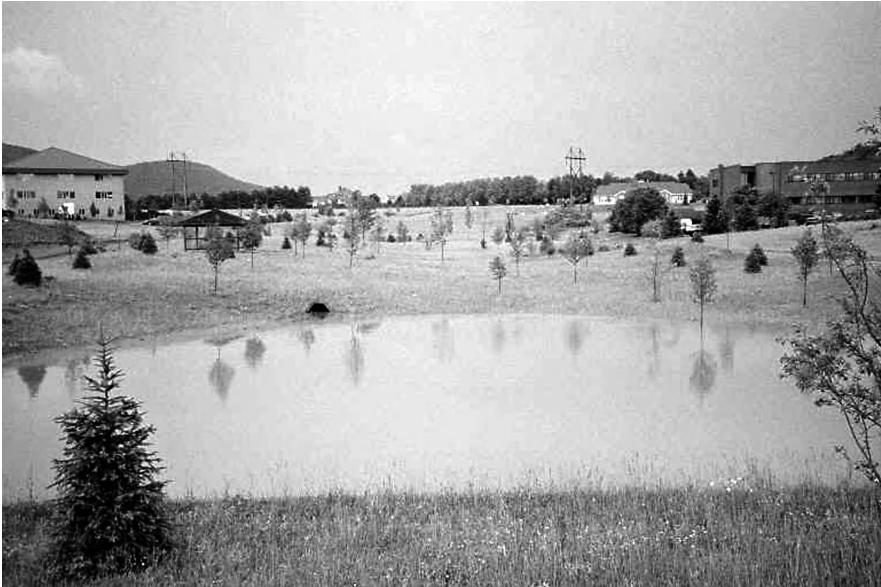
Figure 1.6 A retention basin in a professional office park (courtesy of S. Brown, Penn State University).
