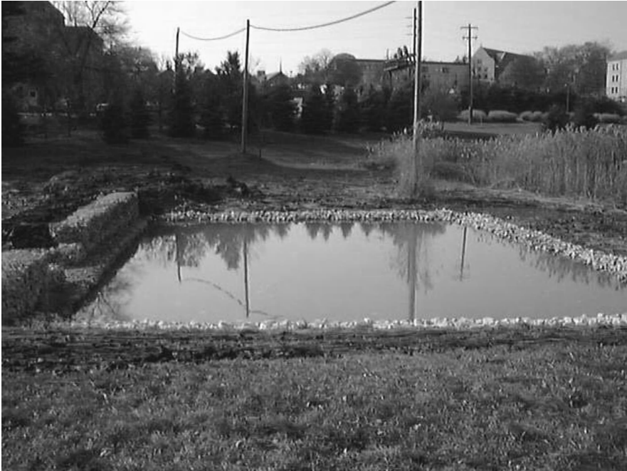
Figure 1.2 A sediment forebay used to capture the first flush of runoff (courtesy of R. Traver, Villanova Urban Stormwater Partnership, Villanova University).
