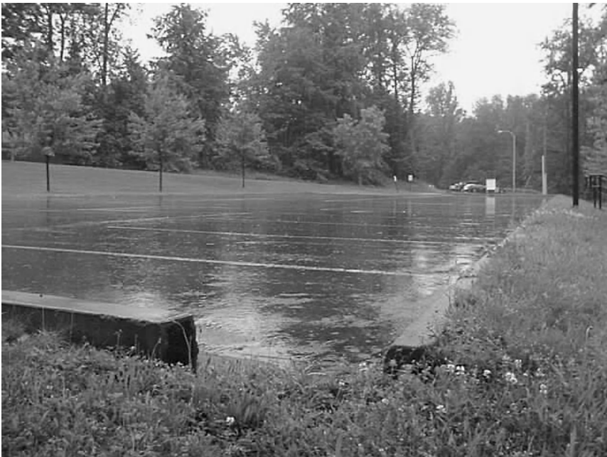
Figure 5.2 This very small watershed comprises a paved parking lot bounded by curb gutters. The curb opening in the foreground acts as the watershed outlet (T. Seybert).
