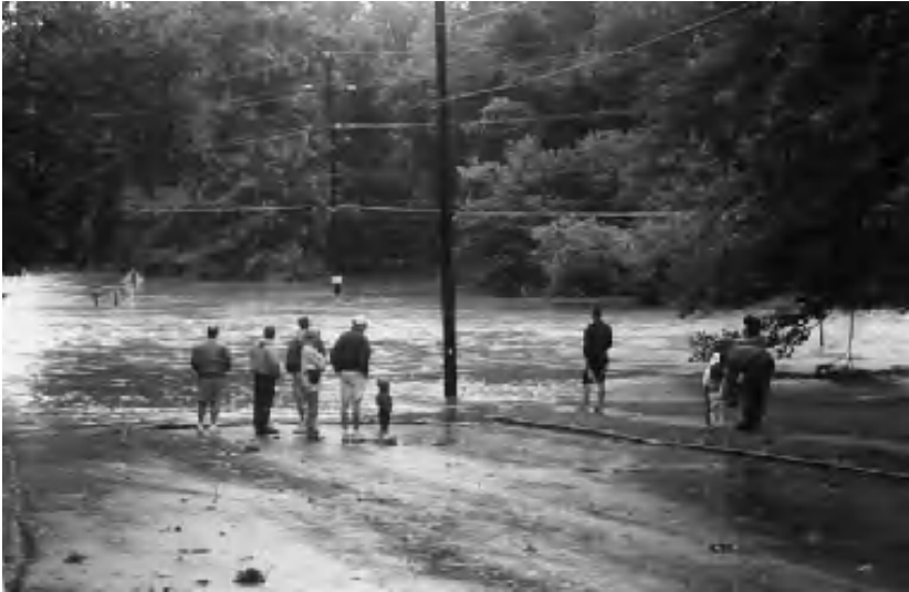
Figure 1.1 Channel and roadway flooding caused by upstream land development (courtesy of F. Thornton, Darby Creek Valley Association, Delaware County, PA).
