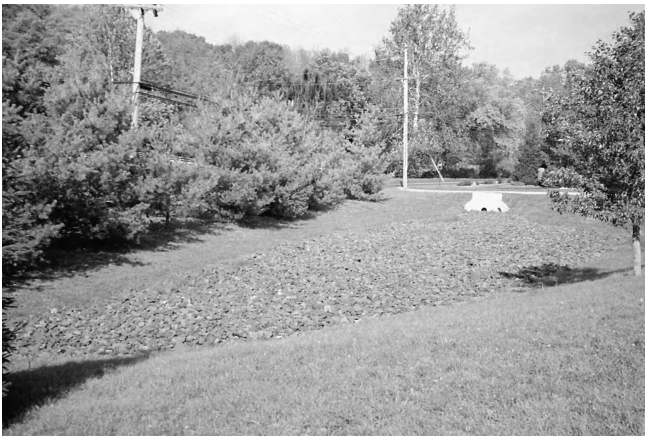
Figure 1.4 Groundwater recharge through an infiltration trench (courtesy of P. DeBarry, Borton-Lawson Engineering, Wilkes-Barre, PA).
