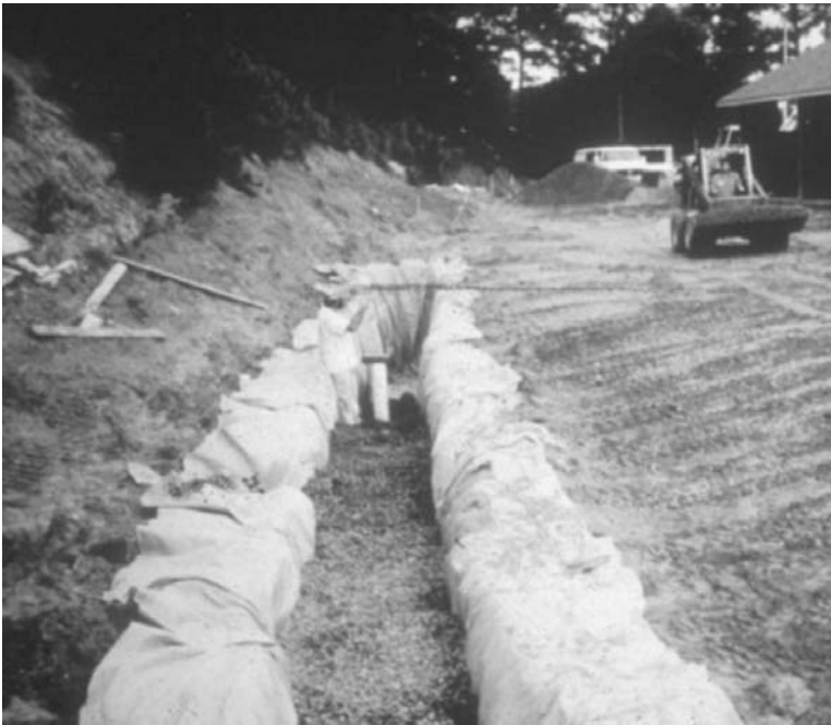
FIGURE 13-84 Infiltration trench construction.
