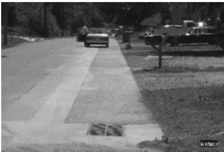
FIGURE 13-90 Porous pavement street ribbon edge.
