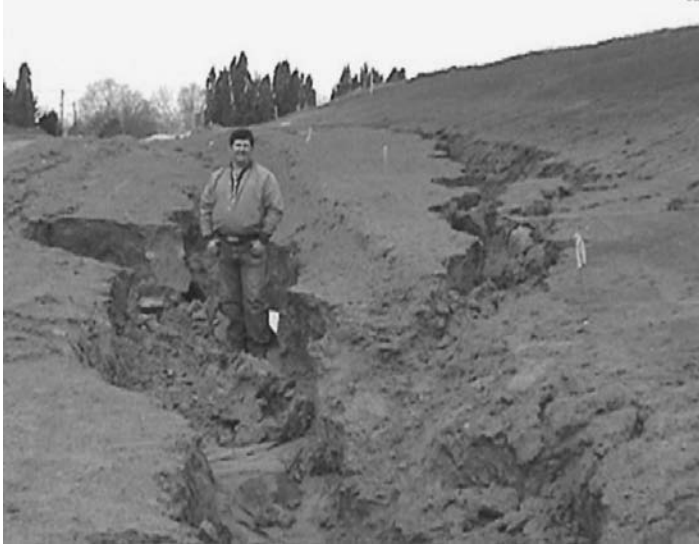
FIGURE 15-16 Construction site erosion problems.
