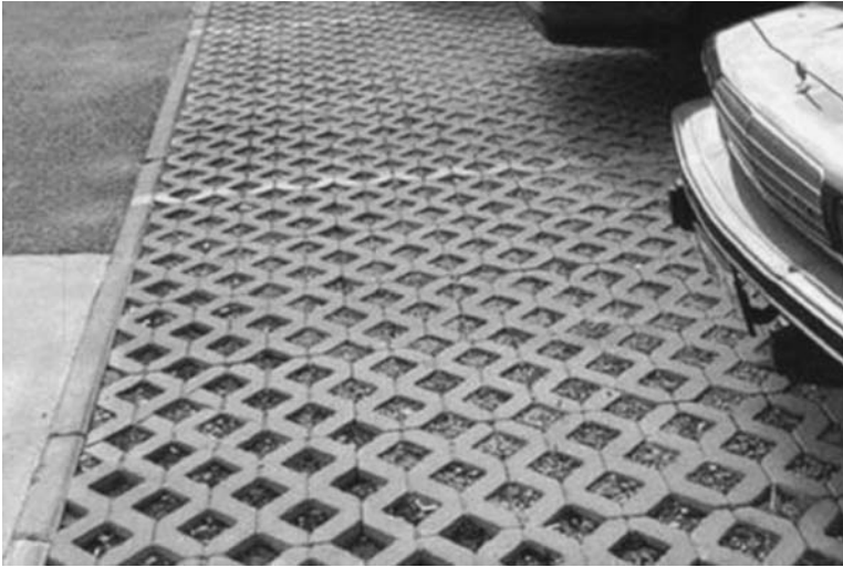
FIGURE 13-95 Lattice-type paver system.
