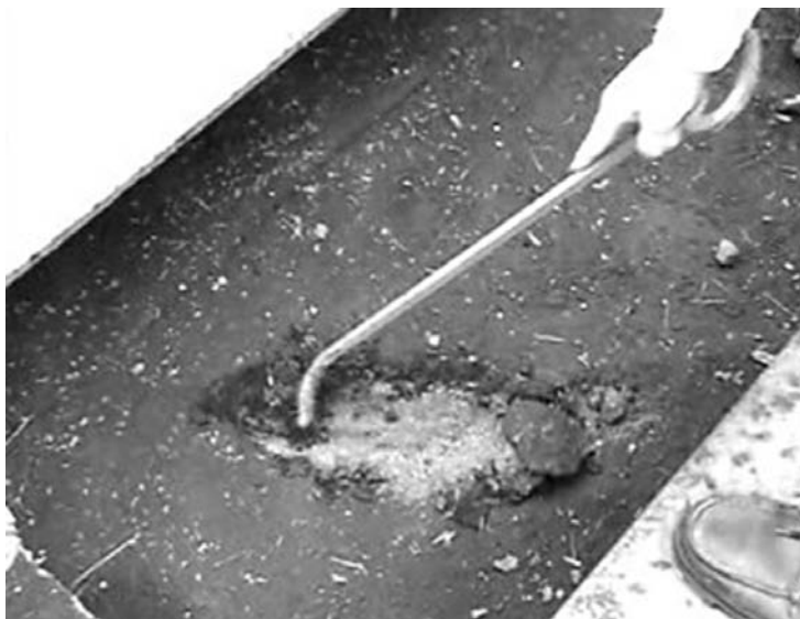
FIGURE 13-56 Scraping polluted surface of sand filter.
