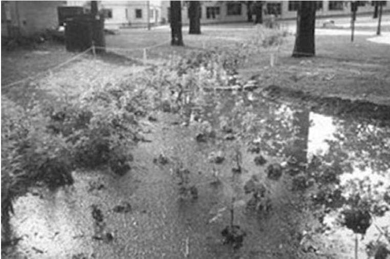
FIGURE 13-52 Bioretention area after a storm.
