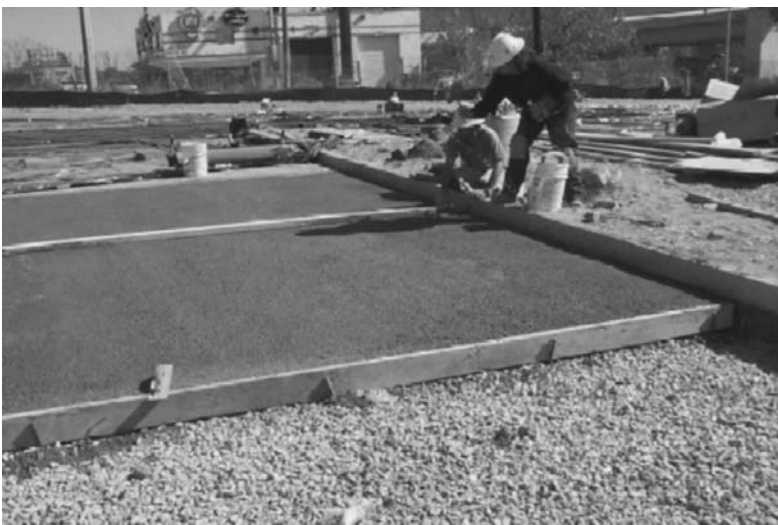
FIGURE 13-93 Porous pavement placement. (From Atlanta Regional Commission, Georgia Stormwater Manual, 2002.)
