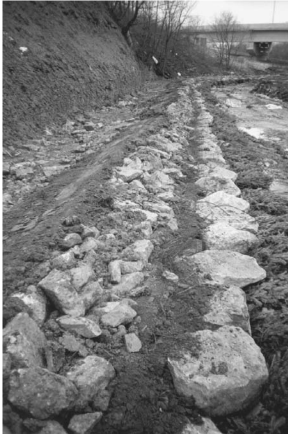
FIGURE 10.24 Riprap vegetation combination for bank protection.
