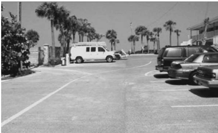
FIGURE 13-89 Porous pavement parking lot.
