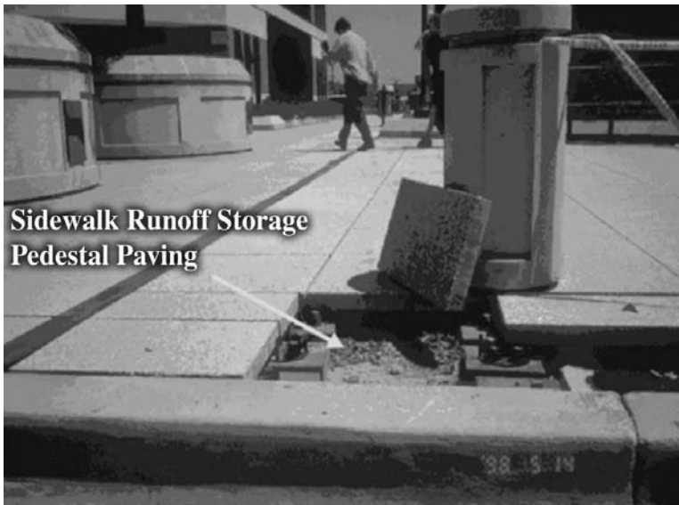
FIGURE 13-99 Pedestal paving for sidewalks.
