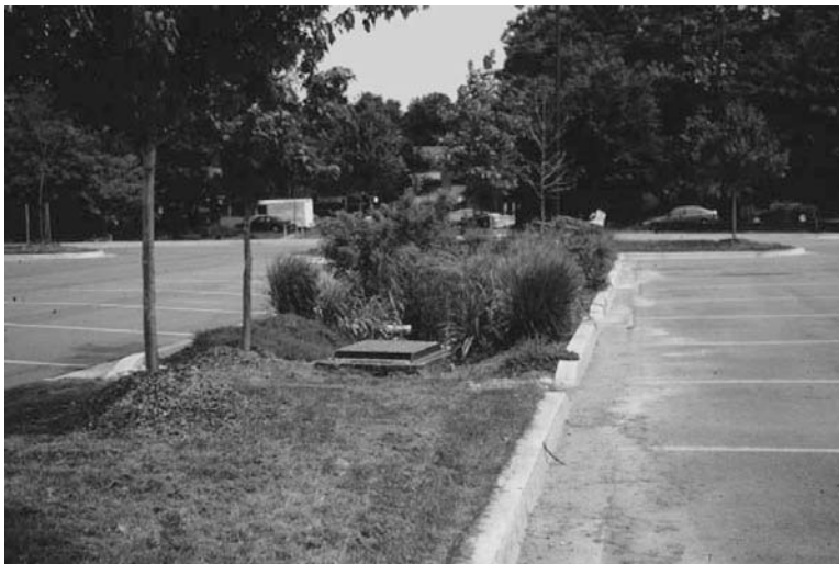
FIGURE 13-50 Parking island bioretention.
