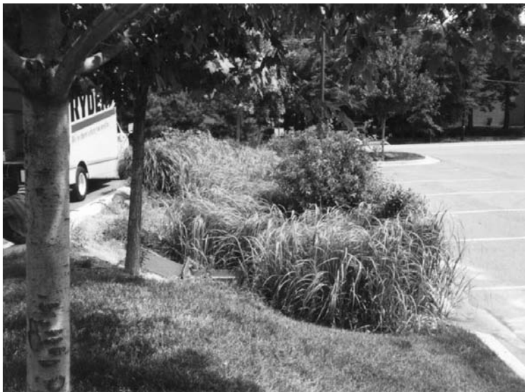
FIGURE 13-49 Parking lot bioretention area.
