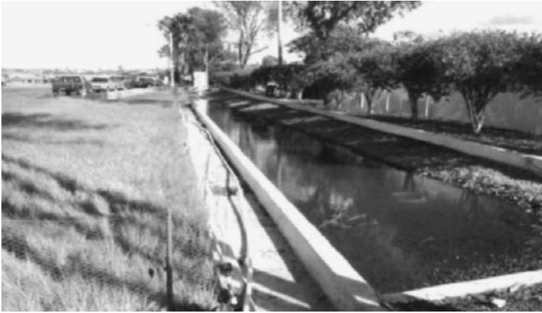
FIGURE 13-83 Infiltration trench in San Diego, California. (From CALTRANS.)
