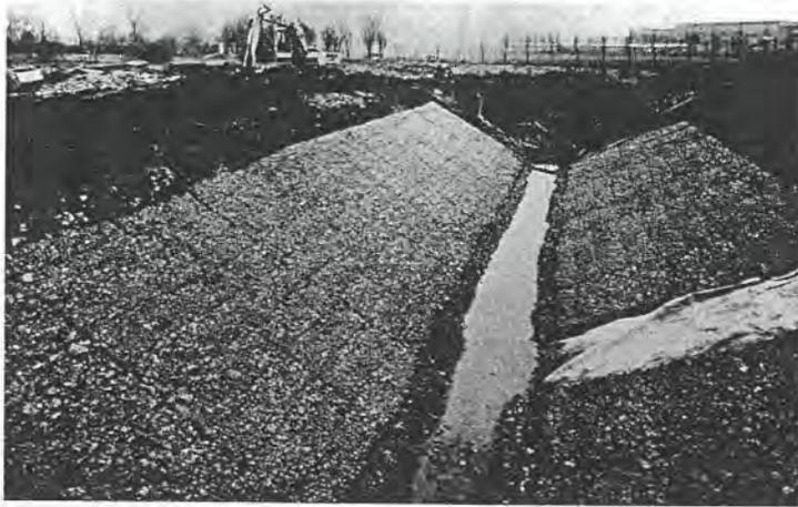
Fig. 10.25. Bank protection by stone mattresses (by courtesy of Maccaferri Gabions).
