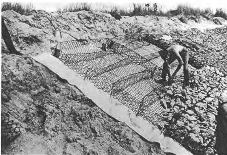
Fig. 10.28. Placing of mattresses over plastic fiber cloth (by courtesy of Maccaferri Gabions).
