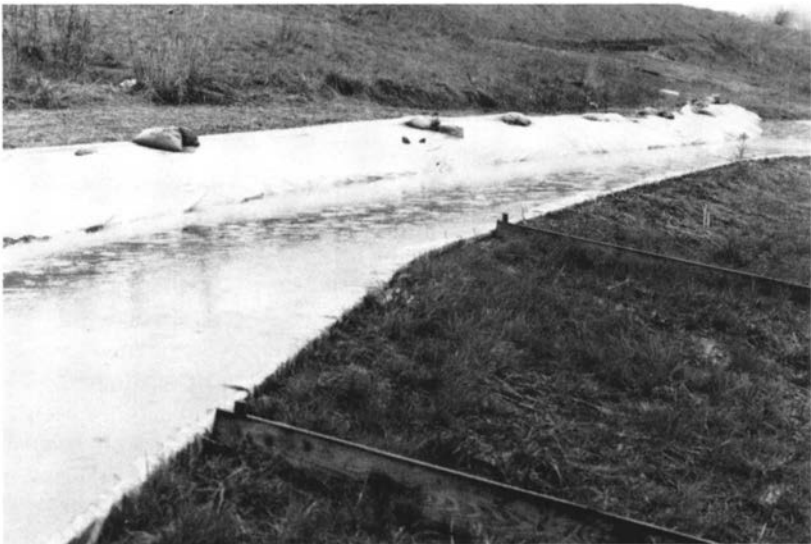
Figure 4. Level spreader with vegetative buffer strip.
