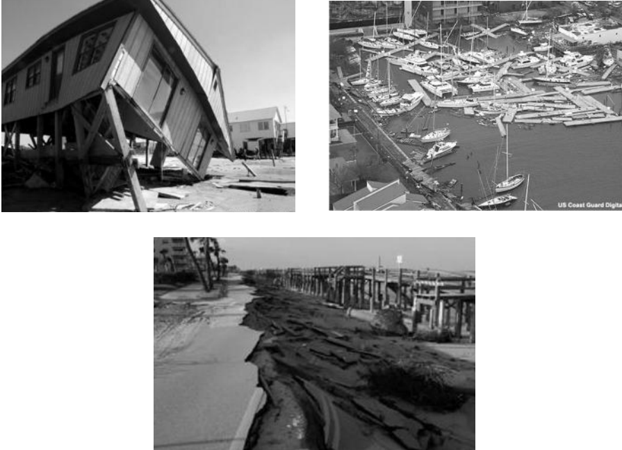
Figure 14.15 Damage due to storm surge. (Source: http://www.nhc.noaa.gov/ssurge )
