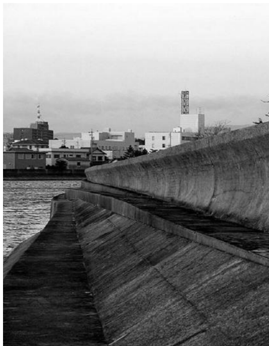
Figure 14.8 Tsunami walls to protect coastal areas. (Source: http://en.wikipedia.org/wiki/Tsunami_Generation_mechanisms )
