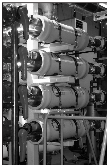
Figure 3-8 PX™ Pressure exchanger device installation in Sand City, Calif.
