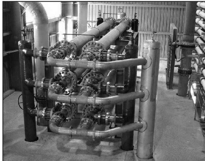
Figure 3-10 Installation of Flowserve DWEER energy recovery device
