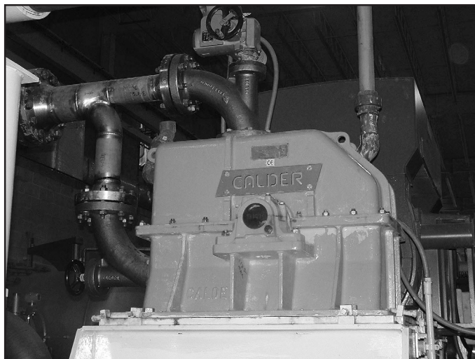
Figure 3-4 Pelton wheel generators at Tampa Bay SWRO facility
