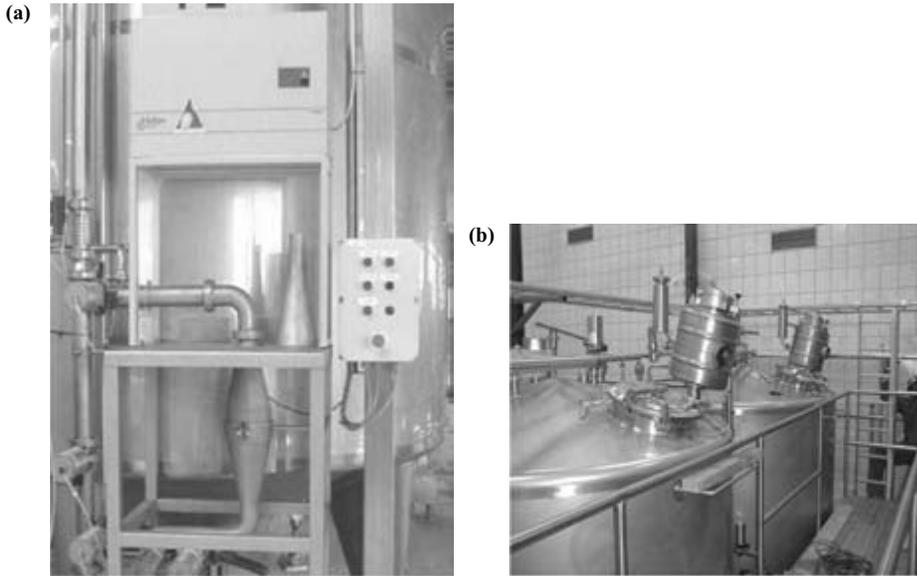
**Fig. 5.10** (a,b) In-line inoculation of the processed milk with freeze-dried starter culture. By permission of Tetra Pak AB, Lund, Sweden.
