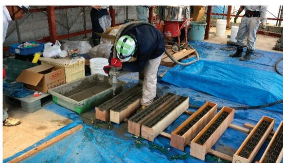
**Figure 3.** Spraying PCM on the removed section of RC beams.
