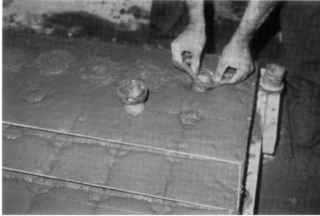
FIGURE 4.10 Inserting sleeve by rocking action.
