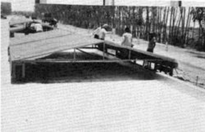
**Fig. 11.6** Using shades for curing of fresh concrete
