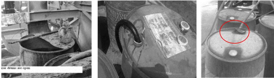
Highly incorrect method of pumping admixture with drum lid cut open
