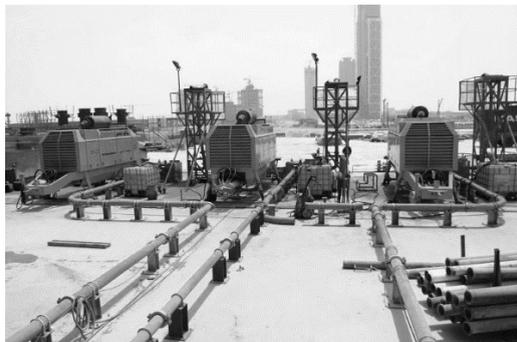
**Fig. 10.4** Proper anchoring of horizontal pipeline with anchors at both ends of coupling (if couplings are 3m apart, one more support is desirable)
