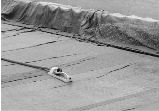
**Fig. 11.8** Automatic sprinkling arrangement to keep hessian cloth continuously wet
