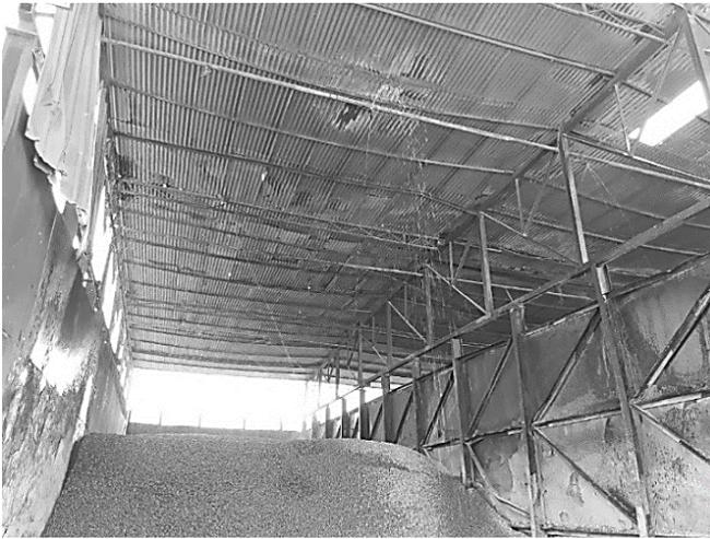
**Fig. 8.9** Keeping aggregate under shade and sprinkling of water for cooling of aggregate
