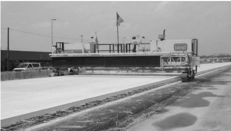
**Fig. 11.14** Applying curing compound with spray machine on concrete pavement
