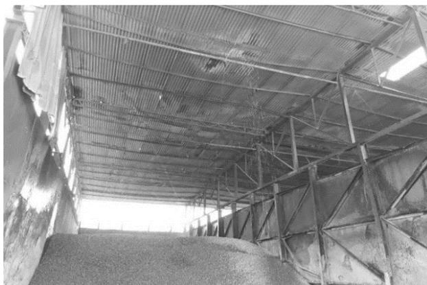
**Fig. 3.6** Providing shade over aggregate stockpile
