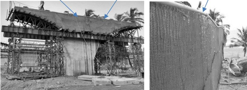
**Fig. 11.9** Curing of vertical members with water kept in drum connected to perforated pipes
