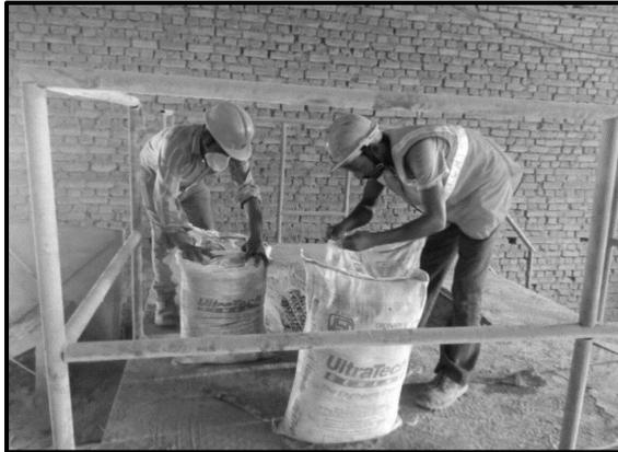
**Fig. 2.7** Opening of cement bags by removing thread on hopper platform
