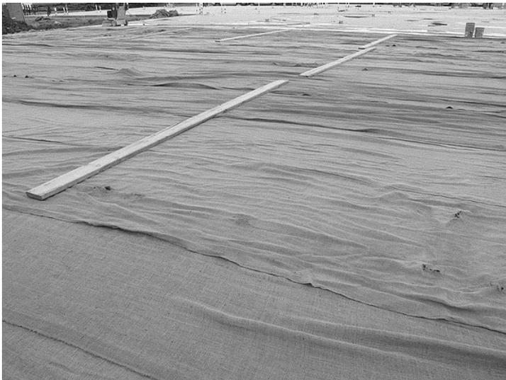
**Fig. 11.7** Curing of concrete with wet hessian cloth
