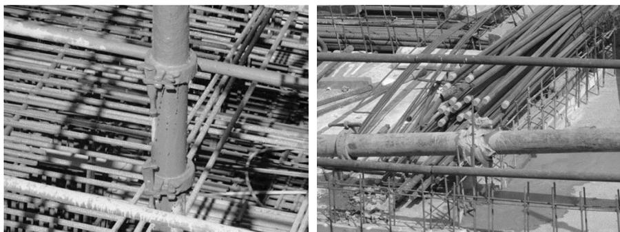
**Fig. 10.6** Leaking pipelines and coupling joints can cause serious quality & pumping issues
