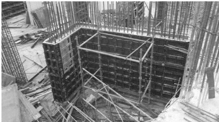
**Fig. 12.9** Plastic formwork
