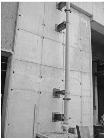
**Fig. 10.5** Proper anchoring of vertical pipeline with anchors at both ends of coupling (if couplings are 3m apart, one more support is desirable)
