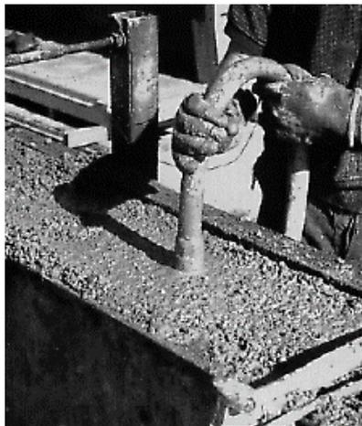
**Fig. 10.8** Use of an immersion vibrator
