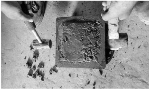
**Fig. 12.18** Tamping by wooden / rubber mallets on both sides of the mould simultaneously
