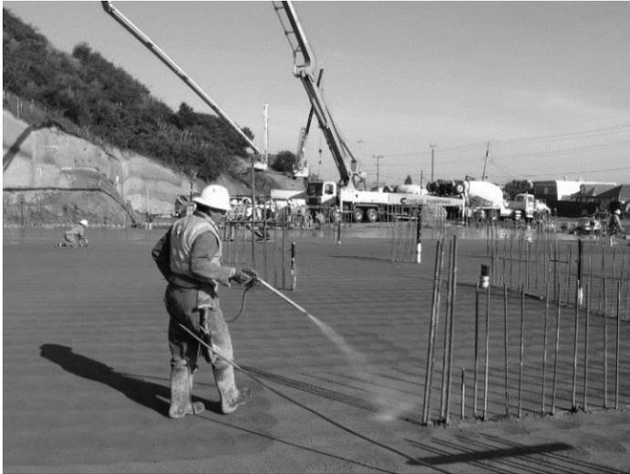
**Fig. 11.10** Sprinkling water for curing concrete slab
