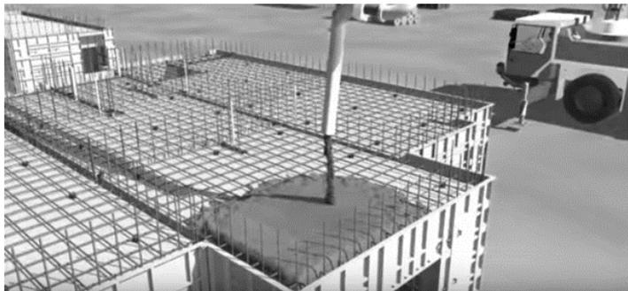
**Fig. 12.8** Mivan aluminium formwork system
