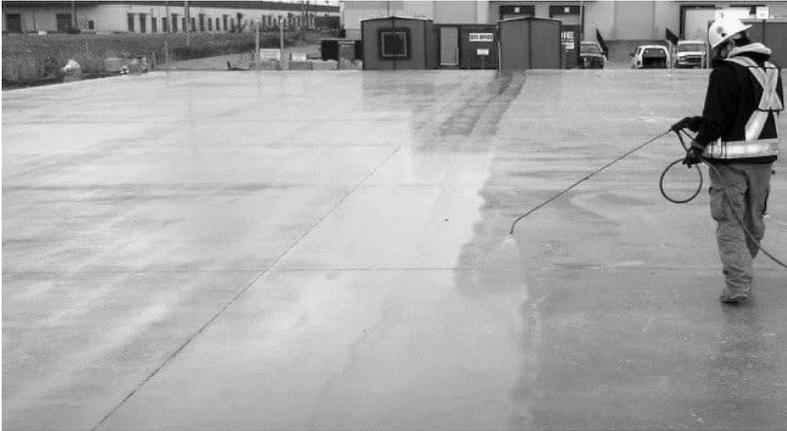
**Fig. 11.13** Spraying curing compound on flat concrete surface
