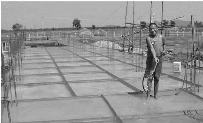
**Fig. 11.11** Curing of concrete by ponding method
