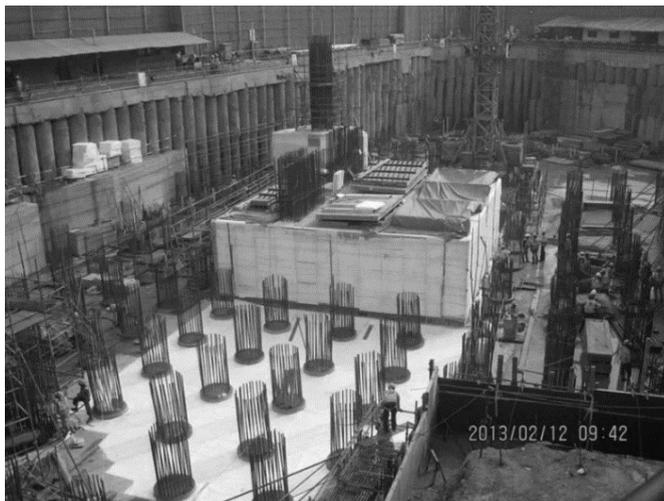
**Fig. 8.11** High density thermocol used for covering the concrete raft pour to control temperature differential
