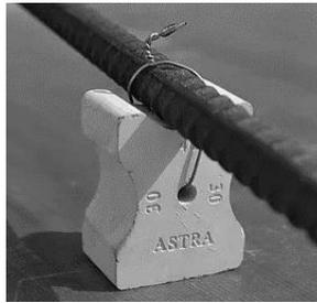
**Fig. 12.5** Factory made cover blocks
