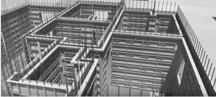
**Fig. 12.7** Mivan aluminium formwork system
