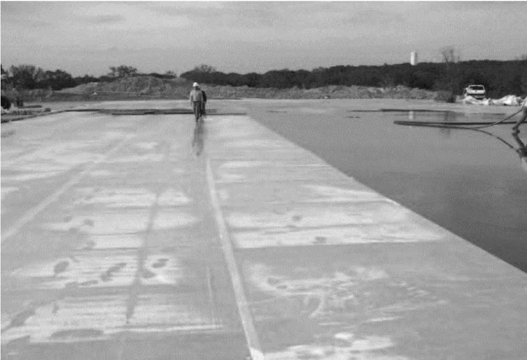
**Fig. 11.12** Curing concrete by covering with plastic sheet
