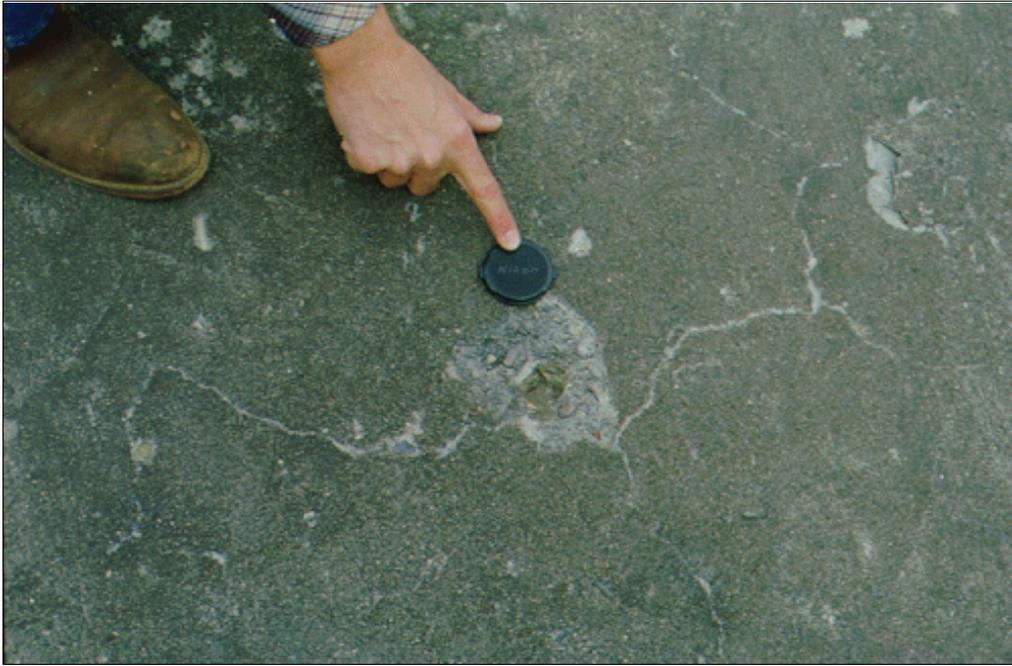
Figure 5.—Absorptive aggregate popout on spillway floor.
