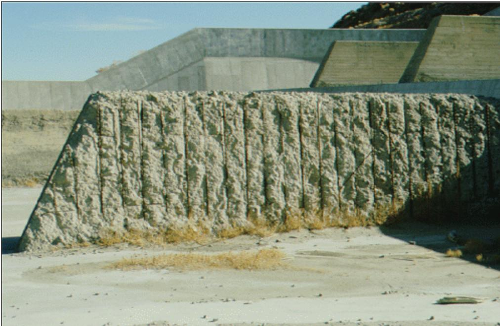
Figure 4.—This freezing and thawing deterioration should have been repaired before it advanced to the point that wall replacement or removal is the only option.
