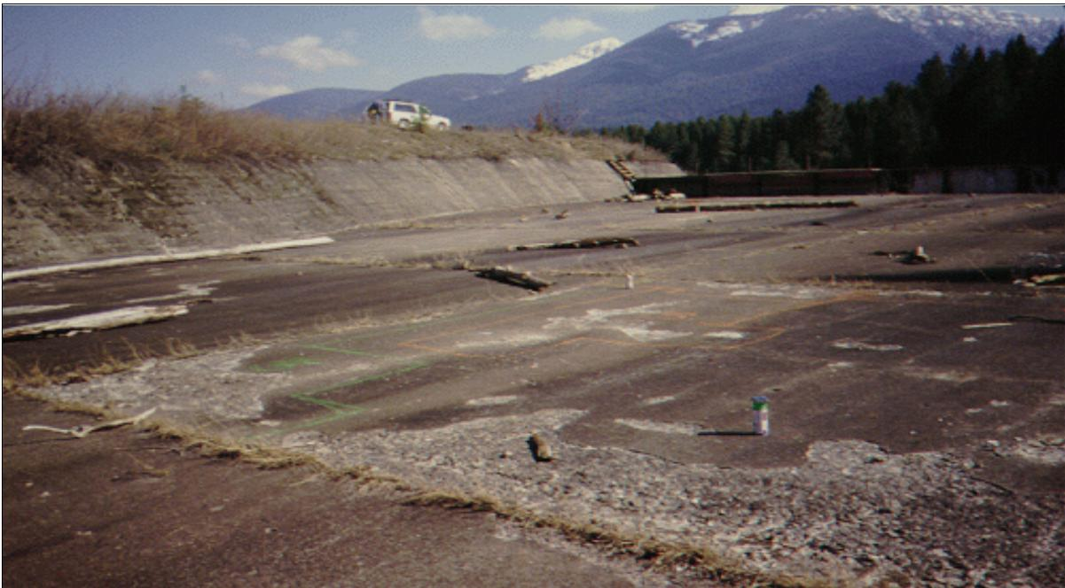
Figure 21.—Freezing and thawing deterioration on spillway concrete.
