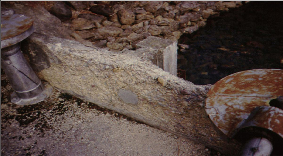
Figure 20.—Freezing and thawing deterioration on small irrigation gate structure.
