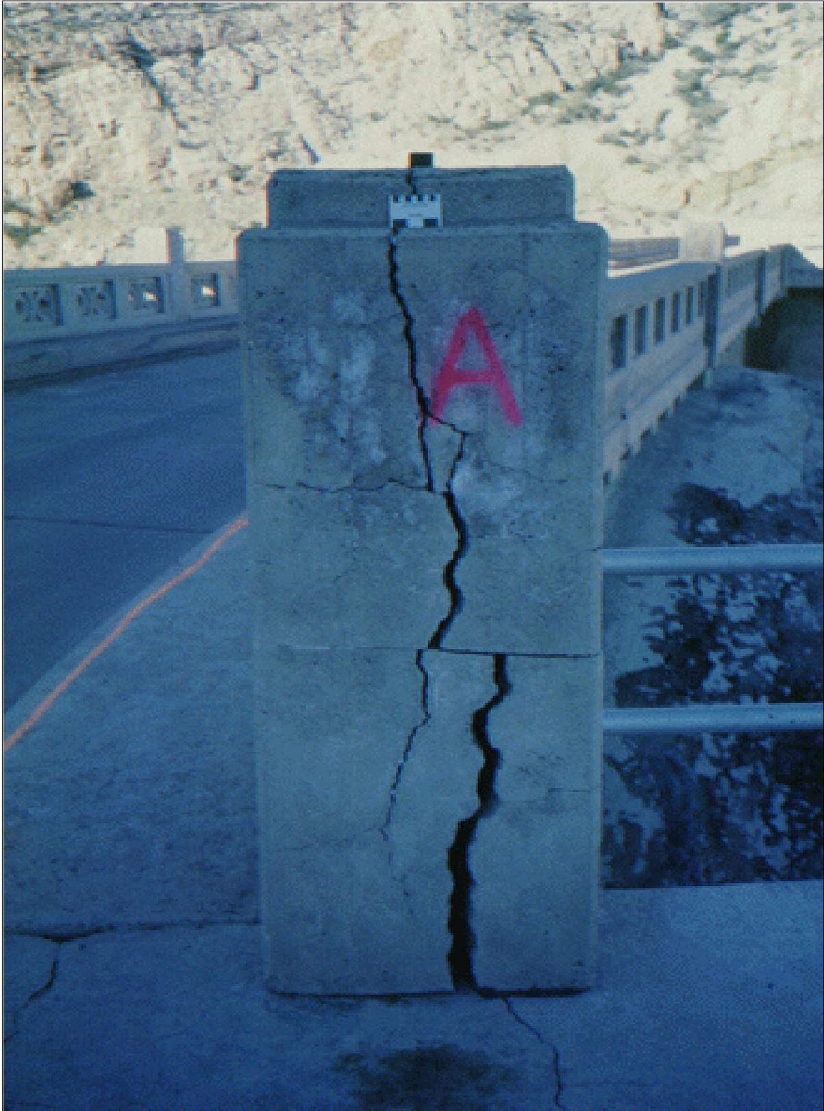
Figure 19.—Severe cracking caused by alkali-aggregate reaction.
