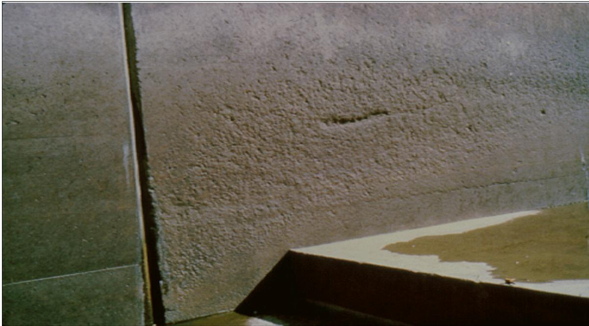
Figure 25.—Early stages of abrasion-erosion damage.
