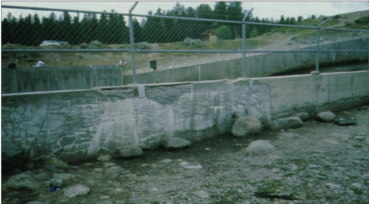
Figure 22.—D-cracking type of freezing and thawing deterioration.
