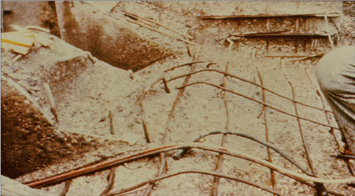
Figure 23.—Abrasion-erosion damage in a concrete stilling basin.
