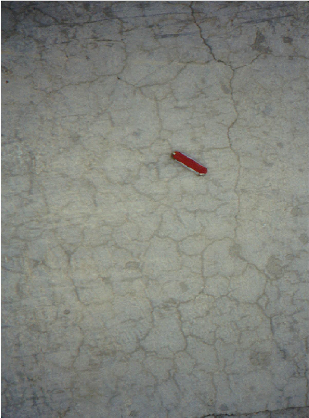
Figure 32.—Typical appearance of drying shrinkage cracking.
