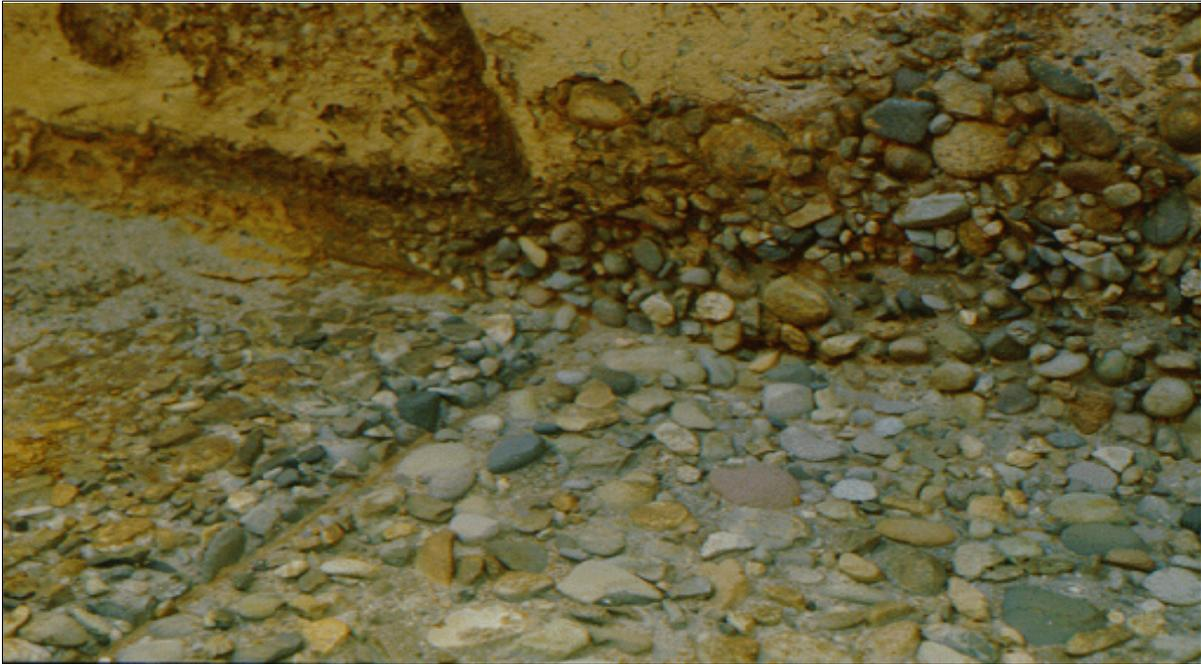
Figure 30.—Concrete deterioration caused by acidic water.
