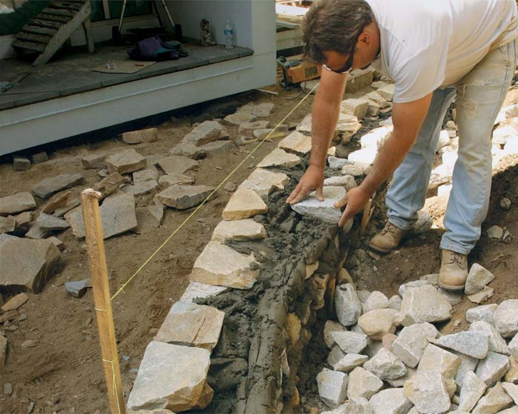
**BUILD UP THE BACK SIDE.** After setting a few courses of stone on the face of the wall, the author builds up the back side with less expensive blasted ledge stone set in plenty of mortar.
