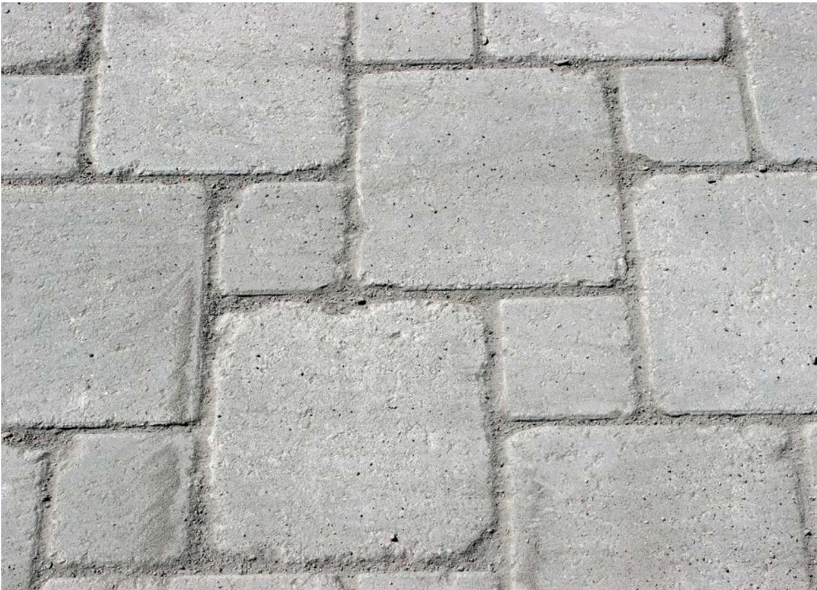
**FINALLY FILLED.** When done, the filler should end just below the level of the pavers.
