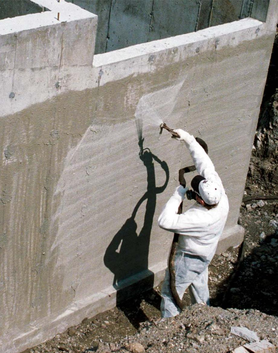
**WATERPROOFING, NOT DAMPPROOFING**, seals the foundation walls. More expensive than asphalt-based mixtures, a rubber-based membrane sprayed onto foundation walls remains flexible and waterproof.
