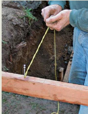
**PLACE THE LOOP OVER A NAIL**, pulling on the free end of the line while feeding the fixed end toward the nail.
