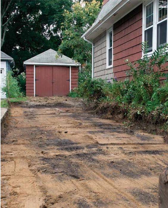
**GET THE BASE RIGHT.** A good excavator is crucial. When digging down to the required depth of the base stone, be sure that the subgrade is flat so that the succeeding layers are of a consistent depth.
