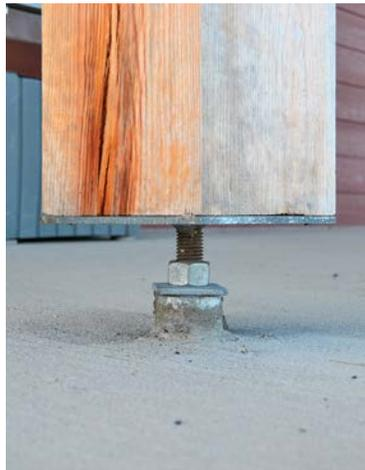
**ADJUSTABLE HEIGHT.** In some jurisdictions, a threaded stalk can be used to fine-tune the height of column bases.
