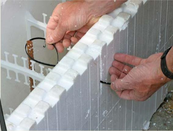
**AFTER THE FIRST COURSE HAS BEEN LAID, SLICE THE SIDE OF** one block and loop a zip tie around the vertical rebar that extends from the footing. Pull the tail end of the zip tie through the slot so that it's accessible from outside the form.
