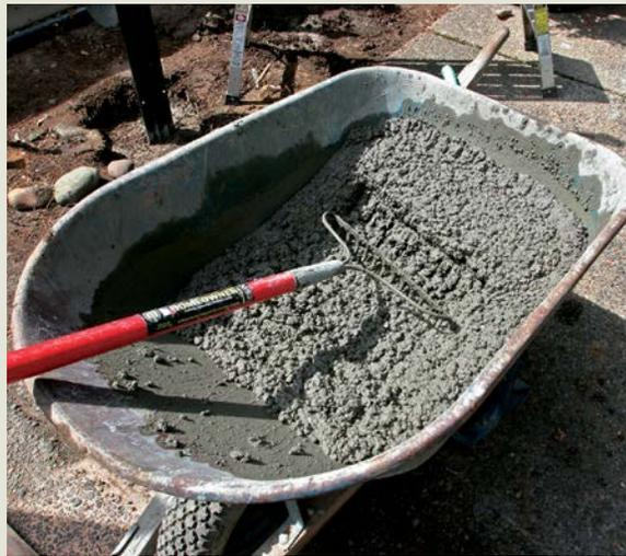
**6 THE FINAL TEST.** I'm done when all the concrete is wet and I've scraped the rake along the bottom and sides to remove any dry pockets. The mix passes my personal slump test when it's all wet but still firm enough for the rake's furrows to hold their shape.
