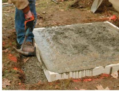
**6 TAP THE SIDES OF THE FORM.** Lightly hammer the form all around the slab until you see bubbles rising from the concrete. This step makes for a smoother slab edge that won't collect water, which can freeze and spall the concrete.
