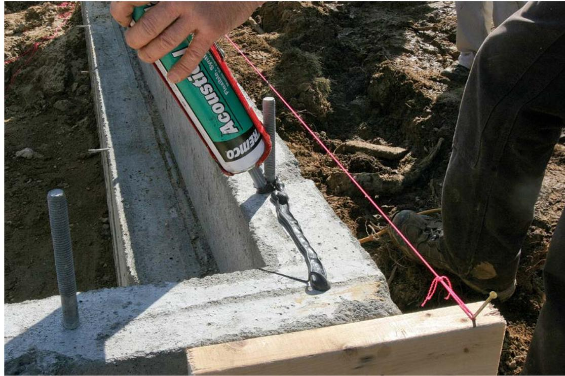
**STACK THE LAYERS.** The primary air-seal in this assembly is Tremco acoustical sealant. Highly elastic and sticky right out of the tube, this sealant won't harden over time like construction adhesives, so it creates a reliable air-seal at vulnerable joints.
