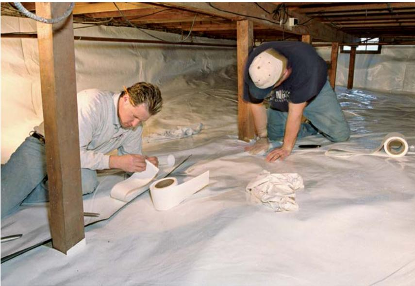
**SEEMS LIKE A SINGLE SHEET, BUT IT'S NOT.** Overlapping seams of the liner sections are sealed with caulk and matching tape for a seamless barrier.
