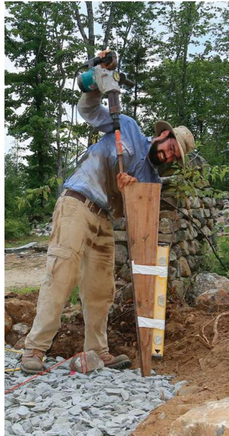
narrower (6 in. on each side) at its top. With flatter stones, a steeper batter like 1:10 may be appropriate, while a batter of 1:6 makes a wider base that's better for more irregular stone.
