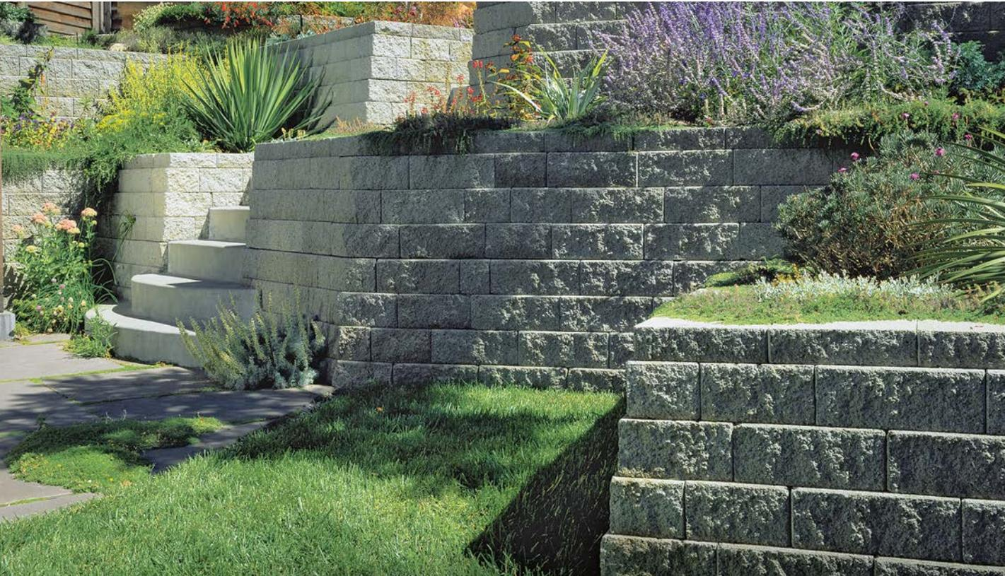
**MODULAR BLOCK** is versatile in design and interlocks for strength.
