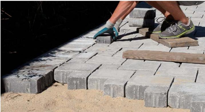
**LAY THE PAVERS.** Place the pavers carefully so that they maintain proper contact with each other. Standing on boards spreads out your weight and prevents the set pavers from tipping.
