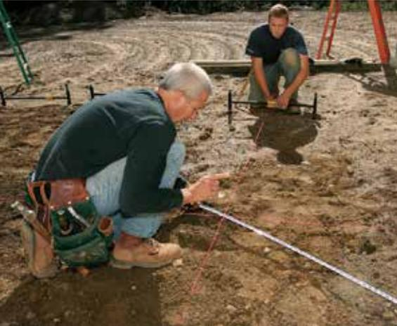
**3**  $A^2 + B^2 = C^2$ . Pulled diagonally from the foundation, my tape forms the hypotenuse of a right triangle. A helper shifts the line that extends from the house to intersect with the right measurement, identifying the center of the far-corner pier.
