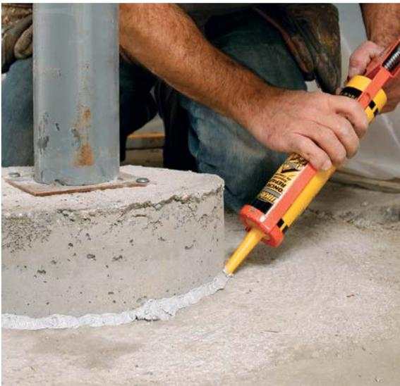
**FINISH THE PIER.** Remove the exposed builder's tube by scoring it with a utility knife where it meets the slab. Masonry caulk, such as Quikrete® concrete repair ([www.quikrete.com](http://www.quikrete.com)), cleans up and protects the seam.
