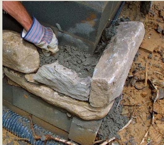
**PACK MORTAR BEHIND THE STONES.** Mortar holds the stone in place, and wall ties embedded into the mortar tie the stone veneer to the block wall. Lay a mortar bed on top of each stone course for the next course.
