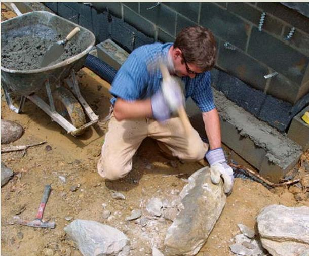
**TRIM ROCK WITH A BLUNT HAMMER.** Break bumps off the back and bottom to improve fit and to reduce the chances that the stone will move as rocks are piled on top of each other.
