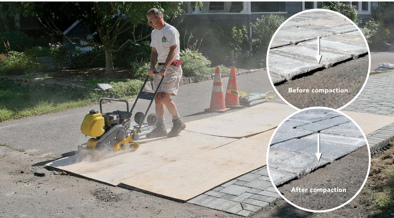
**POUND 'EM DOWN.** With a layer of plywood as protection, use a plate compactor to set the pavers firmly in the sand bed.
