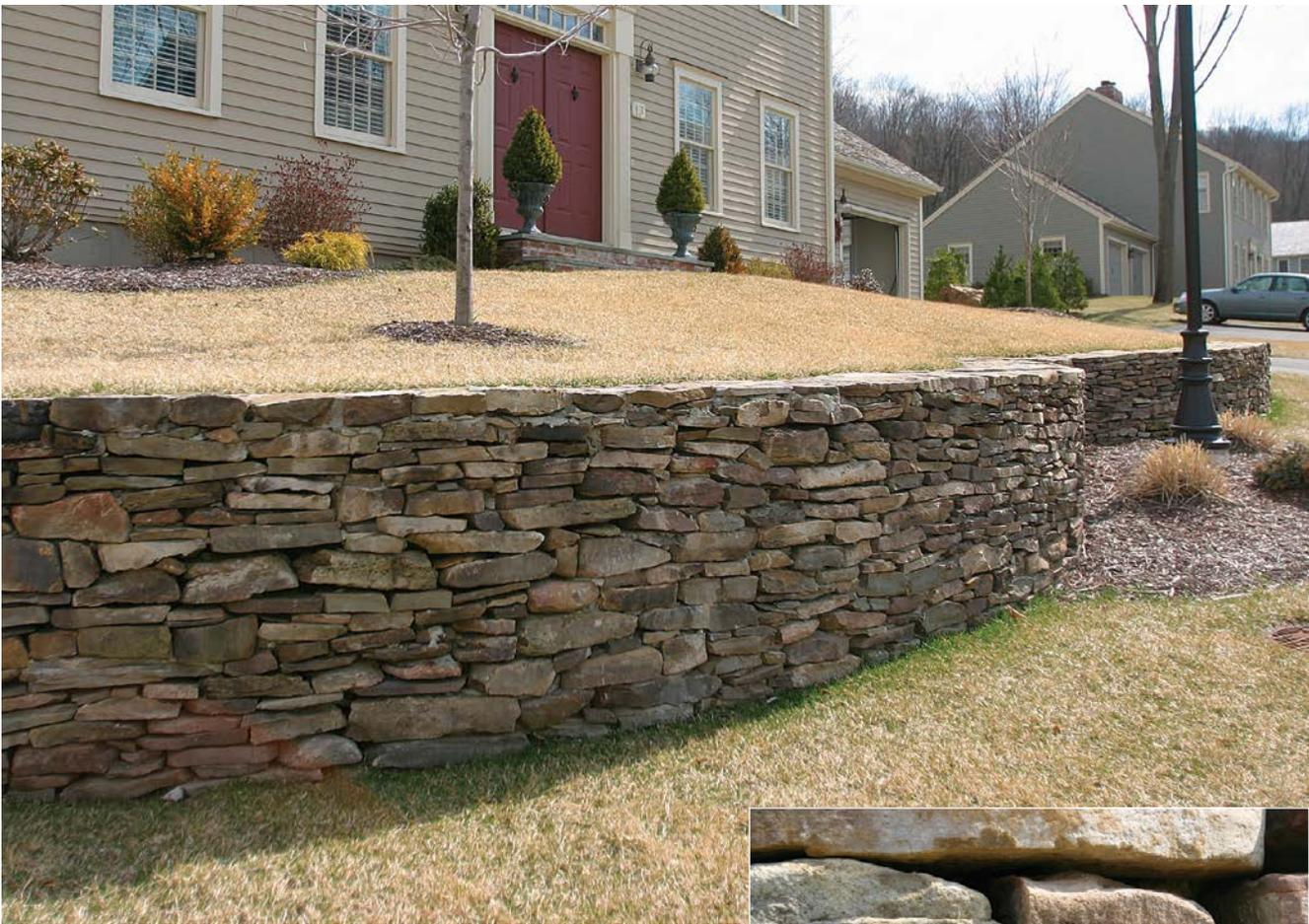
**STONE WALLS CAN BE DECEIVING.** From a distance, this stone retaining wall appears dry-stacked. A closer look reveals that the stones actually are mortared. Mortared backfill is a good idea for taller walls or walls that will be walked on or sat on.
