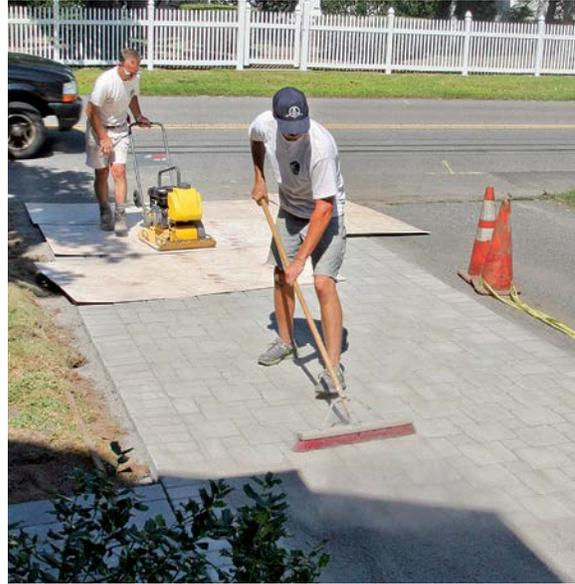
**FILL THE JOINTS AGAIN.** Sweep in more joint filler after compaction to bring it up to the level of the pavers.
