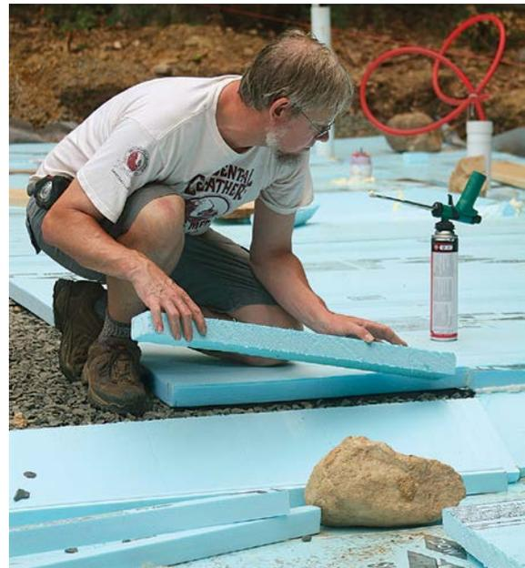
**LAYING DOWN FOAM IS DIRTY SIMPLE.** Make sure the foam fully contacts the gravel. Foam sheets don't need to fit tightly. Gaps can be filled with scrap pieces and spray foam.
