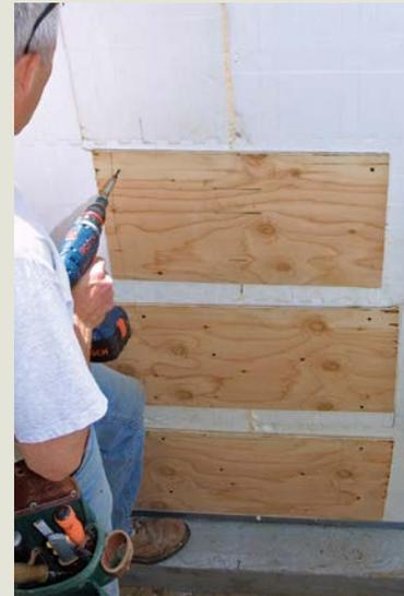
**PLYWOOD BANDAGES.** After gluing large vertical seams with foam, reinforce them with plywood scabs screwed to the embedded fastening strips found on both sides of the seams.
