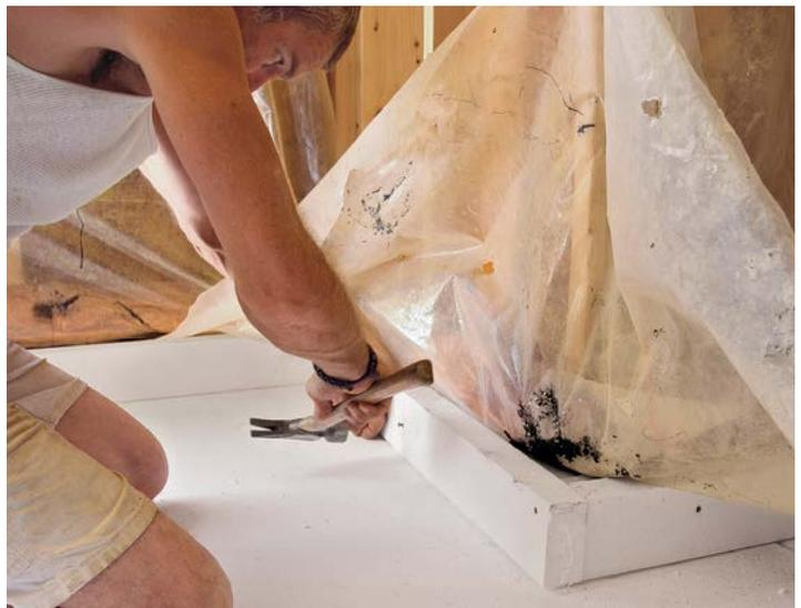
**TACK ON THE EDGE.** The innermost pieces of perimeter foam come last and act as the screed level for the concrete slab. After applying a bead of spray foam to the outer perimeter foam, a worker tacks the inside pieces to that first layer of foam with nails every few feet to keep them from shifting until the spray foam sets up.
