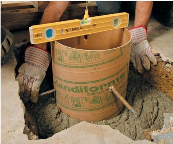
**CREATE THE PIER SUPPORT.** Into the wet concrete, set a 16-in.-long, 12-in.-wide builder's tube fitted with two pieces of rebar that protrude 6 in. from each side, and level it. The exposed rebar, which sits a few inches below the height of the slab surface, helps tie the pier to the rest of the footing.
