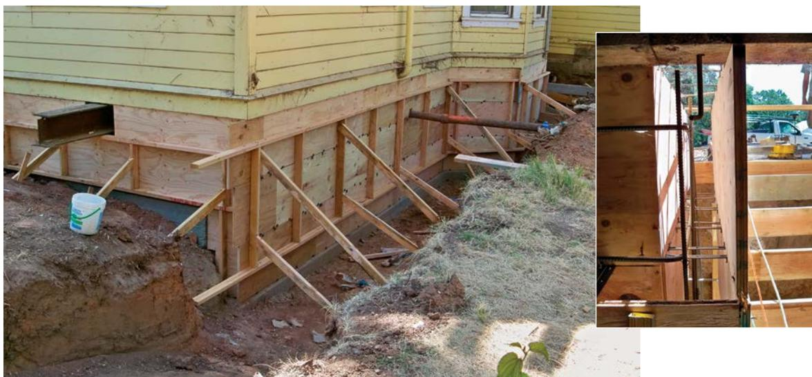
**ON THIS PROJECT, WE BUILT 140 LIN. FT. OF FORM** using 2×4s for walers, 1½-in. plywood, and snap ties. You can certainly sub out this work, but building forms goes quickly. I've found that building forms costs less than hiring a concrete subcontractor to do the work.
