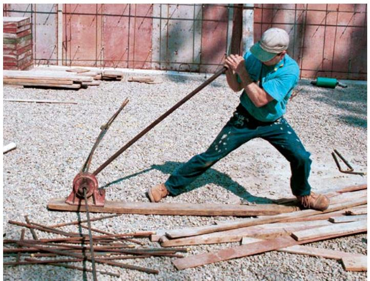
**ALTHOUGH CHOPSAWS OR TORCHES** can make quick work of cutting rebar, at a site without electricity, the stock can be cut with the cutter/bender.
