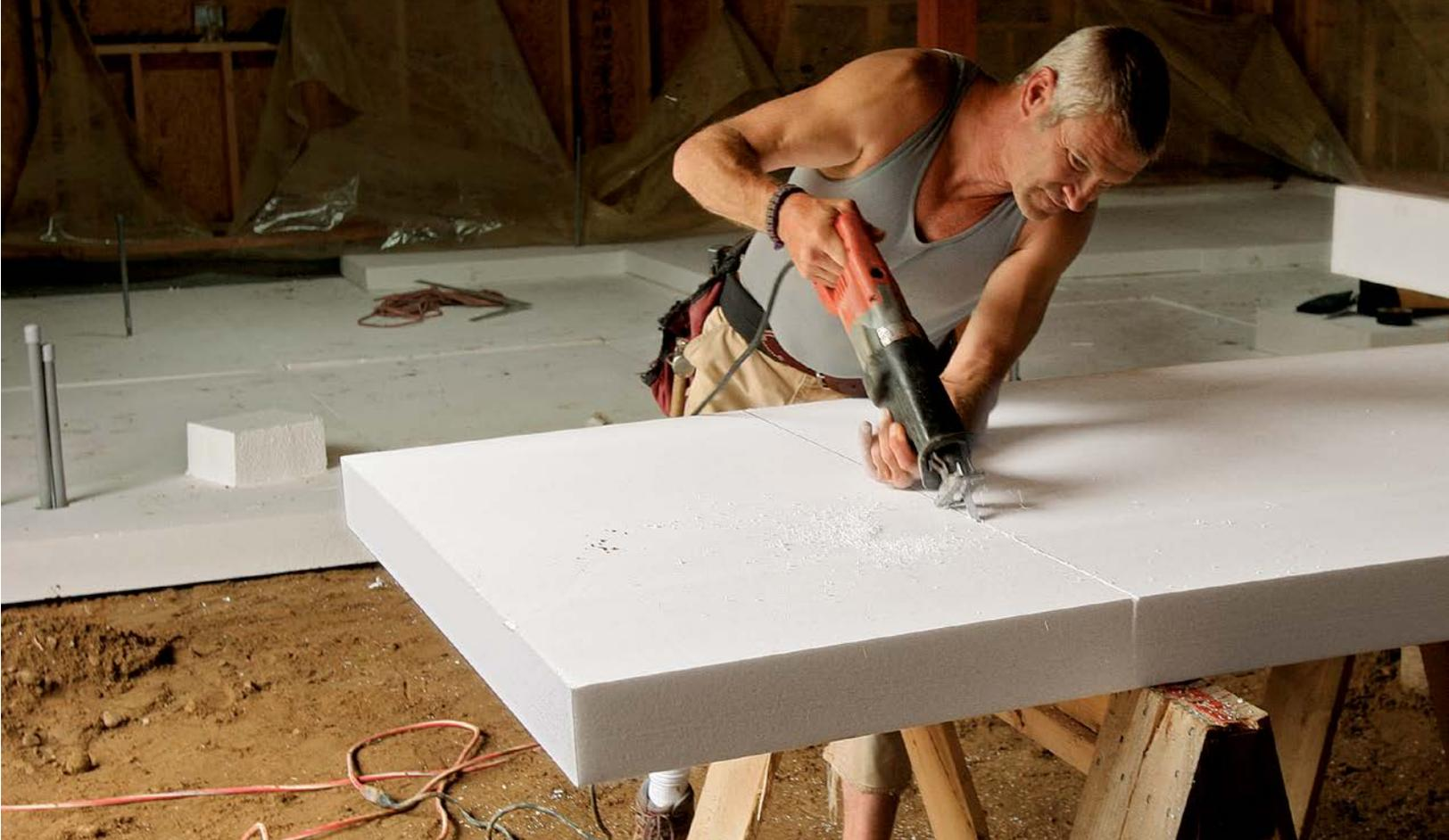
**THICK FOAM MEANS NEW TECHNIQUES.** Because the dense foam panels are too thick to be cut with a tablesaw or circular saw, the builders rely on a reciprocating saw with a 12-in. coarse-tooth blade for making crosscuts, rip cuts, and notches.
