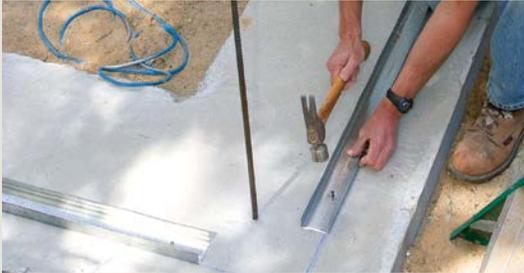
**ANCHOR THE FIRST COURSE OF ICF BLOCKS** by fastening steel track along the chalklines with 1-in. masonry nails spaced 2 ft. to 3 ft. o.c. (left). I set the corners of each course first to eliminate any need to cut, and thereby weaken, this structurally vital part of the foundation (below).
