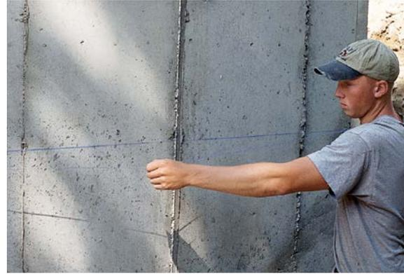
**THIS WALL WAS DAMPPROOFED** using a spray-on product called Pene-Krete® ([www.super-krete.com](http://www.super-krete.com)). If using a dampproofing membrane, stop it 4 in. below final grade. Reduce installation errors by snapping a chalkline on the foundation wall at this height.
