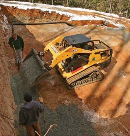
**GRAVEL DEPTH VARIES DEPENDING ON SOIL TYPE.** In this case, the gravel footing is 4 in. thick. A perimeter drain is buried in the footing to direct groundwater away from the foundation. The pipe extends to the steep drop-off at the right edge of the photo.
