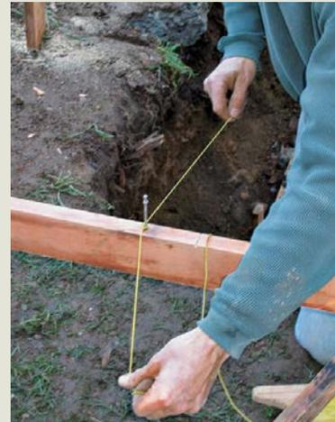
**WHEN THE STRING IS BANJO-TIGHT**, pull the free end back toward the nail. The twists will ball up into a knot. To loosen, pull the free end in the opposite direction.
