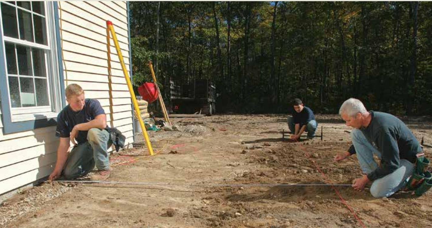
**2 THE PIER CENTERLINE RUNS PARALLEL TO THE HOUSE.** The batter boards I use make it easy to adjust the string line until it's exactly the right distance from the house foundation. I set the batter boards a couple of feet beyond the corner-pier locations so that the boards won't be disturbed when holes are dug.
