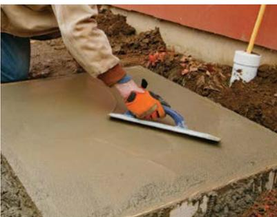
**9 SMOOTH THE RAKE MARKS WITH A MAG FLOAT.** Keep the leading edge of the float up. When the surface water dissipates, float the slab again. This is the final finish for exterior slabs. For a smooth interior slab, work it again with a steel float when the surface begins to lose its wet sheen.
