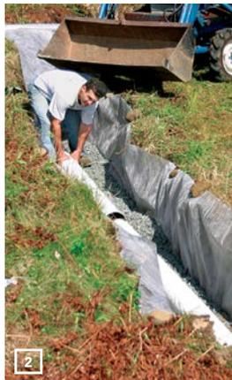
**SET THE PIPE IN A BED OF GRAVEL.** Filter fabric lines the trench to keep silty sediment from clogging the pipe. You can adjust the pitch of the ditch before laying the pipe by varying the thickness of the gravel layer.
