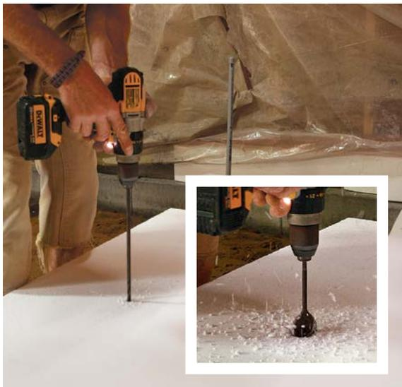
**DRILL FROM BOTH SIDES.** When you need to drill holes for pipes and other penetrations in the thick foam, a standard spade bit or hole saw won't be long enough. Instead, use a long bellhanger-style drill bit to bore a pilot hole all the way through the foam. Then, using a standard spade bit, widen the pilot hole from both sides of the panel. For holes of a larger diameter, skip the drill bits and go right for the reciprocating saw.
