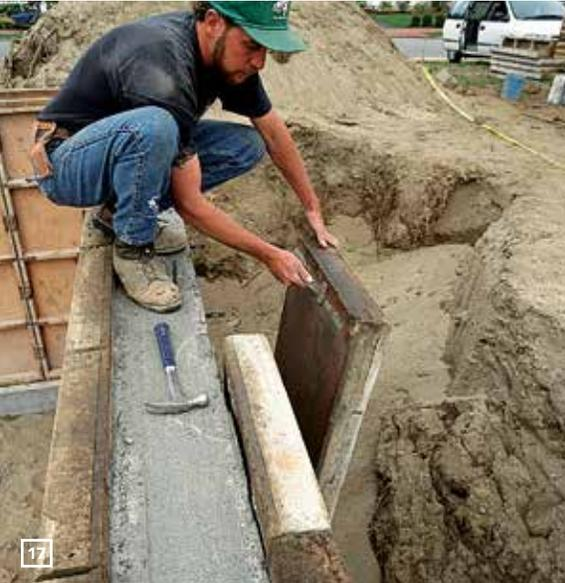
**17 AS EACH FORM IS REMOVED**, excess concrete along the top is scraped off.
