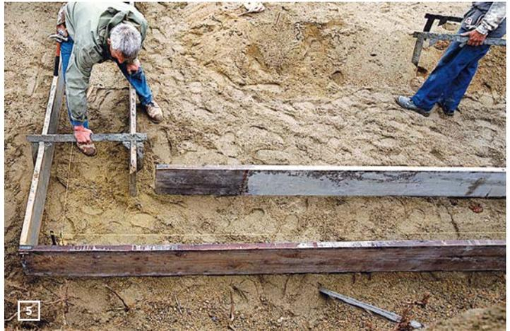
**4** OUTSIDE FORMS ARE SET UP FIRST. Starting at one corner, the outside forms are set at a given distance off the foundation line.
