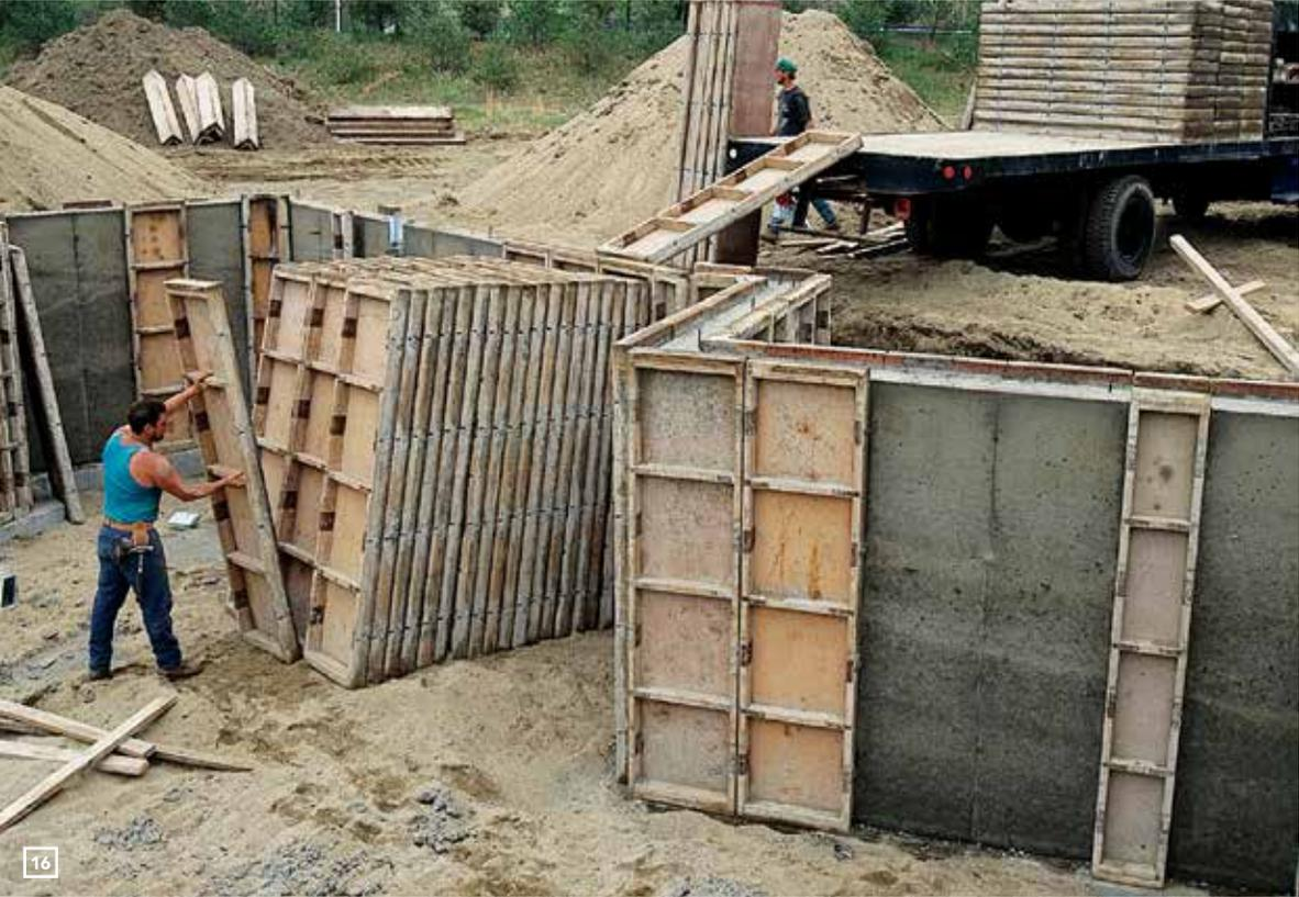
**16 FORMS ARE STRIPPED** and carried to the truck. After the concrete has cured overnight, the crew strips off the forms and takes them to the truck to be stacked.
