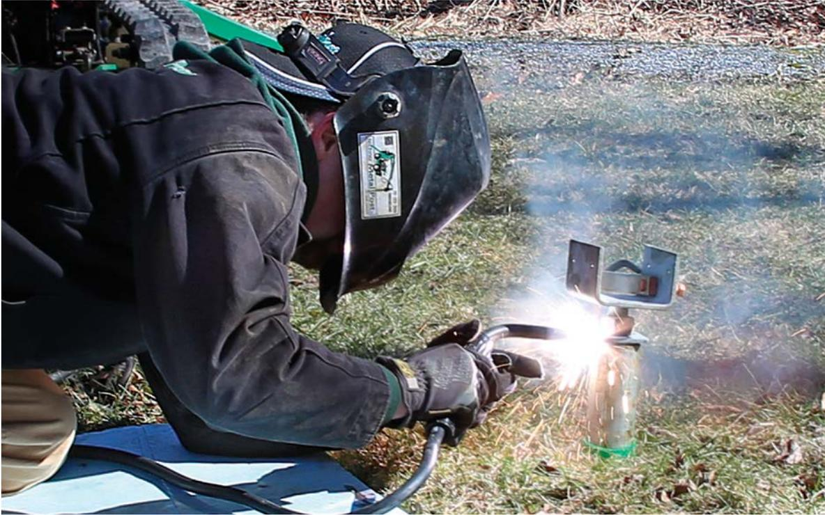
**WHERE THE METAL HITS THE WOOD.** Providing bearing and uplift resistance is only half the battle. You also need to attach the helical pile to the structure, and that requires some kind of cap. A welded connection between the head and the pile transfers lateral and uplift loads from the structure to the pile.
