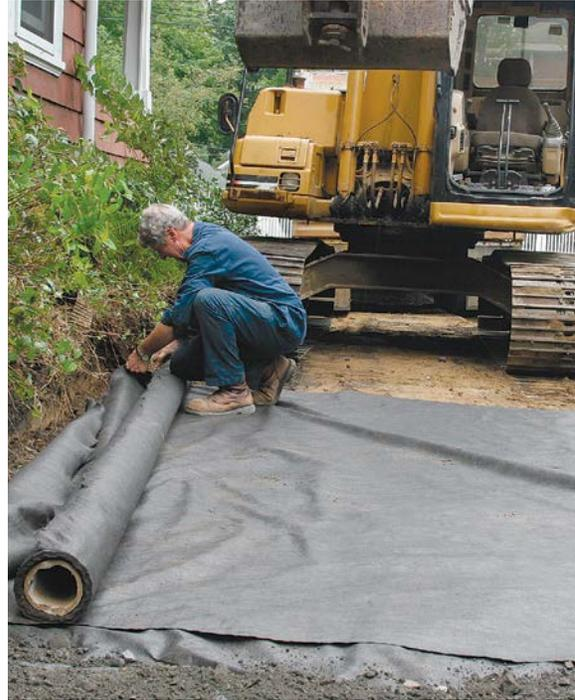
**GEOTEXTILE SEPARATES THE LAYERS.** The main purpose of geotextile is to prevent the crusher run from mixing into the subgrade over time and losing its bearing capability.
