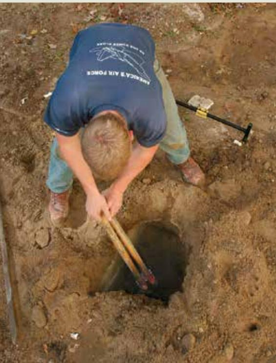
**5** **THE BEST HOLES HAVE NO ROCKS.** But just in case you encounter a few, make sure to have a long digging bar in addition to a post-hole digger. Take care not to disturb the batter boards or their settings because you'll have to reattach the string lines later. Dig down deep enough so that the bottom of the pier rests on undisturbed soil below the frost line.
