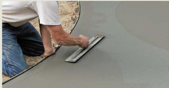
**FINISH WITH A STEEL TROWEL.** The final finishing tool is a large steel trowel, which forces the cream back down into the surface for a smooth, durable finish. Trowels with curved corners are less likely to leave tracks.
