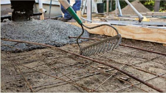
**PULL UP THE REINFORCEMENT.** You can place rebar and reinforcing mesh on small metal stands, called chairs, ahead of time or you can raise them as you spread the wet concrete.
