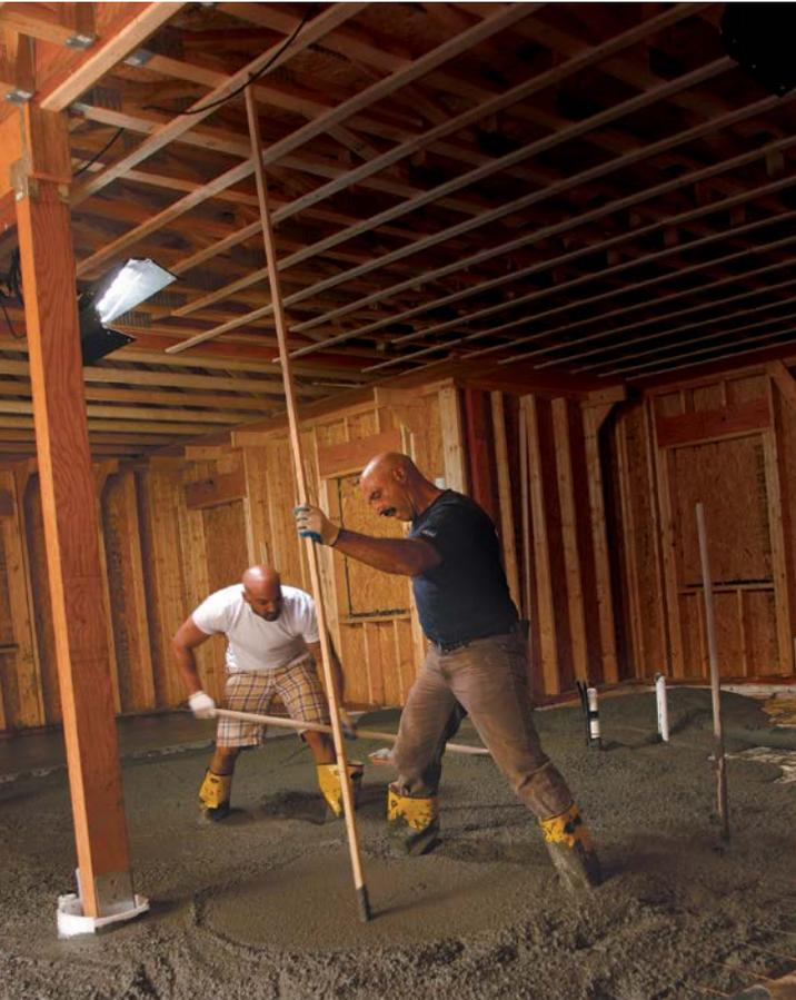
**GRADE DOWN FROM ABOVE.** As the pour progresses, the concrete crew uses a reference stick placed against the ceiling joists to establish the surface of the slab. Working in a small area, the crew adds or removes concrete until the stick just brushes the surface. The area is then marked with an X and used as a reference when screeding the slab surrounding it.
