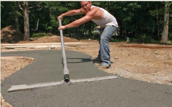
**BULL FLOAT FIRST.** Take two or three passes with a magnesium bull float to level the surface and to push the aggregate into the mix. Raising the leading edge of the float will prevent it from digging into the surface. Additional handle sections provide extra reach on large pours.
