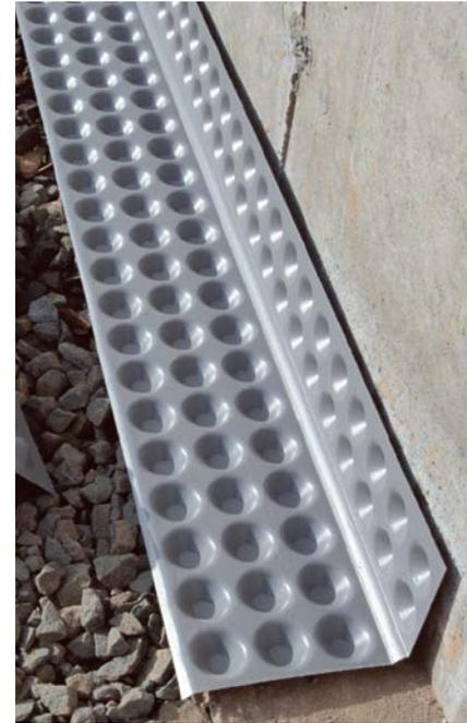
**DRAINAGE FLASHING IS A SIMPLER, LESS-EXPENSIVE INTERIOR DRAIN.** Installed at the junction of wall and footing, this flashing has a dimpled profile that allows any water from the walls to flow beneath the slab and into the sump pump. Obviously, it's important to keep the top of the flashing clear when pouring the slab (left).
