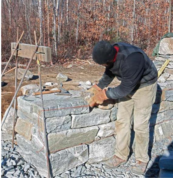
The best stones for ends are long and large with flat and parallel top and bottom surfaces. Cube-shaped stones won't tie back and will force the creation of a running joint in at least one direction on the next course. The contact points below each stone should be close to the outside corners. You will likely need to shape stones used in wall ends and corners, so plan to spend time on these features.
