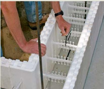
**ZIP TIES SECURE THE CORNERS.** Because the corners are the weakest points in the form assembly, it's important to secure corner blocks to adjacent straight blocks with plastic zip ties.
