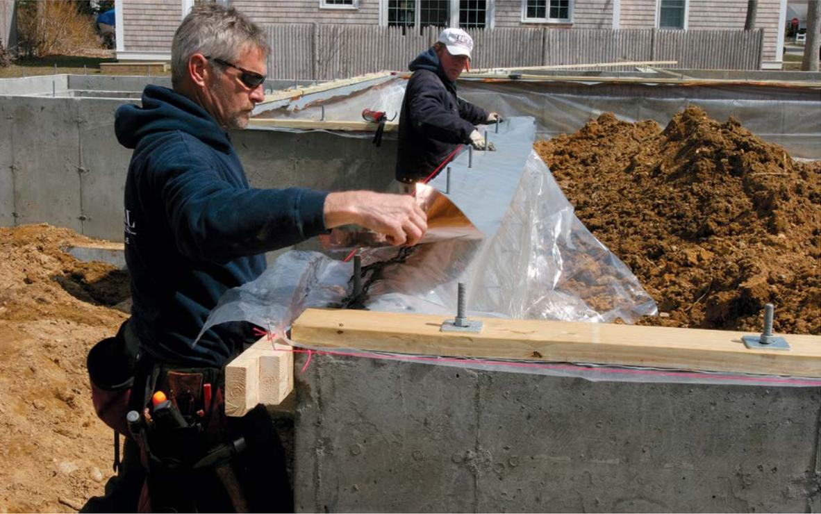
**TERMITE SHIELD.** Another bead of acoustical sealant is laid across the top of the poly before the termite shield, a copper-polymer composite membrane called YorkShield 106 TS™ ([www.yorkmfg.com](http://www.yorkmfg.com)), is placed over it.
