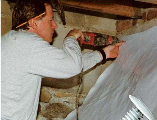
**HOLES ARE DRILLED THROUGH THE LINER** into the foundation (above), and nylon expansion fasteners are driven into the holes (top right).
