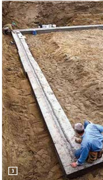
**1 LOCATE THE FOUNDATION CORNERS.** Working on the floor of the foundation hole or on top of the footings, you first have to find the outside point for every corner or jog in the foundation.
