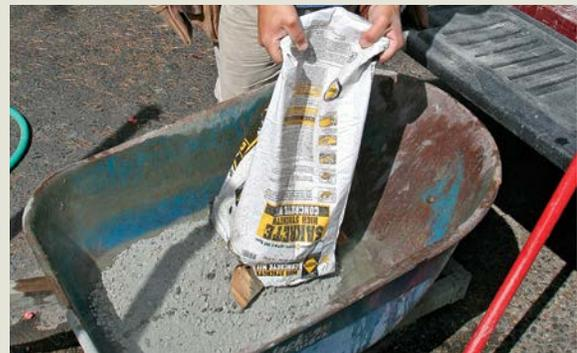
**2 ADD THE CONCRETE.** Place the unopened bag in the water. Then use a utility knife to open the bag with a single cut along the end. Grab the bottom of the bag and tip it up so that the concrete slides out rather than pours out. This technique minimizes dust.
