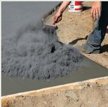
**APPLY RELEASE AGENT.** Before stamping, cover the entire surface with a release agent. Shaking it on with a broom is fast and easy, but be careful not to hit the wet concrete with the bristles.
