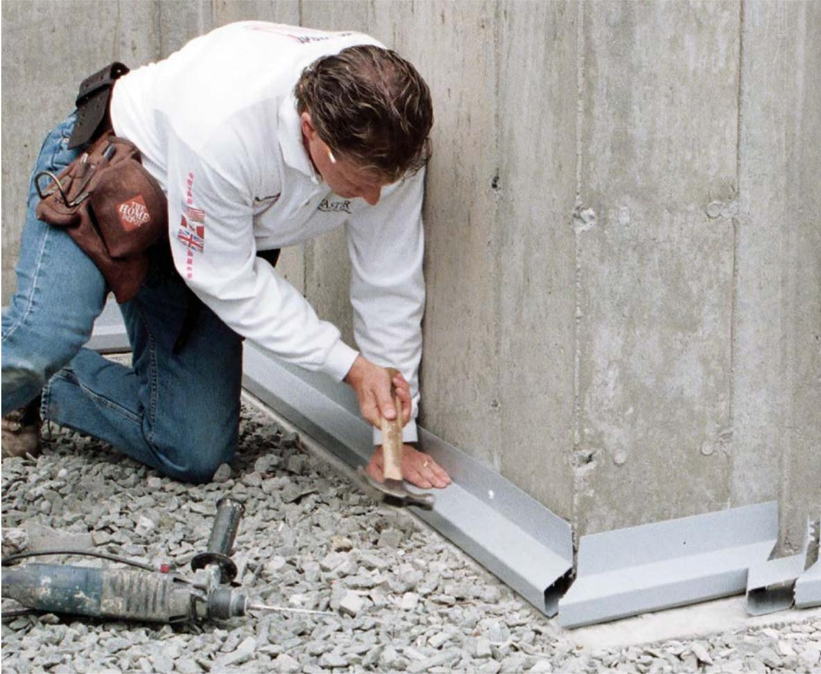
**INTERIOR PERIMETER DRAINS ARE GOOD INSURANCE** in new construction or retrofits. Plastic drains on top of the footing collect water that leaks in through the walls and channel it to the sump pump. The entire drain is to be covered with concrete, except the opening facing the wall.
