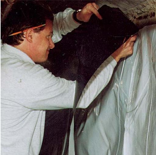
**TO KEEP WATER AND INSECTS AWAY** from floor framing, the liner is cut in place 2 in. below the top of the wall.
