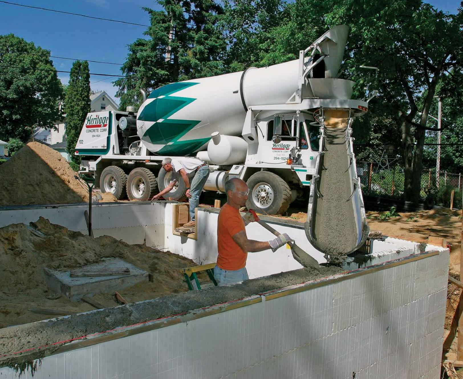
stronger the concrete. The primary characteristic that you need to consider is the required strength for the use, which is measured in pounds per square inch (psi). Concrete with a psi of 3,000, for instance, will withstand 3,000 lb. of compression per square inch before breaking.
