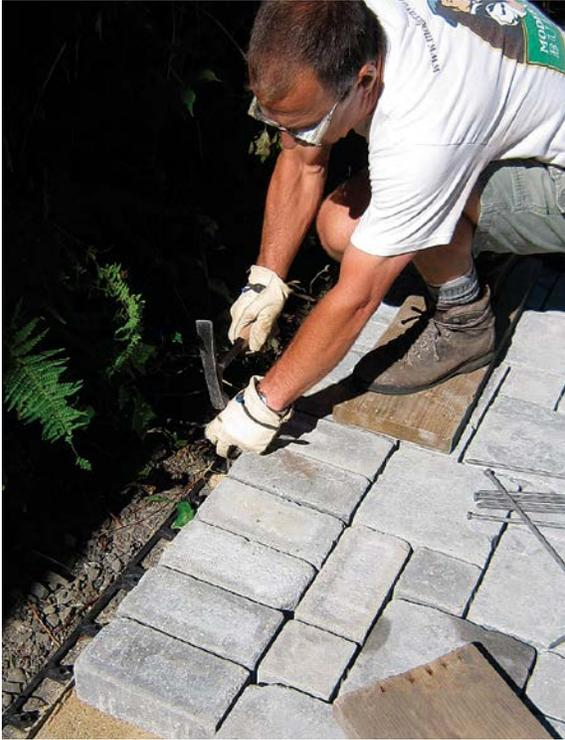
**INSTALL EDGING.** Spike plastic edge restraints to the ground as the job progresses.
