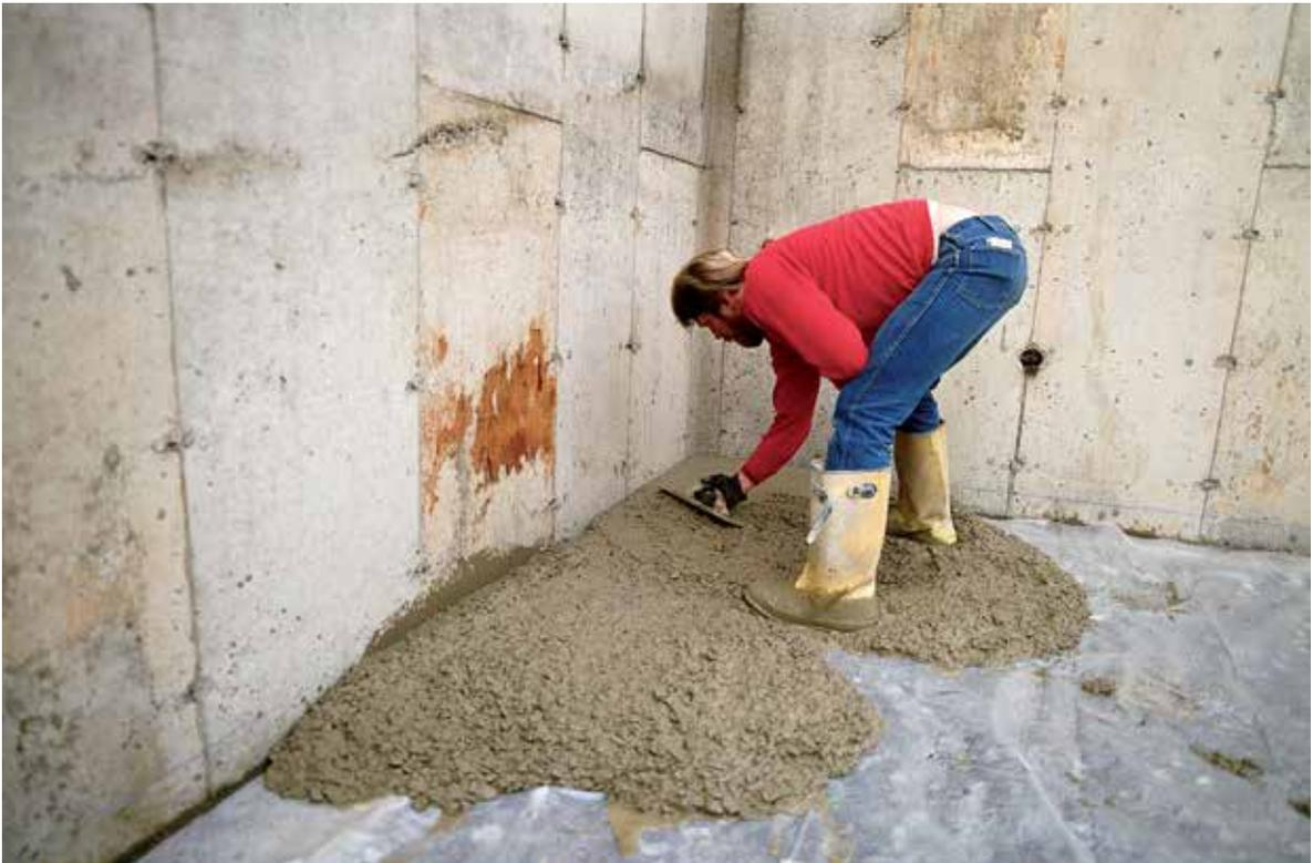
**ESTABLISHING A PERIMETER SCREED.** A magnesium hand float is used to push the concrete up to the chalkline. This strip of wet concrete, placed along the foundation walls, is a perimeter screed.
