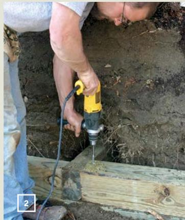
Drill pilot holes so that spikes or rebar can be driven easily, with less chance of splitting.
