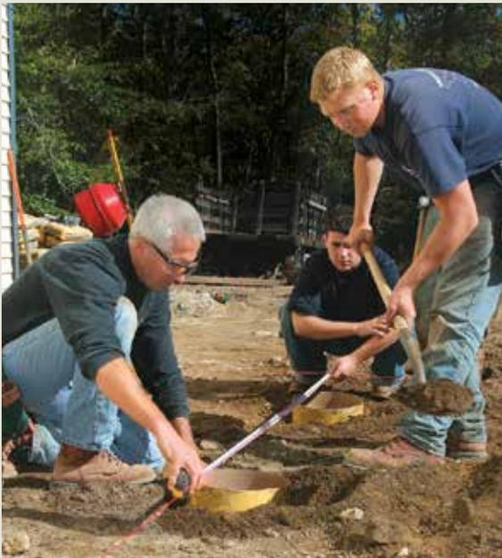
**1 BACKFILL WITH MEASURING TAPE AND SHOVEL.** I cut the builder's tubes so that they stick out a few inches above grade when placed in the hole. To make sure a tube is placed precisely, I hold it on its layout while a helper backfills. Pack the soil around the tube every so often as you go.
