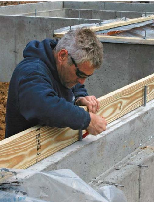
**PREP THE PLATE.** To locate the bolts accurately, the mudsill is laid on edge across the top of the stemwall, and each bolt location is scribed onto the face of the 2x6.
