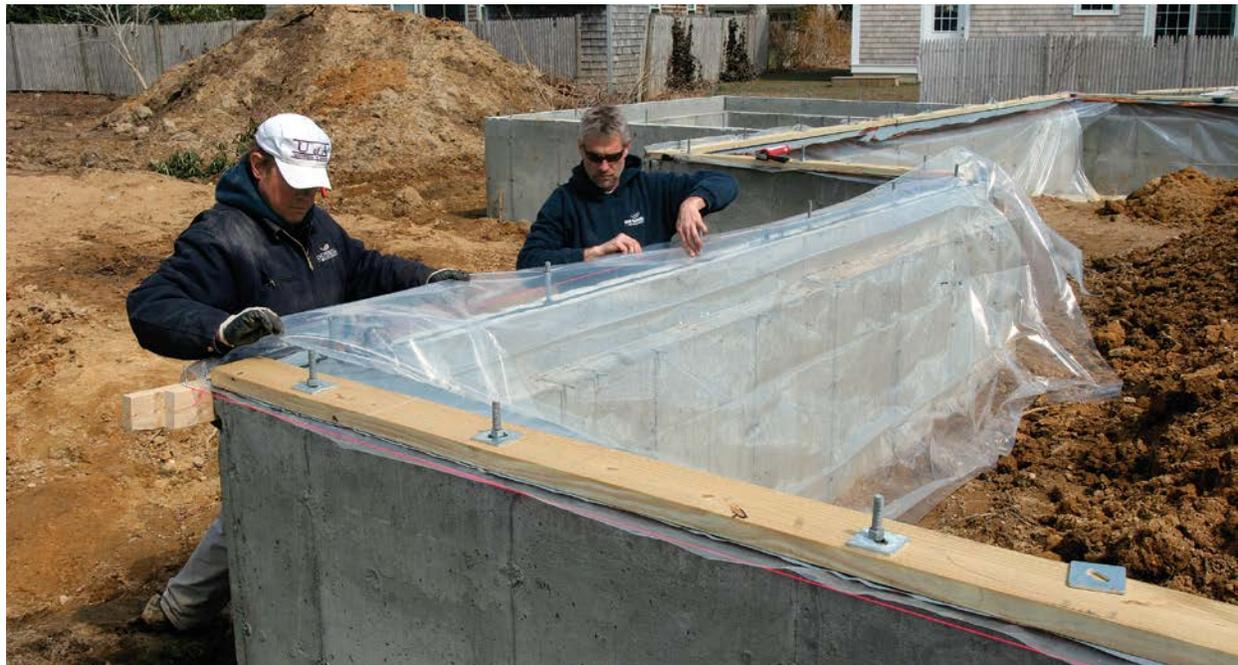
**PLASTIC COMES FIRST.** After applying a thick, continuous bead of acoustical sealant to the top of the concrete, the carpenters lay the poly vapor retarder in place. They use hand pressure to push it firmly into the bead of sealant.
