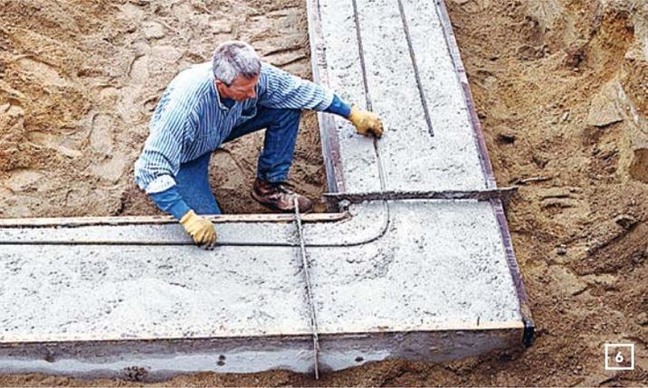
**6 REBAR IS INSERTED INTO THE WET CONCRETE.** The footing forms are filled to grade, and the concrete is worked with the flat side of a shovel until the footings are level. Then ½-in. rebar is pushed down into the fresh concrete.
