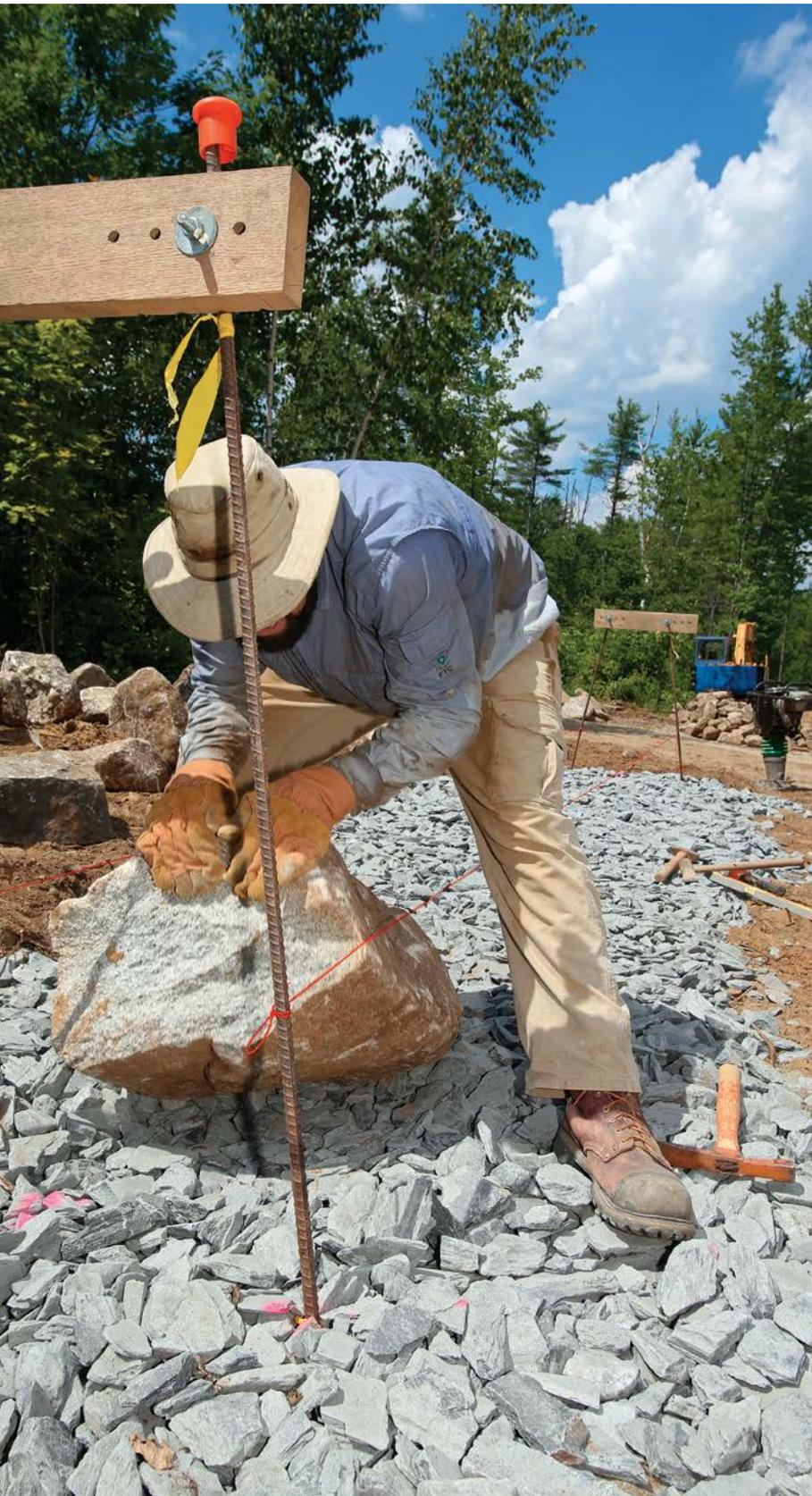
**LEFT: TIE STRINGS TO THE FRAMES.** Set strings level with each other, just above course height. Sight between the string and batter frame to locate the edges.
