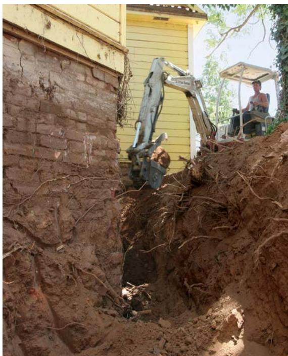
**WE CREATE A TRENCH WIDE ENOUGH**, about 6 ft., to allow the Bobcat to drive down to the grade of the slab. This makes removing the old foundation material a lot easier. It also creates a large, safe working zone for those building the new footings and foundation walls.
