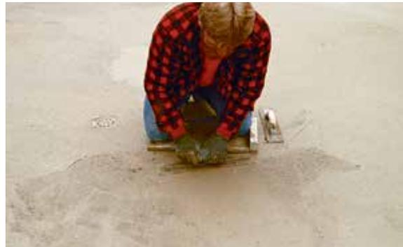
**TWO HANDS! TWO HANDS!** As the concrete sets up, working it with a steel trowel may require the strength of two hands. The back of the trowel is angled up as you push it away (left), and the front of the trowel is angled up as you pull it toward you (right).
