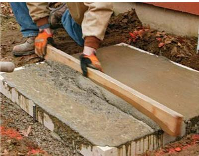
**7 SCREED THE SLAB.** Flatten the concrete using a straight 2x4 that's about 1 ft. longer than the form width. Move the board forward with a back-and-forth sawing motion while keeping it on the form.
