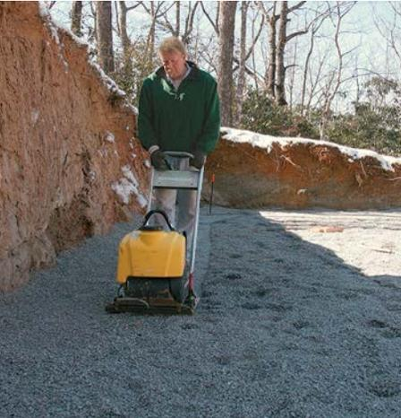
**A GAS-POWERED COMPACTOR** is used along the perimeter of the foundation line. Because the foundation crew does the fine-tuning, the gravel needs to be within only 1 in. of level.
