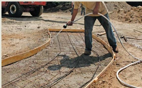
**WET THE GROUND.** Concrete needs adequate water to cure properly. Prevent water from being drawn out of the concrete by thoroughly wetting the ground just before you start pouring.
