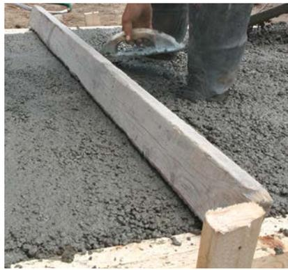
**4 FILL AND SCREED.** Fill the forms so that the wet concrete is just over the tops of the forms, then screed off the excess, using the forms as a guide. A helper or two moving concrete ahead of the screed makes this process easier.
