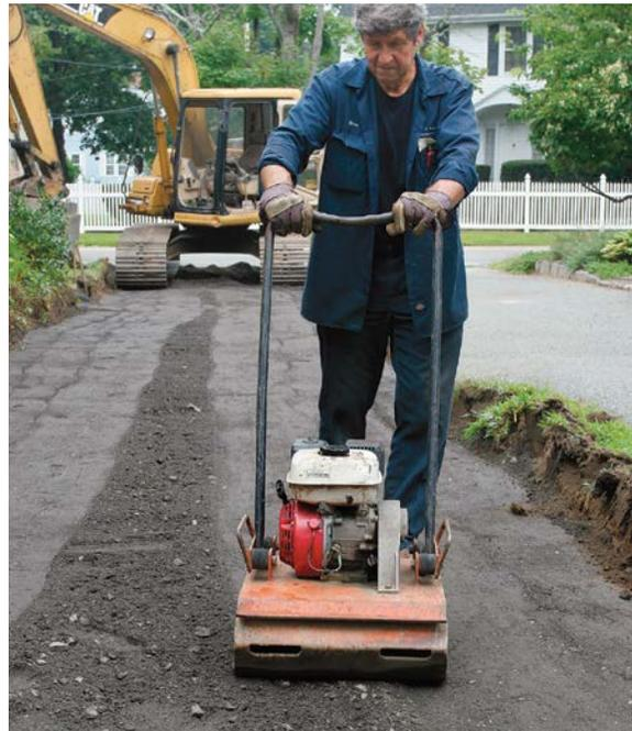
**TAMP TO PREVENT SETTLING.** Place the crusher run in two 4-in.-deep lifts. Compact the first lift, then place and compact the second.
