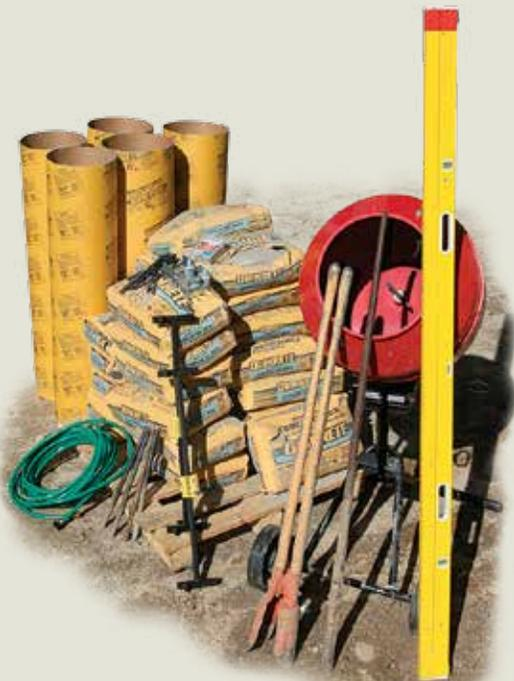
Rather than try to cut tubes to the exact height, I leave them long and pour concrete to the desired height inside the tube. In most cases, I like the pour to come a couple of inches above the finished grade. If the piers are on a pitched elevation, the tops of the piers won't be level with each other. On this job, the finished grade was level, so I used a long level to carry the elevation across the piers.
