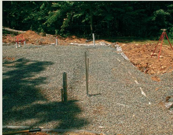
**GRAVELED AND READY FOR FOAM.** Strings between batter boards define the foundation perimeter. Conduit for electrical and phone lines is in the front, while stubs for plumbing stick up in the back. Perimeter drains are visible along the right.
