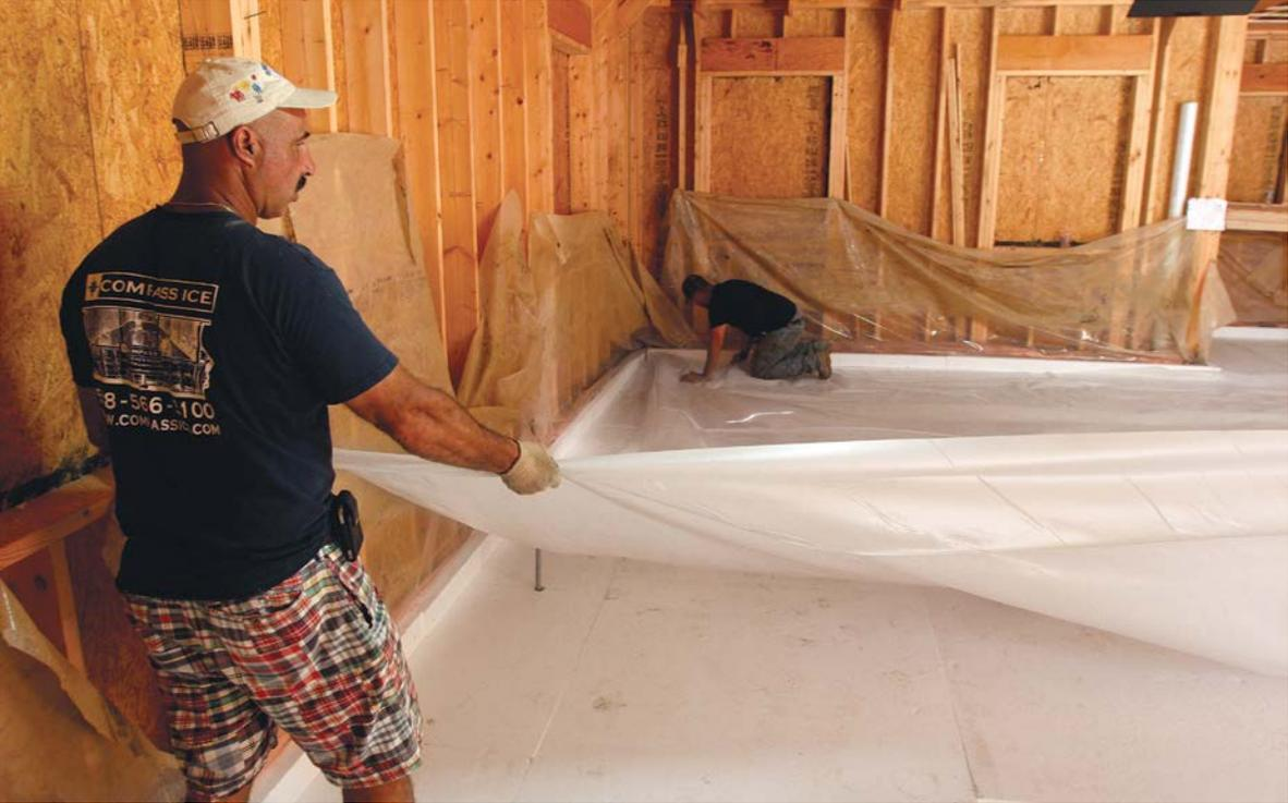
**ABOVE: TAPE TO AVOID ICEBERGS.** After laying out the poly vapor retarder over the foam base, the inner flap of the poly that was installed as part of the mudsill assembly is folded down and taped along all edges. This taped seam prevents concrete from getting under the foam panels and causing them to float—a hard-learned lesson from one of the architect’s previous projects.
