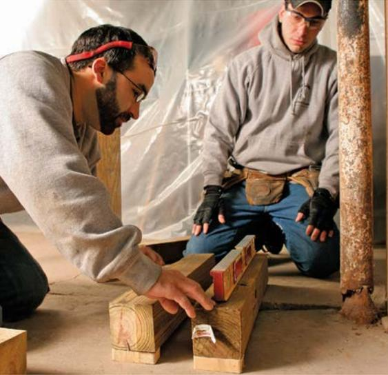
**START LEVEL, STAY STRAIGHT.** Use small scraps of lumber to bring two 3-ft.-long 4×4 pieces of pressure-treated lumber to level. The next two pieces are stacked perpendicular to the first two. The top layer then is screwed to the bottom.
