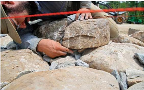
**TOP: TIE THE SIDES TOGETHER.** It's typical to let through-stones extend 1½ in. past the wall face to allow for flexibility in their length and for the wall to settle without slipping off them.
