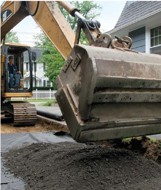
**SPREAD THE CRUSHER RUN.** A mix of stone from  $\frac{3}{4}$  in. to dust, the crusher run helps to spread the loads from the pavers above to the subgrade below.
