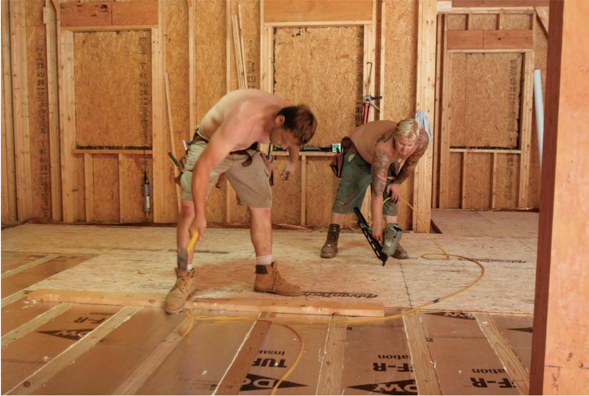
**INSULATED SUBFLOOR.** Using powder-actuated nails, the builders fasten pressure-treated 2×4 sleepers to the slab at 16 in. on center. To increase the overall R-value of the floor system, they fit pieces of rigid foam between the sleepers and fill remaining gaps with expanding foam. Finally, they fasten the ¾-in. subfloor.
