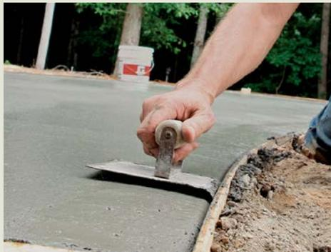
**EDGE THE CORNERS.** After mag floating, use an edging tool on the slab corners. Rounded edges resist weather better than do sharp corners.
