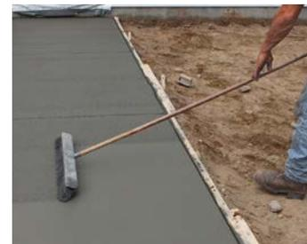
**8 BROOM FINISH FOR TRACTION.** Special concrete brooms exist, but a regular push broom with stiff bristles works fine too. Keep the texture perpendicular to the traffic direction. Once you've finished brooming, go over the corners and control joints again.
