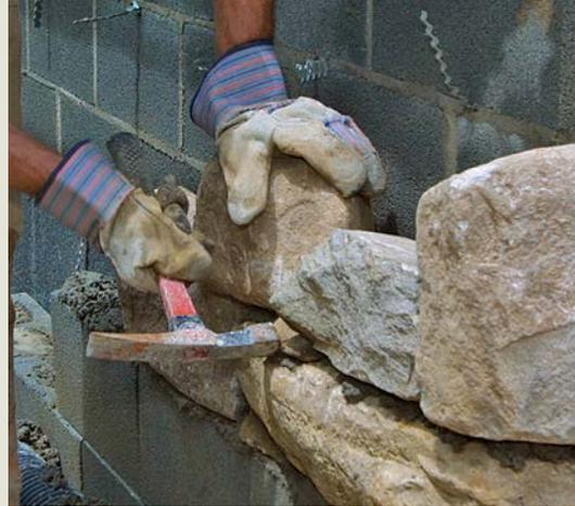
**USE SHIMS TO SET THE STONES MORE SECURELY.** The rock-fragment shims can be used in one of two ways: either as temporary shims until the mortar sets up or as permanent plugs to fill gaps between stones, giving a tighter appearance.
