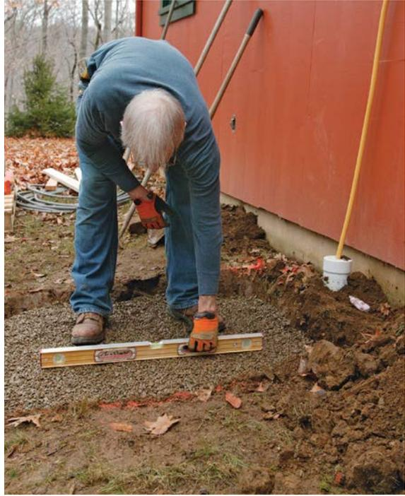
**2 GRADE THE GRAVEL.** Fill the excavation with 4 in. of gravel. Rake it flat, and use a level to make sure it's pitched about  $\frac{1}{4}$  in. per foot so that the slab, which will parallel the base, drains water.
