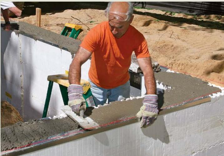
**SMOOTH THE SURFACE.** Once the walls have been topped off, use steel track as a guide to remove excess concrete and to smooth out the surface before inserting anchor bolts.
