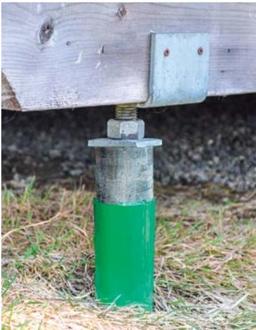
**SADDLE UP.** This U-shaped bracket makes a stout attachment for a deck beam.
