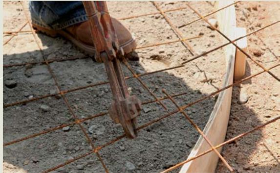
**ADD REINFORCEMENT.** Place sections of reinforcing mesh so that the panels overlap by 6 in., and cut away the excess so that the wire is about 2 in. away from the sides of the form. Then put in rows of  $\frac{3}{8}$ -in. rebar spaced about 1 ft. apart. Overlap the bars by 1 ft. and tie them together at both ends of the overlap.
