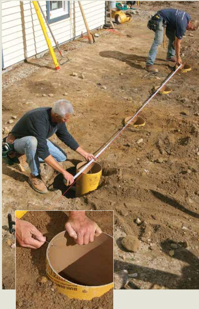
**2 DOUBLE-CHECK THE CORNERS.** I spend a little extra time checking the location of the final corner pier to make sure that it's in the right spot because I won't get a chance to move it once the concrete is poured. Use a nail to mark the finished height of the piers, keeping it a couple of inches above the finished grade. If you need to have piers all at the same height, use a long level or a transit to locate their finished height.
