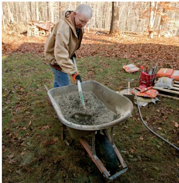
**4 MIX THE CONCRETE.** Dump two 80-lb. bags of mix in a wheelbarrow for each batch. Add 3 qt. of water per bag, and mix thoroughly with a hoe. Add small amounts of additional water if necessary to bring the concrete to a consistency that's about the same as thick cake batter.
