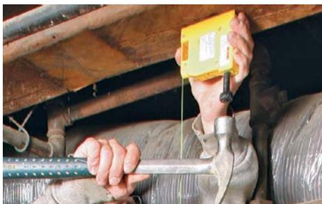
**TAP IT INTO PLACE.** After cutting the column to length (be sure to consider the thickness of the plates when measuring for length), place the column on the bottom plate. Add the top plate to the column, and tap the assembly into place with a sledgehammer. Check to be sure the column is plumb.
