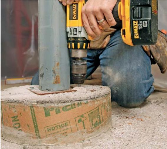
**SECURE THE PLATES.** Drill pilot holes through the screw holes of the bottom plate, and secure the plate with 3-in. Tapcon® screws or concrete anchors. Attach the top plate to the beam with 2½-in. lags, never with nails.
