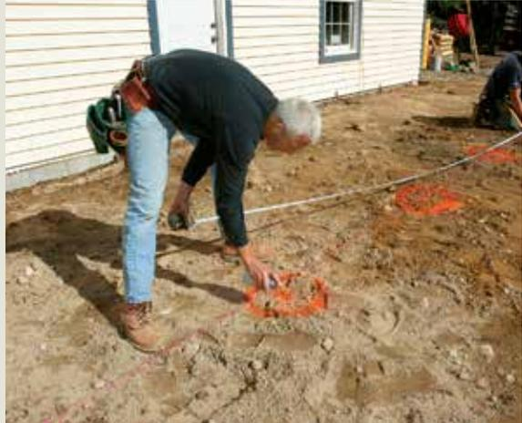
**4** **MARK PIERS WITH PAINT.** Measure the remaining piers from the far-corner pier. A dot marks the center point, and a rough circle highlights where to dig. Pull the string lines and prepare to dig, but keep the batter boards in place.
