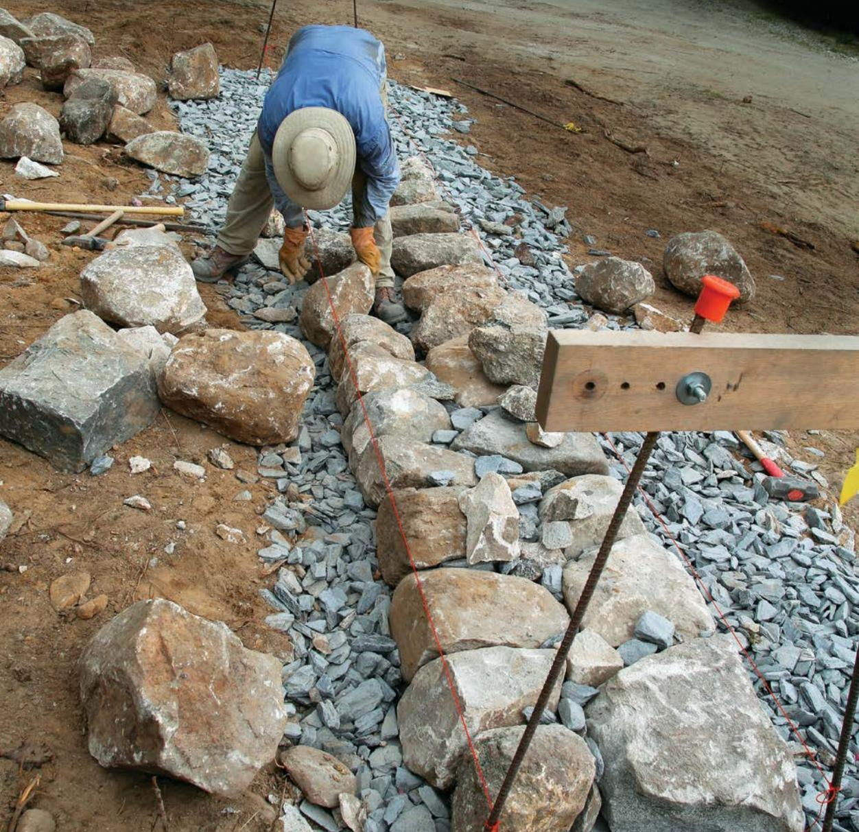
**ABOVE: START BIG.** Roll foundation stones into place and level their tops by digging into the soil or gravel below.
