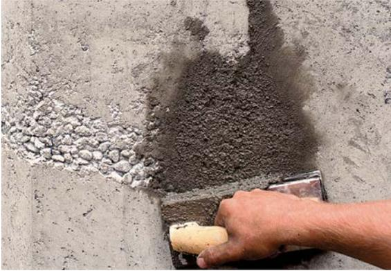
**I SPECIFY THE DRIEST CONCRETE MIX** that my plant will supply for optimum strength and that will cure properly in my climate, which usually demands the use of additives. Drier concrete, however, sometimes leads to small voids in the wall after the forms are stripped.
