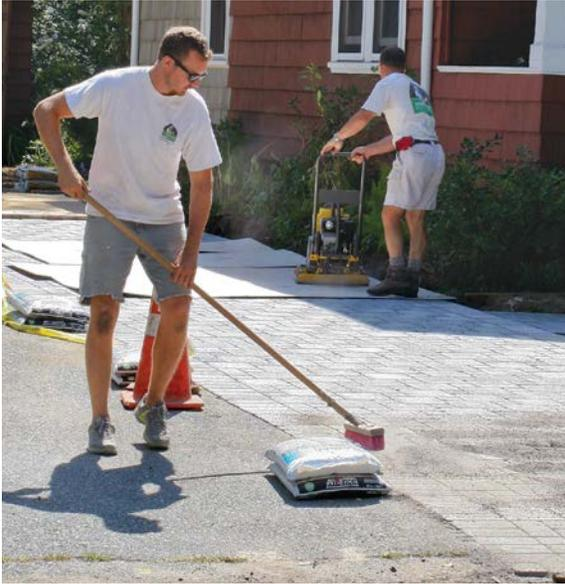
**FILL THE JOINTS.** Sweep a graded material such as fine stone dust over the pavers until the joints are full.
