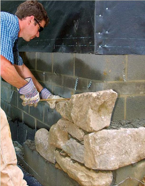
**KEEP THE ROCKS PLUMB.** Regardless of how thick the rocks are, the faces should be in the same plane. If the foundation wall is plumb, you can measure to the face of the rocks consistently.
