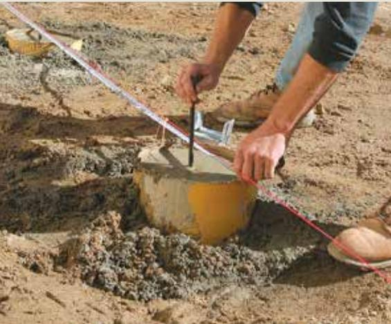
**4 PLACE ANCHOR BOLTS ACCURATELY.** Once all the piers are poured, I go back and insert anchor bolts in the center of the piers. I measure from the line running perpendicular to the house to set anchor bolts accurately. Be sure to leave the threads high enough so that a post base, washer, and nut can be added later.
