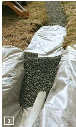
**KEEP THE FABRIC NEAR THE SURFACE.** The top layer of filter fabric eventually clogs. If that top layer is close to the pipe, you'll have to do a lot of digging to fix the problem. By folding the fabric over the gravel a few inches below the surface, you leave it accessible.
