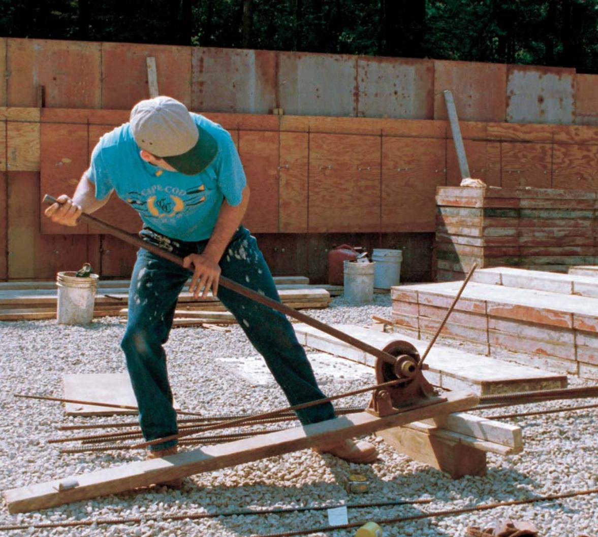
**CUTTING AND BENDING REBAR** is a matter of leverage and muscle. The cutter/bender's head provides a lever and fulcrum that makes simple bends; more complex bends can be made from individual pieces lapped together.
