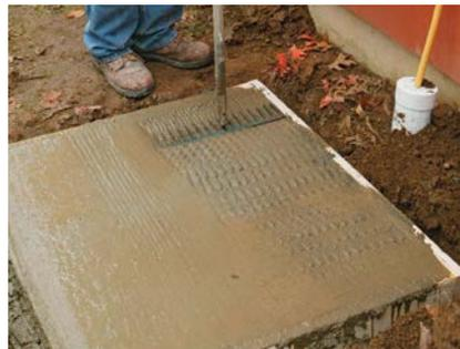
**8 TAMP THE SURFACE WITH A RAKE.** Gently tamp the entire surface of the slab. The rake pushes down the gravel that's part of the concrete mix, and brings up a mixture of cement and sand that's easier to smooth.
