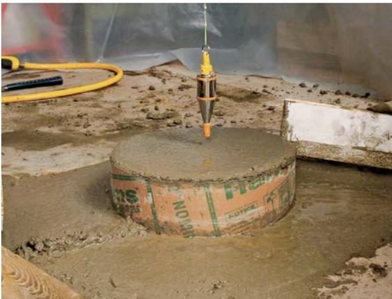
**FILL IT UP, AND SCREED IT AWAY.** Pour concrete in and around the builder's tube until the concrete is slightly proud of the slab and the lip of the builder's tube. Push two 16-in.-long pieces of rebar into the pier—so that their top end is 2 in. to 3 in. below the finished concrete—before screeding off the excess concrete and feathering the surrounding concrete into the slab. During the pour, make sure you're maintaining center by checking the pier location with a plumb bob.
