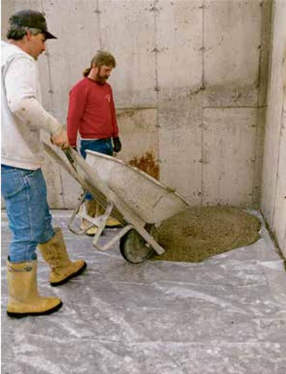
**FIRST MUD.** With the vapor barrier in place and the chalklines snapped, the first load of concrete is dumped in the far corner of the foundation. The mason dumps the concrete away from the wall so that he won't cover the chalkline.
