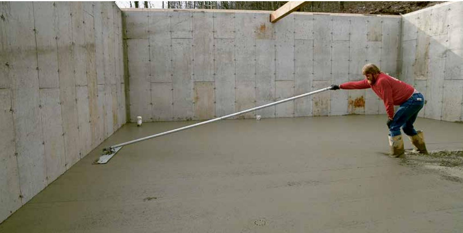
**OPERATING A BULL FLOAT.** After the concrete is screeded, a bull float pushes stones down and brings up the fines—sand and cement—that make a smooth, finished surface. To use a bull float, lower its handle as you push it away, and lift the handle as you pull it back.
