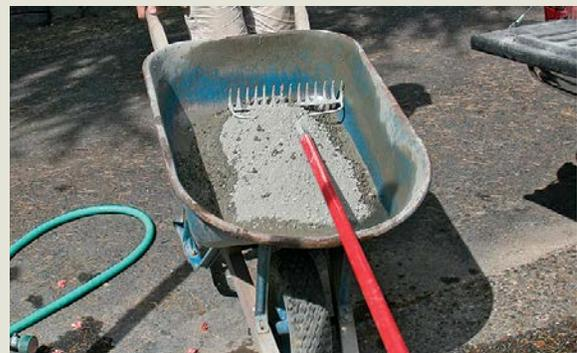
**3 MOVE THE MIX TO WHERE IT'S NEEDED.** To maneuver through tight areas without hanging up the rake, put the working end of the rake in the wheelbarrow with the handle pointing ahead.
