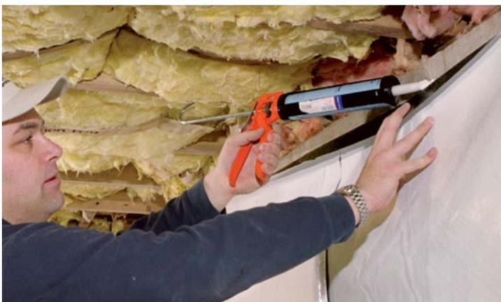
**SEAL THE LINER** to the foundation with polyurethane caulk.
