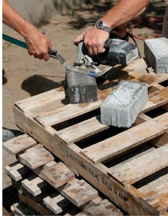
**A CIRCULAR SAW WITH A DIAMOND BLADE CUTS PAVERS EASILY.** A light water mist cools the blade, extending its life and preventing it from warping due to heat, and it keeps the silica-laden dust down. Make sure to be plugged into a GFCI-protected outlet.
