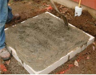
**5 SETTLE THE CONCRETE.** After dumping the mixed concrete in the form, jab into it all along the edges with a shovel. This helps ensure the mix fills the form without leaving voids.
