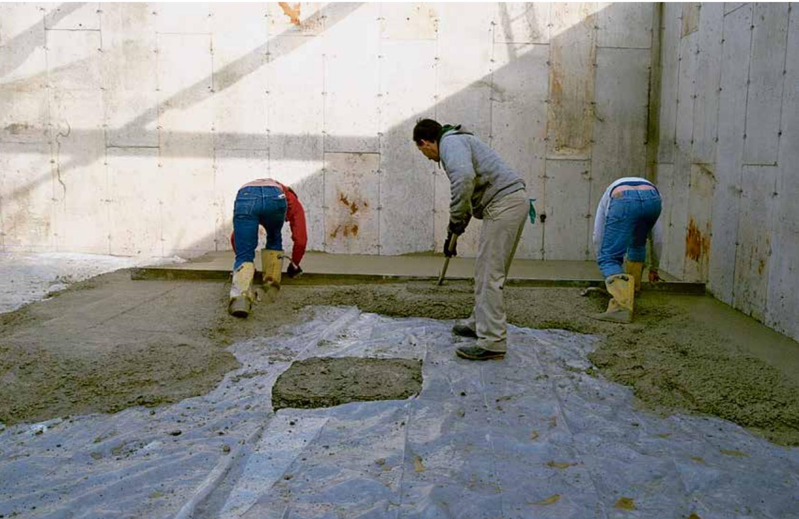
**RAKER'S ROLE.** As the screed rail levels concrete between the perimeter screed (right) and the center screed (left), the raker pulls away excess concrete or fills low spots. A rebar spike set at finish-floor height and subsequently driven below the concrete's surface establishes the center screed's level.
