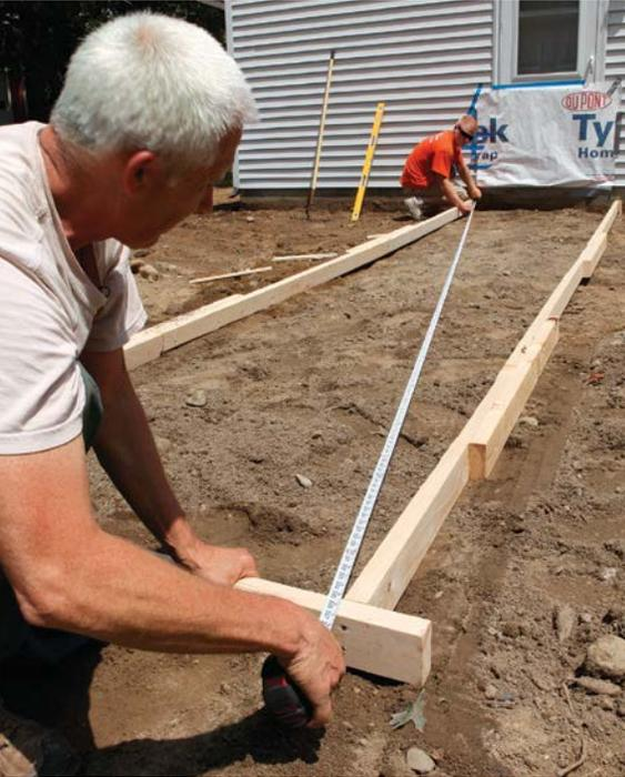
**1 SQUARE THE FORMS.** With a formboard on the end of the side forms (opposite the house) establishing the width of the walk, shift the formwork left or right until measurements from opposite corners are equal, which means the forms are square. Drive in stakes on both sides to keep the forms from shifting, but don't attach the screws just yet.
