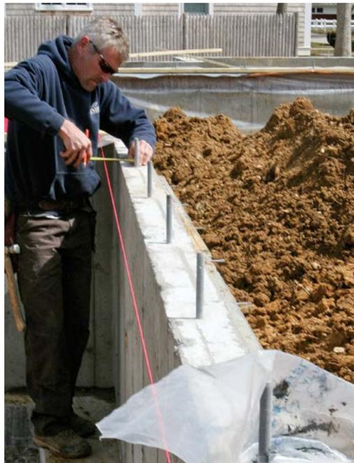
**NARROW WALLS REQUIRE OFFSET STRINGS.** The tops of these stemwalls are only wide enough to carry the 2x6 walls, so the carpenters attach 2x spacer blocks to the stemwalls, and then they fasten an offset stringline to the blocks to use as a reference for measuring.
