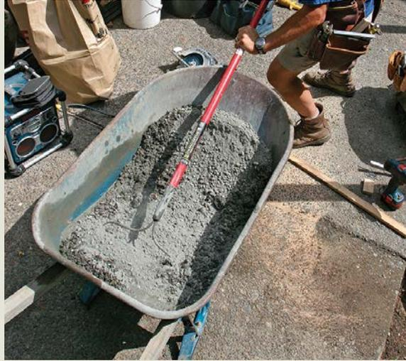
**4 STAND IN FRONT TO MIX.** Pull the concrete to the front, and water will flow in behind it. Because I'm standing at the front of the wheelbarrow, I now can work the concrete without having the wheelbarrow move as I push back and forth. Let the water flow in after each push-and-pull stroke. Keep mixing until most of the water is absorbed.
