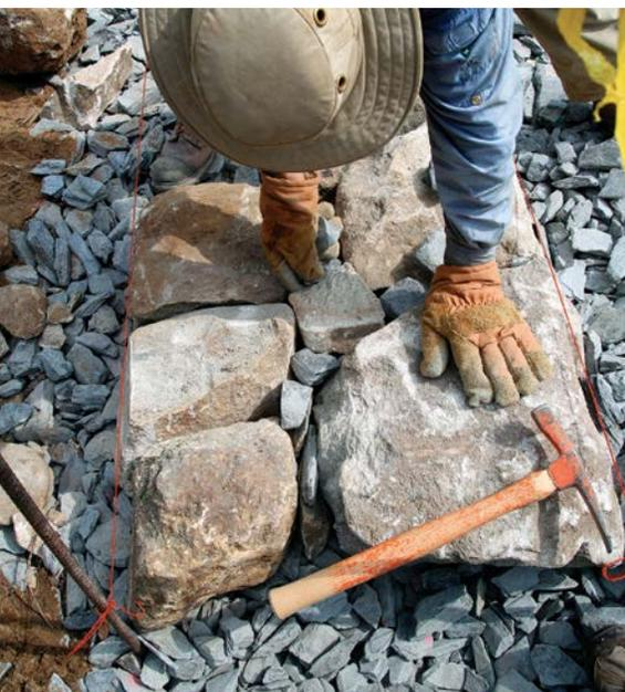
**LEFT: THERE WILL BE VOIDS.** Face stones don't have to meet tightly inside the wall. Just pack the spaces full of hearing stones.
