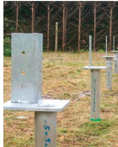
**HOLD THE HOUSE DOWN.** Steel plates are lined up and welded to the piles. The vertical legs provide attachment for perimeter beams.
