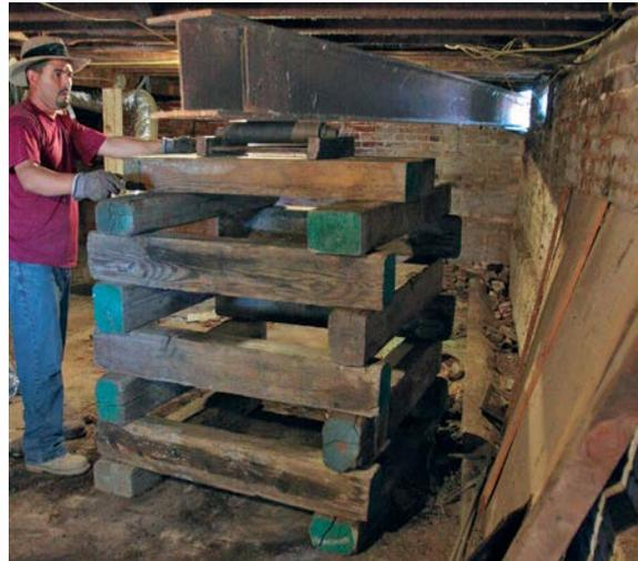
**THE BEAMS ROLLED UNDER THIS HOUSE** were lifted with individual 30-ton jacks. Some outfits use a unified hydraulic-jack system that raises and lowers the house evenly in one shot. Those systems require less labor, but the individual jacks that were used on this job work well, too.
