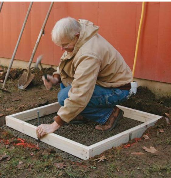
**3 MAKE AND SET THE FORM.** Most 4-in. slabs are actually the  $3\frac{1}{2}$ -in. depth of standard 2x4s. Nail the corners together, and place the form on the graded gravel, making sure it doesn't rock. Drive 12-in. lengths of rebar to just below the top of the form to keep it from moving.
