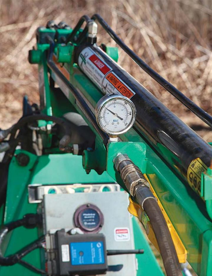
**LEFT: VERIFYING A PILE'S BEARING CAPACITY.** There are two ways to verify bearing: a high-tech approach based on hydraulic pressure and a low-tech approach that involves whacking the pile with a sledgehammer. Hydraulic pressure equates to torque and bearing capacity. The more torque needed to drive a pile, the greater its bearing capacity. Think of a wood screw. The harder it is to spin the screw into the wood, the harder it will be to pry the screw out or to hammer it farther in.
