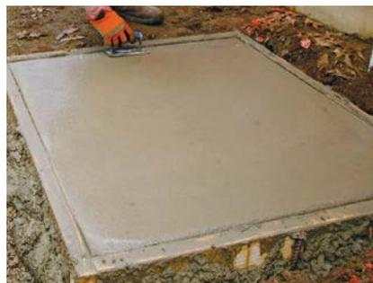
**10 ROUND THE CORNERS.** This leaves smooth, friendly edges that are less likely to chip. Use an edger once after each mag floating; on interior slabs with exposed edges, use it after the steel float. After the slab hardens for a day or more, pry the joints apart and remove the form.
