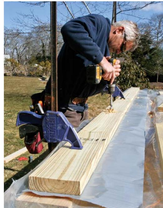
**DRILL THE LAYERS AS A SANDWICH.** Although they started out marking and boring through each layer separately, the carpenters quickly learned that it's faster to stack up the poly, termite shield, and 2x6 mudsill; clamp them together; and drill through everything at once.
