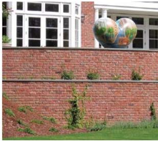
**CONCRETE WALLS TAKE ON THE LOOK** of the surface treatment: here, stucco (left) and brick (right).
