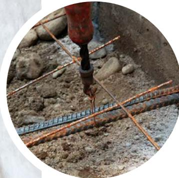
**3 ADD STEEL FOR STRENGTH.** Three rows of  $\frac{3}{8}$ -in. rebar and a grid of 4-in. reinforcing mesh add strength and help to control shrinkage. Rebar dowels inserted into the foundation prevent the walk from sinking near the house. Make the holes with a rotary hammer.
