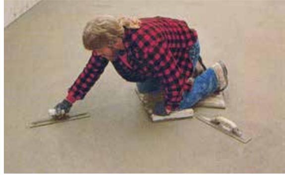
**START WITH A MAG; FINISH WITH STEEL.** After bull floating, use a magnesium float (left) to smooth out bumps and fill in low spots. The resulting finish will be coarse. Later, use a steel trowel (right) to get a smooth, dense finish that won't crumble when it's swept.
