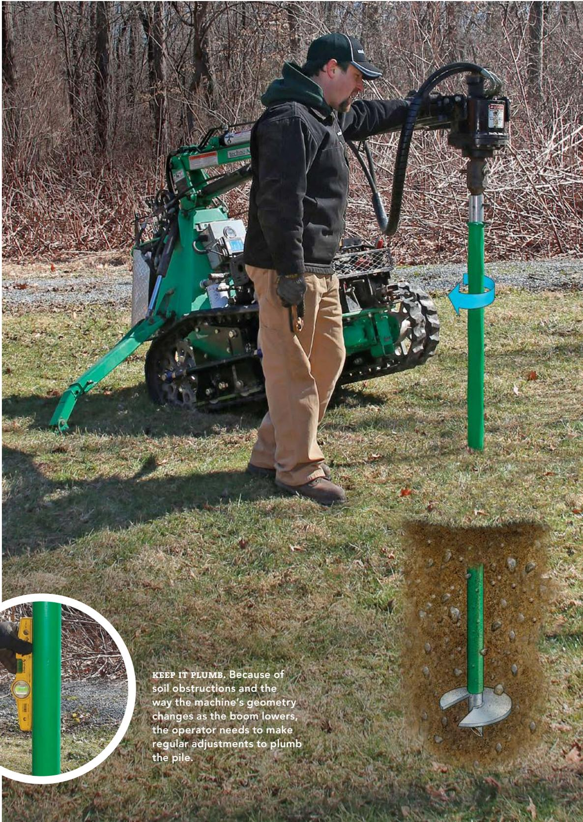
**KEEP IT PLUMB.** Because of soil obstructions and the way the machine's geometry changes as the boom lowers, the operator needs to make regular adjustments to plumb the pile.
