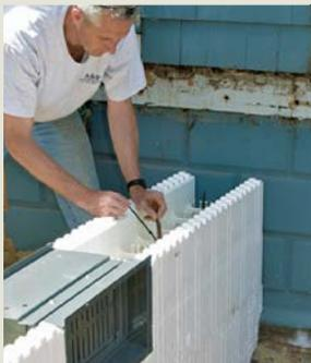
**WHEN THE AUTHOR DROPS IN ANOTHER LENGTH OF VERTICAL REBAR** from above, it is carefully threaded into the looped zip tie, which then is pulled tight with a pair of pliers to tie the rebar together.
