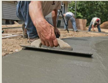
**BRING UP THE CREAM.** A smaller float made of magnesium, aluminum, or wood brings cement particles and fine aggregate to the surface. The resulting cream fills small voids and smooths the surface.
