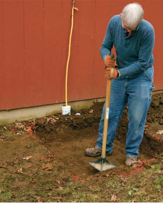
**1 PREPARE THE SUBGRADE.** Dig 6 in. beyond where you want the slab edges and 8 in. deeper than where you want the top of the slab. Make sure the subgrade pitches away from the building, and tamp down loose soil.
