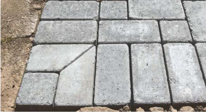
**START IN A SQUARE CORNER.** This helps create two straight edges to work from, easing the balance of the installation. The mitered corner blocks are a simple custom touch.
