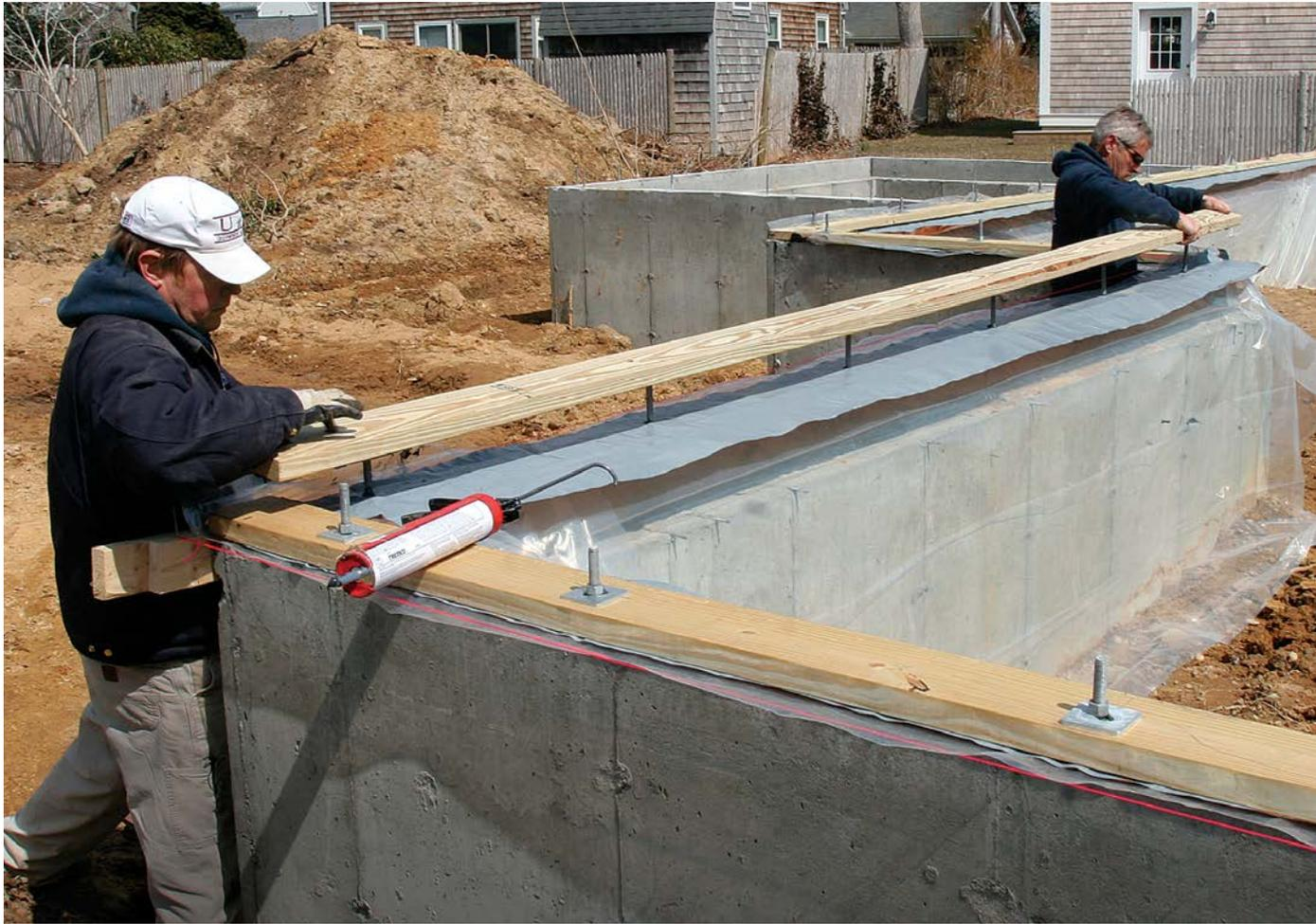
**BUTTER THE BUTT JOINTS.** Before placing the next 2×6 sill, a thick bead of sealant is applied to the edge of any adjoining sill. This is a commonly overlooked weak spot in an air-sealed assembly.
