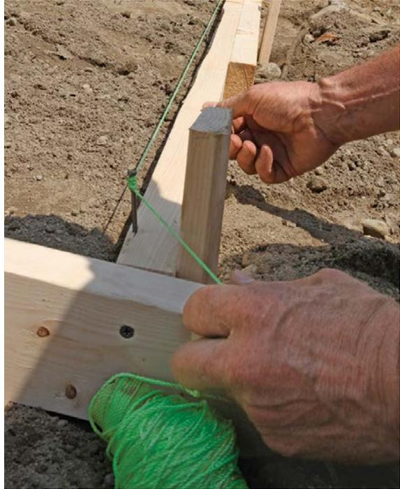
**2 STRAIGHTEN THE SIDES.** Use a taut string to straighten the sides of the formwork. Drive in stakes every 2 ft., and screw through them into the sides of the form. Backfill against the forms with soil or gravel to prevent bulging.
