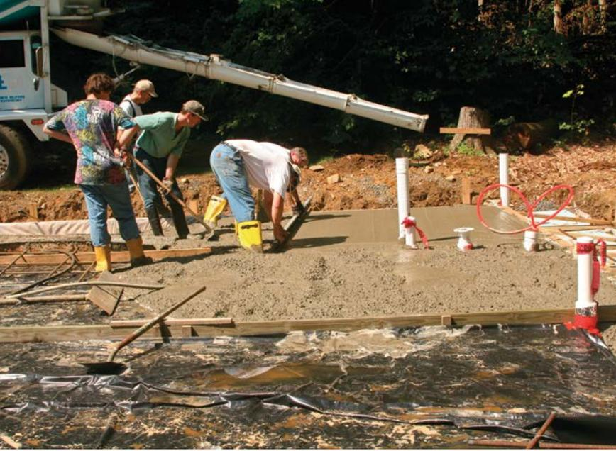
**CONCRETE DAY.** Screed guides made from 2×s run the length of the foundation, breaking the 28-ft.-wide slab into narrower sections that can be screeded easily. The guides are pulled out as the pour progresses, and their trenches are shoveled full of concrete.
