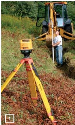
**USE A LEVEL TO MAKE SURE THE TRENCH ISN'T.** The trench should slope away from the center point to prevent puddling. Don't overdig because backfilling with uncompacted soil causes settling and low spots.
