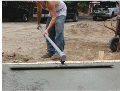
**5 BREAK OUT THE BULL FLOAT.** Level the surface, and force the aggregate into the mix with a bull float. Keep the leading edge raised as you push or pull to avoid digging into the surface. Two or three passes is enough.
