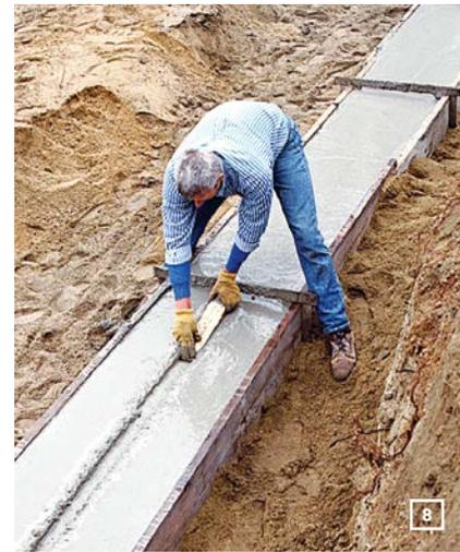
**7 THE TOP IS TROWELED SMOOTH,** and **8 a keyway is formed by dragging a 2x4 down the center of the footing.**
