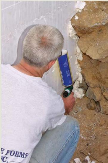
**FOAM FILLS THE GAPS.** Expanding foam can be used to seal seams, plug holes, and tighten rough scribe work.
