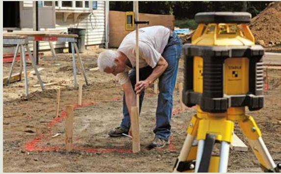
**DRIVE THE STAKES.** Space the stakes every 1 ft. in the curved sections and every 2 ft. in straight sections. Then, using a rotary laser equipped with a receiver (a water or spirit level works, too), mark the stakes no less than 4 in. above finished grade. Once they're marked, cut them off with a circular or reciprocating saw so that the screed board can pass easily.
