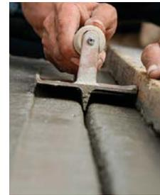
**6 MAKE CREAM WITH A MAG FLOAT.** After the bleed water has evaporated, use a magnesium float to bring up the layer of water and cement particles called cream. Then round the corners with the edging tool, and make control joints every 5 ft. with a 2×4 and a groover.
