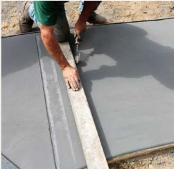
**TRANSITION AT CURVES.** A stripe with a simple contrasting pattern provides a convenient place to hide control joints and to eliminate odd transitions where the walk changes direction.
