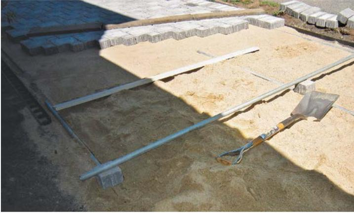
**MAKE A FLAT SAND BED.** First, determine the elevation. A piece of conduit resting atop a few pavers determines the height of the sand bed. The partially buried pieces of conduit are used as screed guides. Set them  $\frac{1}{2}$  in. high to allow for compaction.
