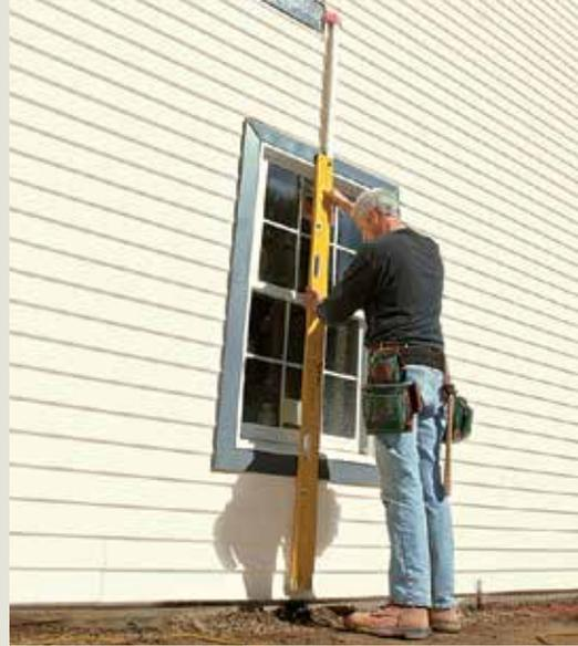
**1 PLUMB DOWN FROM A HIGH LEDGER.** With a Stabila plate level ([www.stabila.com](http://www.stabila.com)), I carry one end of the ledger down to the grade. I drive a stake into the ground here to anchor a line that will run perpendicular to the house.
