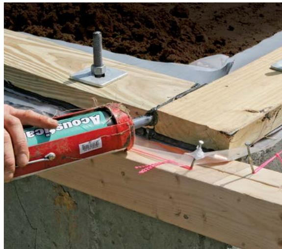
**BELT AND SUSPENDERS.** After all of the layers are in place and the foundation bolts have been fully tightened, another bead of sealant is applied to the exterior joint between mudsill and stemwall and at all butt joints.
