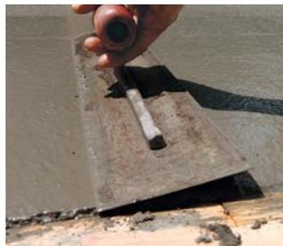
**7 USE A STEEL TROWEL FOR A SMOOTH FINISH.** With the grooves cut and the corners rounded, use overlapping arcs with a steel finish trowel to tighten up the surface before brooming.
