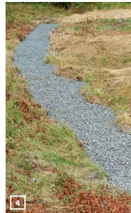
**TOP THE TRENCH WITH GRAVEL.** For a better look, you can buy decorative gravel that matches the landscape for the top layer. Where the underlying pipe is nonperforated (beyond the curtain drain and into the bulk-water removal), you can skip the top layer of gravel and plant grass.
