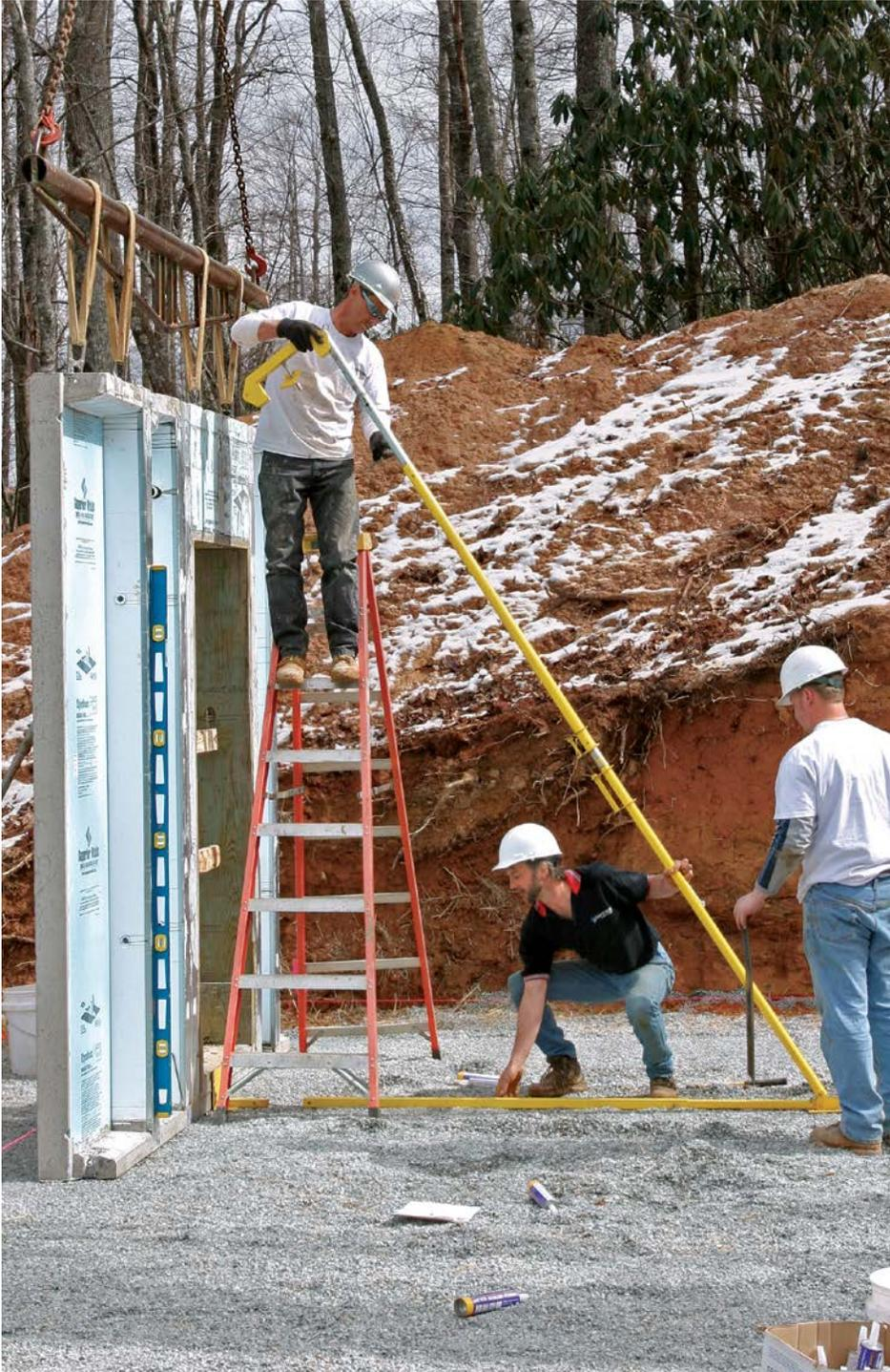
**STARTING IN A CORNER**, the crew aligns the first panel with a string line and then braces it plumb. No additional braces are needed because the corners stabilize the walls. Additional panels are set to the string and bolted together top and bottom.
