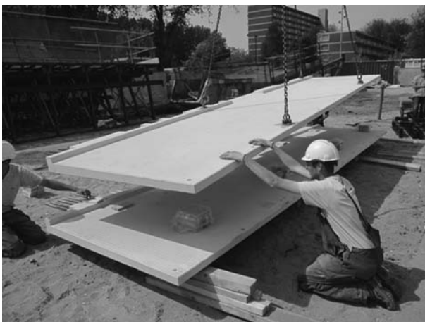
Fig. 7.54 Balcony slab for a high-rise building project, Poptahof, Delft, The Netherlands [165]
