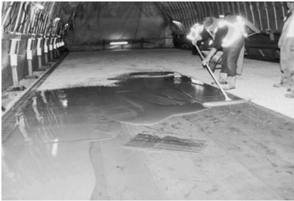
Fig. 6.11 Applying the layer of epoxy resin to the steel plate
