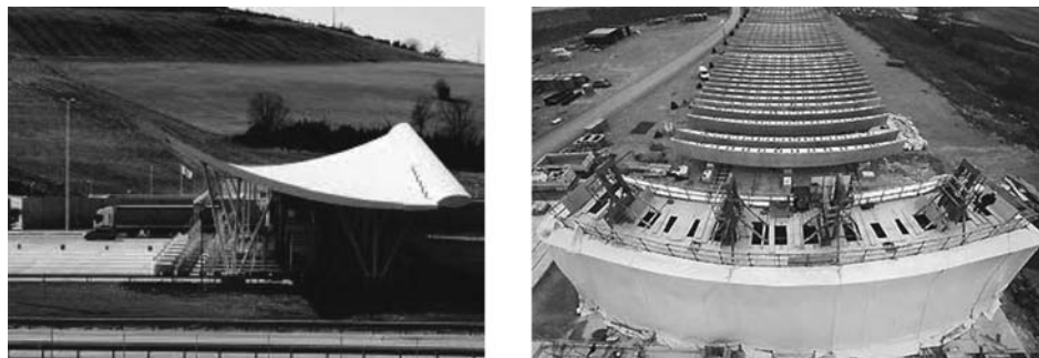
Fig. 7.58 UHPC roof shell at Millau viaduct, France [168]
