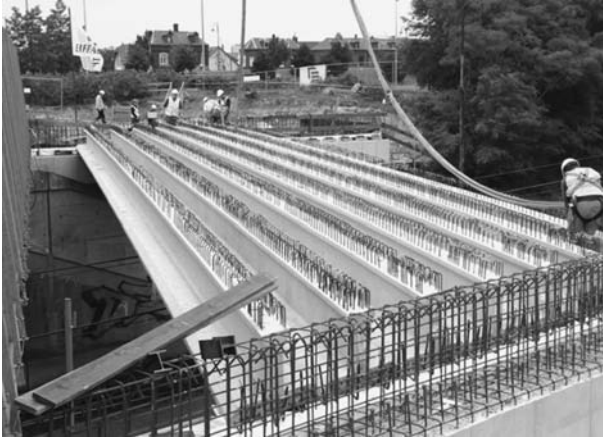
Fig. 7.6 Pont Pinel under construction
