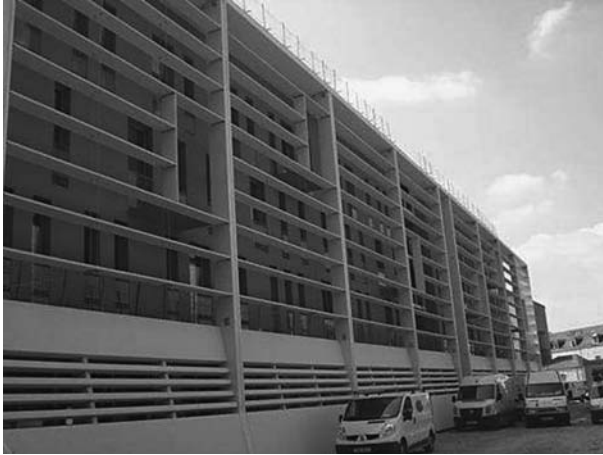
Fig. 7.51 Police headquarters in Nantes: sunshades after erection [163]
