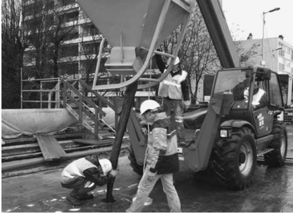
Fig. 7.9 Placing the UHPC through an opening in the road deck
