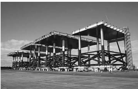
Fig. 7.61 Steel substructure with stainless steel jackets [Nippon Steel Corp.]
