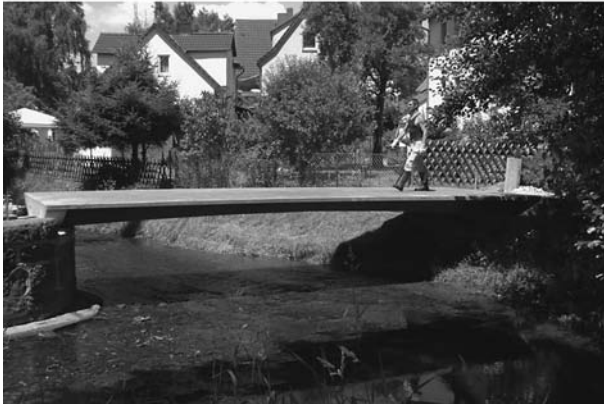
Fig. 7.26 Two further UHPC precast bridges over the River Nieste: a) section, b) view of one of the bridges
