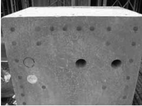
Fig. 7.47 Sawcut through UHPC test column for Park City Musashi-Kosugi high-rise building, Tokyo [161]
