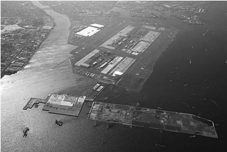
Fig. 7.60 New runway, Haneda Airport: a) computer image of design [170] for runway D, b) runway during construction. (Ductal®)
