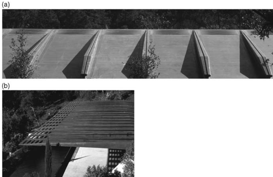
Fig. 7.59 Roof of precast UHPC segments at Villa Navarra, Le Muy, France [169]. a) several of the 17 identical, ribbed elements; b) cantilevering part
