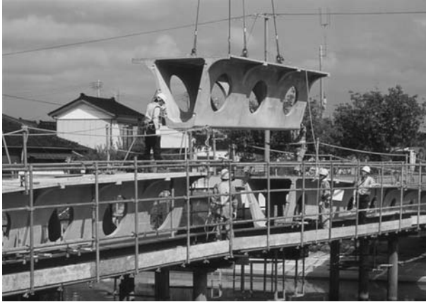
Fig. 7.11 The segments being erected on temporary supports [Ductal®]
