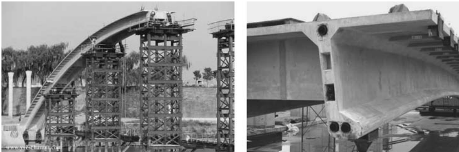
Fig. 7.19 Erecting the arch and view of segment [150]
