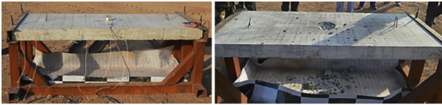
Slab after test
