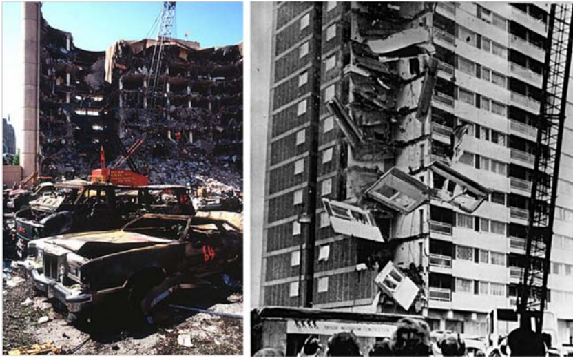
Figure 1.5 Structural progressive collapse induced by blast loads. Left: 1995 Alfred P. Murrah Federal Building ( http://en.wikipedia.org/wiki/Alfred_P._Murrah_Federal_Building ); Right: 1968 Ronan Point Building ( http://en.wikipedia.org/wiki/Ronan_Point ).
