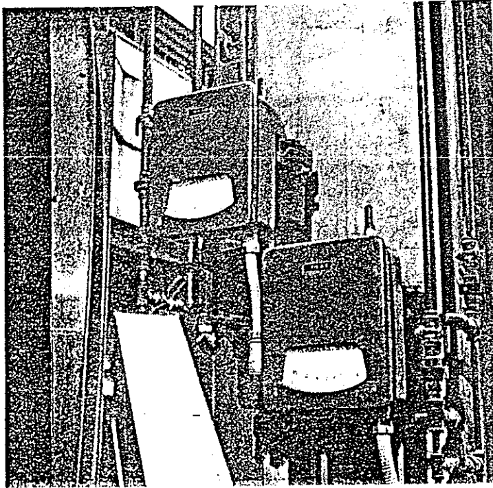
Fig. 15.5 Each of these flow transmitters sends measurement signals to a recorder or controller. ( The Foxboro Co. )
