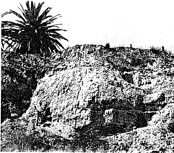
Fig. 1.1 Remains of underground furnaces that were used by early California Settlers for burning limestone to make lime. ( Riverside Division, American Cement Corp. )
