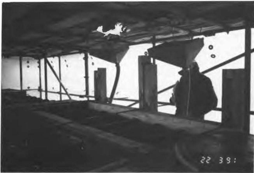
Fig. 5 Placement by funnel and tube
