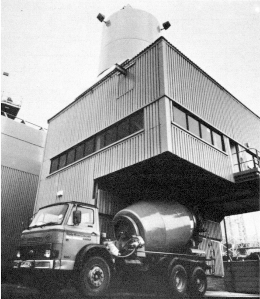
Figure 8.2 Urban plant with central mixer. Courtesy RMC (UK) Ltd
