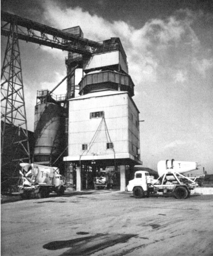
Figure I.1 Early towerplant with truckmixers and agitator. Courtesy of Tilcon Ltd
