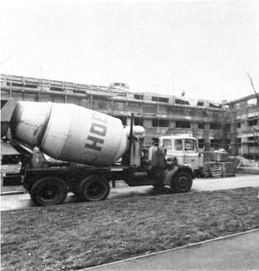
Figure 10.2 Truckmixer on site. Courtesy Wimpey Hobbs Ltd
