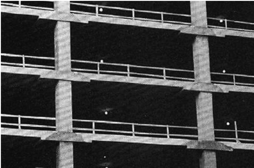
Figure 10.11 Color contrast of darker column concrete (containing silica fume), with slab concrete. Courtesy of American Concrete Institute.
