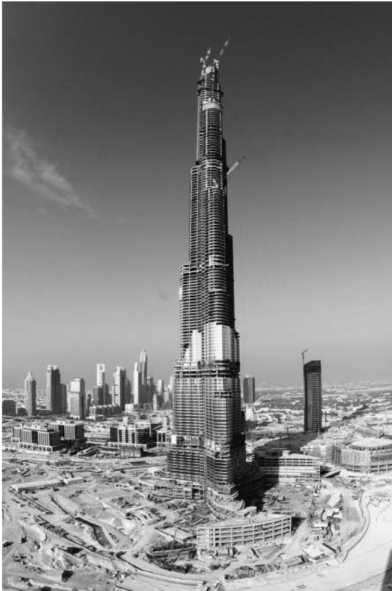
Figure 1.5 At this point in its construction, the super skyscraper Burj Dubai had already attained the title “world’s tallest building.” Courtesy of Samsung Engineering and Construction.
