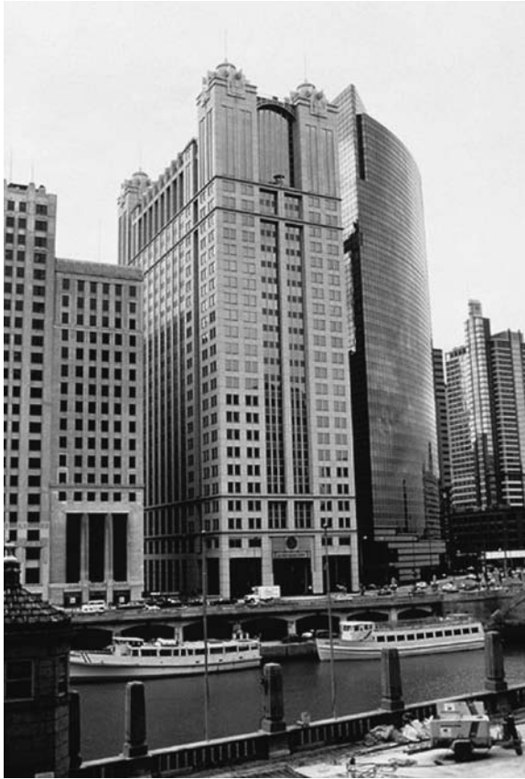
Figure 1.1 Office building at 225 West Wacker Drive, Chicago: constructed with 96 and 117 MPa (14,000 and 17,000 psi) concrete. Courtesy of Portland Cement Association.
