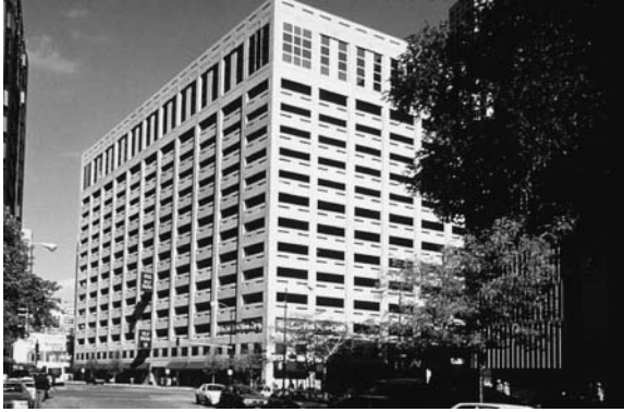
Figure 1.4 Parking structure at 900 N. Michigan Ave, Chicago. High-strength concrete helped to reduce column sizes in this 15-story structure. Courtesy of Portland Cement Association.
