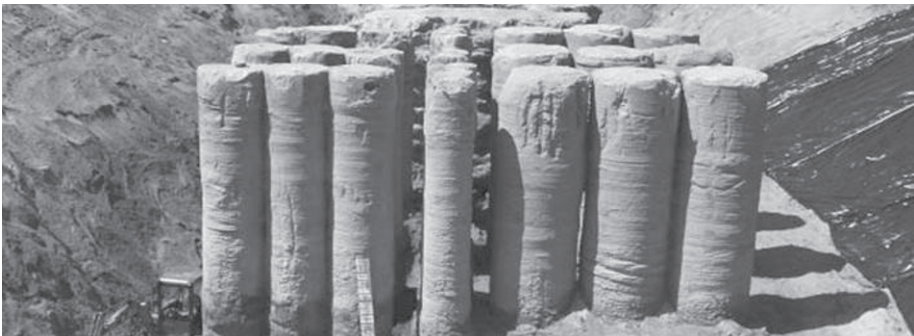
Figure 21.8 Dense network of solidified DSM columns (courtesy of Treviicos, 2013).
