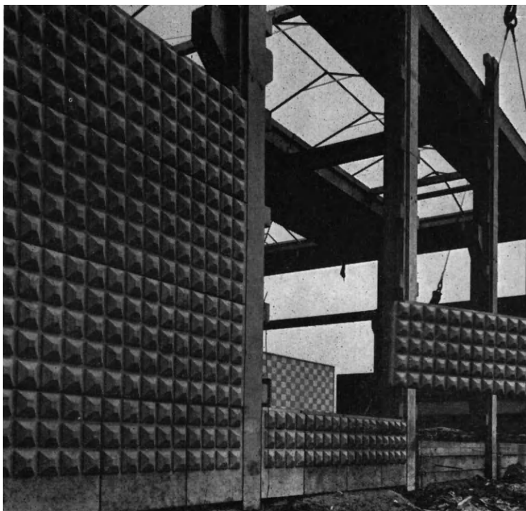
Plate 18. Profiled precast facing slabs.
