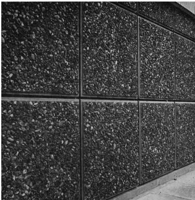
Plate 17. Exposed aggregate facing slabs.
