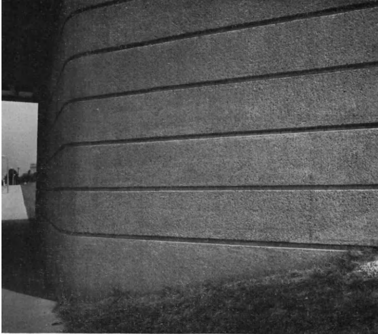
Plate 12. Surface texture produced by light tooling.
