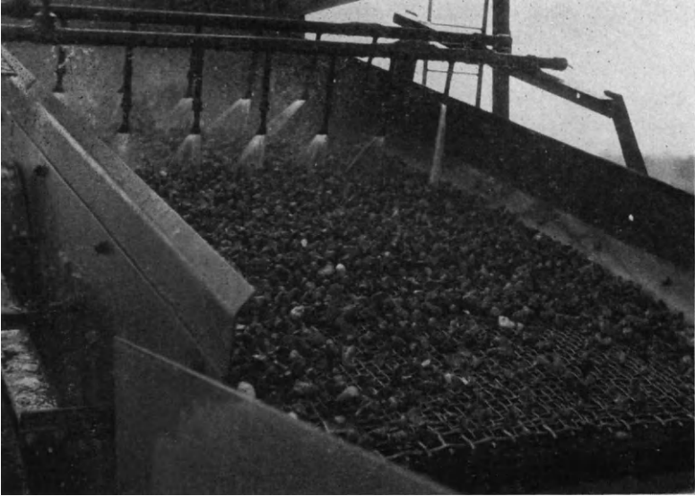
Plate 3. Washing aggregate on vibrating screen.
