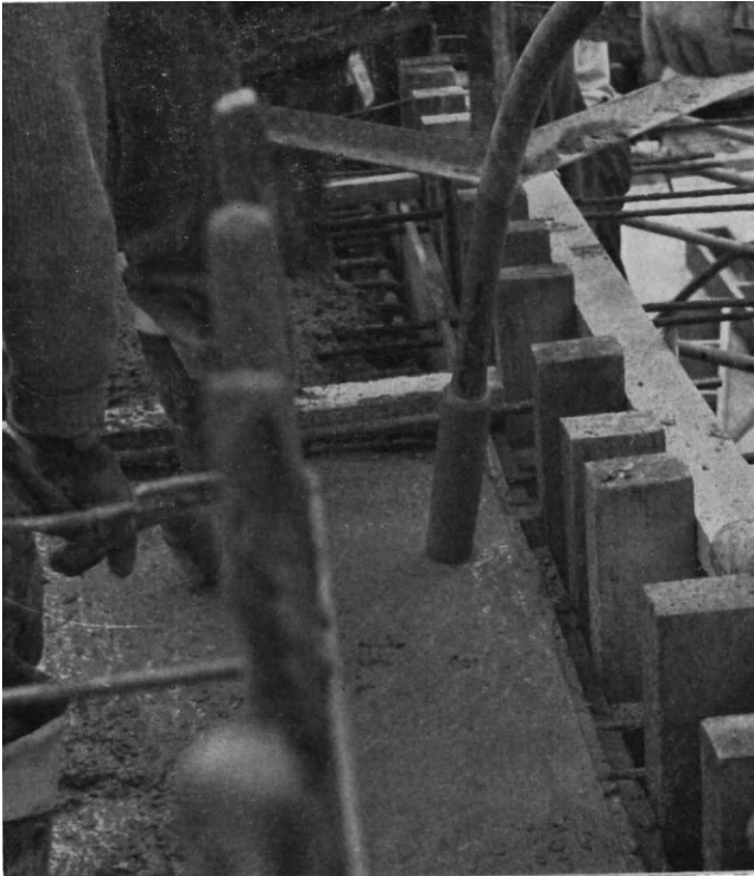
Plate 6. Compacting concrete around congested reinforcement by internal vibrators.
