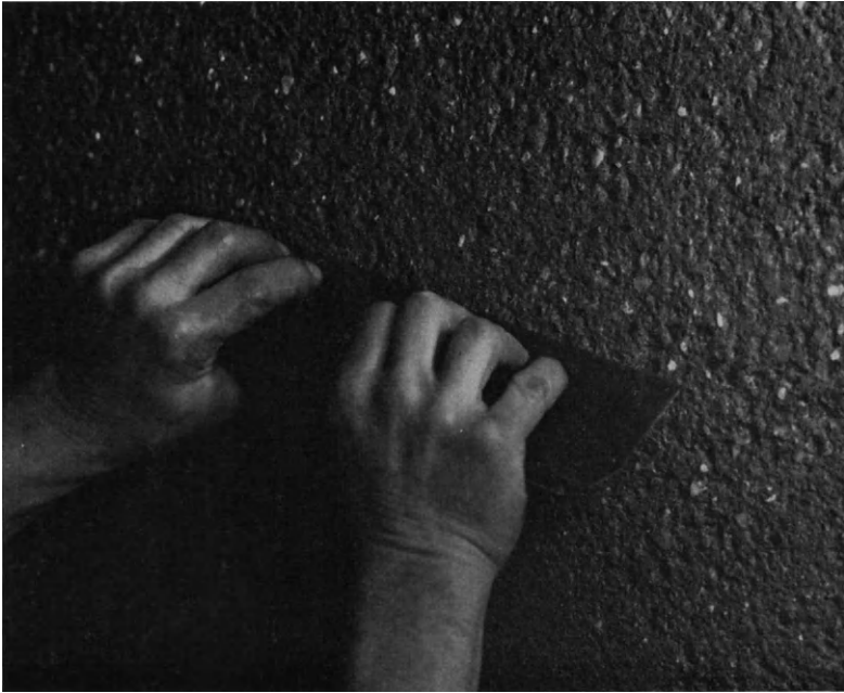
Plate 14. Texture produced by scraping with saw blade.
