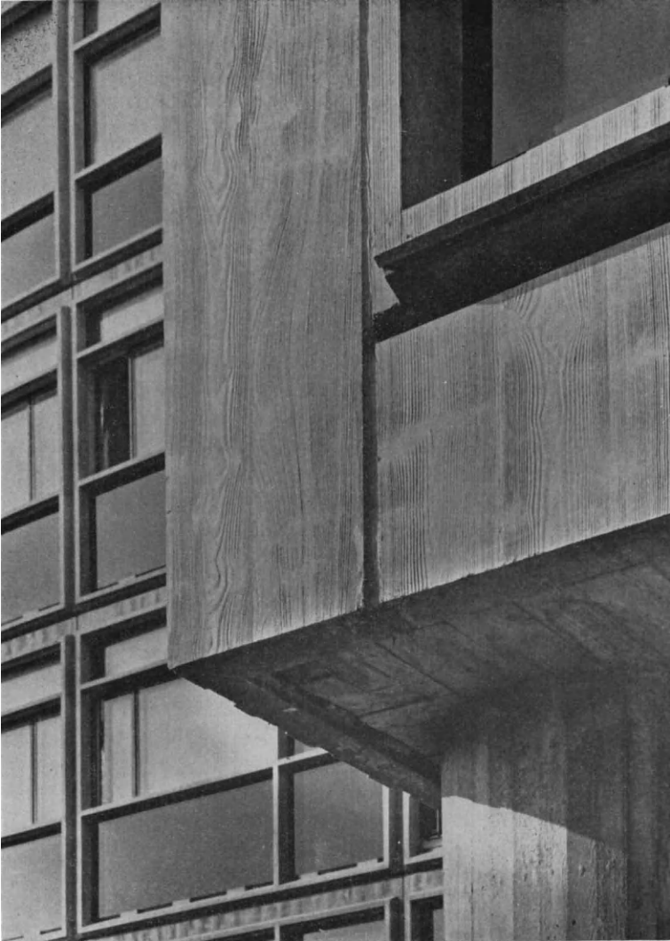
Plate 9. Texture achieved by casting against sand-blasted pine.
