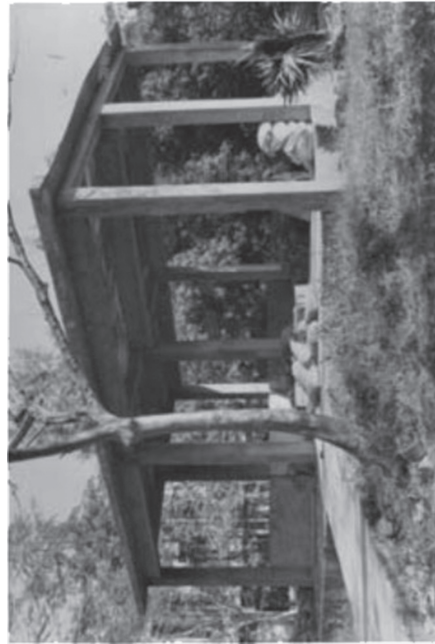
FIGURE 10.9 An experimental structure built with calcium sulfoaluminate–belite cement and its long-term exposure. (From A. K. Chatterjee, Indian Concrete Journal , Vol. 84, No. 11, 2010, pp. 7–19.)
