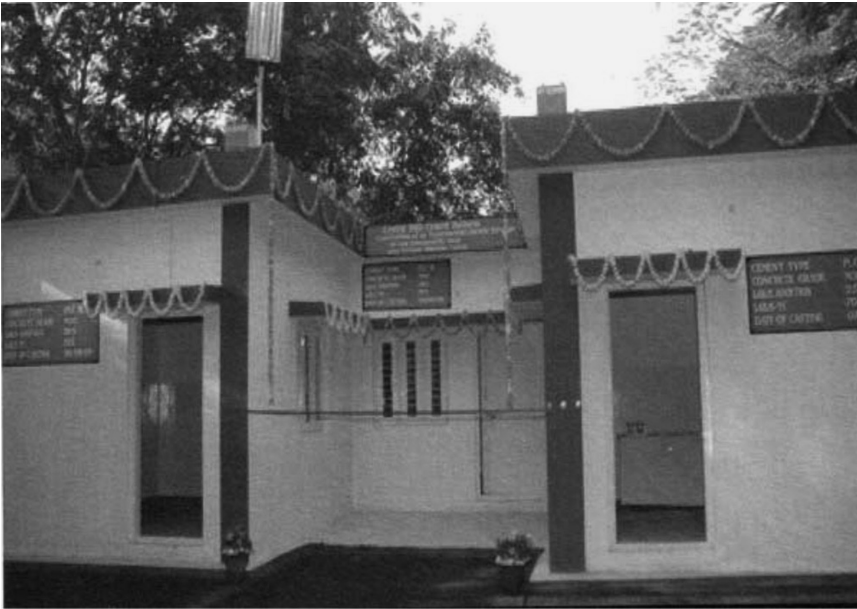
FIGURE 10.11 An experimental structure built entirely with Portland limestone cement.
