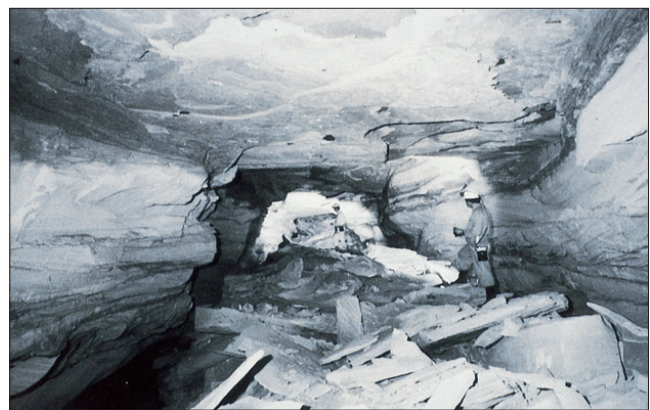
Figure 4. Example of a failed parting
