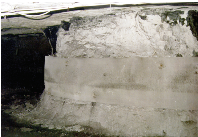
Figure 15. Conveyor belt wrapping around a pillar
