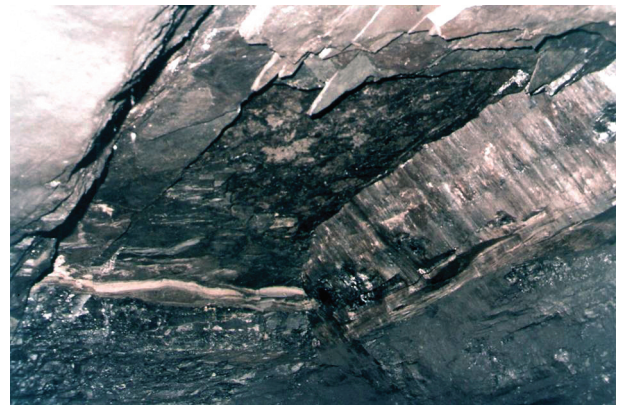
Figure 21. Example of a wedge formed by joints
