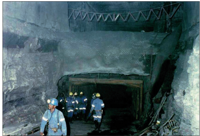
Figure 3. Example of a stable 2 m thick parting in sandstone
