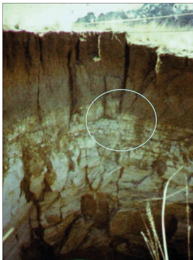
Figure 2. Photograph taken of the sidewall of a sinkhole that occurred at the face end of a subsidence trough. The sinkhole was caused by a face break underground that required loading out a substantial amount of rock. Inside the circled area it can clearly be seen that discrete blocks of rock are displaced relative to one another and that the blocks undergo tilting relative to one another
