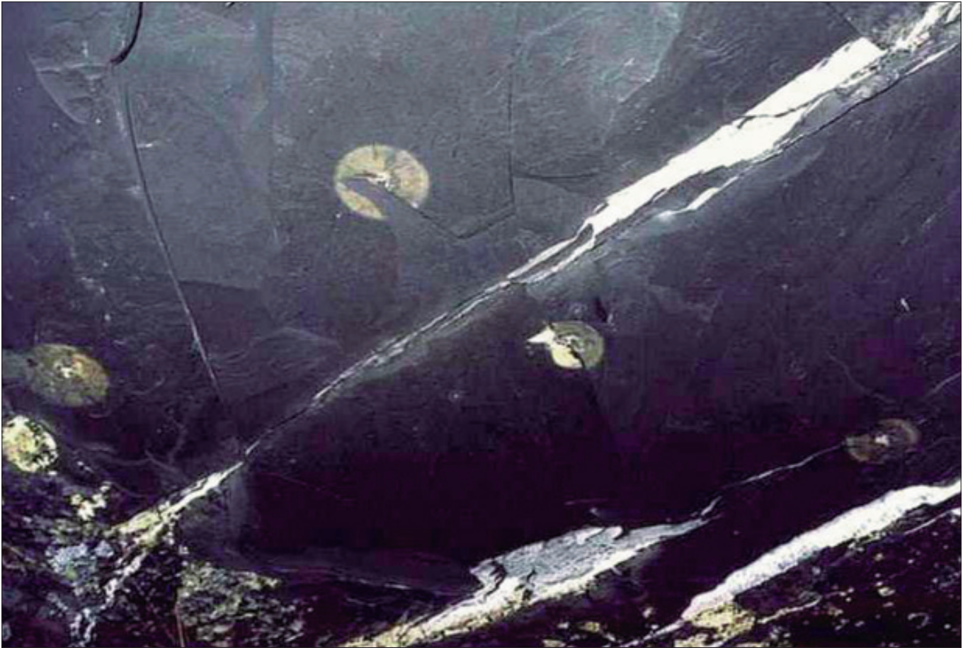
Figure 6. The rust rings are clearly visible at the anchor positions of the holes
