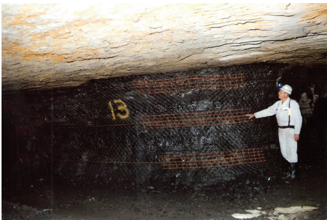
Figure 14. Wire mesh and oslo-straps installed
