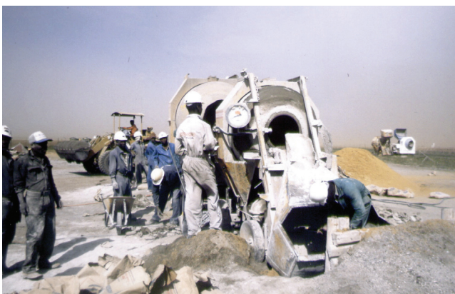
Figure 22. Direct filling from surface through boreholes into the excavated dyke
