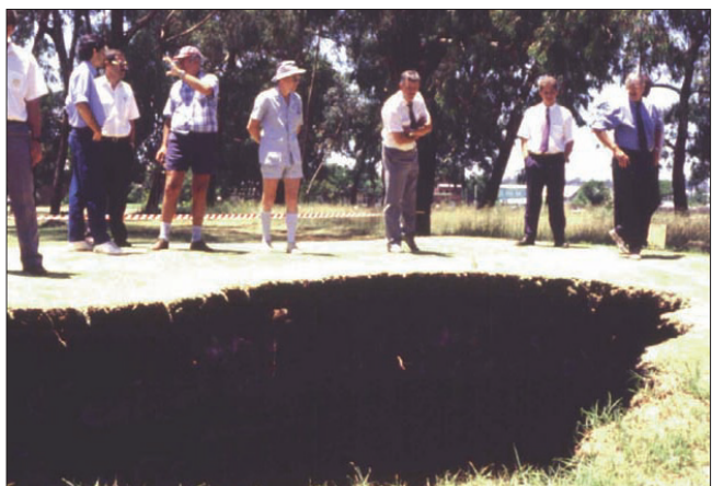
Figure 21. A recent sinkhole on a golf course. The hole was approximately 4 m deep
