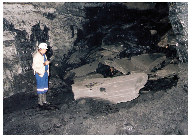
Figure 16. Shale layers sliding into heading, note timber ‘policeman’ knocked out
