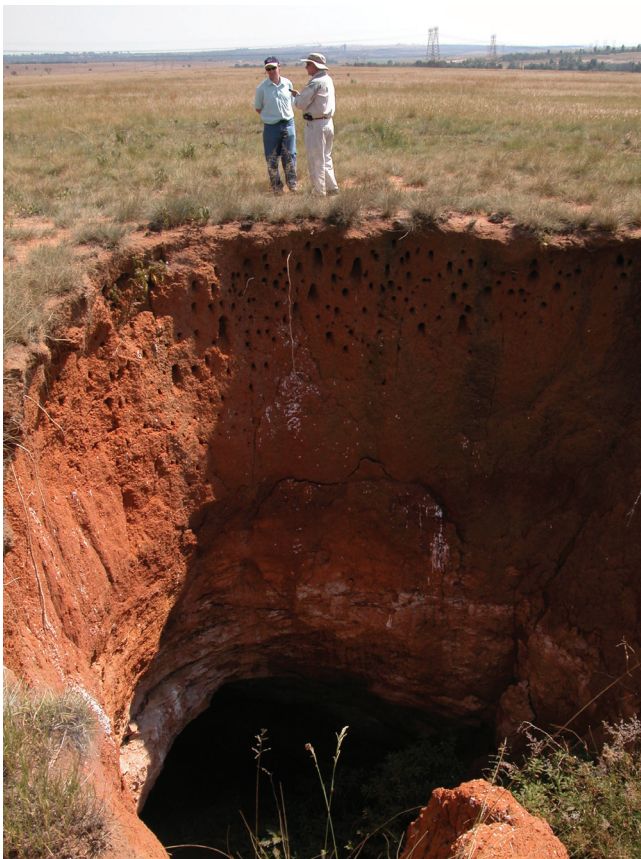
Figure 3. Example of a sinkhole
