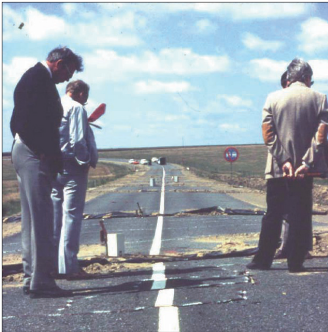
Figure 8. Examples of discontinuous (on the left) and continuous (on the right) horizontal displacement. The slightly curved centre line on the road in the right-hand photograph is the original centre line, which was repainted after the road had subsided
