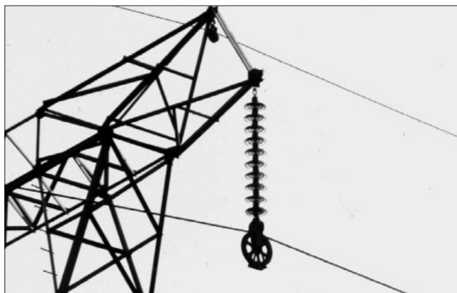
Figure 30. Temporarily suspending the conductors on rollers instead of the normal fixed fittings frees the pylon to move without damaging the structure
