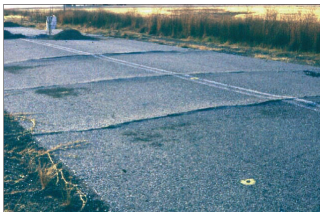
Figure 27. Example of smaller, dispersed compression ridges
