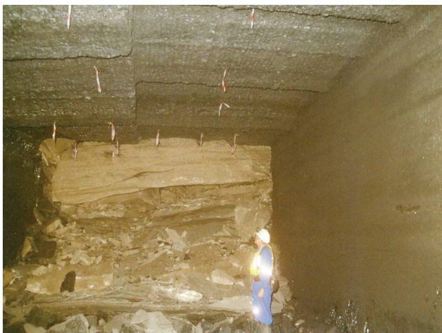
Figure 15. Competent sandstone layer goafing on pillar edge
