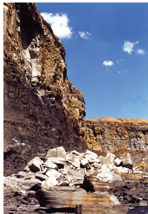
Figure 2. Joints oriented sub-parallel to the highwall face line, resulting in instability
