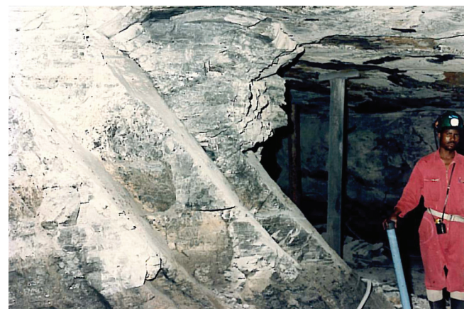
Figure 5. The effects of discontinuities on pillar stability
