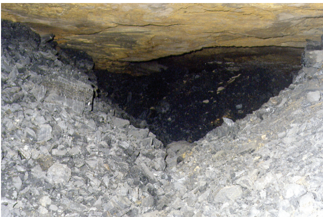
Figure 12. View inside a panel where the pillars had failed
