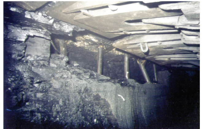
Figure 10. A view of the ash fill that was mined through by longwalling. The ash was placed to stabilize the inter panel pillars that were too small for mining without being reinforced
