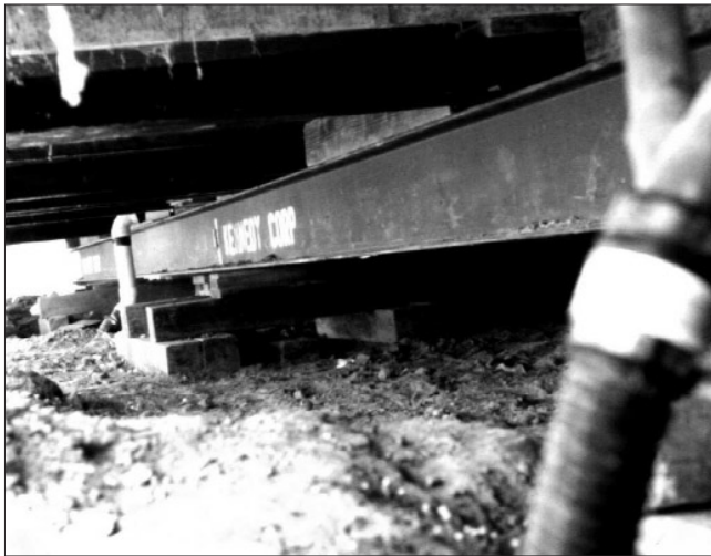
Figure 32. Steel beam underneath a timber house during undermining in the USA
