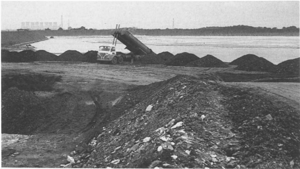
Plate 3. General View of Minestone Lagoon Embankments
