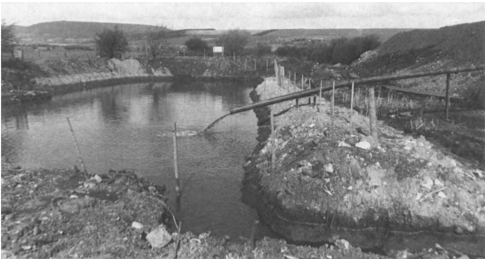
Figure 7 Lagoons like this may not always be feasible or permitted by the planning authority.
