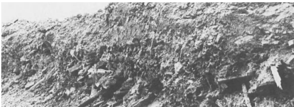
Plate 2. Loosely placed fill in a Spoil Heap.
