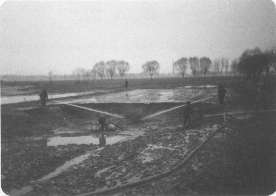
Fig. 12. Soil-overlay operation by means of hydraulic dredging unit.
