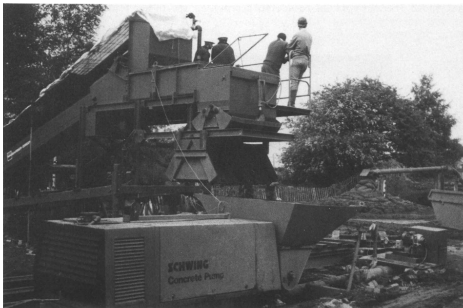
Fig. 5 - Rock paste plant for trial infilling during heap test pumping
