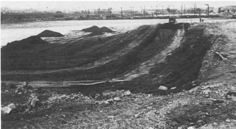
Plate 7. Minestone used to Reclaim Derelict Steelworks site for Retail Park, Rotherham.
