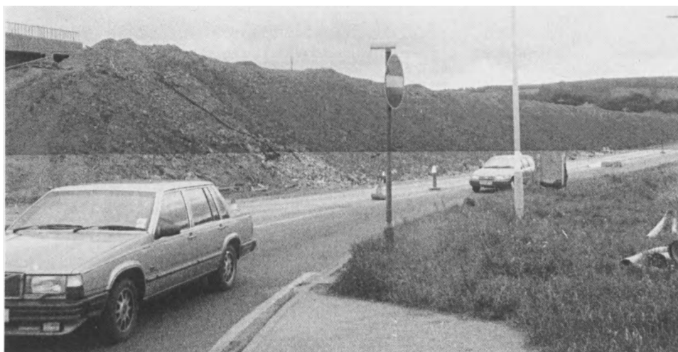
Plate 5. Burnt Minestone utilised as a 'free-draining' material in a Highway Embankment in Gateshead.
