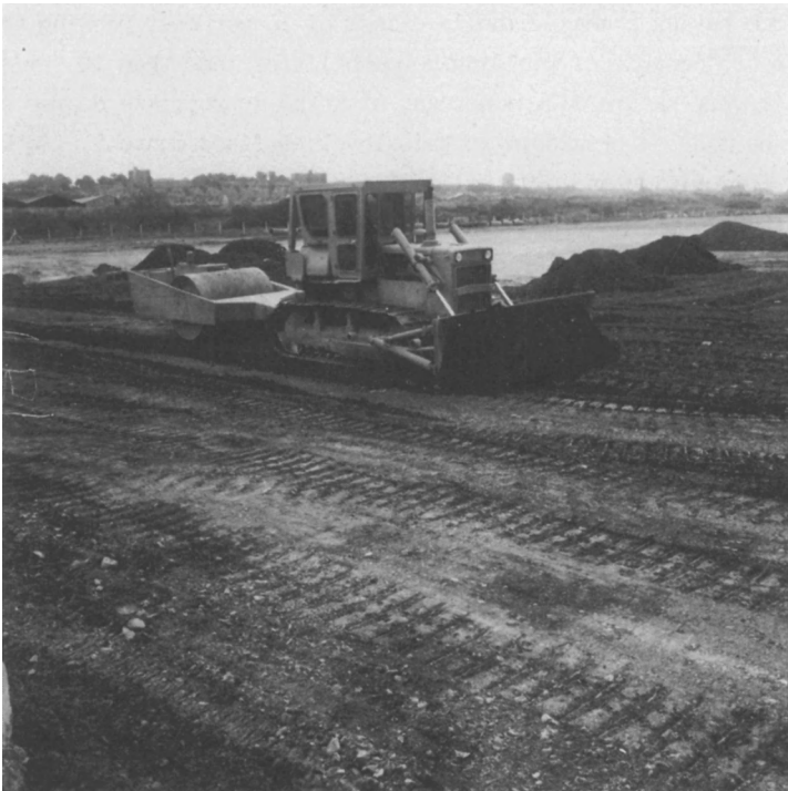
Plate 4. Typical Placement and Compaction of Minestone Layer
