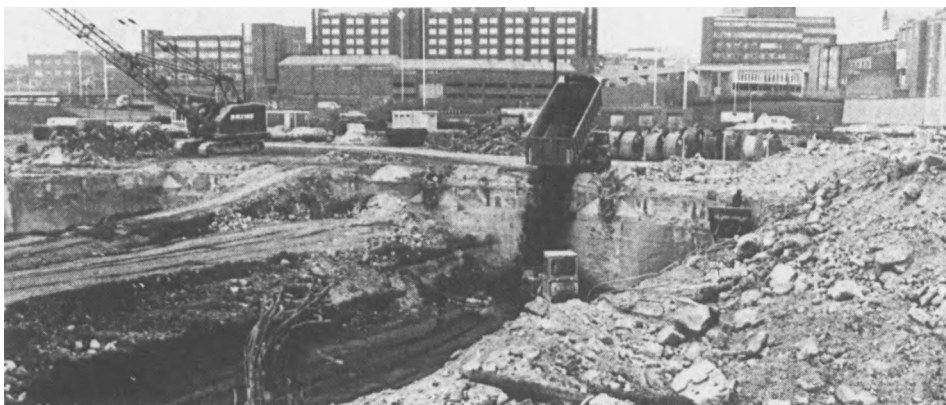
Plate 1. Reclamation of Derelict Site, Newcastle-upon-Tyne by infilling with Minestone.
