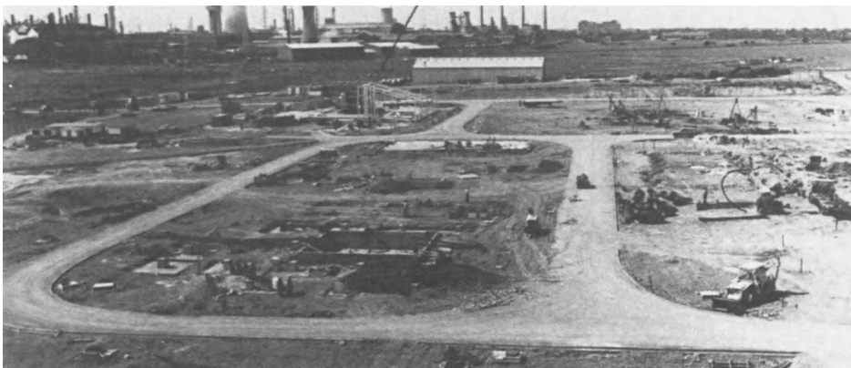
Plate 7. Burnt Minestone used as Road Sub-base within Chemical Works site, Teesside.
