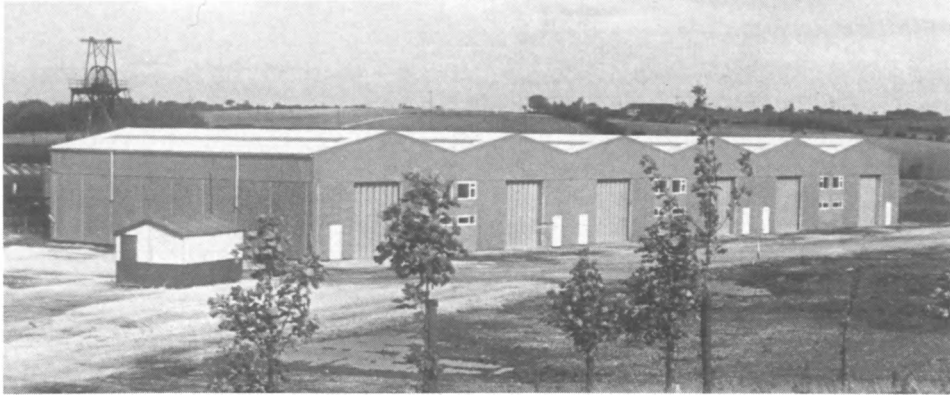
Plate 6. Industrial Development on reclaimed Colliery Spoil Heap in Sheffield.
