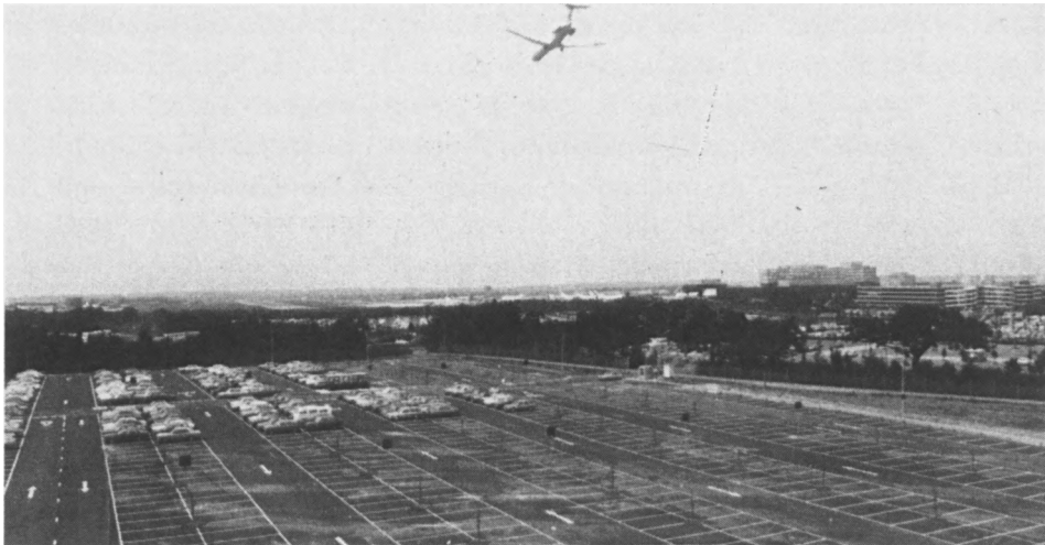
Plate 6. Cement Bound Minestone used as Car Park pavement material at Gatwick Airport.
