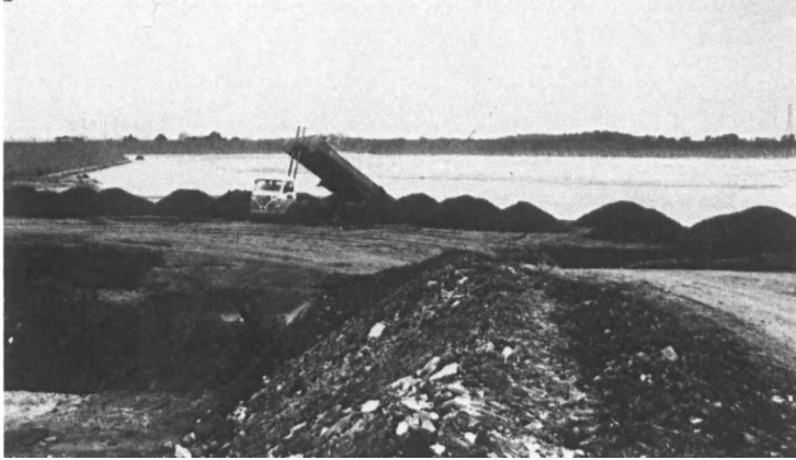
Plate 3. Minestone used to form PFA Lagoons, Gale Common, Yorkshire.
