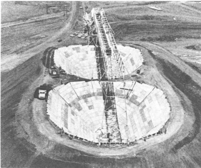
Figure 11. Aerial View of Bunkers (Note reinforcing strips in inner lateritic layer).
