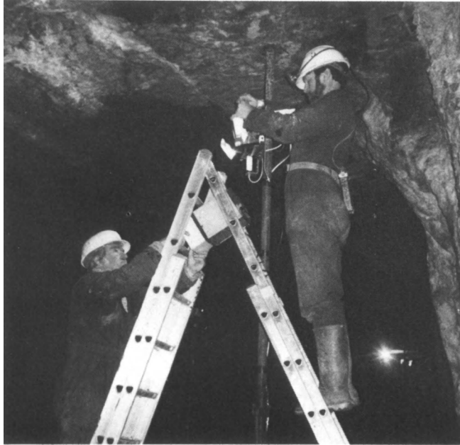
Fig. 6 - Installing closed circuit television system in Castle Fields Mine
