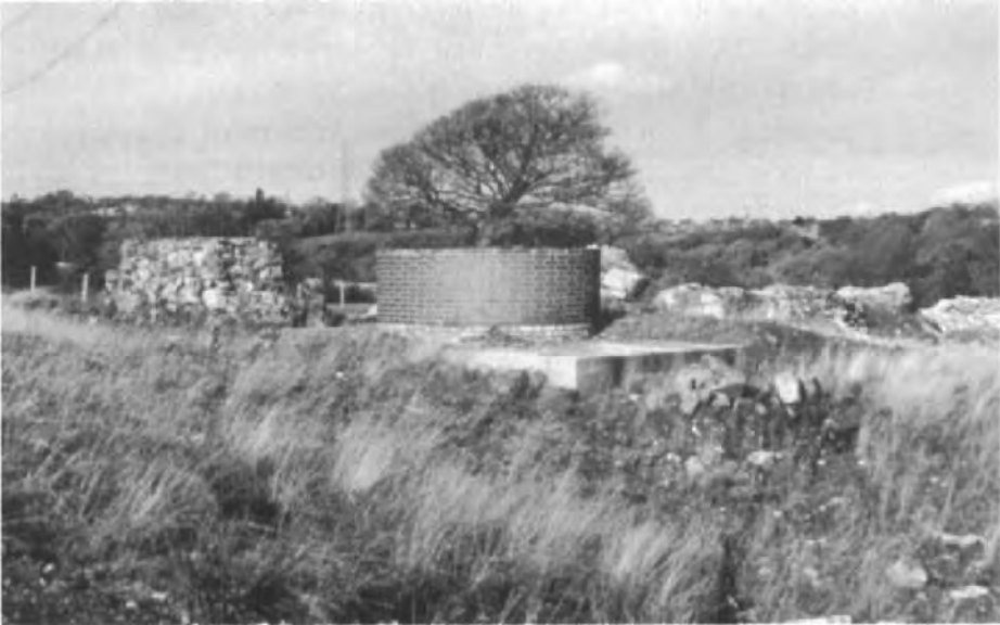
Photograph 15.4: This raised brick cylinder will indicate the location and size of a capped and buried shaft once the surrounding land is regraded (source: Richards, Moorehead and Laing Ltd)
