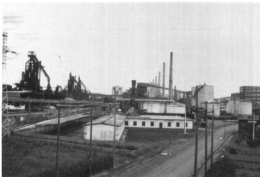
Photograph 4.1: A steelworks site in Asturias, Spain (source: Richards, Moorehead and Laing Ltd)
