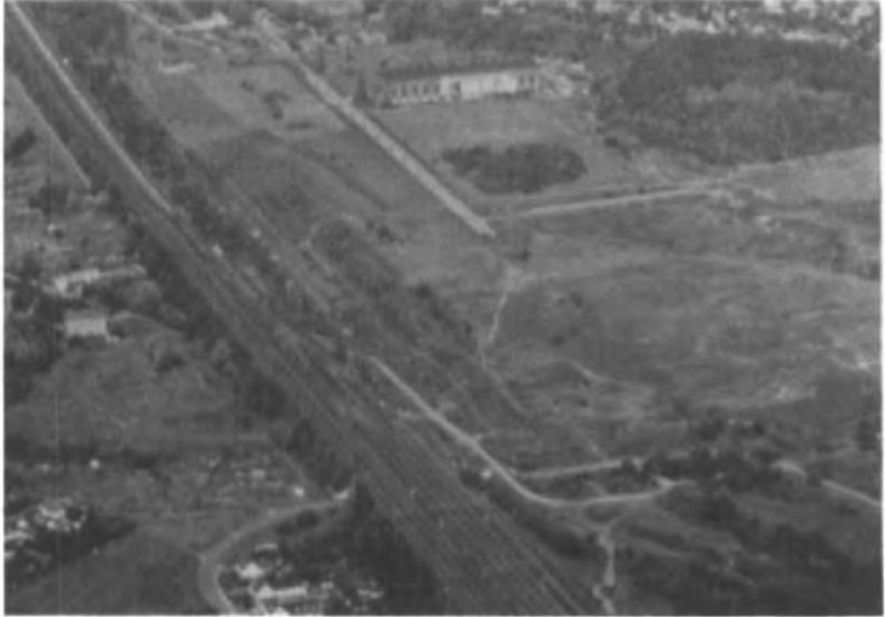
Photograph 17.15: Aerial view of Sachsen mine, Hamm. The large building is the machine hall, the only building on the site which has not been demolished (source: AHU)
