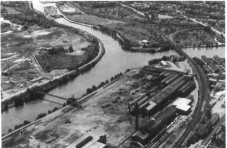
Photograph 13.4: Steelworks typically require a large area of level or terraced land, because of their size, and a good supply of water. This steelworks is already partially demolished (source: Richards, Moorehead and Laing Ltd)
