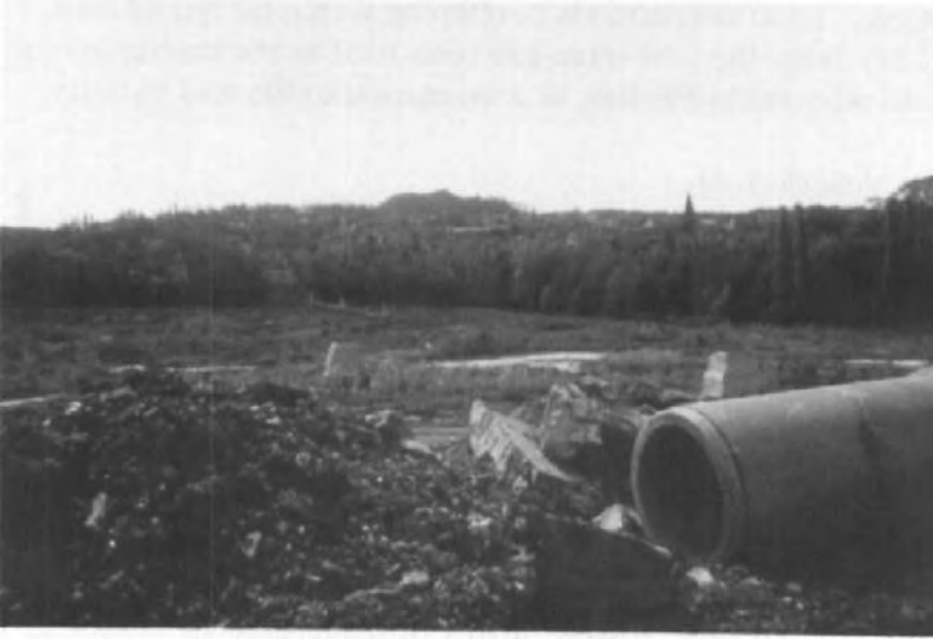
Photograph 17.12: The Aciérie LD site part way through reclamation. The drainage system is being installed (source: Richards, Moorehead and Laing Ltd)
