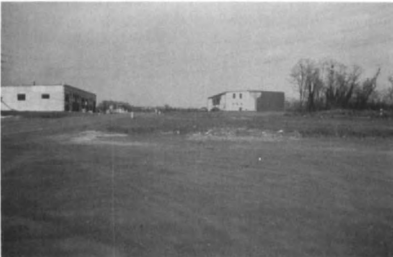
Photograph 17.11: New industrial units at Colard (source: Richards, Moorehead and Laing Ltd)
