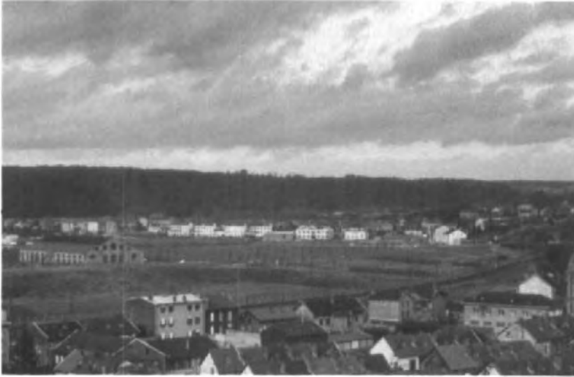
Photograph 17.7: Homécourt. View of the steelworks site after reclamation works and initial landscape works (source: Richards, Moorehead and Laing Ltd)
