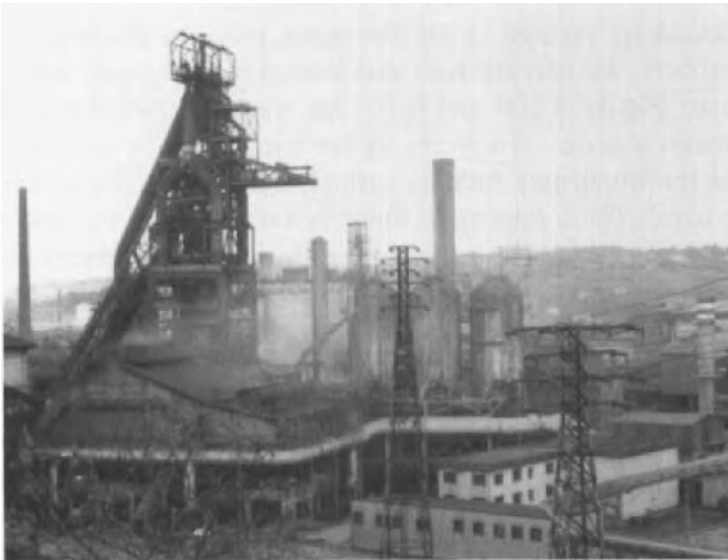
Photograph 9.1: Blast furnaces in Spain (source: Richards, Moorehead and Laing Ltd)
