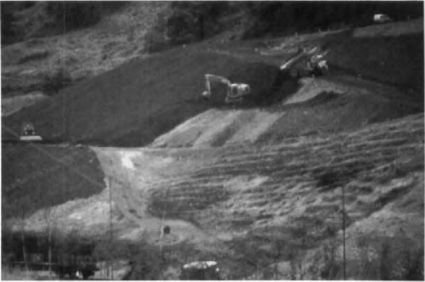
Photograph 14.6: Placing colliery spoil over slag as a growing medium for trees and grass (source: Welsh Development Agency)
