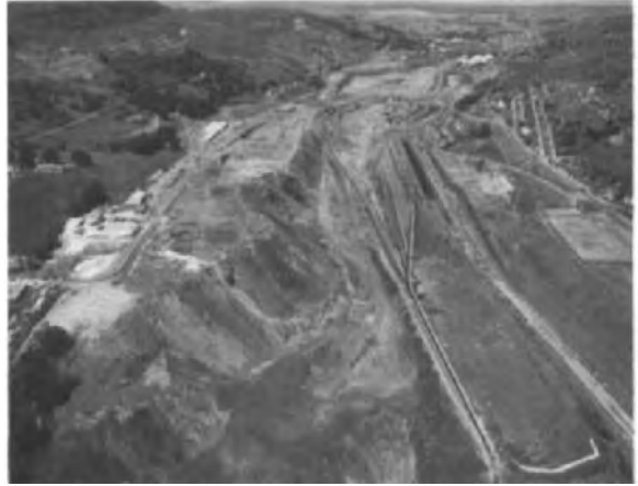
Photograph 13.1: Former steelworks and colliery, Ebbw Vale, South Wales. The large tips to the left of centre comprise slags, whilst to the right of centre is colliery spoil. The river running along this valley was culverted to provide extra tipping space. This site was reclaimed and used for the 1992 Garden Festival, Wales, UK (source: Welsh Development Agency)
