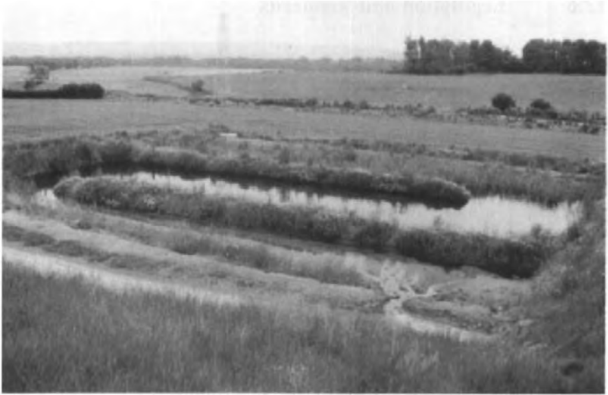
Photograph 12.1: The wetland treatment area at Gilmerton Bing, Lothian, UK. Water draining the colliery spoil enters the lagoon in the foreground from the anoxic limestone drains. Phragmites australis can be seen in the third lagoon of the system (source: Landscape Development).
