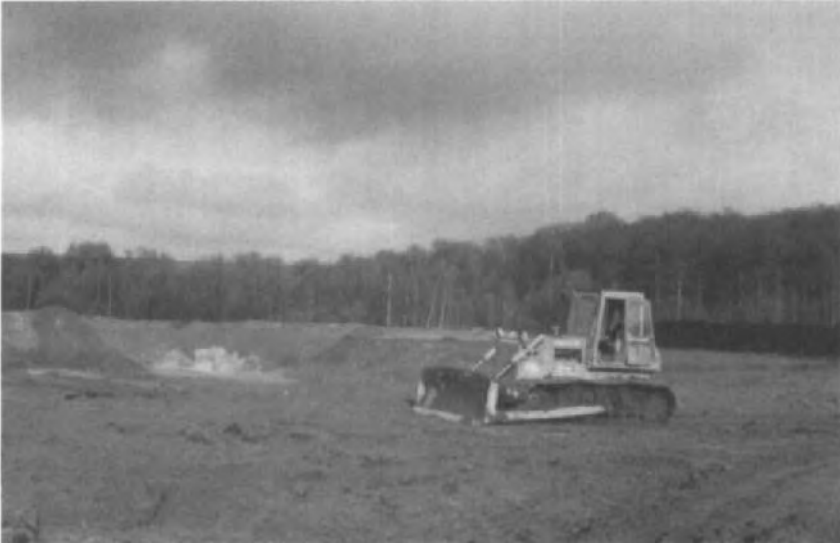
Photograph 17.4: Falquemont. Upper lagoon being filled with ash from the power station (source: Richards, Moorehead and Laing Ltd)
