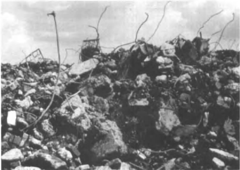
Photograph 5.2: Demolition waste deposited in a colliery spoil heap in South Yorkshire, UK (source: Richards, Moorehead and Laing Ltd)
