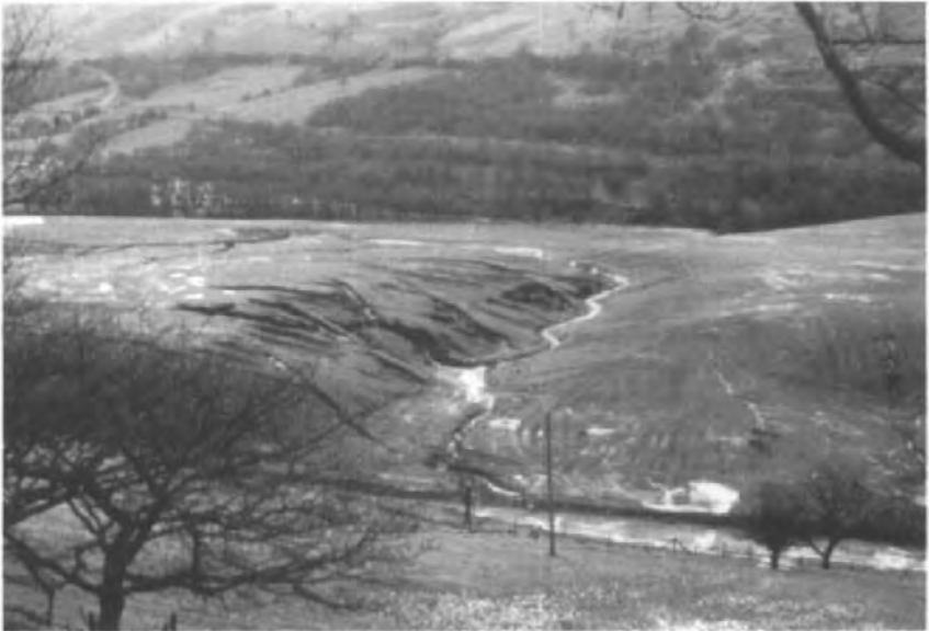
Photograph 5.3: Erosion of washery waste in a poorly designed reclamation scheme (source: Richards, Moorehead and Laing Ltd)
