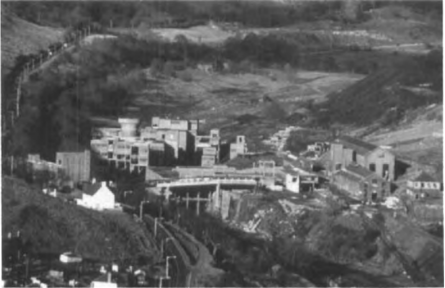
Photograph 4.2: View of an abandoned colliery site in South Wales, UK (source: Richards, Moorehead and Laing Ltd)
