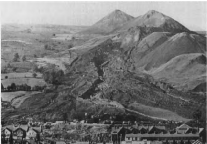
Photograph 1.1: The Aberfan disaster: colliery spoil from tips on the hillside has swept away houses and the local school. In this photograph the operation to clear away the spoil has begun (source: Report of the tribunal appointed to inquire into the disaster at Aberfan on October 21 1966 5 )
