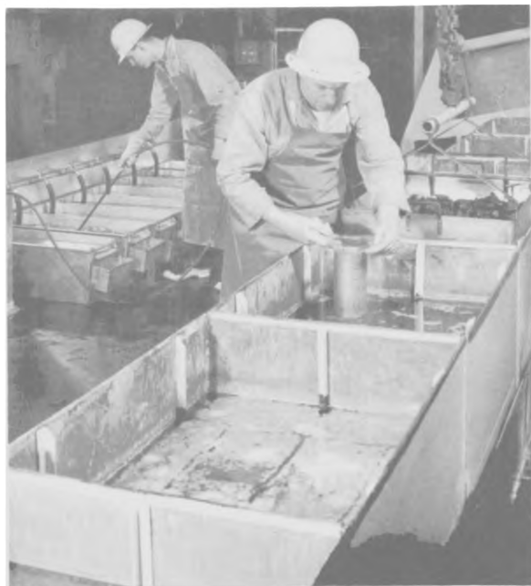
FIGURE 16.—Coarse Coal Testing Apparatus Using Salt Solution.
