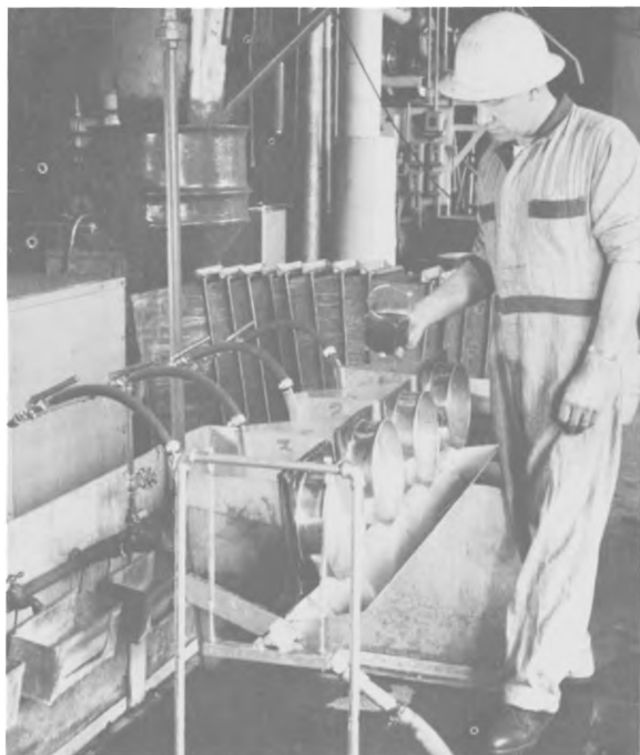
FIGURE 20.—Fine Coal Washing Devices.
