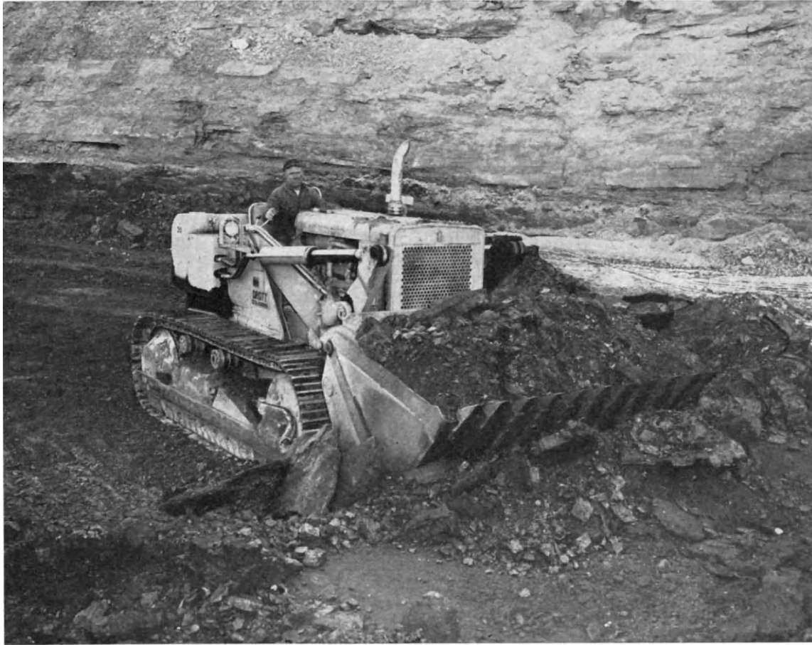
FIG. 17A. Bulldozer with bucket cleaning bottom. (International Harvester Co.)
