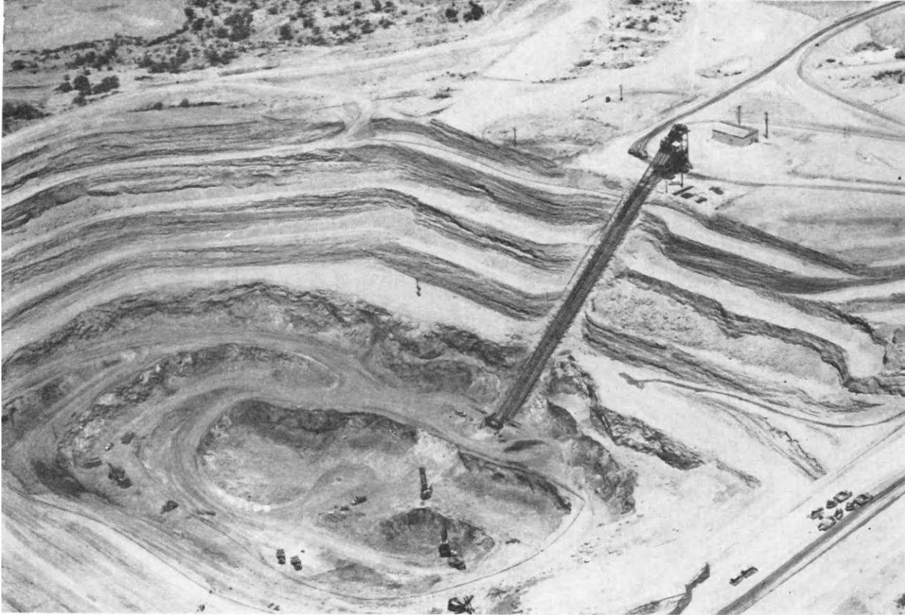
FIG. 21. Skip haulage installation at a copper pit. (National Iron Co.)
