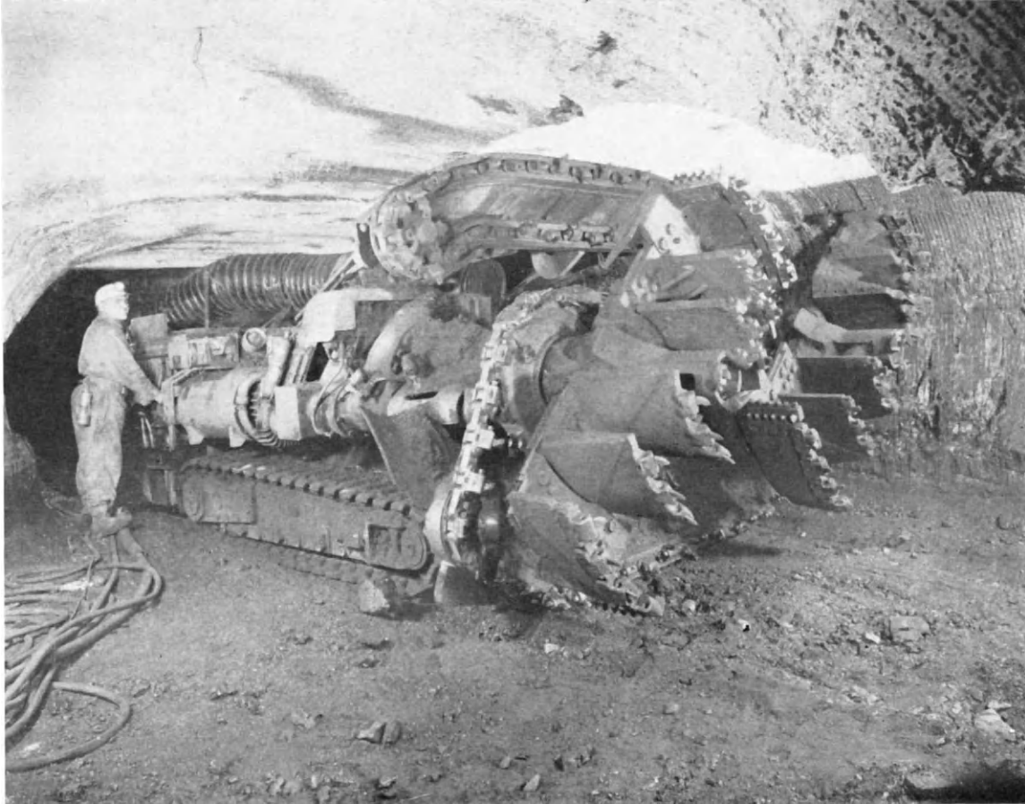
FIG. 7. Joy twin borer continuous miner. (Joy Mfg. Company.)
