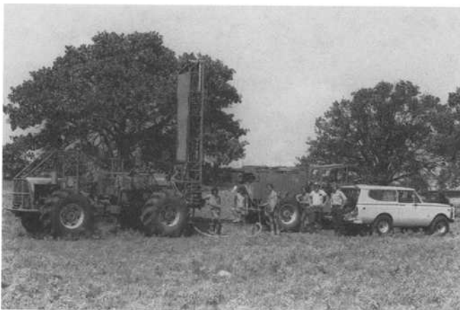
FIG. 4—Buggy-mounted rotary drill rig.
