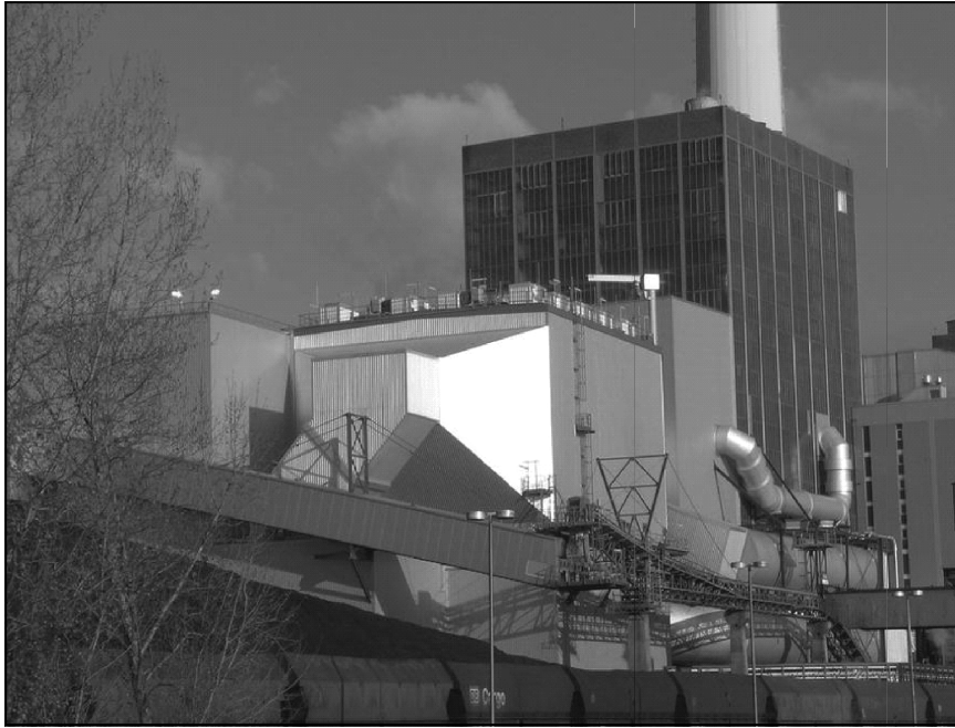
9.4 Hot electrostatic precipitator of Matsushima coal field power station (EPDC).
