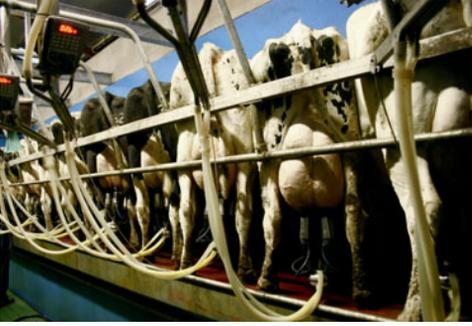
**Plate 5.10b.** High line system, where the milk has to be 'lifted' above the udder.
