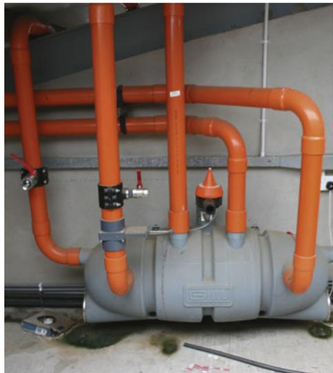
**Plate 5.3.** The regulator should always be fitted to the balance tank if one is present in the system.
