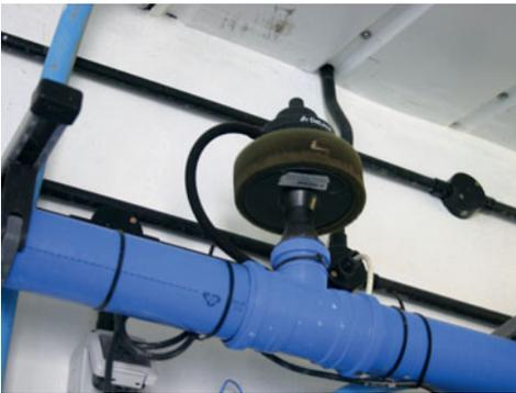
**Plate 5.4.** The regulator should always be sited in a clean dust-free environment.
