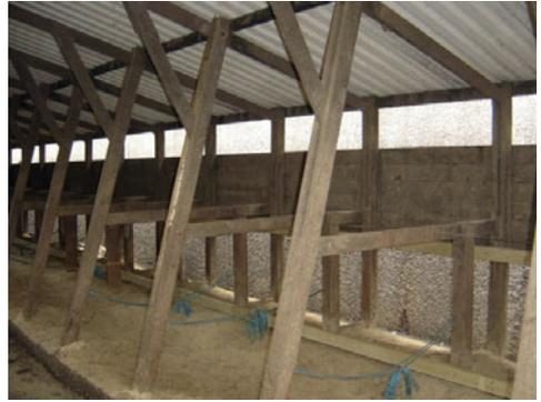
**Plate 8.11.** As this wooden cubicle house was close to an adjacent building, removal of most of the front not only improved cow comfort but also improved air flow and overall ventilation.
