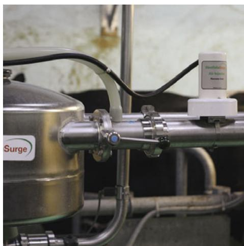
**Plate 5.21.** Air injectors are fitted to the milk transfer line to maximize agitation of wash solutions to ensure that large-volume lines are cleaned.
