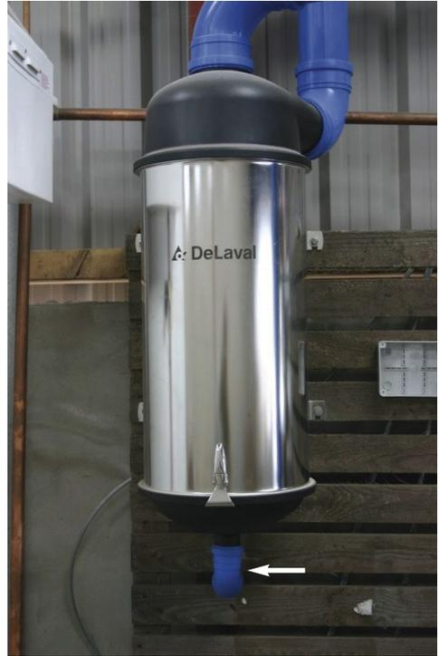
**Plate 5.2.** The interceptor vessel with drain valve at the bottom.
