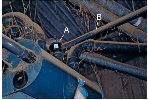
**Plate 5.5.** Regulators fitted with a clean air system are surrounded by a case (A). A pipe (B) feeds air from the external environment through the regulator and into the milking system. Although the surrounding area is dirty the system should prevent this dirt from entering the pipelines.
