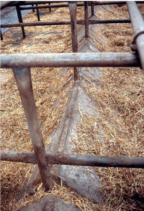
**Plate 8.13.** A concrete pyramid 0.38 m high between two facing rows of cubicles was once used to prevent cows going too far forward. It is no longer popular.
