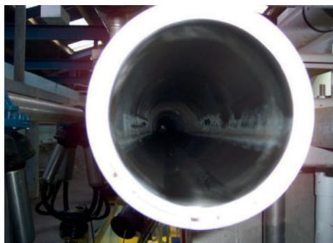
**Plate 10.6.** Soil can be seen half way up the milk transfer line, caused by lack of turbulence during the wash cycle.
