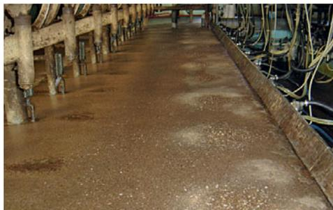
**Plate 8.27.** The cement surface of this parlour floor has been eroded by a barrier teat dip, exposing a white aggregate. This makes detection of mastitis in the foremilk more difficult.
