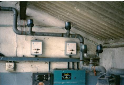
**Plate 5.35.** Multiple weight-controlled regulators.
