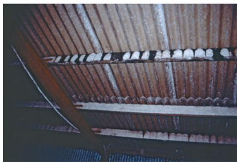
**Plate 8.10.** Condensation dripping from the roof joists is considered to be a sign of poor ventilation.
