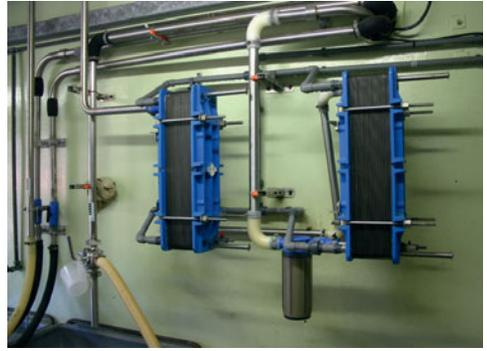
**Plate 10.4.** Plate coolers drop the temperature of milk quickly and slow down bacterial multiplication, while saving energy.
