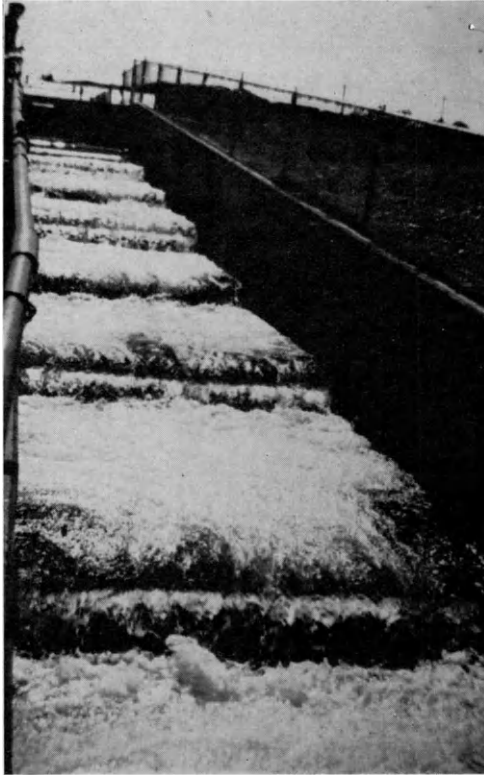
FIG. 66. A fish ladder to allow spawning salmon to go upstream past a dam.
