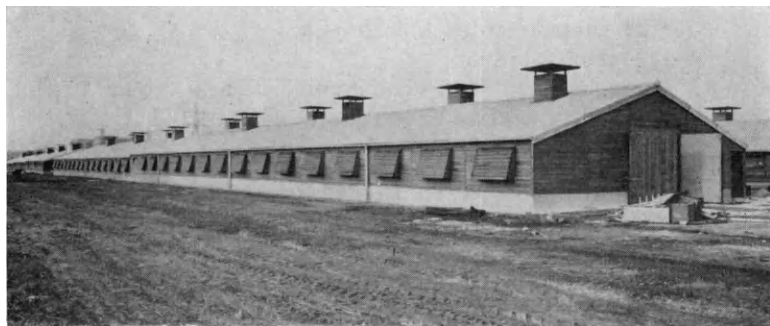
FIG. 31. It is always a good plan to site a row of intensive poultry houses end-to-end, across wind, with the object of minimising the spread of aerial contamination.
