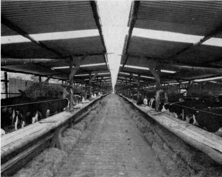
FIG. 5. Cheap buildings are essential, such as simple pole yards with a sleeper road of sufficient width to take a site delivery truck. The open ridge pole yards at Brown Street Farm are 340 yd long.
